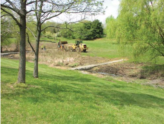
Construction of gabion walls - April 2008
