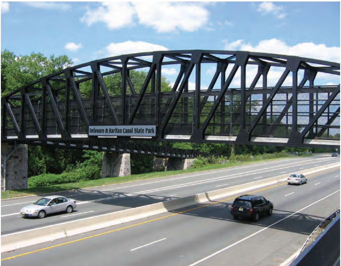
Delaware & Raritan Canal Bridge over Route 1, Lawrence Township, NJ
