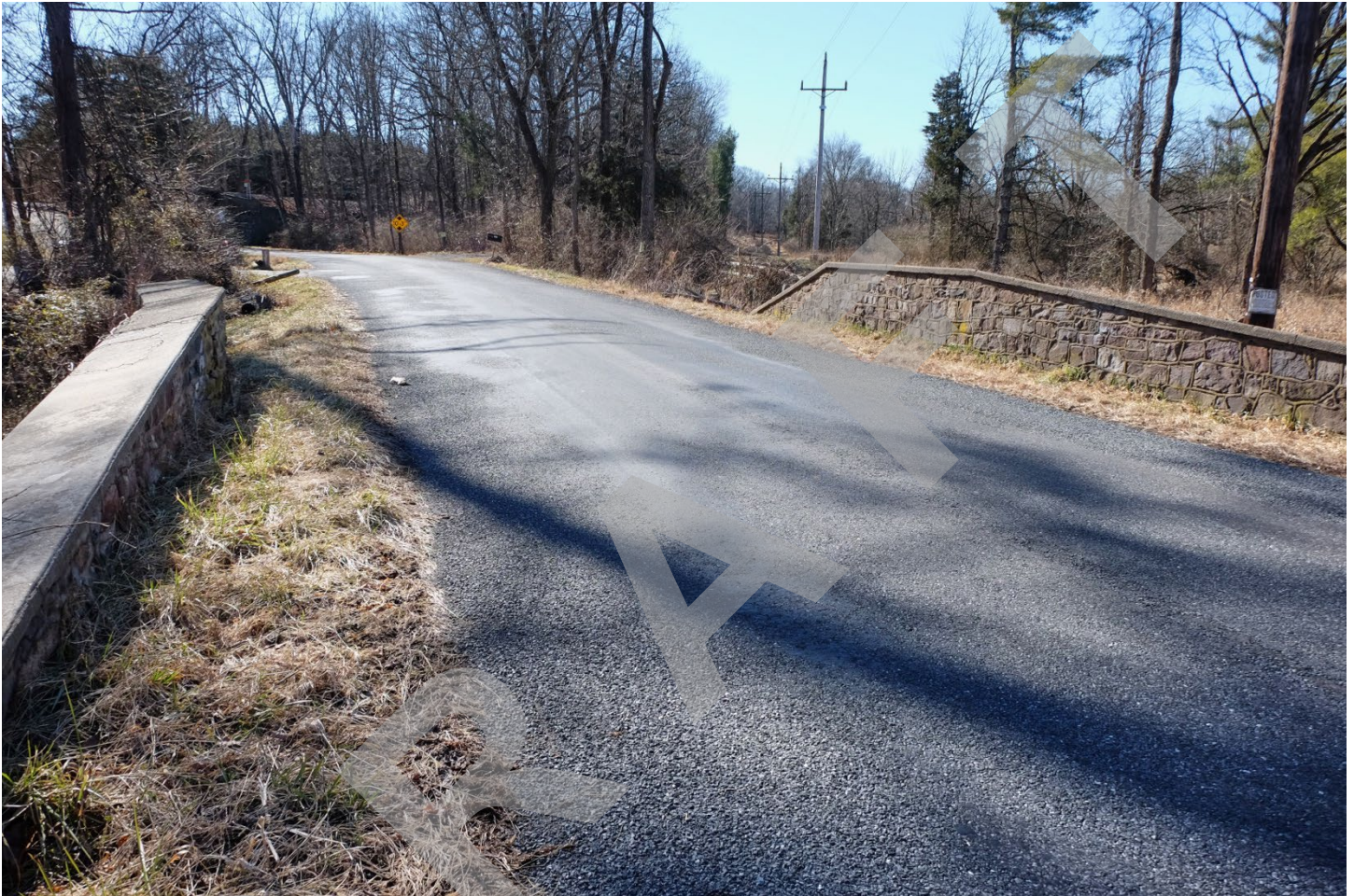
Photo 3: View facing south towards the railroad trestle.
