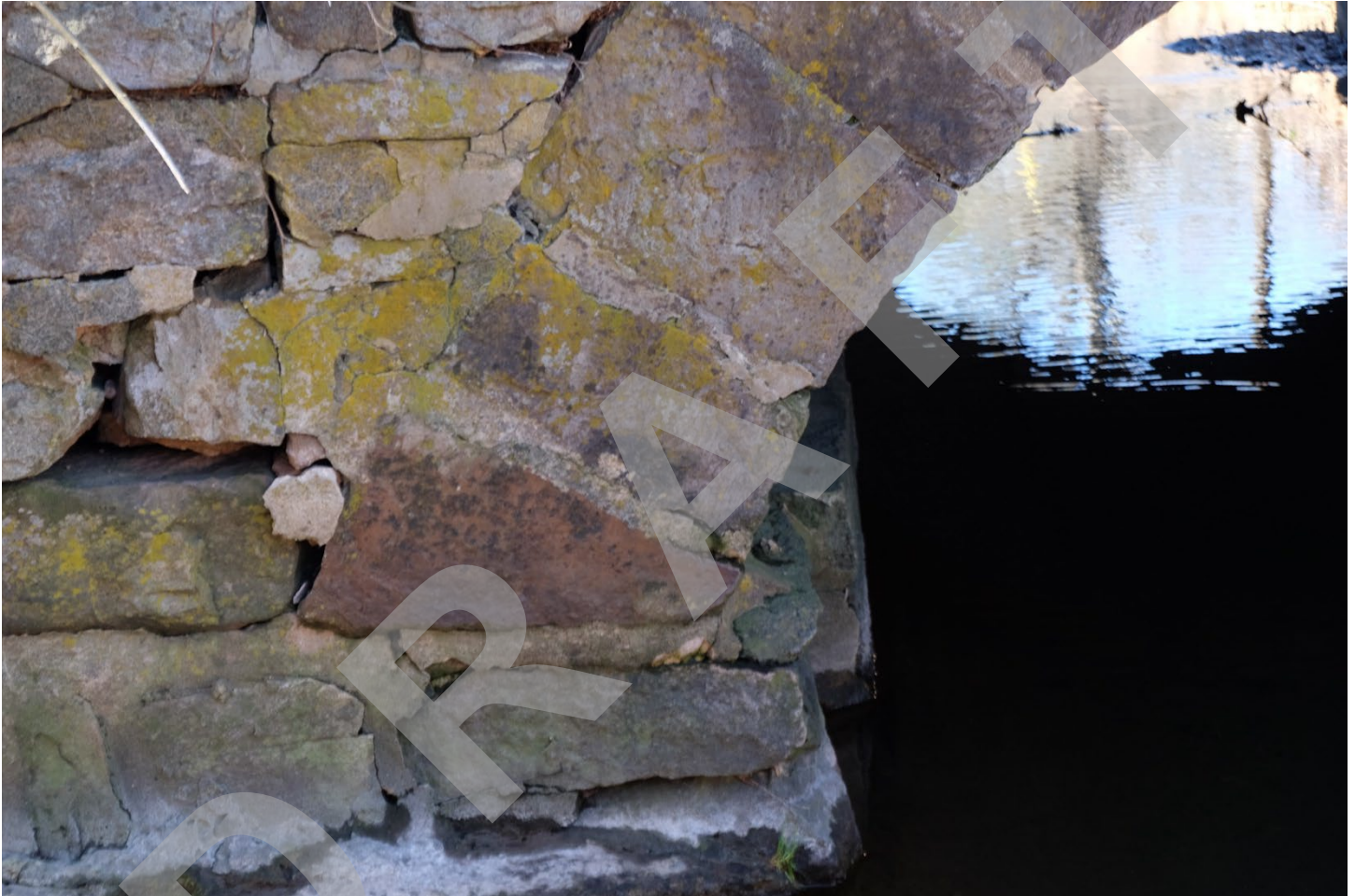
Photo 6: View facing west showing the south triangular springer
