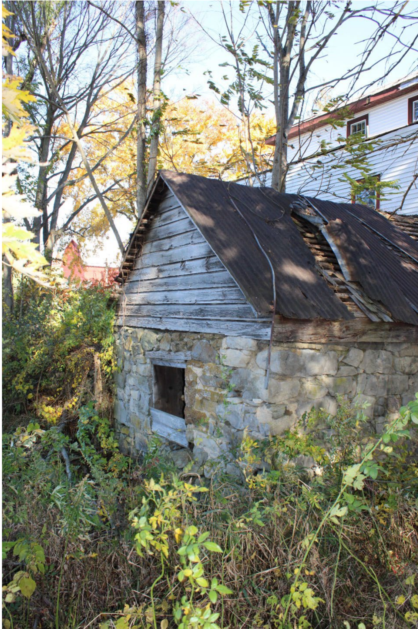
Photo 0003: View of the west side of the farmhouse showing the partial elevation of the main house and its fenestration, camera facing northeast.
