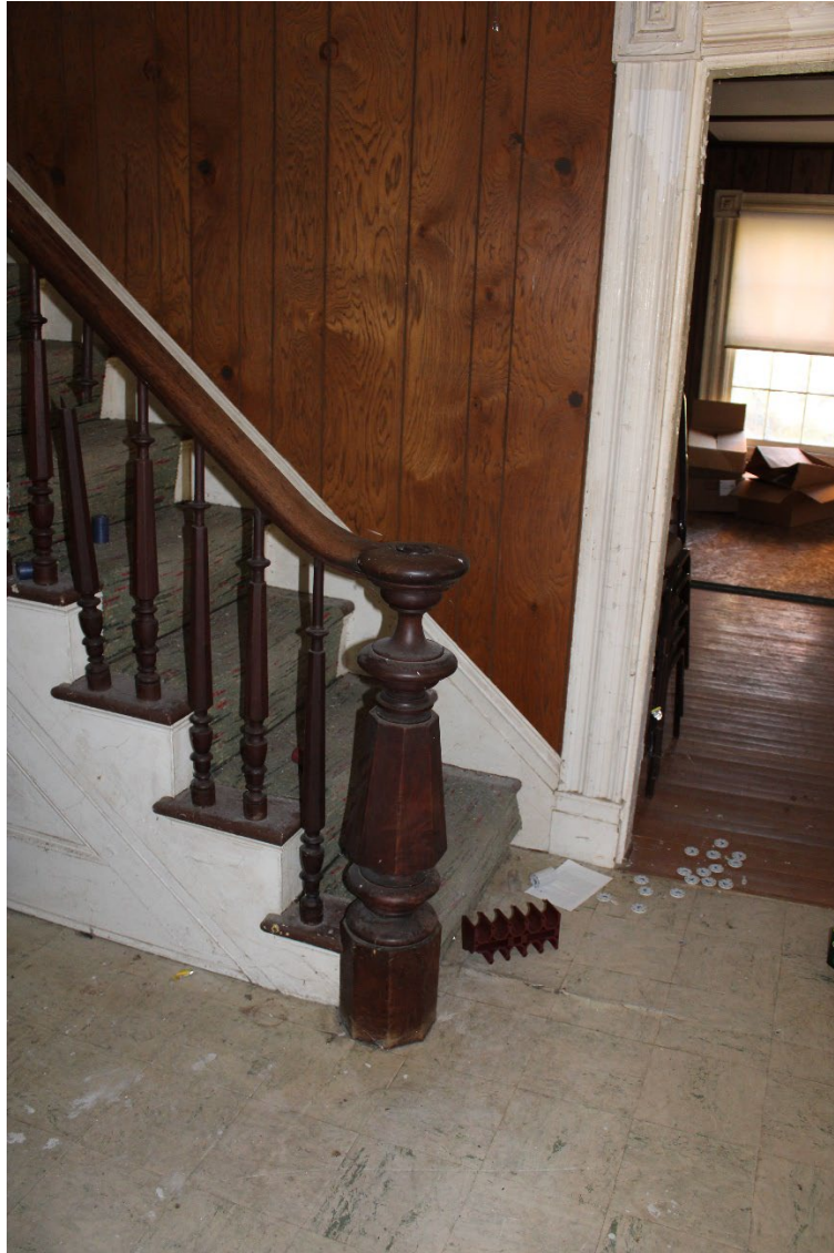
Photo 0009: Detail view of the stair including newel post and balusters beyond, camera facing north.
