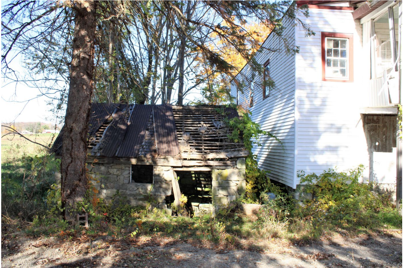
Photo 0015: View of the south elevation of the spring house, camera facing northeast.
