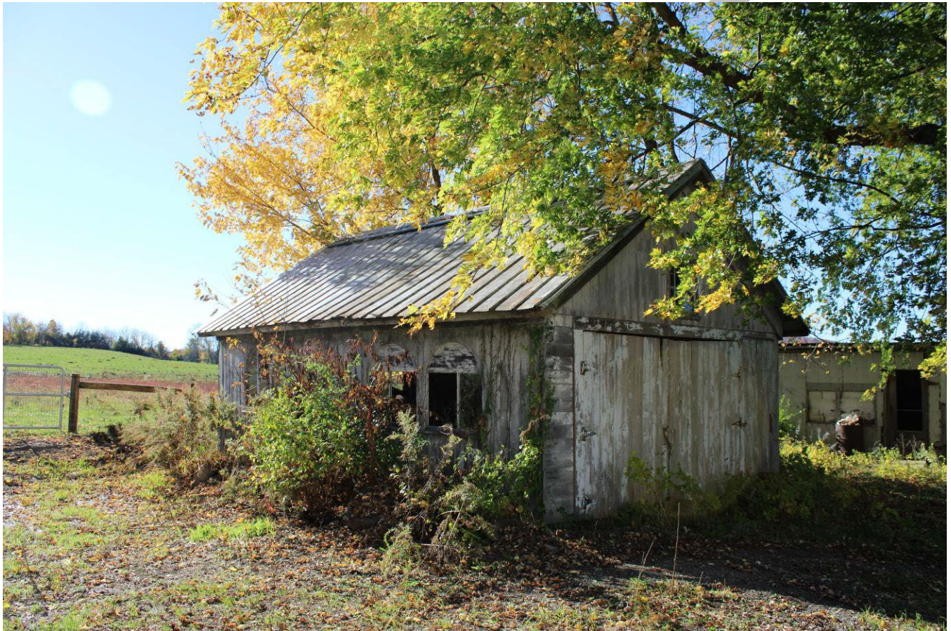
Photo 0018: View of the north and east elevations of the "old" chicken house, camera facing west.
