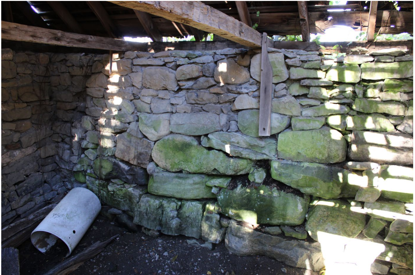
Photo 0017: View of the interior of the spring house, camera facing north.
