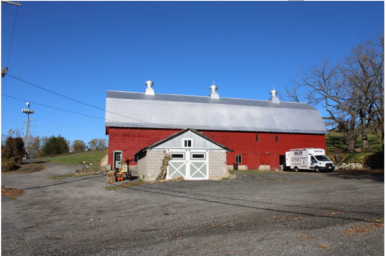
Photo 0020: View of the south elevation of the dairy barn and machine shed, camera facing northeast.
