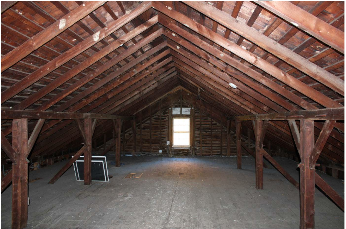
Photo 0014: View of the attic showing the exposed framing and earlier wood roof shingles, camera facing north.
