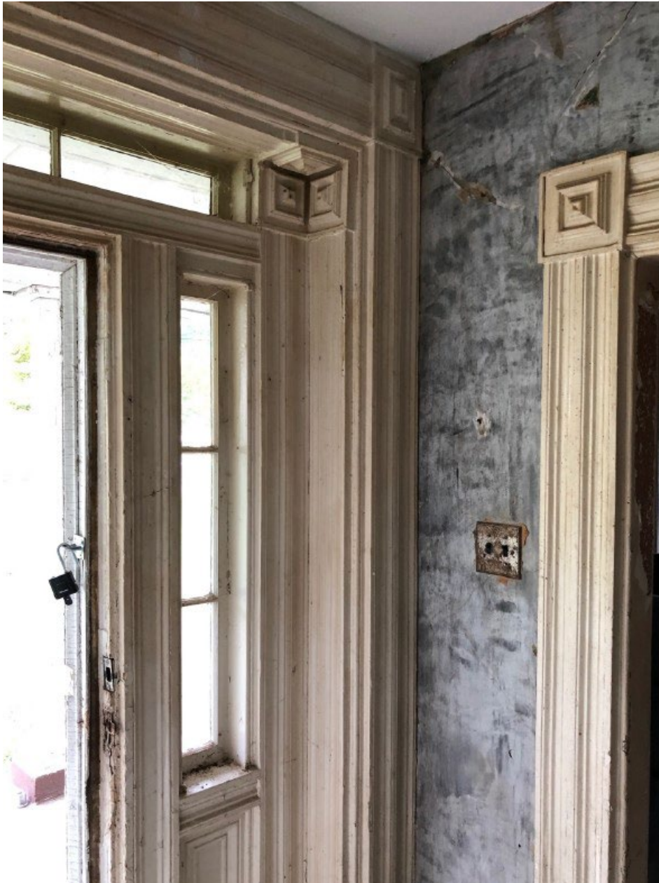
Photo 0008: Detail view of the front entrance trim and moldings, camera facing south.
