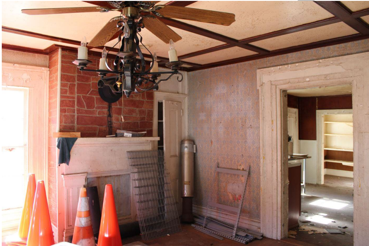
Photo 0011: View of Room 102 showing simpler eared moldings, camera facing west.
