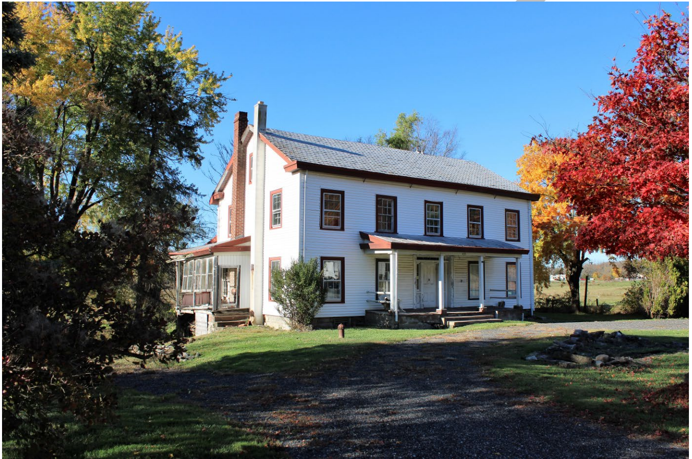
Photo 0001: View of the front (east) elevation of the farmhouse, camera facing north.
