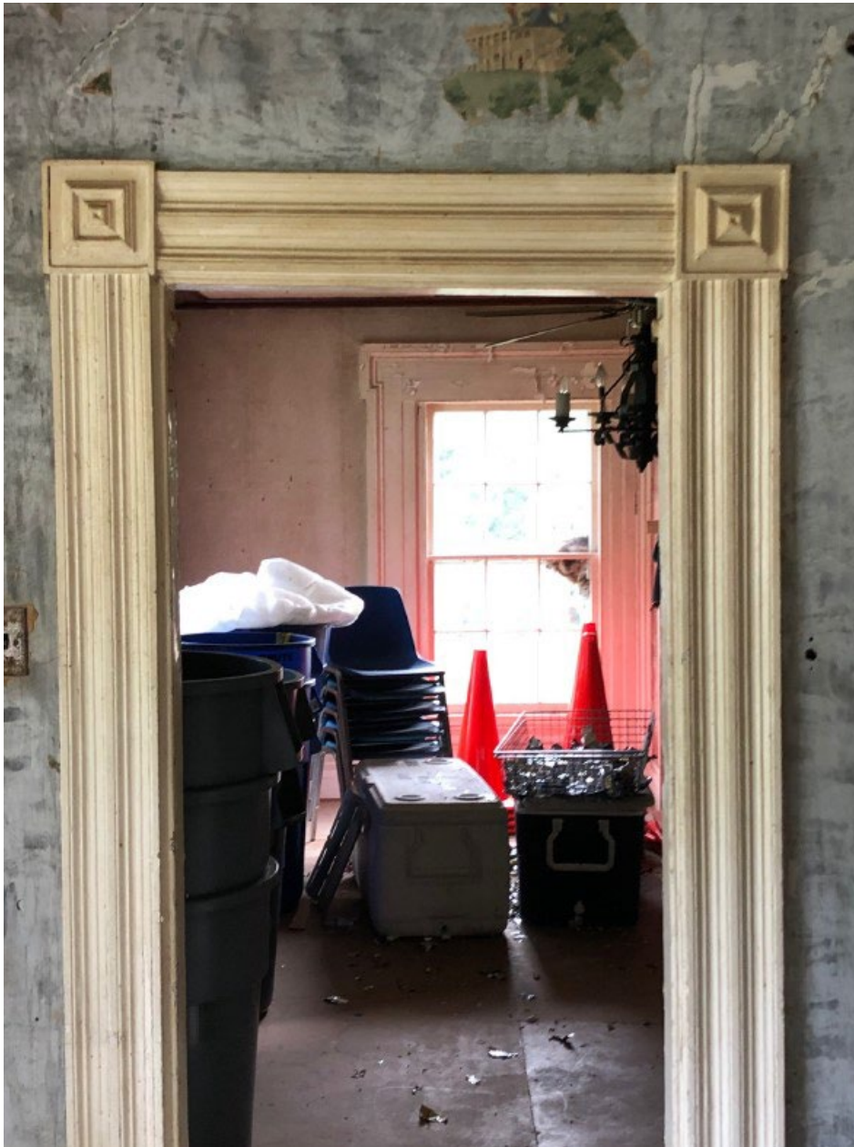
Photo 0010: View of typical fluted door molding, camera facing southwest towards Room 102.
