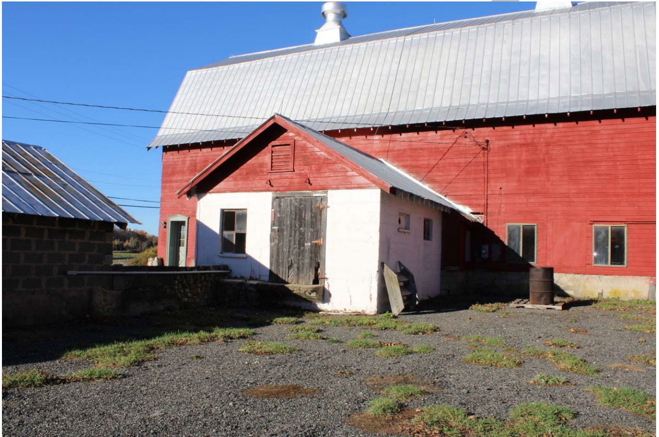
Photo 0022: View of the milk shed on the south elevation of the dairy barn, camera facing north.
