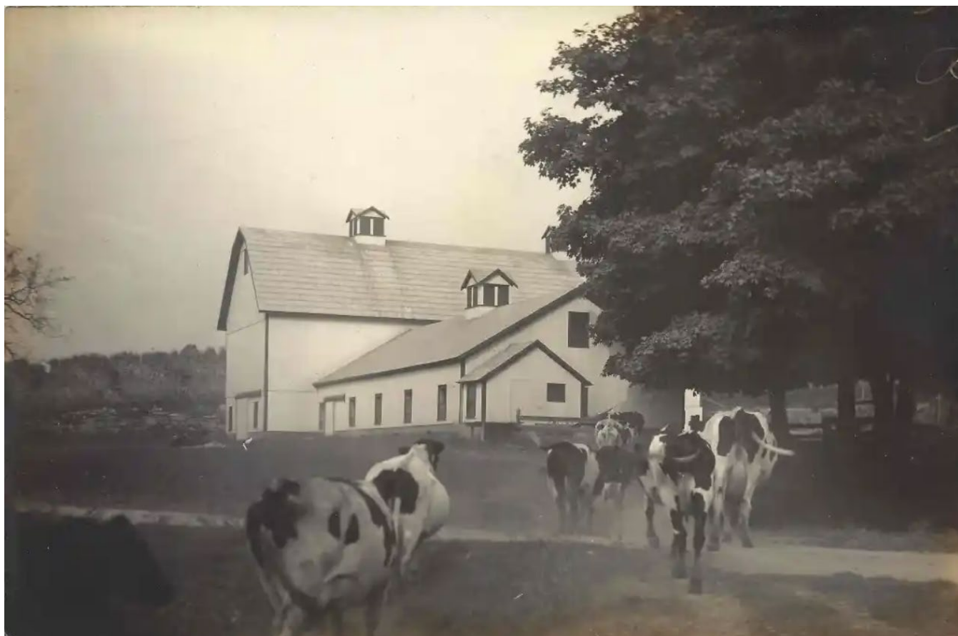
Figure 5. Circa 1912 view of the original dairy barn from the Rickey farmhouse. 4
