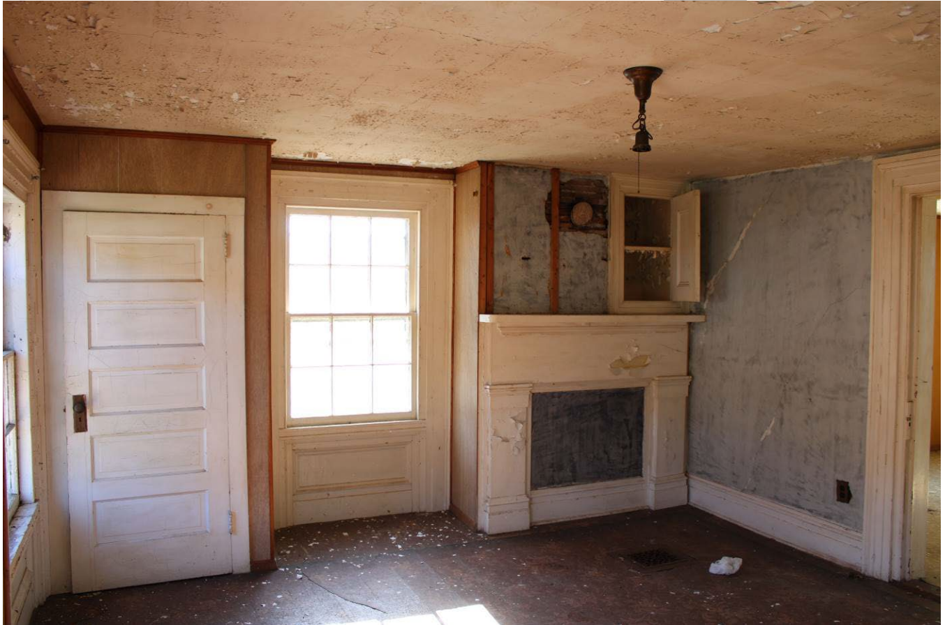
Photo 0013: View of Room 202, camera facing west.
