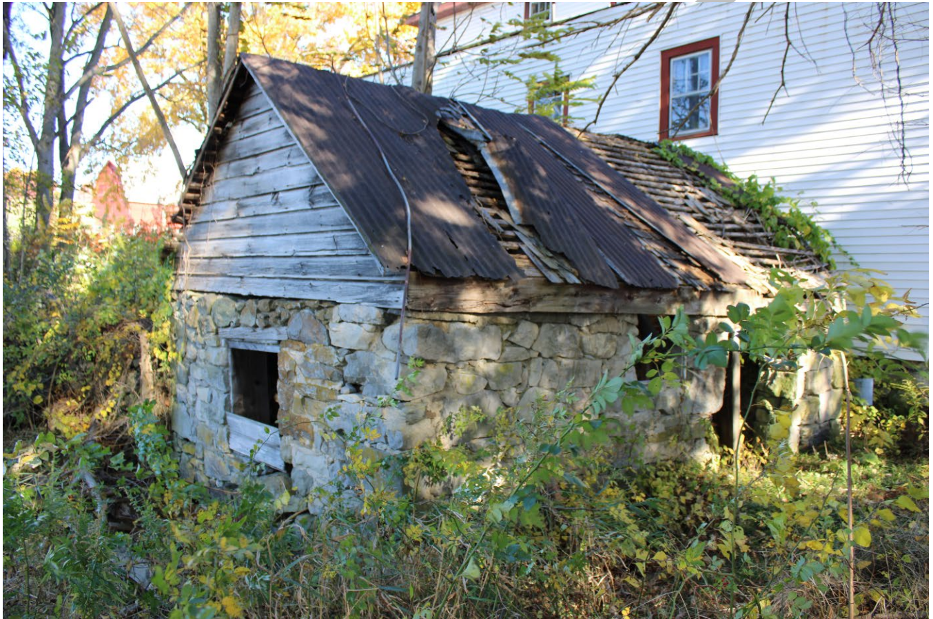
Photo 0016: View of the west and south elevations of the spring house with the west elevation of the farmhouse beyond, camera facing east.
