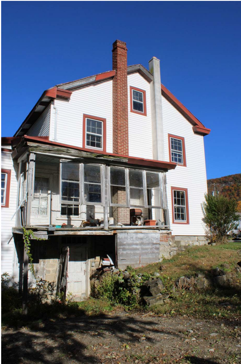
Photo 0002: View of the south elevation of the farmhouse showing the side porch, camera facing northeast.
