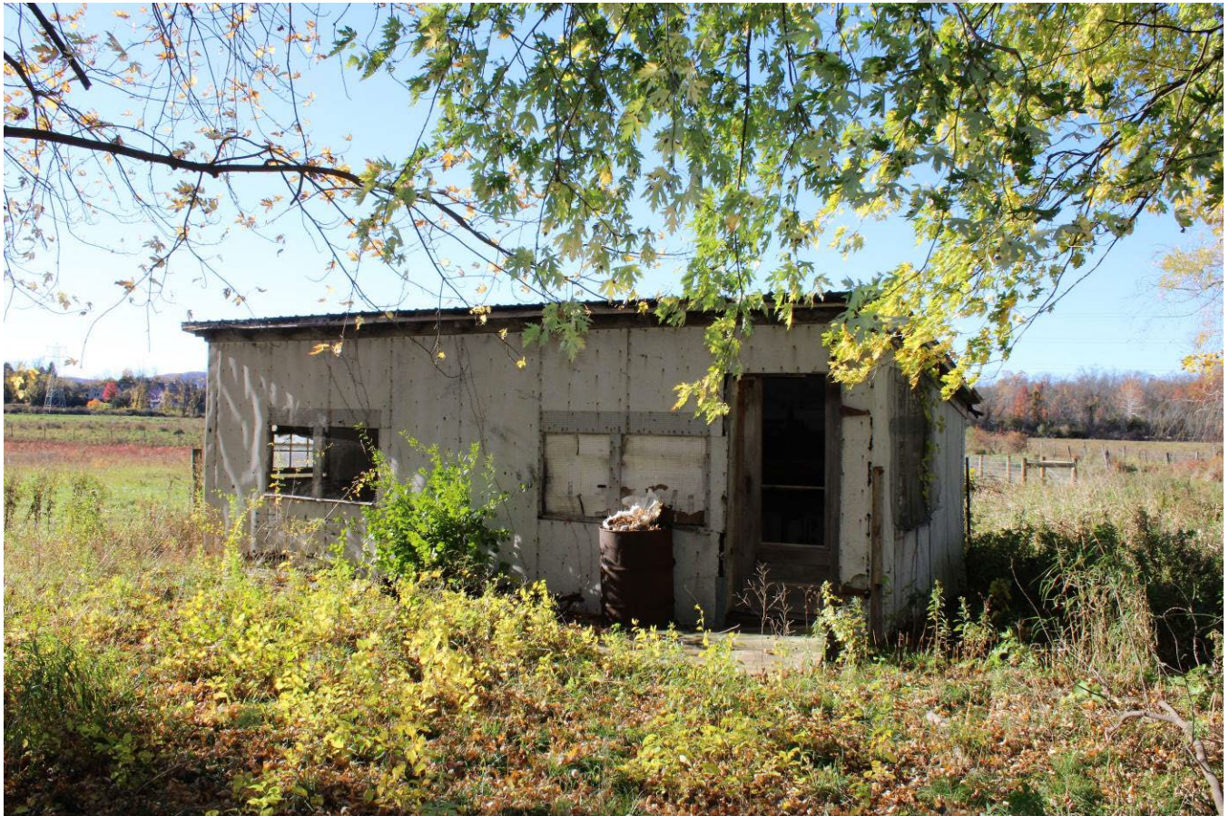
Photo 0019: View of the east elevation of the “new” chicken house, camera facing west.
