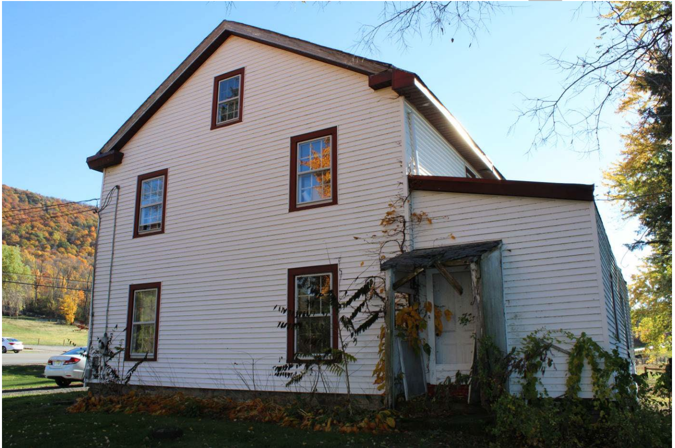
Photo 0004: View of the north elevation of the farmhouse, camera facing south.
