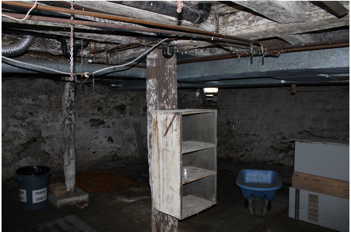
Photo 0006: Overall view of the basement within the farmhouse, camera facing northeast.
