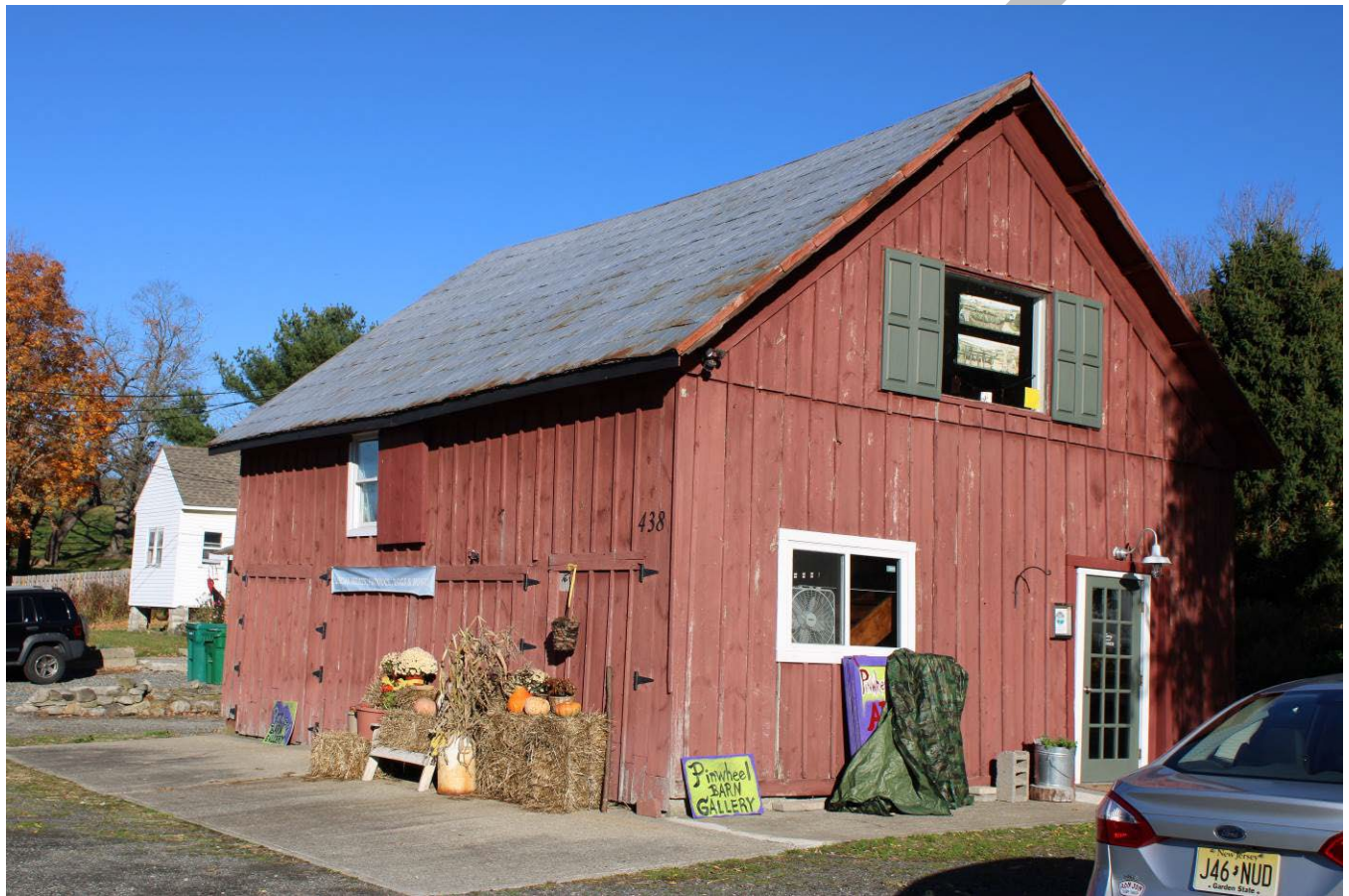
Photo 0025: View of the west and south elevations of the carriage house, camera facing northeast.
