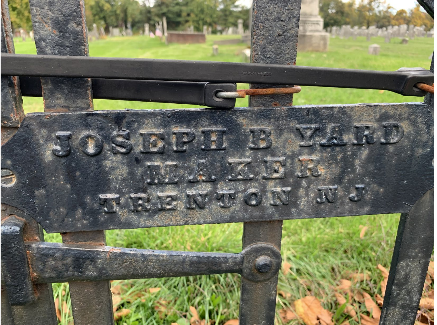
Photo #10: Exterior. Detail of historic gate, labeled by manufacturer, which is a contributing structure.
