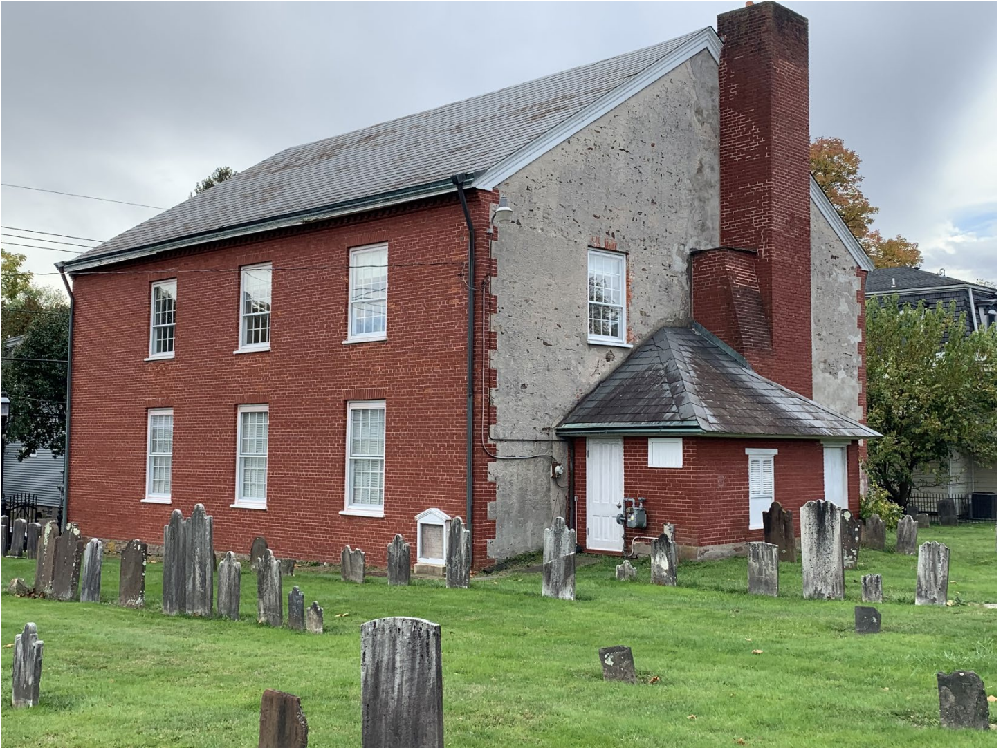
Photo #3: Exterior. Northeast corner of the Old School Baptist Church.
