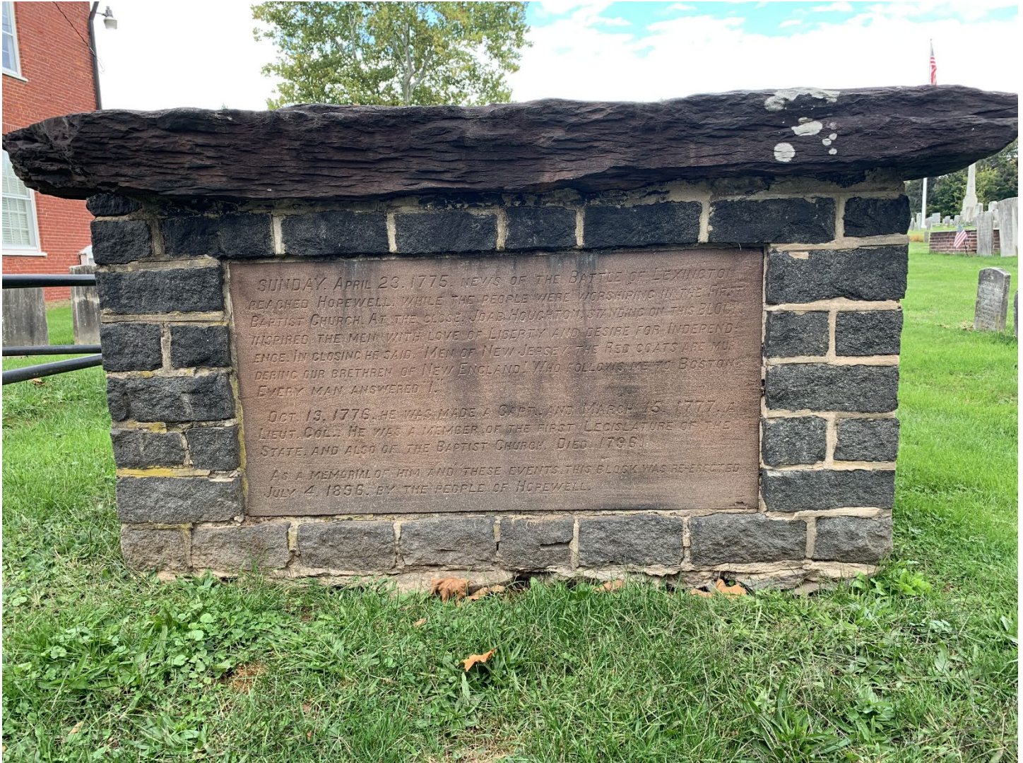
Photo #9: Exterior. Joab Houghton memorial, which is an uncounted object.
