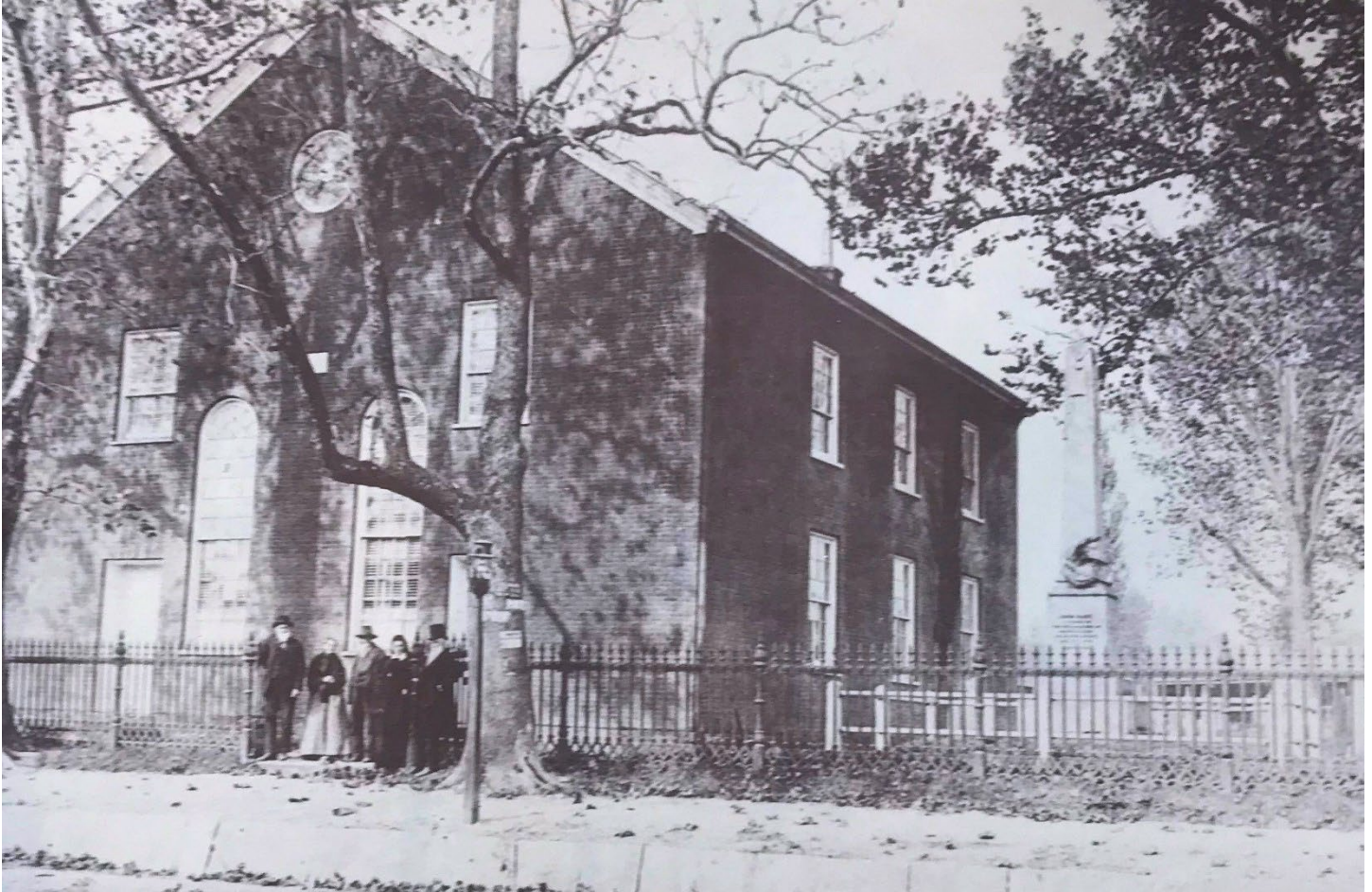
Figure 5: A photograph of the church, fence, and John Hart memorial from 1876. At this time, the fence extended across the front of the church (today it meets the corners of the church building). 5 The fence is an object of significance.
