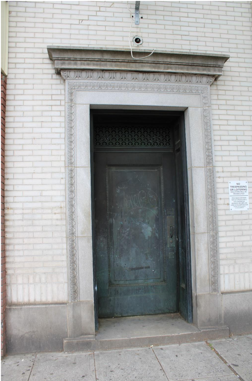
Photo 0009: Detail view of the secondary entrance at the stair tower, which retains its original bronze door and granite surround; camera facing northeast.
