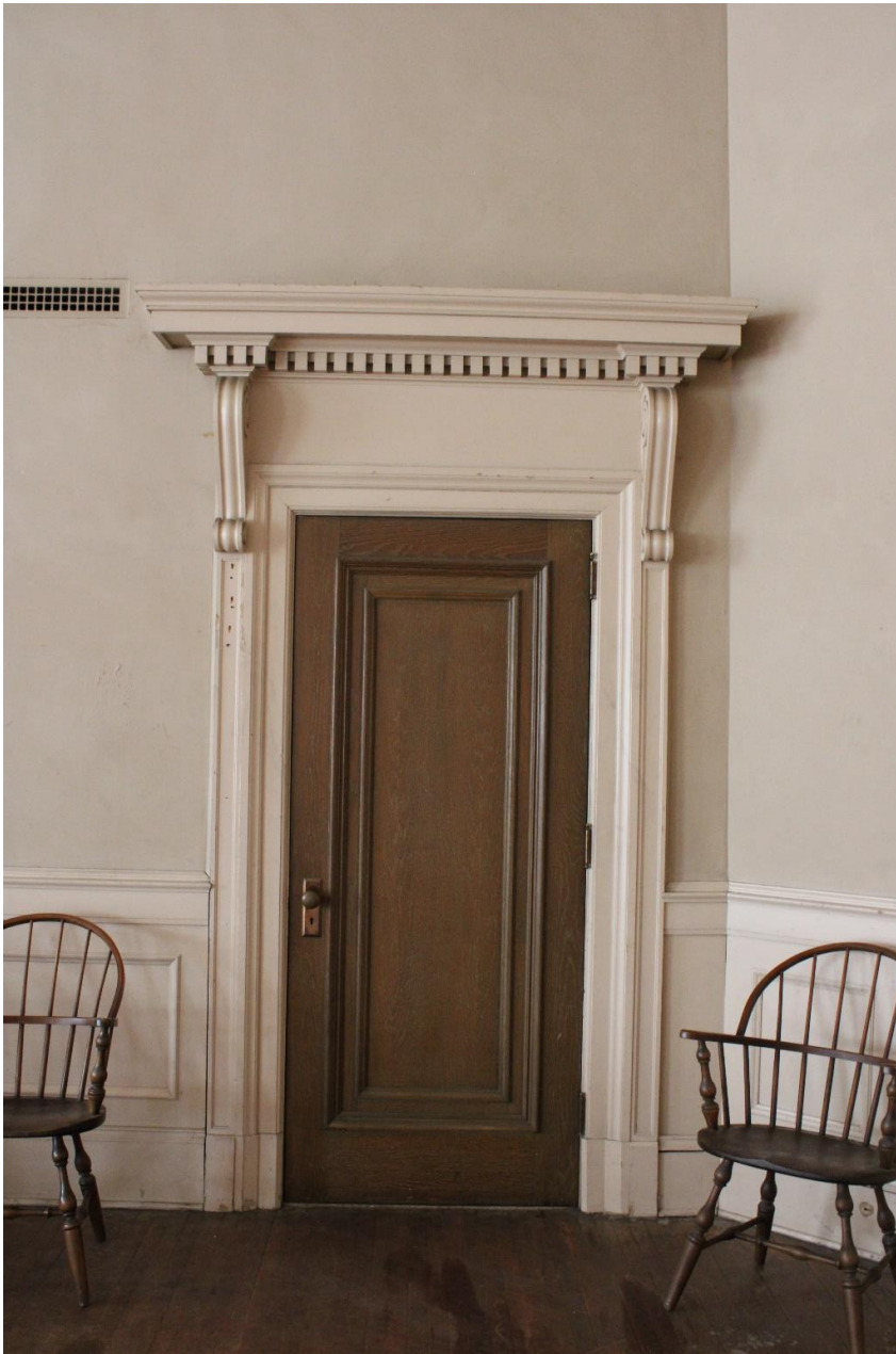
Photo 0020: Detail view of a typical paneled wood door in the assembly room with an elaborate surround.
