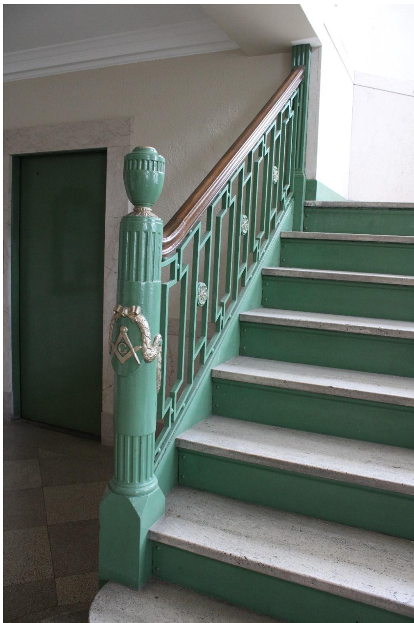
Photo 0017: Detail view of the cast iron stair at the second-floor public hall showing newel post with Freemason iconography and geometric balustrade with rosettes; camera facing north.
