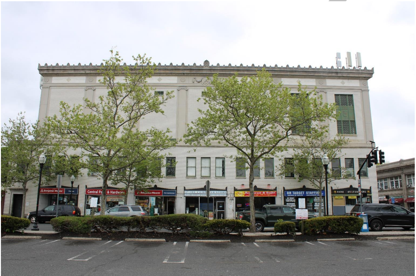
Photo 0006: Overall view of the west elevation facing Park Avenue; camera facing northeast.
