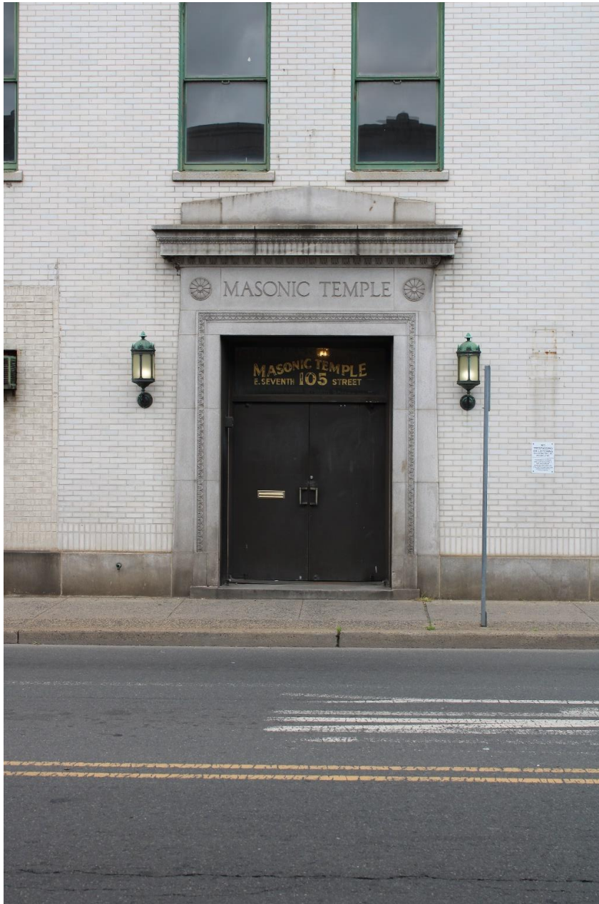
Photo 0003: Detail view of the Masonic Temple entrance on East 7 th Street; camera facing northwest.
