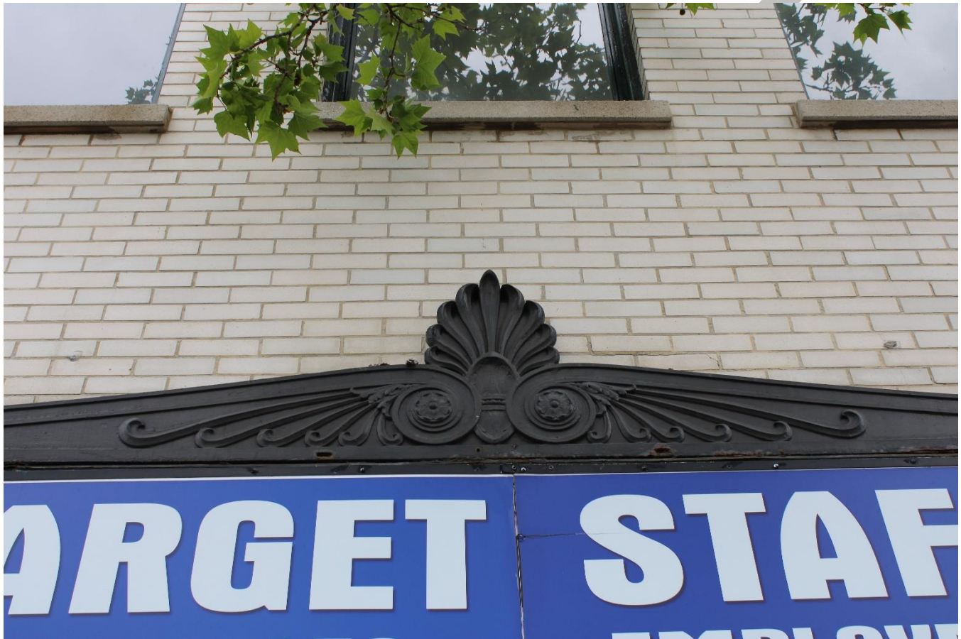
Photo 0008: Detail view of the cast iron anthemion centered atop a storefront; camera facing northeast.
