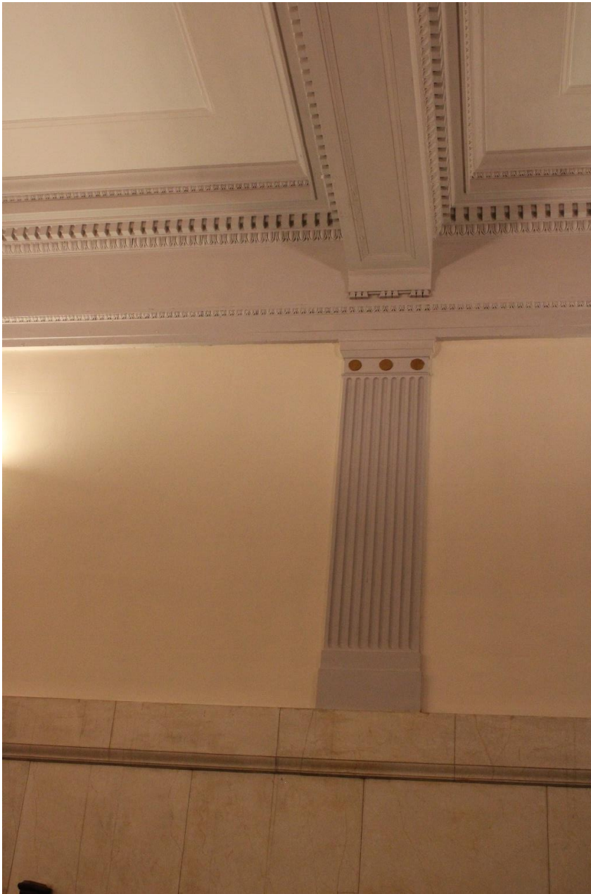
Photo 0028: View of the ornament in the Ionic Room including fluted pilaster, tall molded entablature, and matching molding at the ceiling beam; camera facing northeast.
