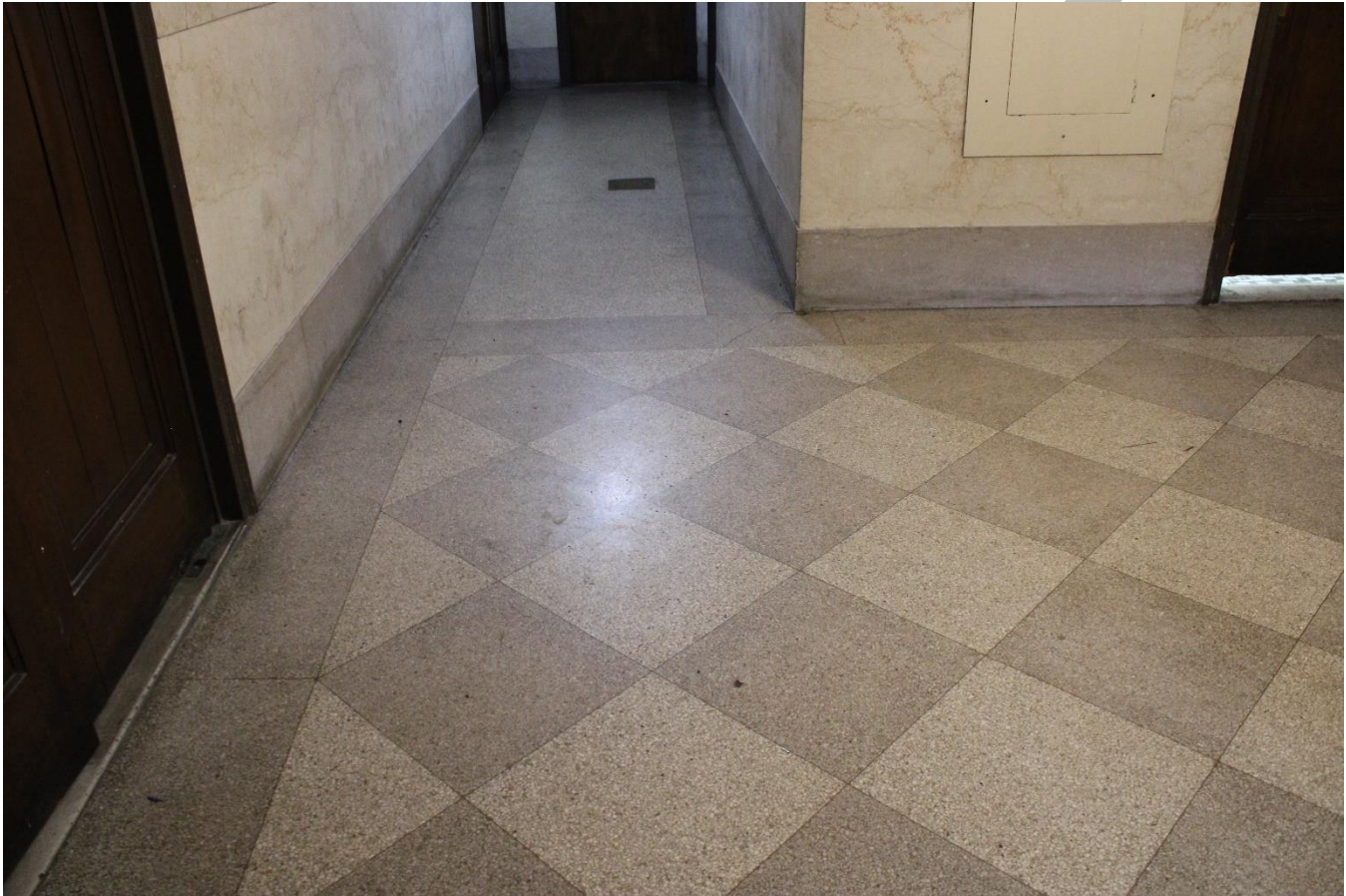
Photo 0014: View showing the terrazzo floor and marble base and wainscot in the basement-level public hall and corridor; camera facing northwest.
