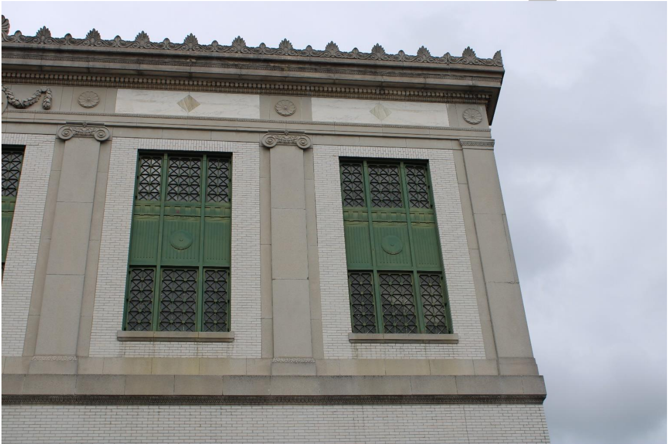
Photo 0004: Detail view of the third and fourth-floor levels showing the Ionic pilasters, steel windows with decorative bronze panel, frieze with rosettes and marble panels, and denticulated cornice, and parapet with anthemion; camera facing northwest.
