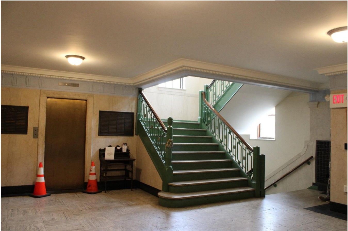
Photo 0015: Overall view of the public hall at the first floor showing the staircase and elevator, travertine flooring, marble walls, and decorative plaster cornice.
