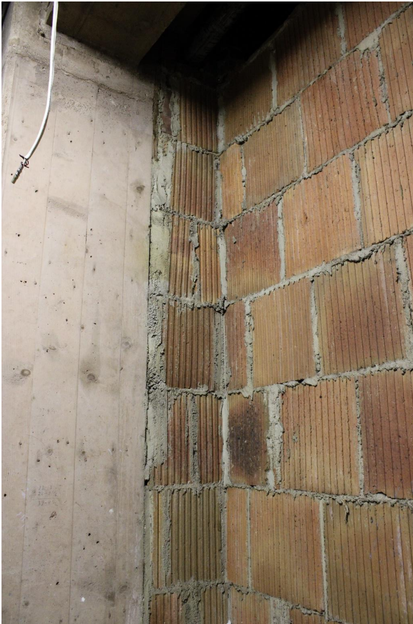
Photo 0012: Detail view showing the structural terra-cotta tile visible in the unfinished storage room in the basement; camera facing southwest.
