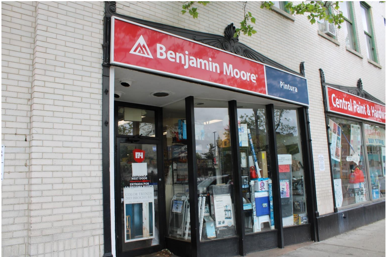
Photo 0007: View of storefronts along Park Avenue showing the original cast iron surrounds that remain; camera facing northeast.
