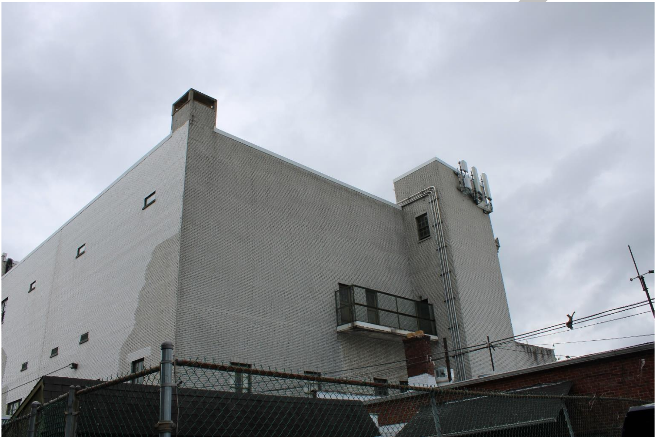
Photo 0010: Overall (partial) view of the north elevation; camera facing southeast.
