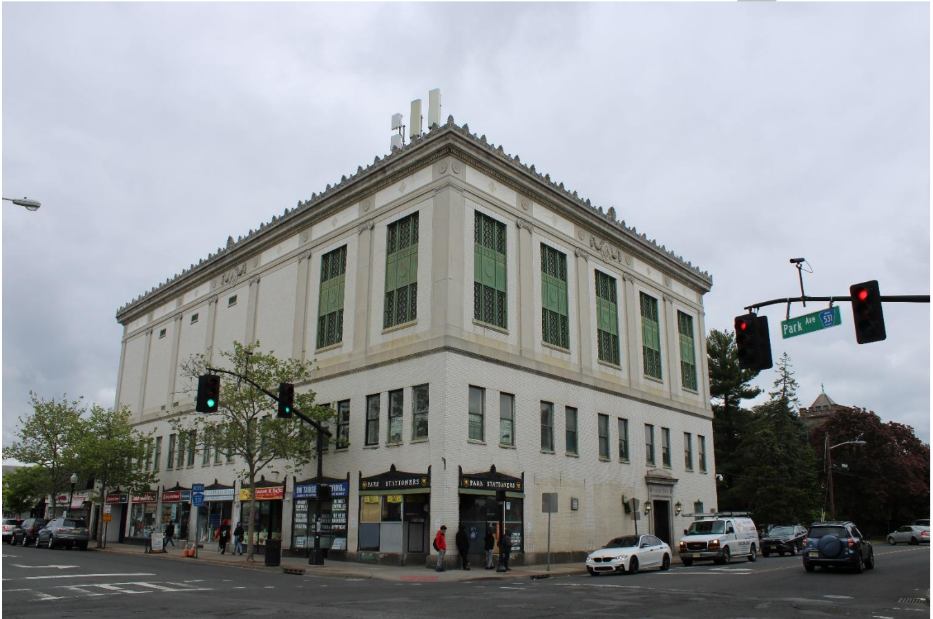
Photo 0001: Overall view of the Plainfield Masonic Temple showing both the East 7 th Street and Park Avenue elevations; camera facing north.
