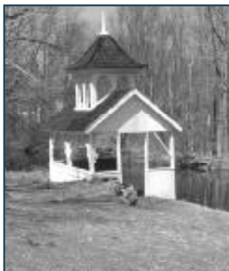
Outbuilding, Saddle River, Bergen County.
