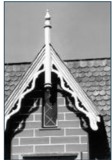
Gable Detail, The Hermitage, Ho Ho Kus Borough, Bergen County.
