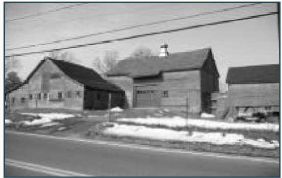
Barn Complex, Park Ridge Borough, Bergen County.
