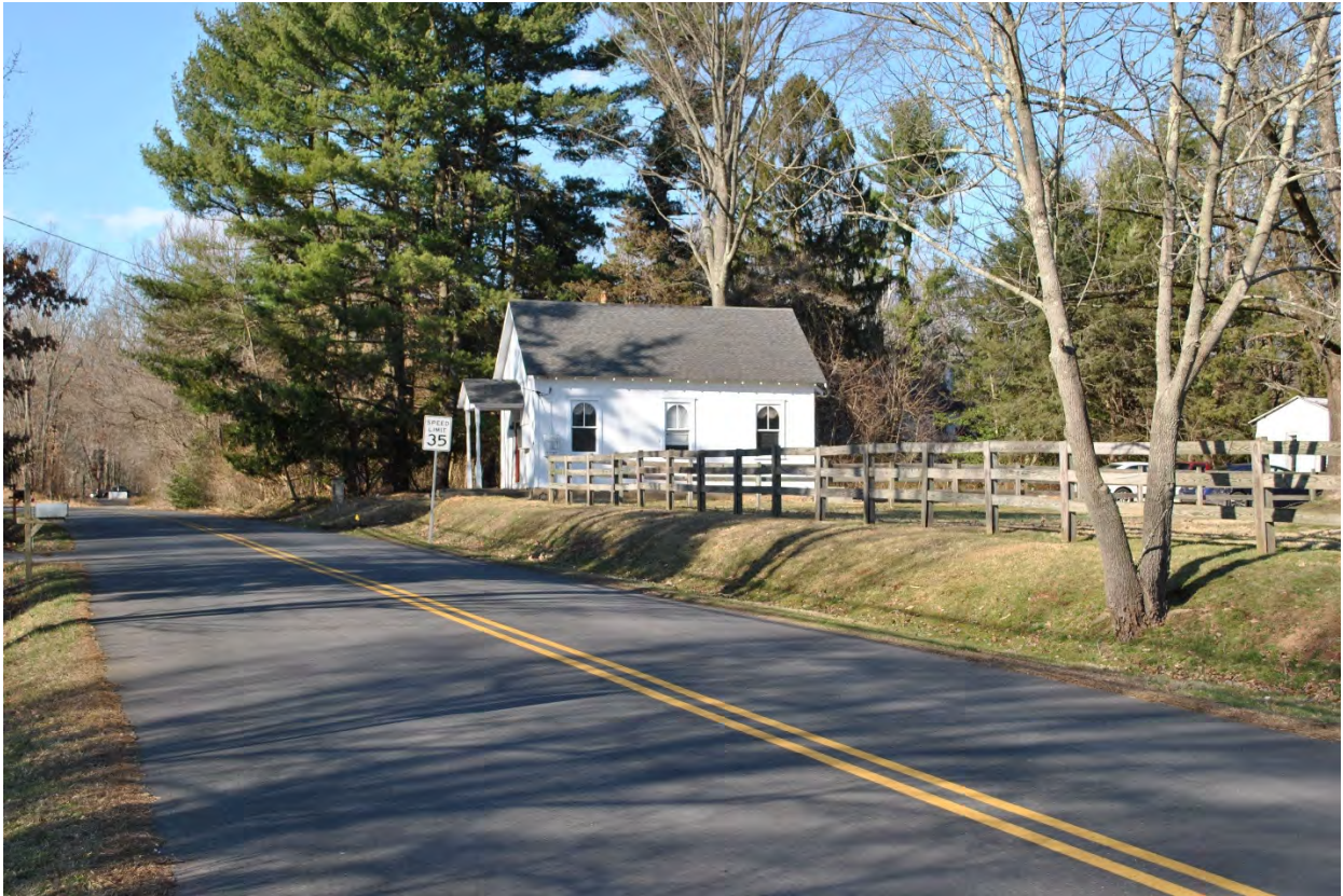
Mount Zion African Methodist Episcopal Church, Somerset County, NJ Photo 1
