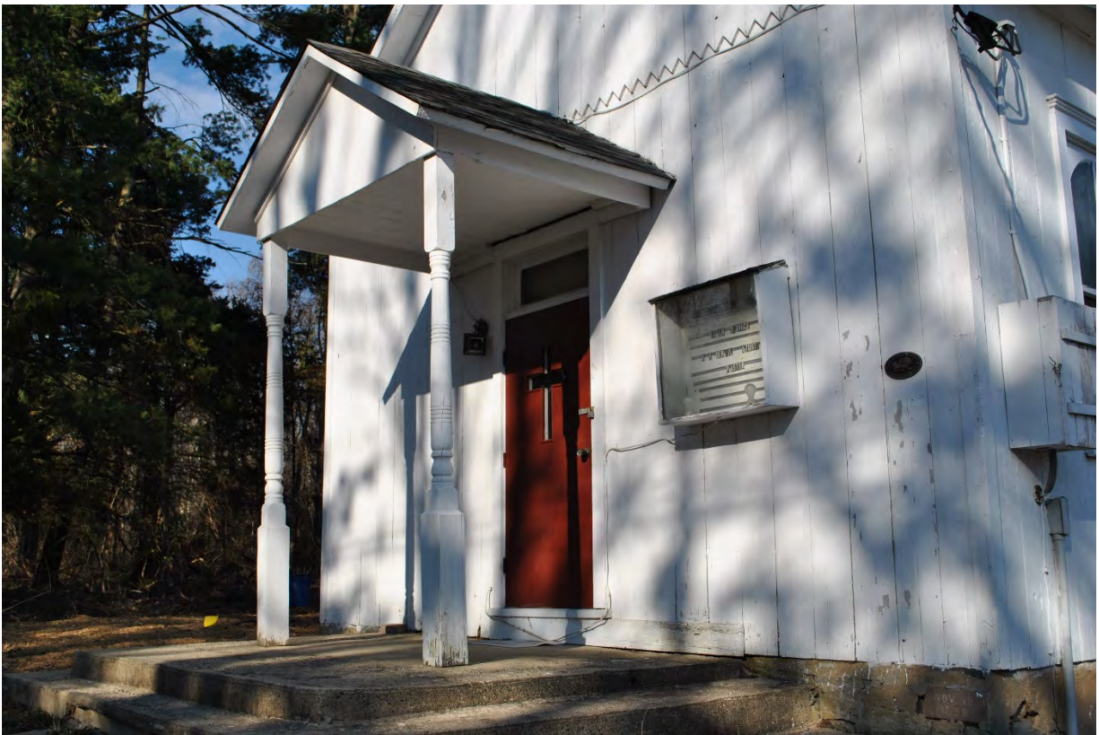
Mount Zion African Methodist Episcopal Church, Somerset County, NJ Photo 6
