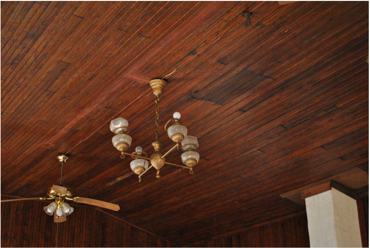
Mount Zion African Methodist Episcopal Church, Somerset County, NJ Photo 9
