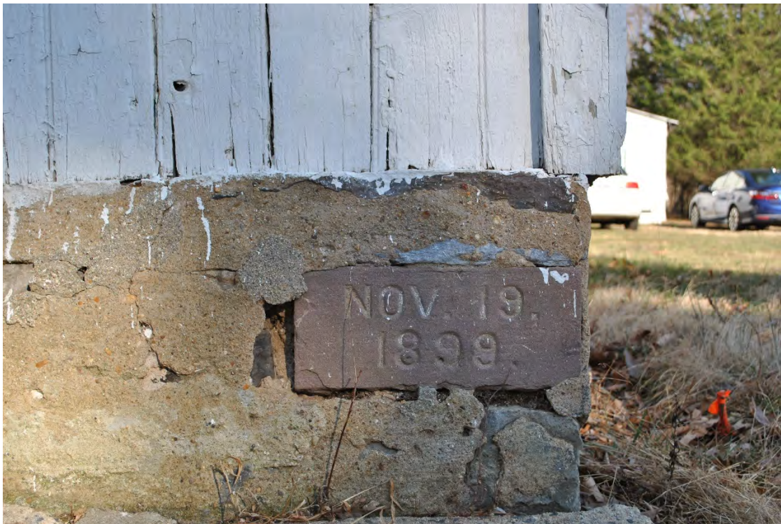
Mount Zion African Methodist Episcopal Church, Somerset County, NJ Photo 8
