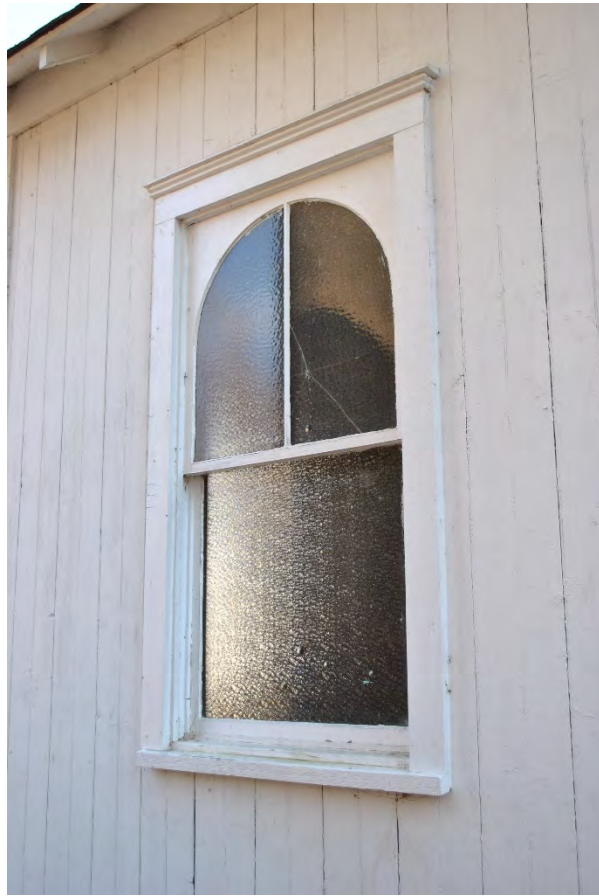
Mount Zion African Methodist Episcopal Church, Somerset County, NJ Photo 7
