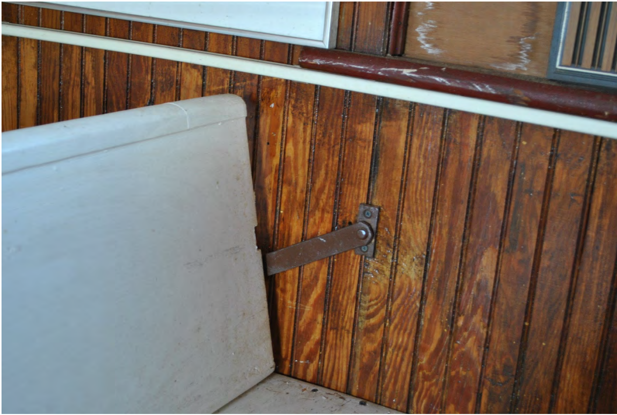
Mount Zion African Methodist Episcopal Church, Somerset County, NJ Photo 13
