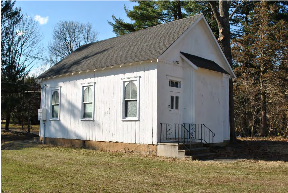
Mount Zion African Methodist Episcopal Church, Somerset County, NJ Photo 5
