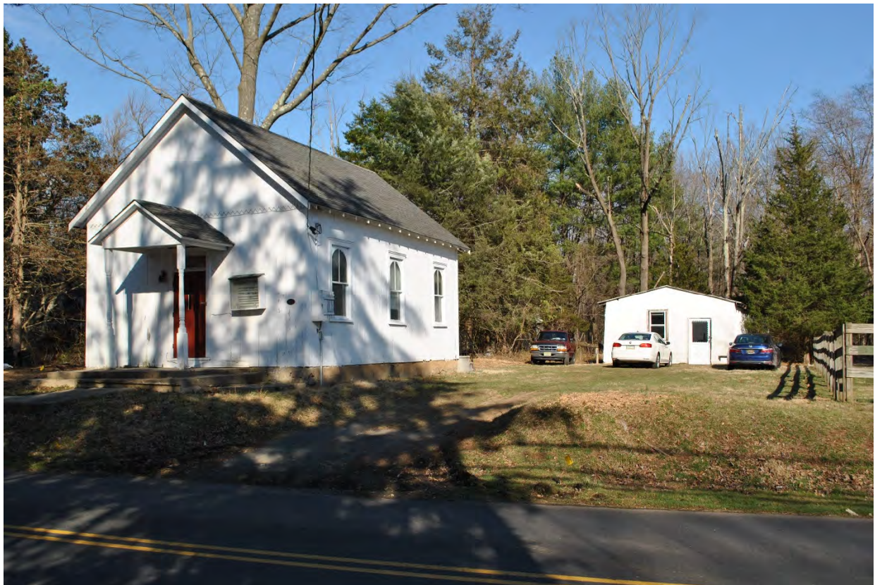
Mount Zion African Methodist Episcopal Church, Somerset County, NJ Photo 2
