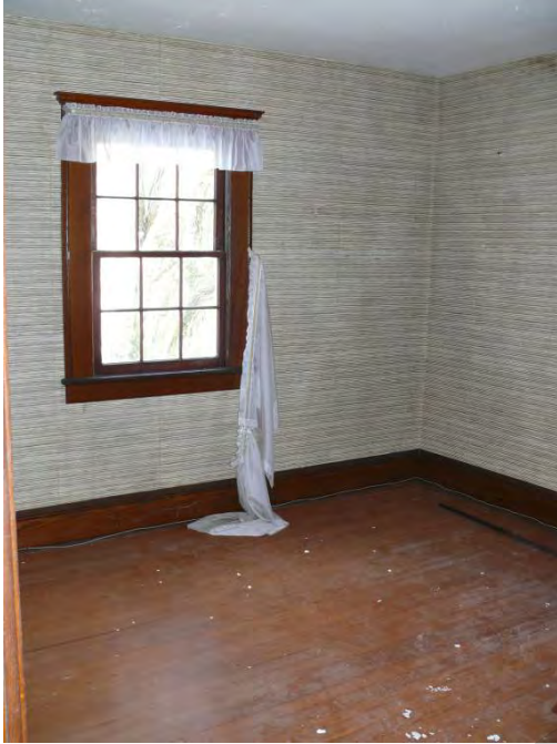
Photo 0019: View of the Northwest Bedroom showing typical second-floor features including six-over- six hung wood window, early-twentieth-century molded wood baseboard and window surround that are finished with varnish rather than paint, wallpapered plaster wall, plaster ceiling, and narrow wood flooring; camera facing northwest.
