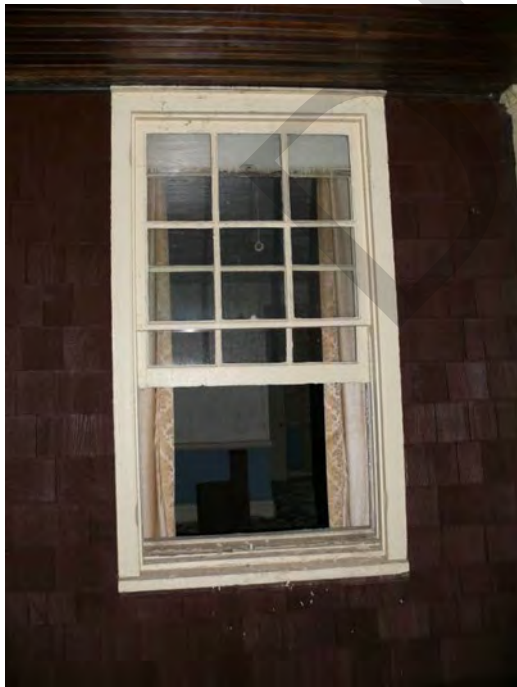
Photo 0006: View of a nineteenth-century six-over-six hung wood window at the front of the c.1840 east section; camera facing north.
