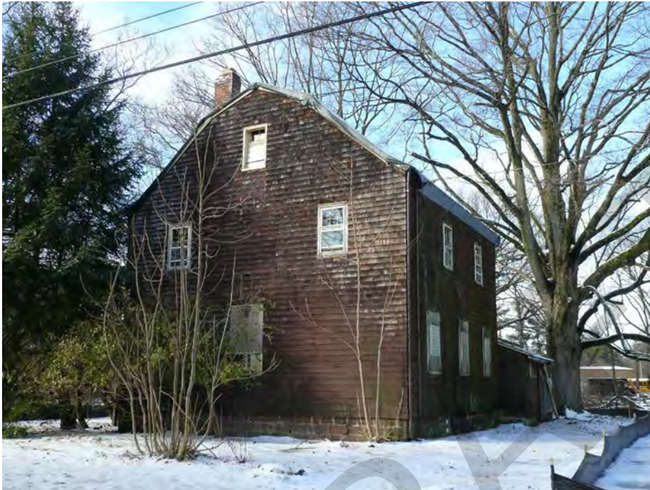
Photo 0009: Overall view of the (side) east elevation; camera facing southeast.
