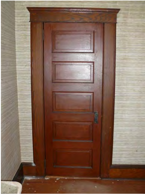
Photo 0021: View of an early-twentieth-century five-panel wood door found throughout the second floor level; camera facing east.
