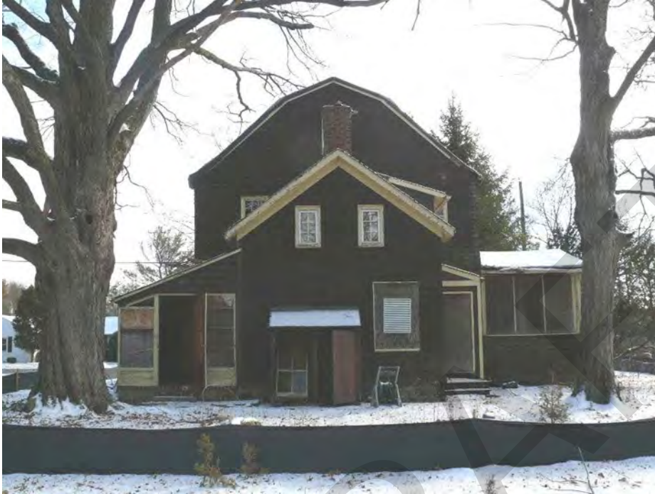
Photo 0007: Overall view of the (side) west elevation; camera facing east.
