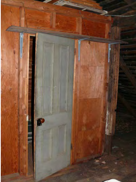
Photo 0023: View of the twentieth-century cedar closet with reused nineteenth-century, four-panel wood door in the attic; camera facing east.
