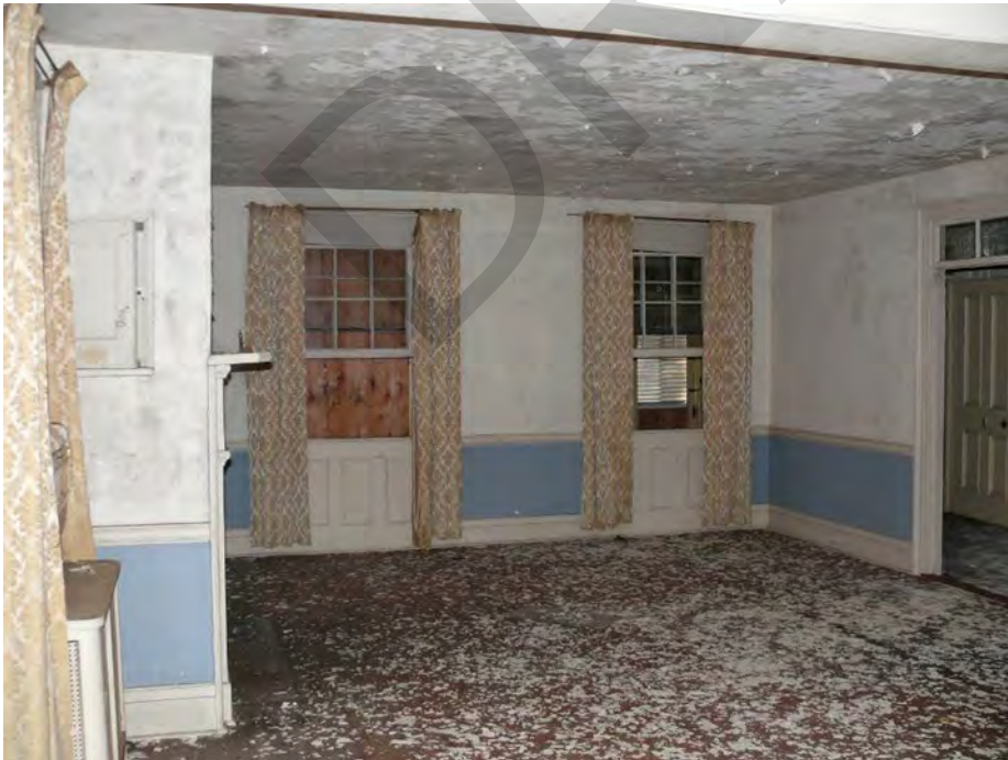
Photo 0014: View of the Parlor showing typical first-floor features including six-over-six hung wood windows set over paneled wainscot, molded wood chair rail and baseboard, plaster wall and ceiling finishes, and narrow wood flooring; camera facing south.
