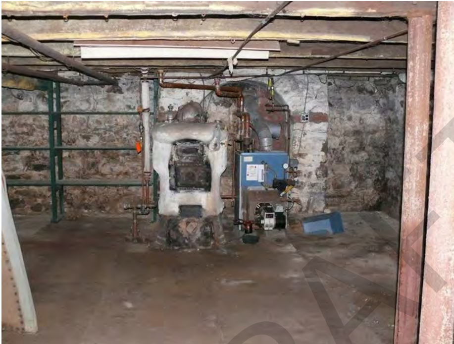
Photo 0011: View of the basement of the c.1840 east section showing whitewashed masonry walls, an arched fireplace support, and exposed heavy timber framing; camera facing east.
