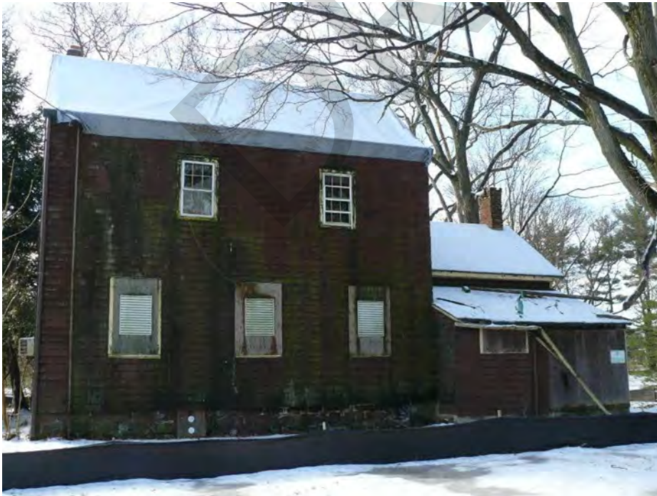
Photo 0008: Overall view of the (rear) north elevation; camera facing south.
