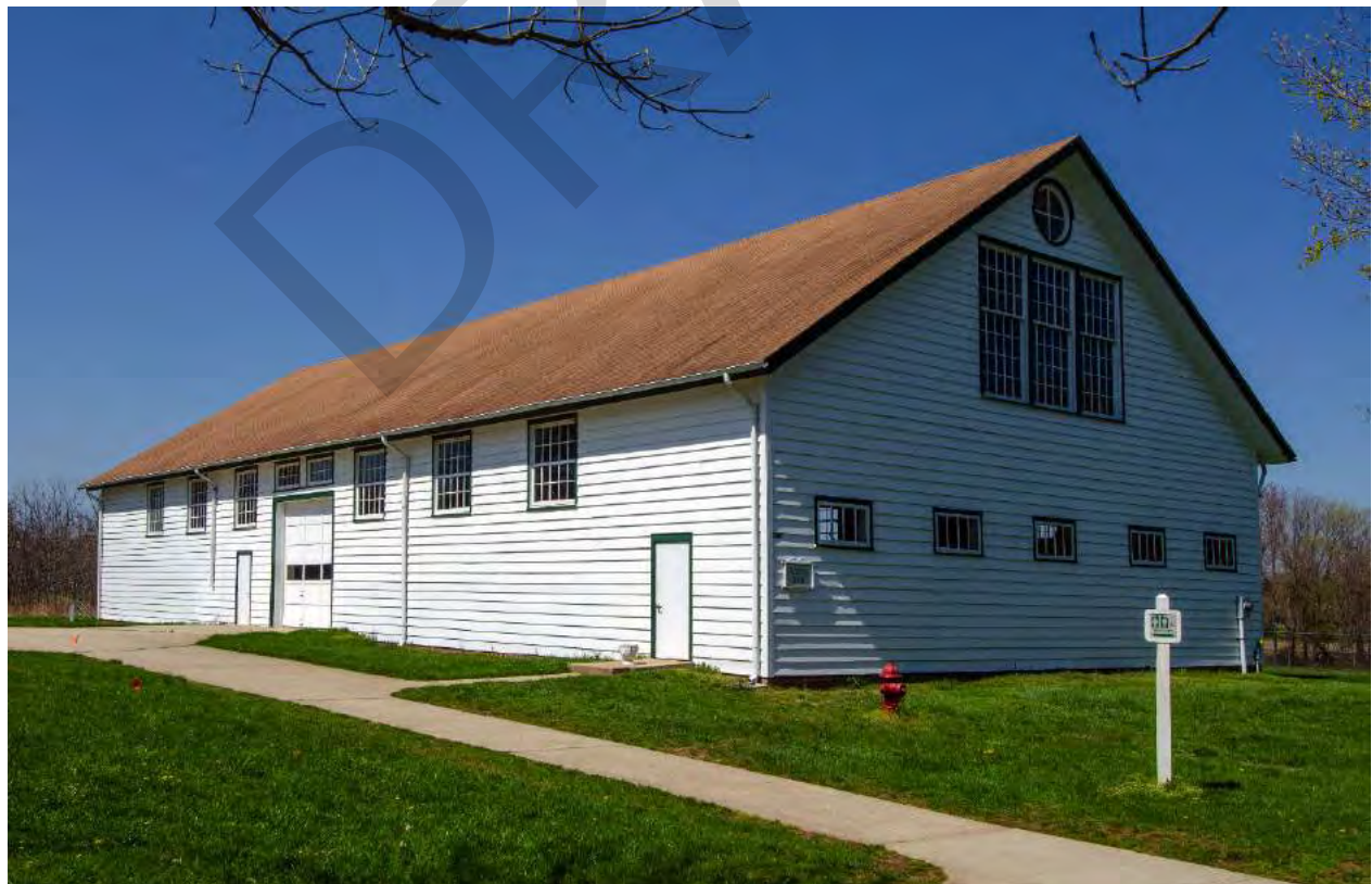
9.2 Yearling Barn 2 - Activity Barn, view west, C.W. Zink.tif
