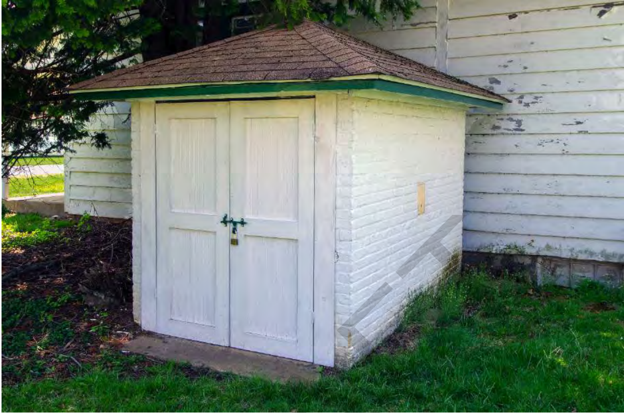
17.1 Hose House - Garbage Shed, view south, C.W. Zink.tif
