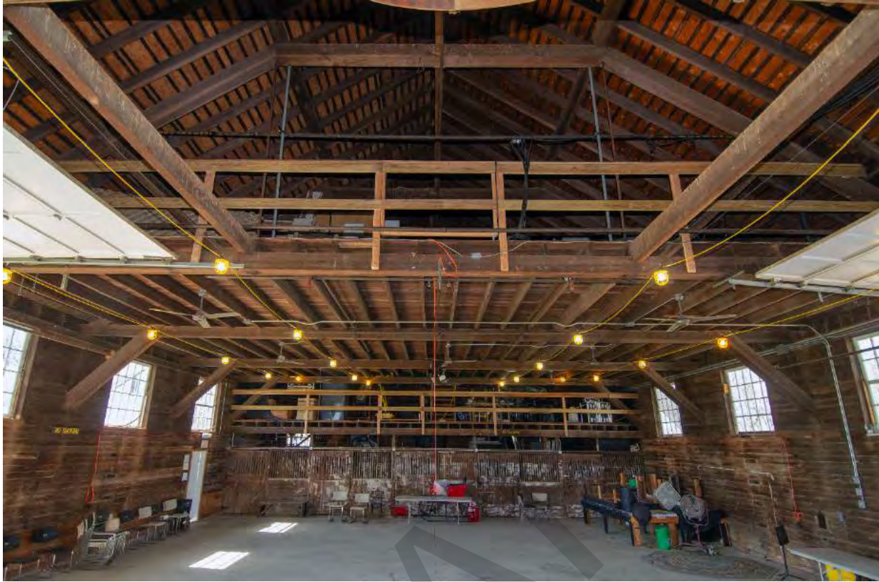
8.3 Yearling Barn 1 - Theatre Barn, view west, C.W. Zink.tif
