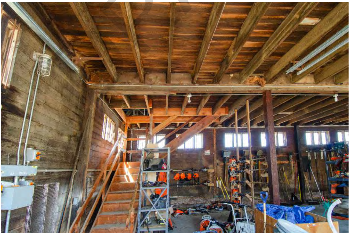
6.4 Ten Mare Barn - Garage Storage, view north, C.W. Zink.tif
