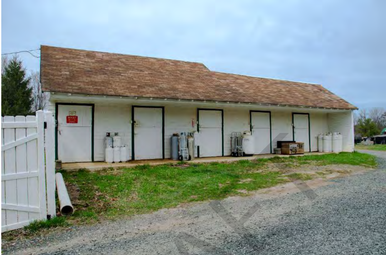
20.1 Five-Stall Stable - Lumber Storage, view north, C.W. Zink.tif
