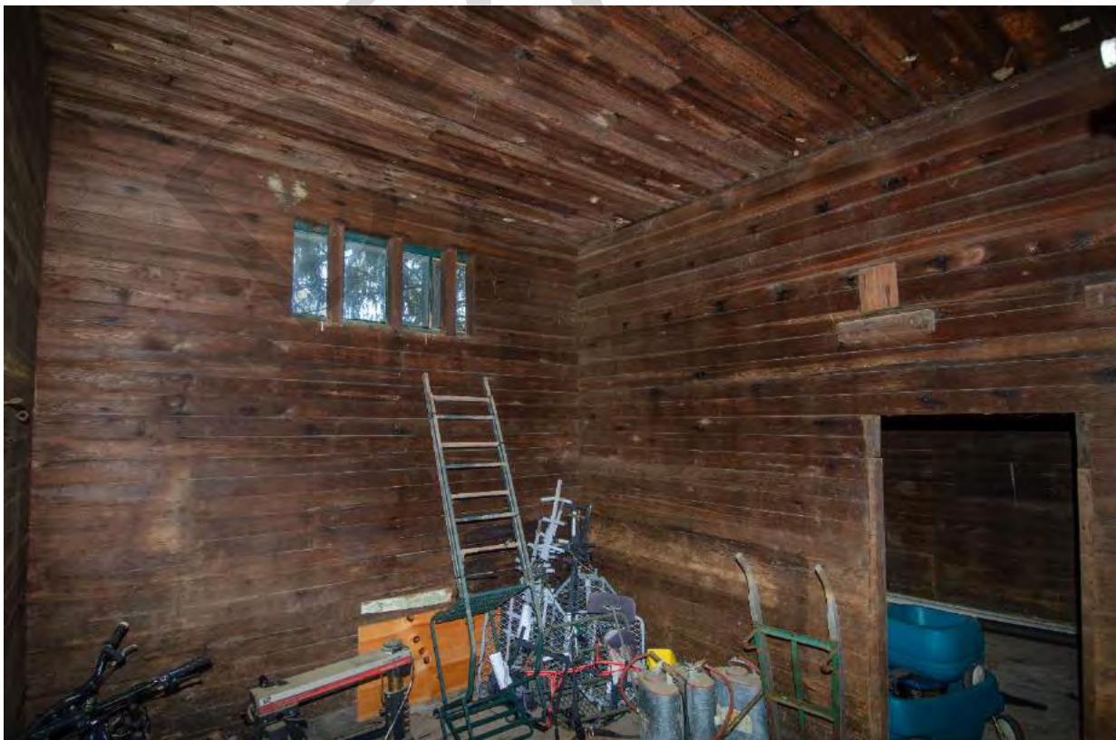
10.2 Two Stall Stable, Administration Storage, view south, C.W. Zink.tif
