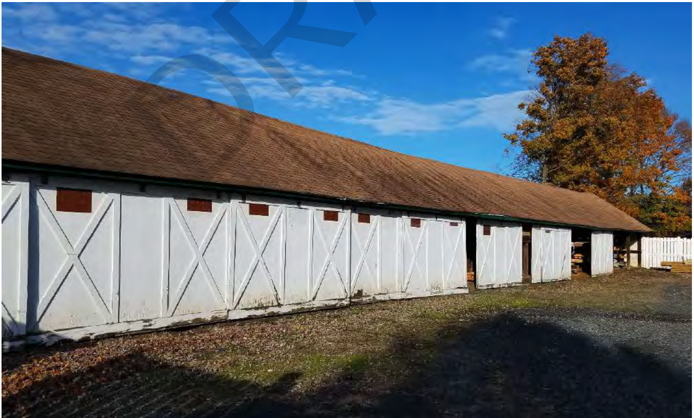
19.1 Shed - Lumber Shed, view north west, K. Norbut.tif
