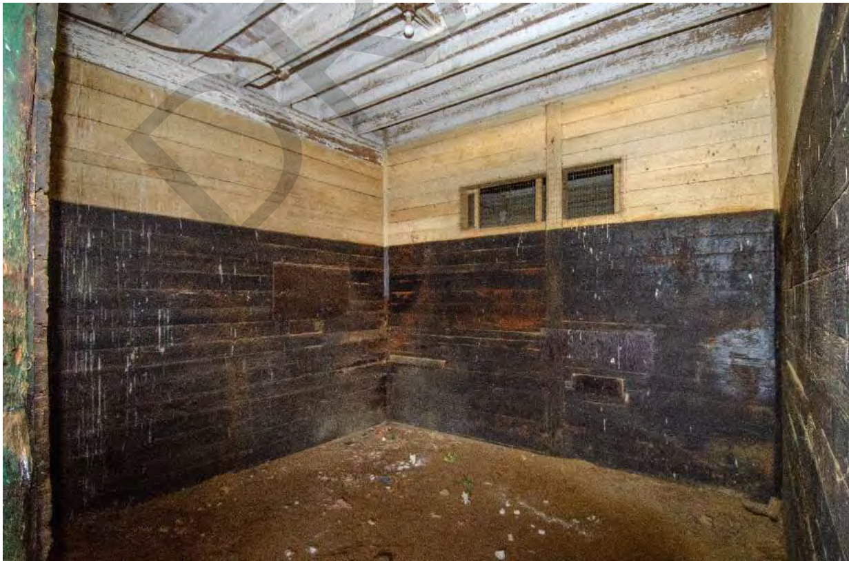
5.8 Training Stable, South Walk Loose Box, view west, C.W. Zink.tif
