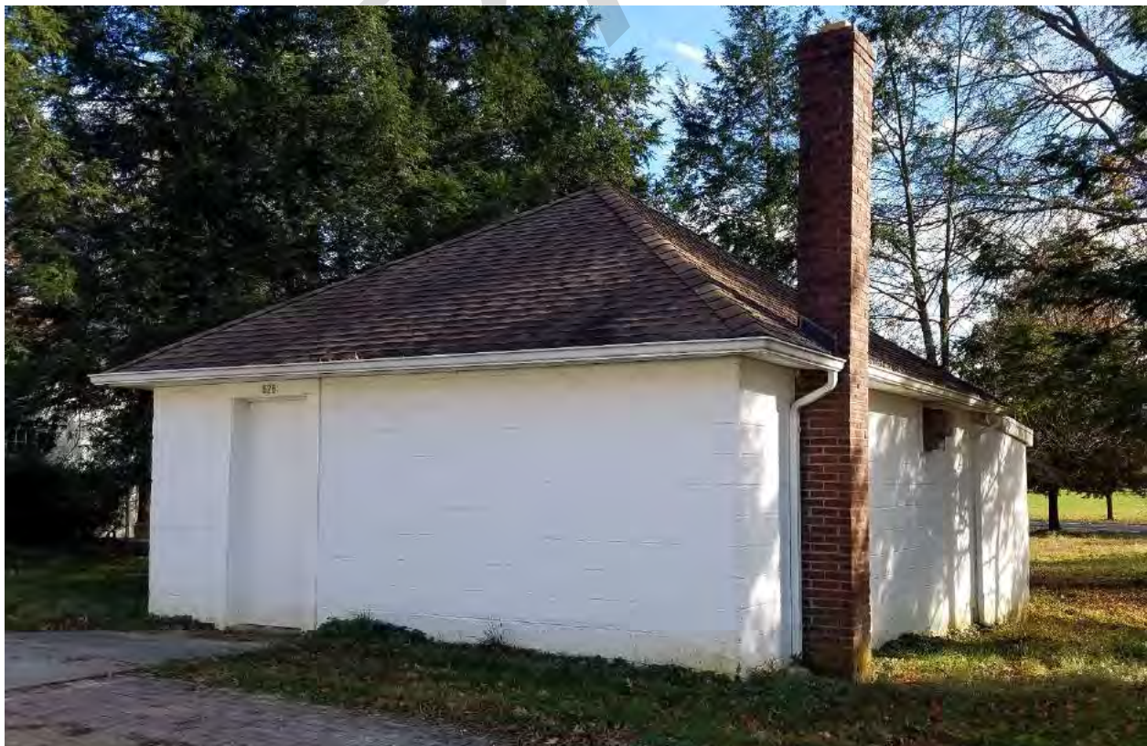
22.1 Construction & Repair Storage, view east, C.W. Zink.tif
