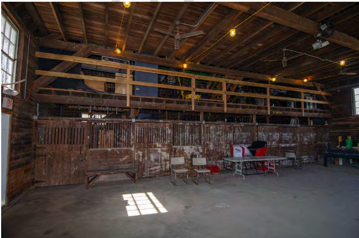
8.4 Yearling Barn 1 - Theatre Barn, view west, C.W. Zink.tif
