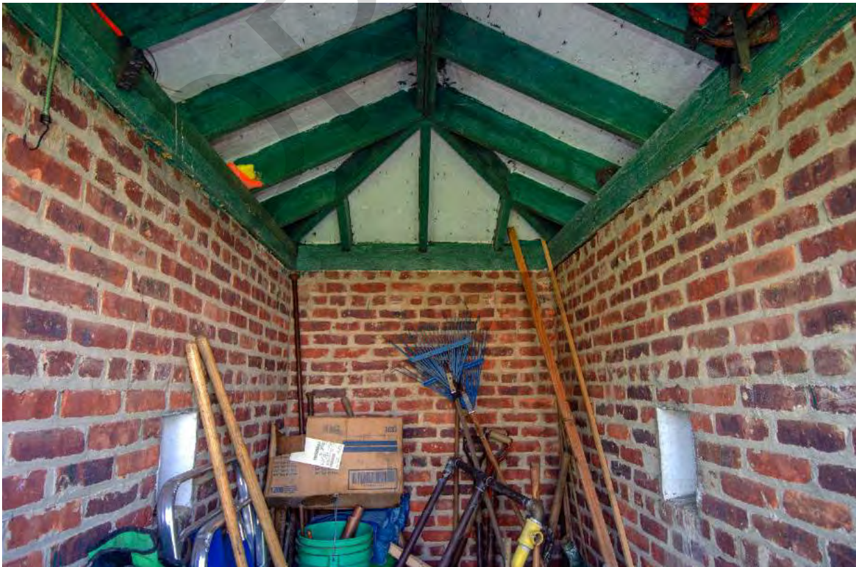
17.2 Hose House - Garbage Shed, view south, C.W. Zink.tif
