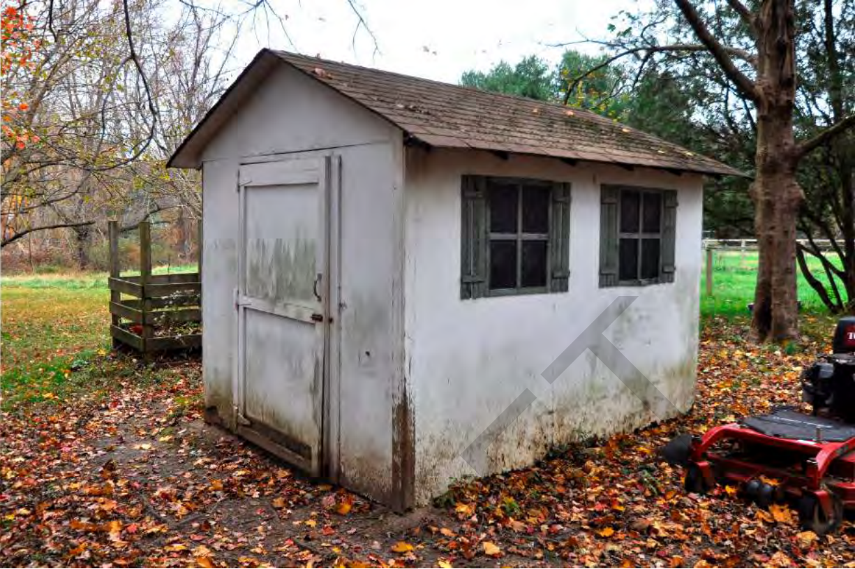
35.1 Storage Shed, view west, K. Norbut.tif
