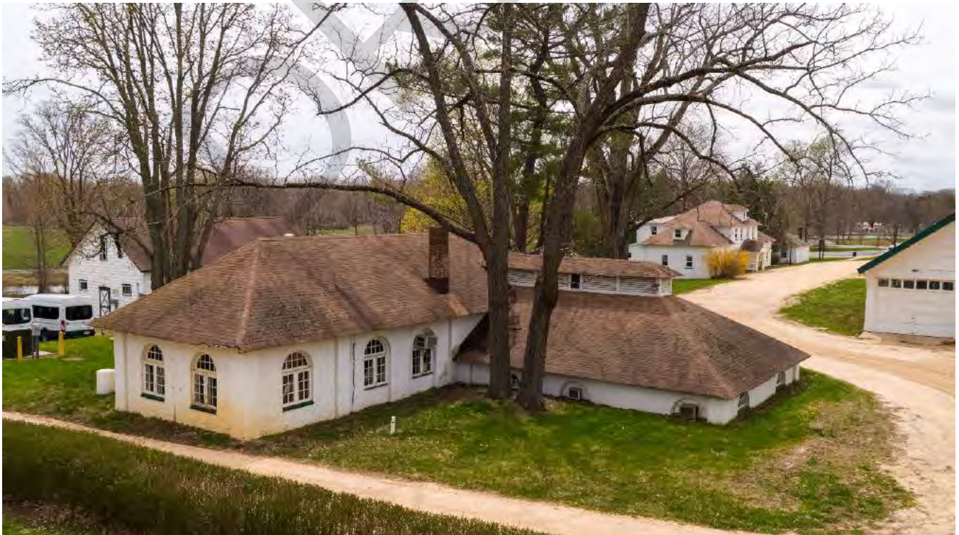
11.2 Pump House & Reservoir - Construction & Sign Shops, view south, B. Parigian.tif
