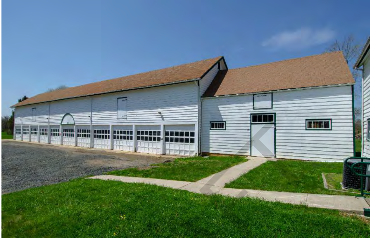
6.1 Ten Mare Barn - Garage Storage & Lloyd Barn 1, view west, C.W. Zink.tif
