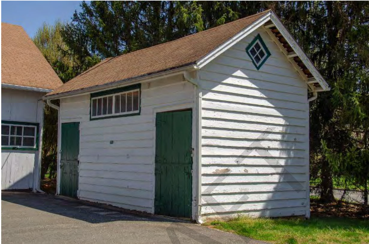
10.1 Two-Stall Stable, Administration Storage, view east, C.W. Zink.tif
