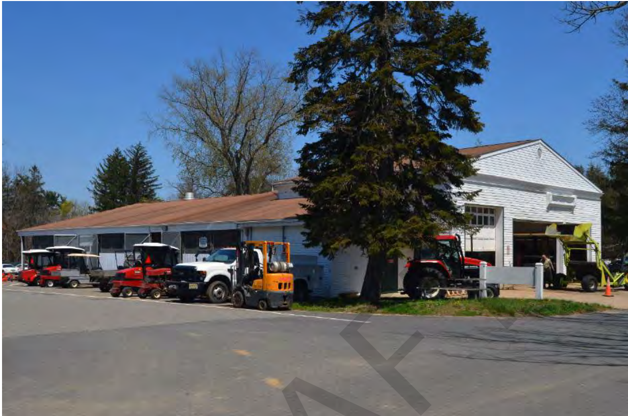
13.1 Garage - Maintenance Shop, view north, C.W. Zink.tif
