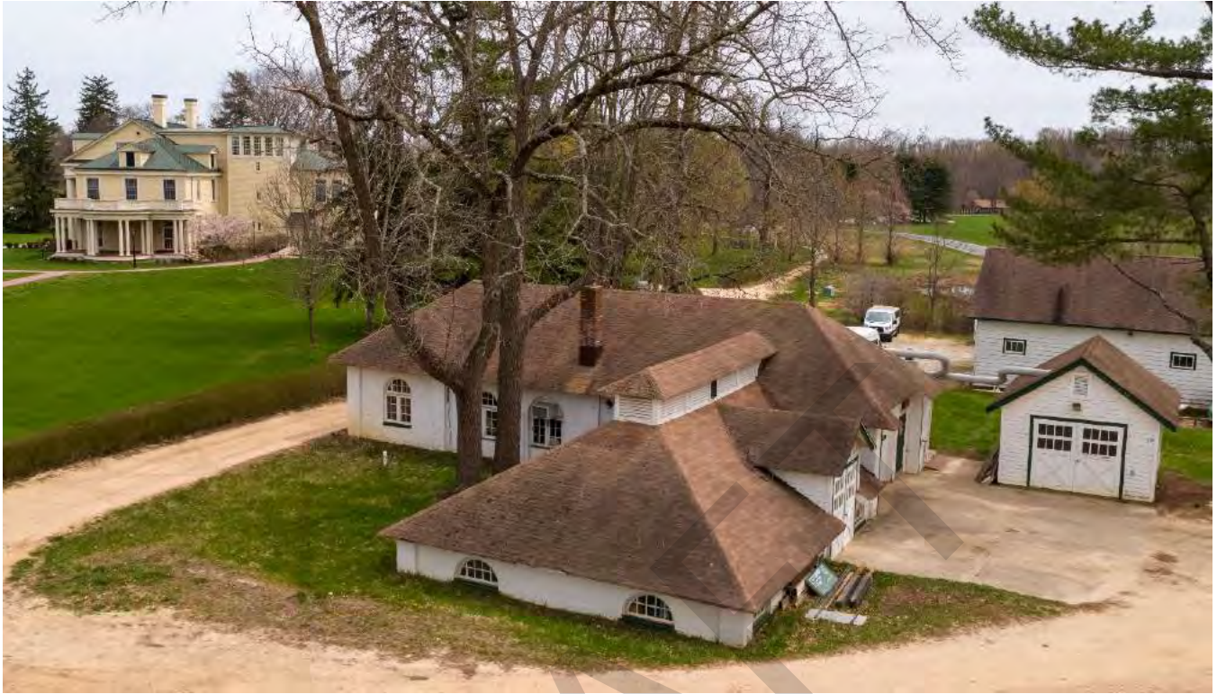
11.1 Pump House & Reservoir - Construction & Sign Shops, view east, B. Parigian.tif
