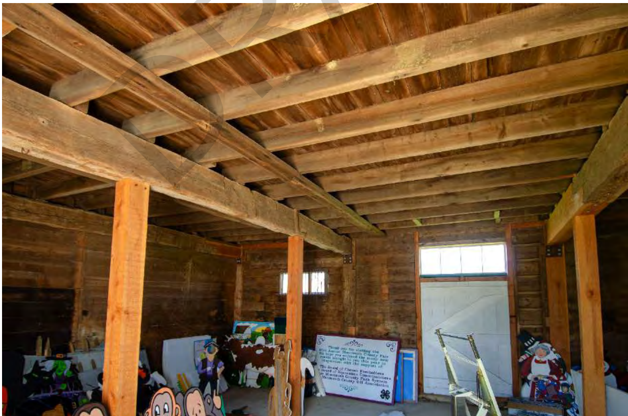
2.2 Lloyd Barn 1 - Garage Storage, view northwest, C.W. Zink.tif
