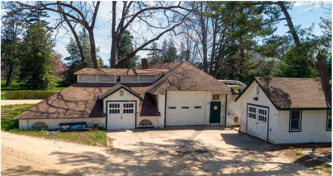
11.3 Pump House & Reservoir - Construction & Sign Shops, view northeast, B. Parigian.tif
