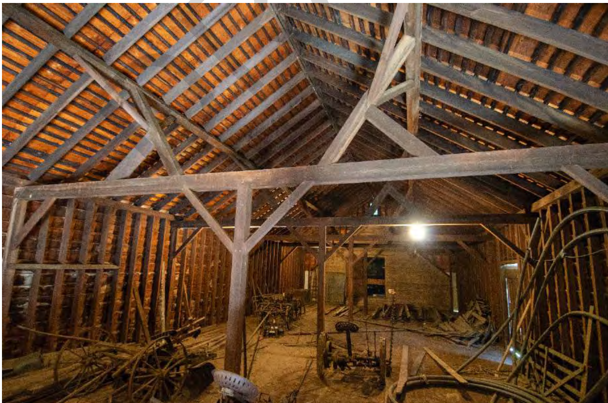
6.6 Ten Mare Barn - Garage Storage, view northeast, C.W. Zink.tif
