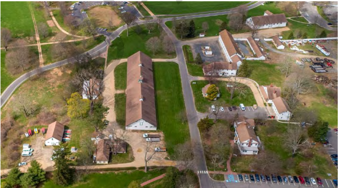
0.4 Brookdale Farm, Operations Area, view southwest, B. Parigian.tif
