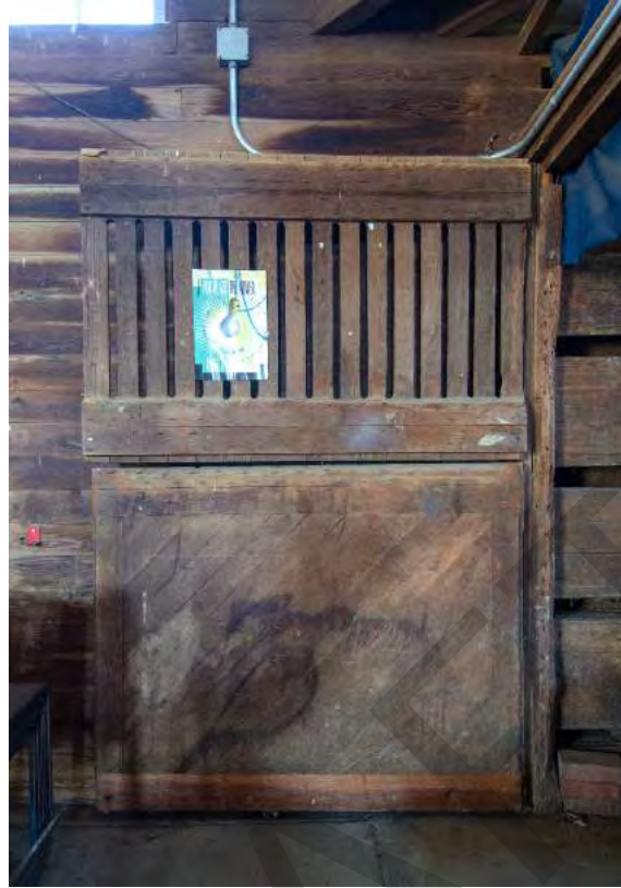
8.5 Yearling Barn 1 - Theatre Barn, view north, C.W. Zink.tif
