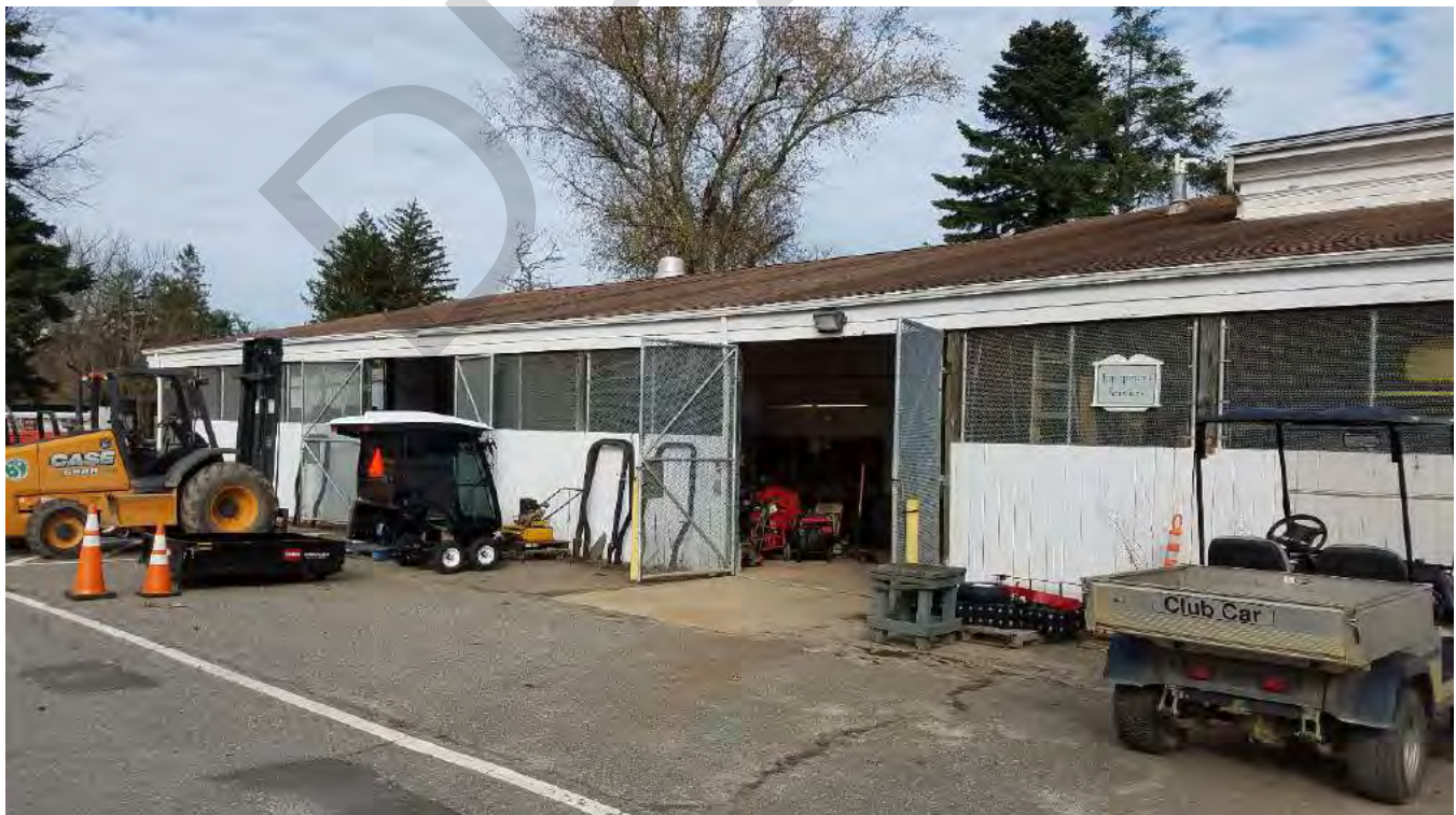
14.1 Garage - Maintenance, view north, C.W. Zink.tif
