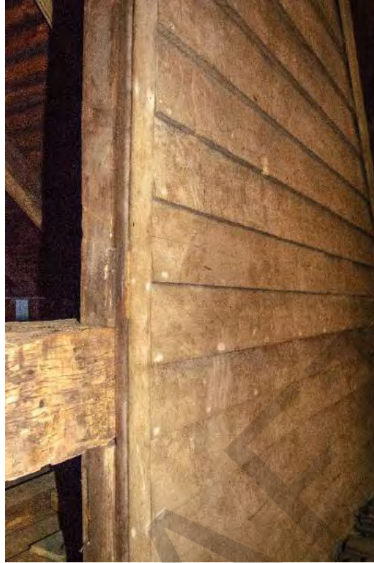
2.5 Lloyd Barn 1 - Garage Storage, view southeast, C.W. Zink.tif
