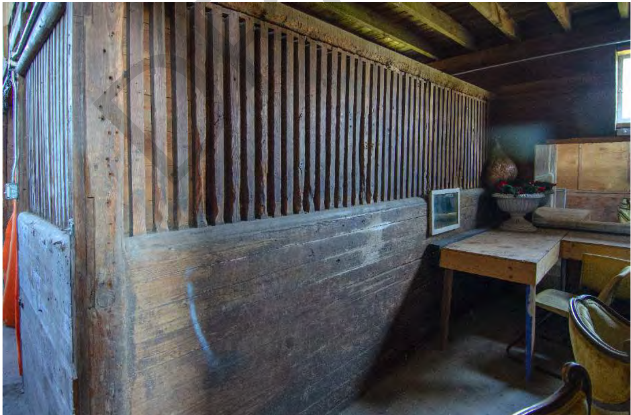
8.6 Yearling Barn 1 - Theatre Barn, view north, C.W. Zink.tif
