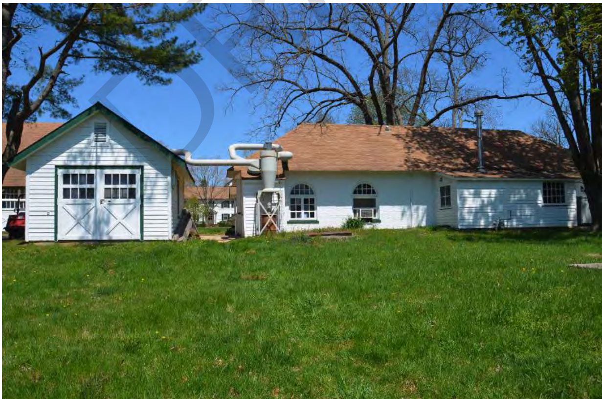
11.4 Saw Building & Pump House, View North, C.W. Zink.tif
