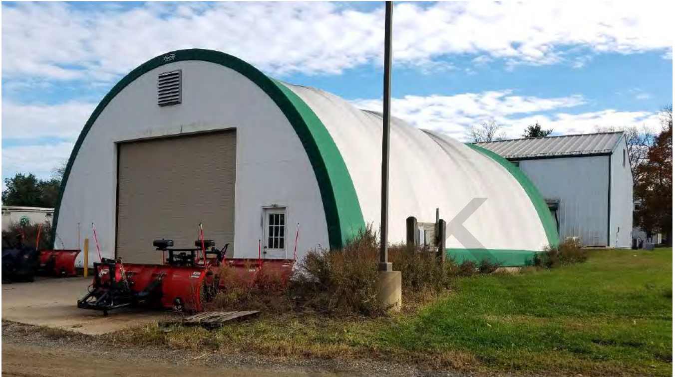
30.1 Sand Storage Building, view south, K. Norbut.tif
