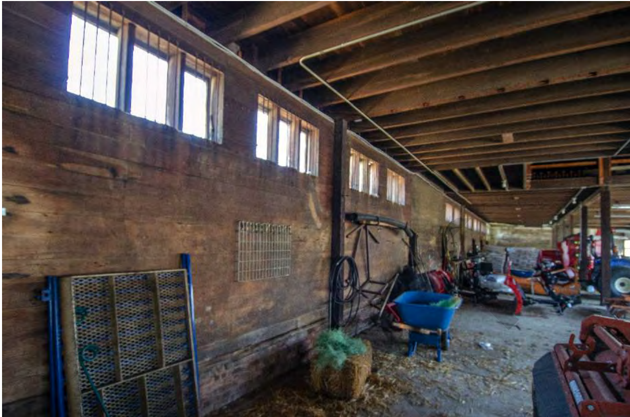
6.5 Ten Mare Barn - Garage Storage, view north, C.W. Zink.tif
