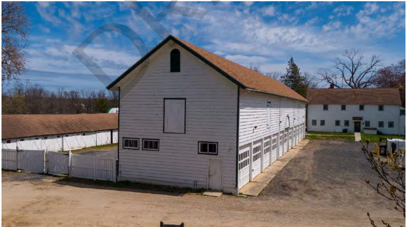
6.2 Ten Mare Barn - Garage Storage, view northeas, B. Parigian.tif
