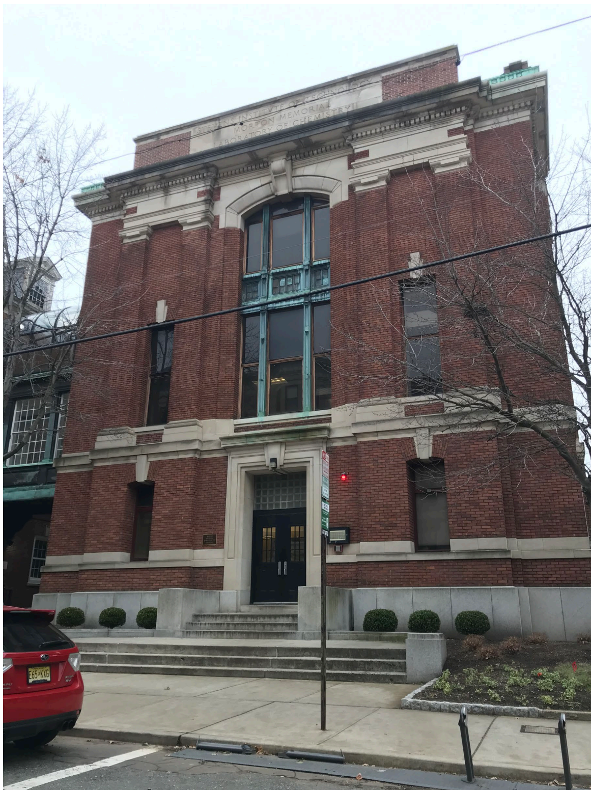
Photo 2. Morton Memorial Laboratory of Chemistry, main (west) elevation. Stevens Institute of Technology, Hoboken (Hudson County), NJ. (Meredith Arms Bzdak, 13 December 2019.)
