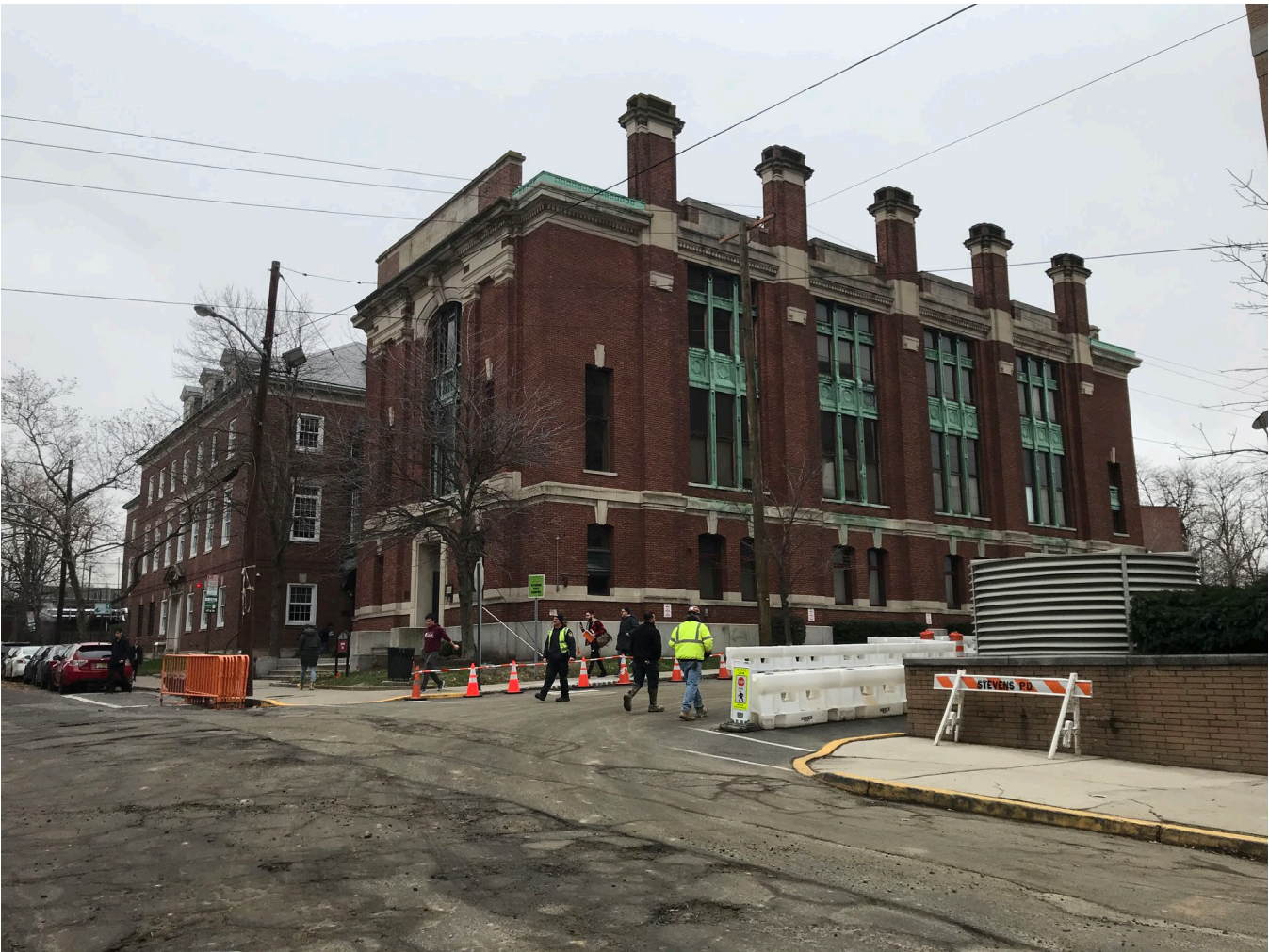
Photo 1. Morton Memorial Laboratory of Chemistry, View of west and south elevations from River Street, with the intersection of River Street and Sixth Street in the foreground. Stevens Institute of Technology, Hoboken (Hudson County), NJ. (Meredith Arms Bzdak, 13 December 2019.)
