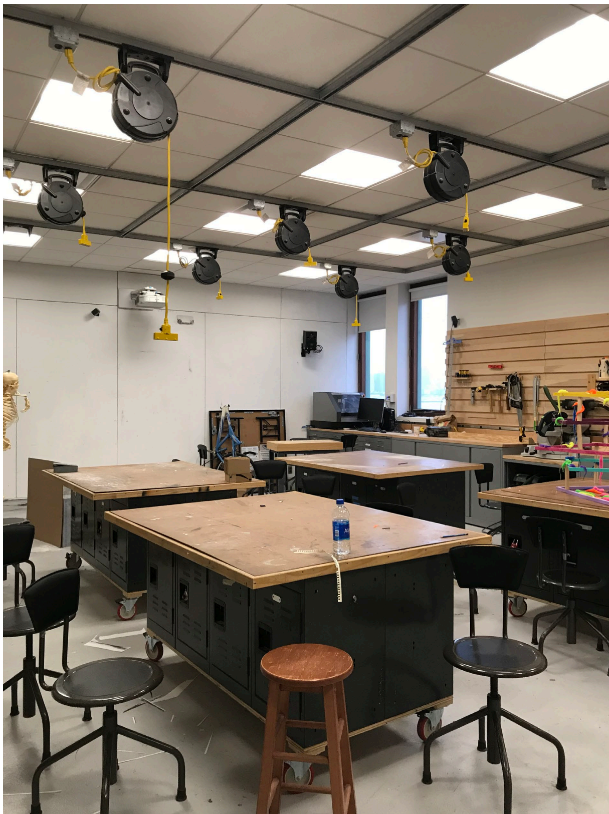
Photo 11. Morton Memorial Laboratory of Chemistry, typical classroom space, second floor. Stevens Institute of Technology, Hoboken (Hudson County), NJ. (Meredith Arms Bzdak, 13 December 2019.)
