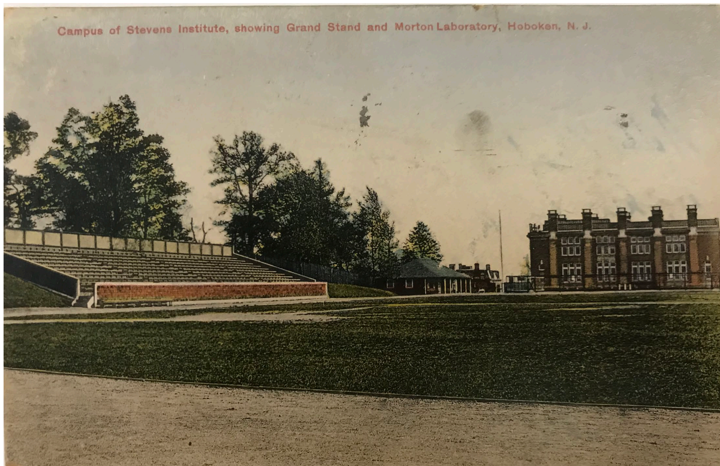
Figure 20. The new “Castle Point Athletic Field,” located to the north of the newly constructed Morton Hall on eleven acres of the formerly private Stevens estate, was completed in 1907 and included a grandstand and a field house (Archives and Special Collections, Stevens Institute of Technology).
