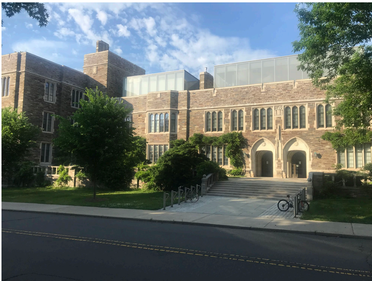
Photo S13. Charles Z. Klauder, Frick Chemistry Laboratory, 1929, Princeton University, Princeton, NJ. (Photo 2020, Mills + Schnoering Architects)
