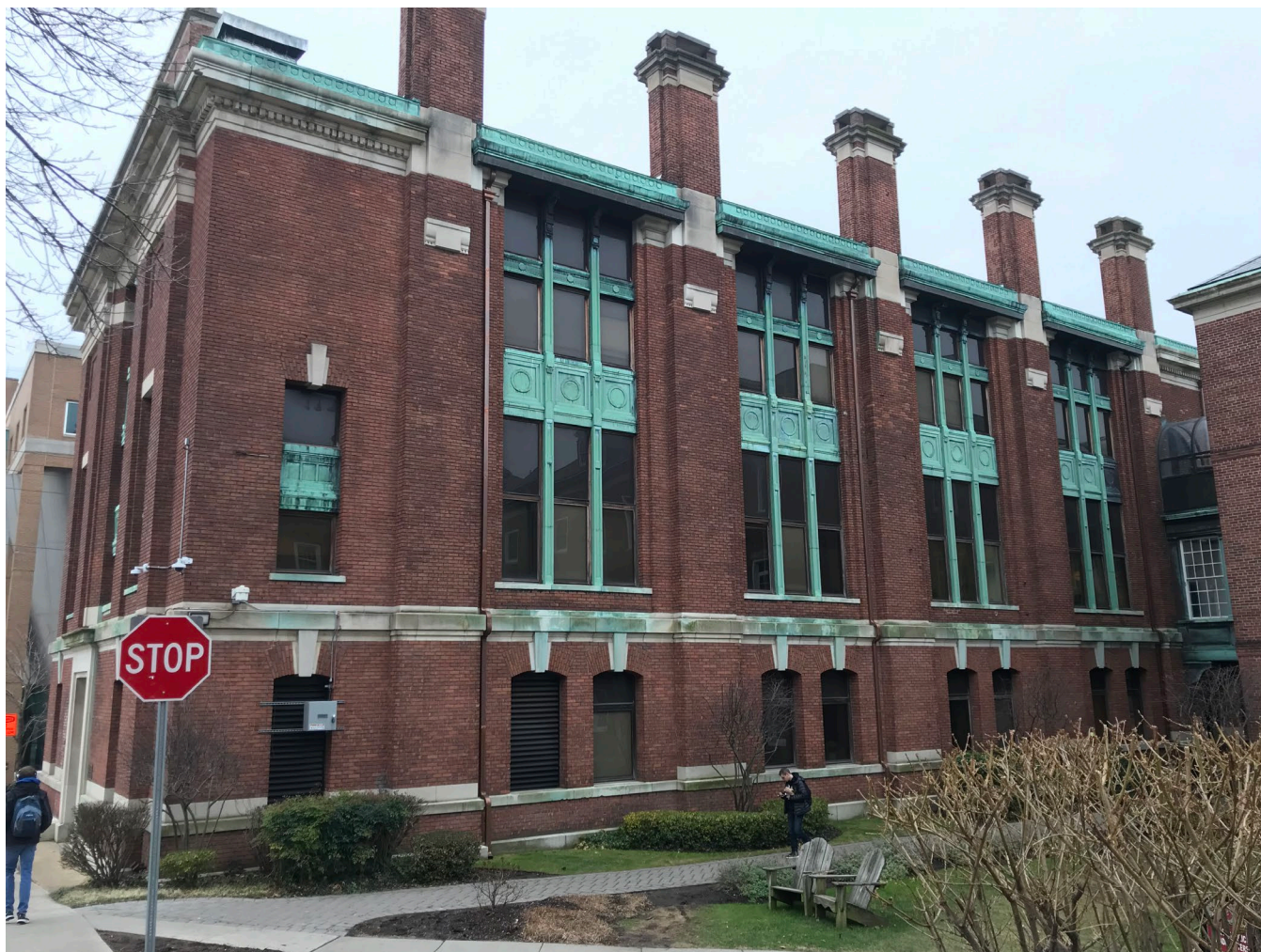
Photo 6. Morton Memorial Laboratory of Chemistry, north elevation, looking southwest. Stevens Institute of Technology, Hoboken (Hudson County), NJ. (Meredith Arms Bzdak, 13 December 2019.)
