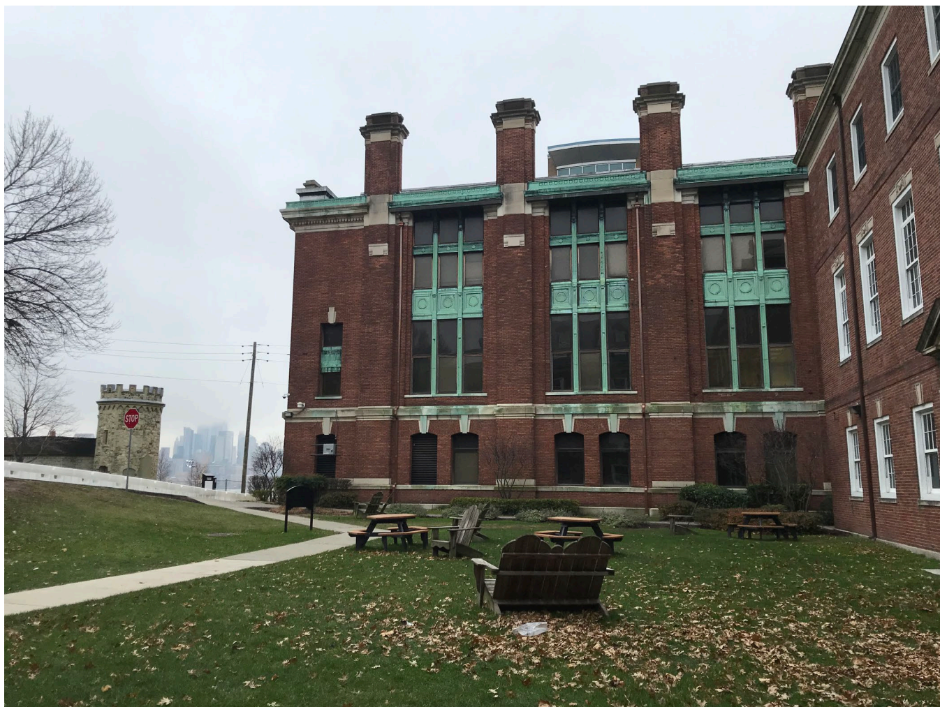
Photo 7. Morton Memorial Laboratory of Chemistry, north elevation, looking southeast (Peirce Hall at the right). Stevens Institute of Technology, Hoboken (Hudson County), NJ. (Meredith Arms Bzdak, 13 December 2019.)
