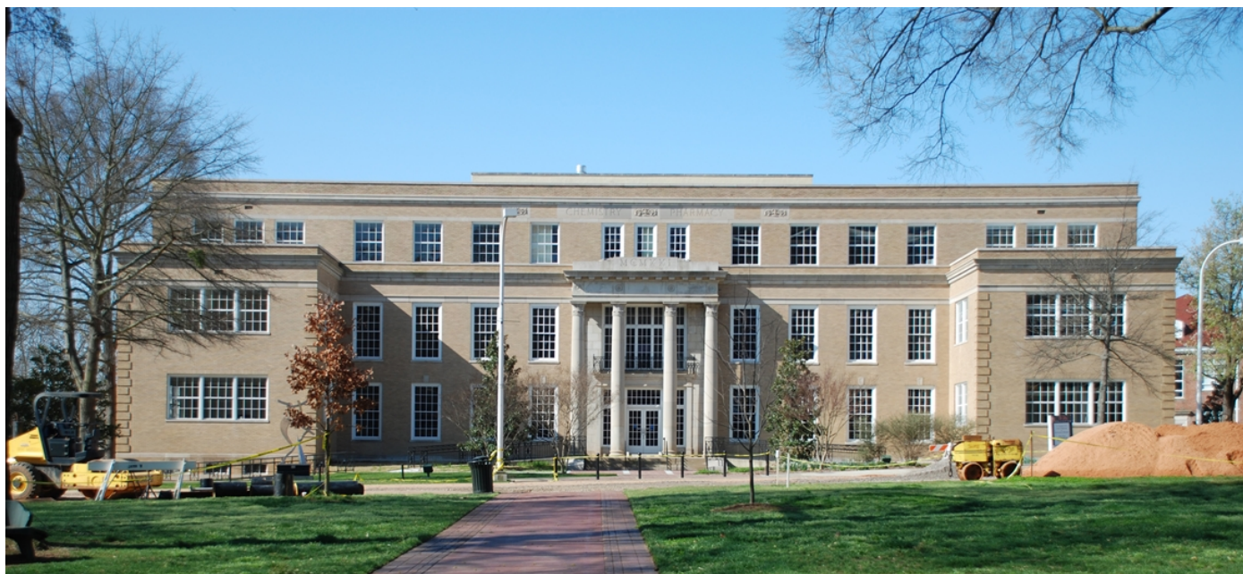
Photo S12. Link & Trueblood, Old Chemistry Building (now Brevard Hall), 1923, University of Mississippi, Oxford, MS (Photo 2008, Susan Tietz, https://www.apps.mdah.ms.gov/Public/prop.aspx?view=facts )
