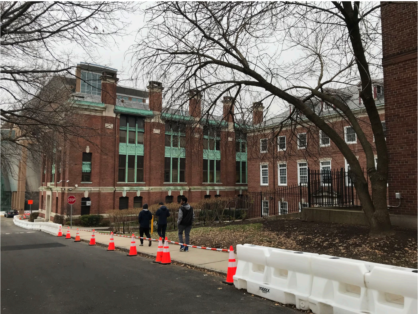
Photo 8. Morton Memorial Laboratory of Chemistry, east and north elevations, looking southwest, showing courtyard formed by the addition of Peirce and Kidde Halls. Stevens Institute of Technology, Hoboken (Hudson County), NJ. (Meredith Arms Bzdak, 13 December 2019.)
