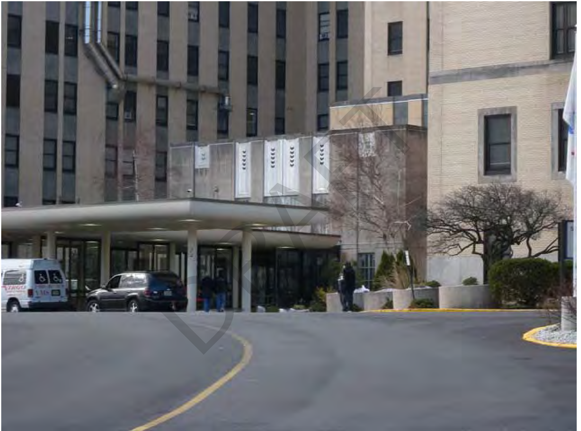
East Orange VA Hospital, Photo 2
