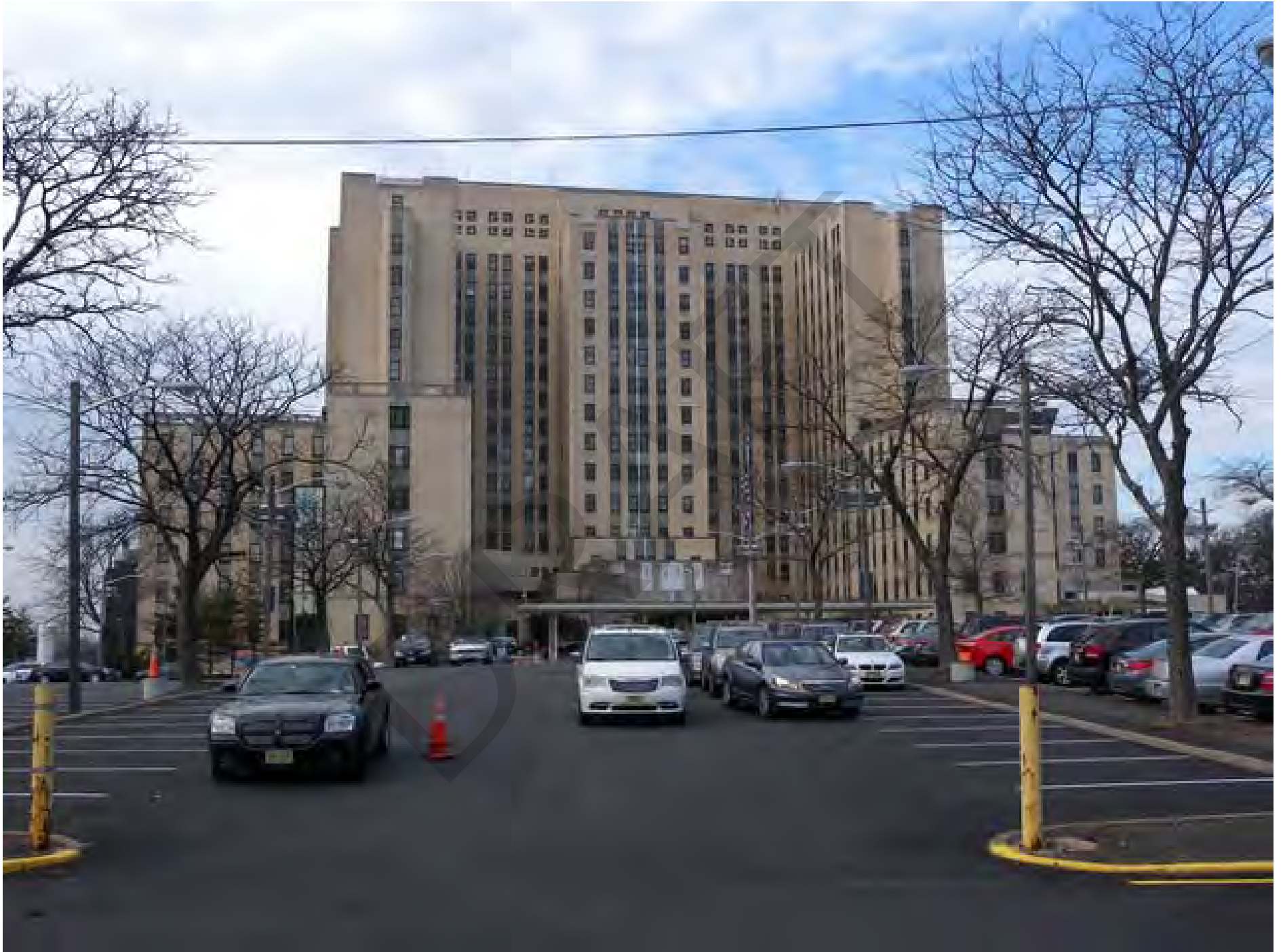
East Orange VA Hospital, Photo 1
