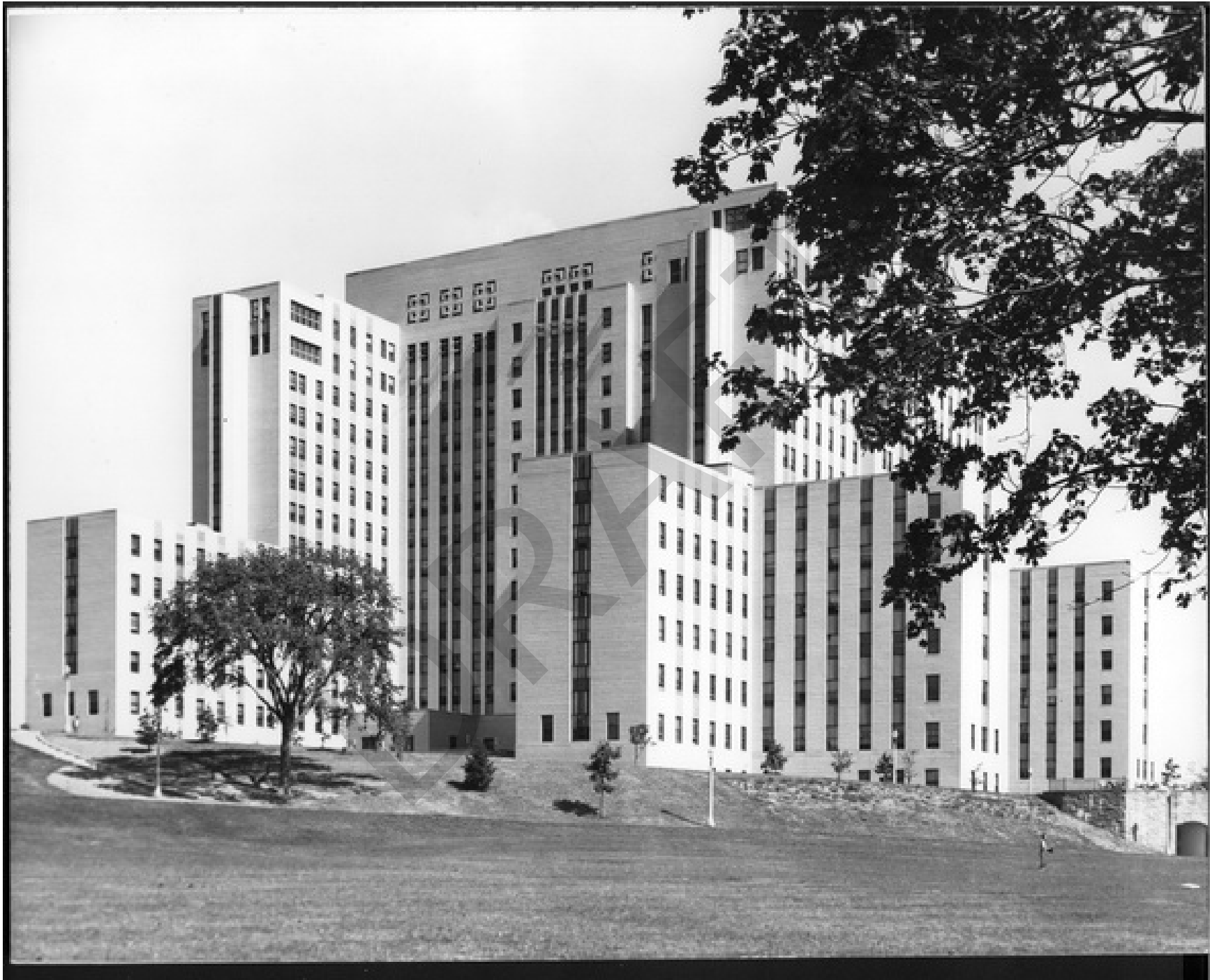
East Orange VA Hospital, Photo 9
