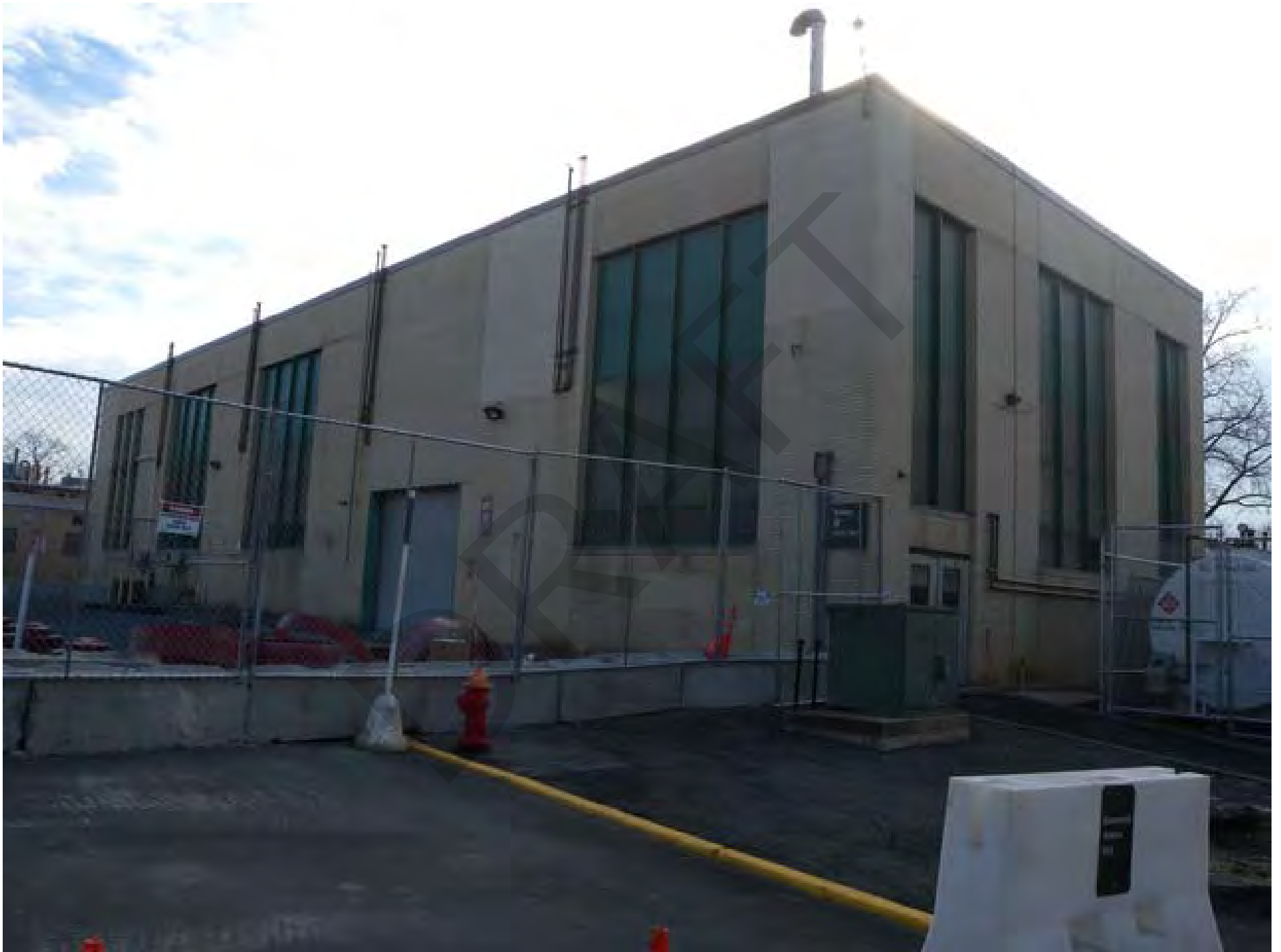
East Orange VA Hospital, Photo 7
