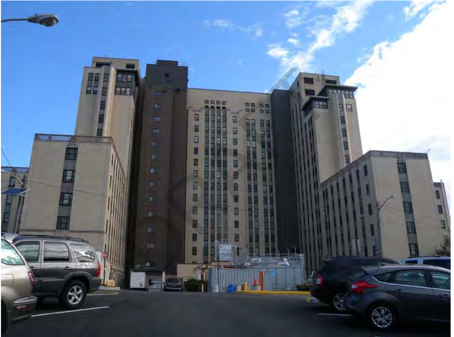
East Orange VA Hospital, Photo 4
