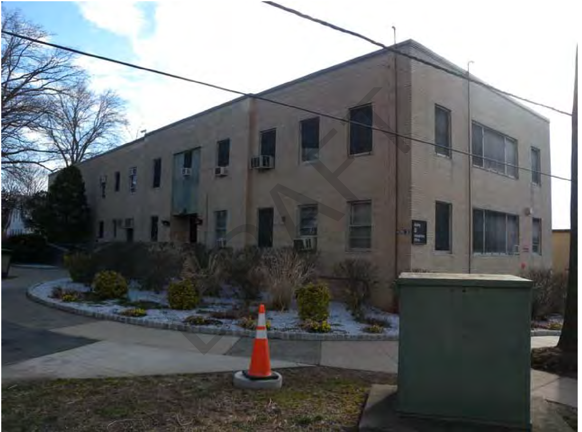
East Orange VA Hospital, Photo 6
