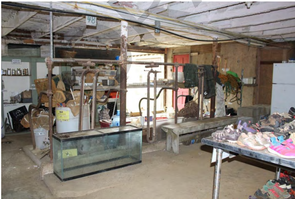
Photo 26: The interior of the barn retains its sloped and curbed concrete floor and cow stanchions, remnant of the dairy operation that began in the 1940s. The barn held as many as 100 cows at times.
