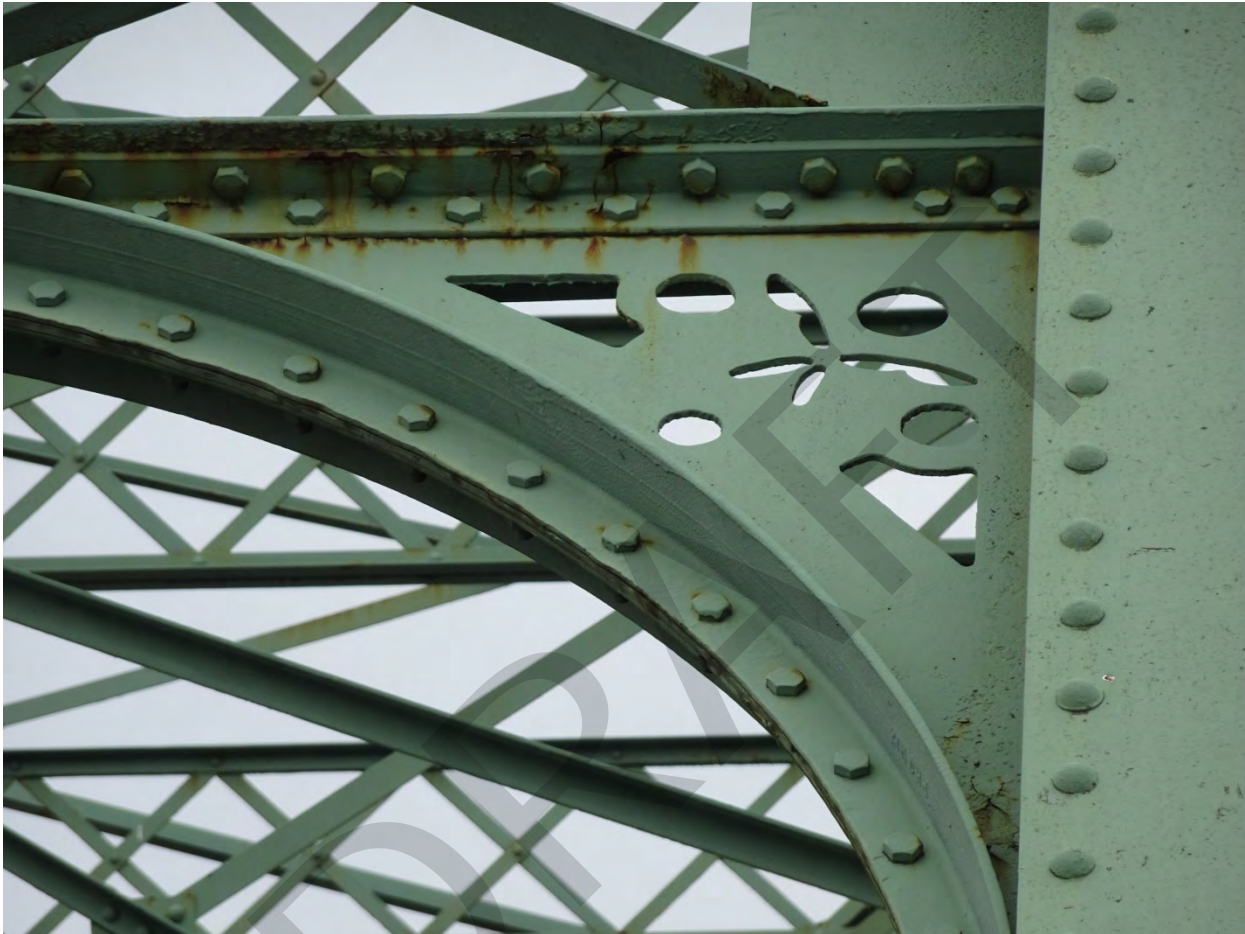
Photograph 8. Detail of decorative stamp in portal bracing, view north.
