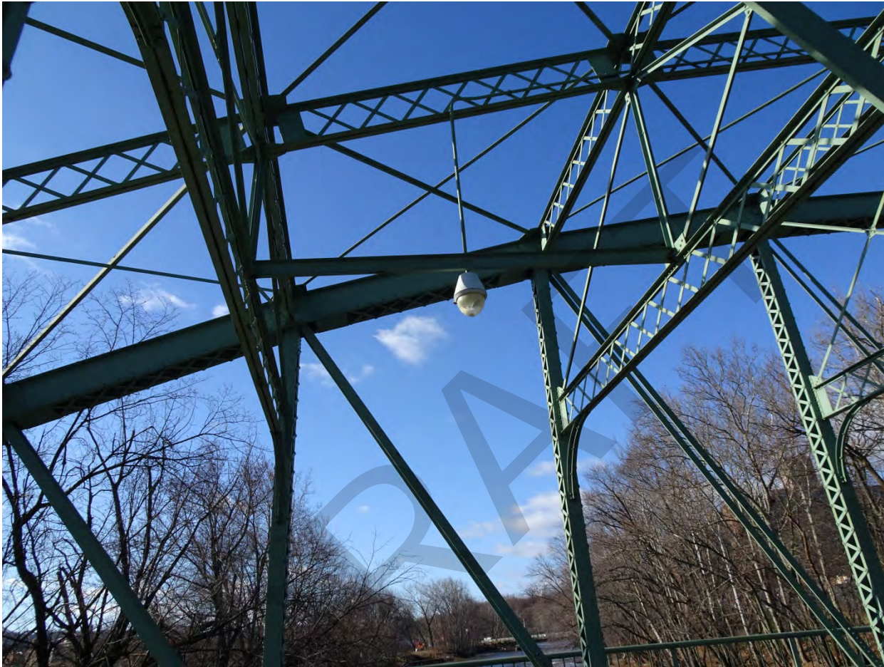
Photograph 7. Truss detail, showing the polygonal top chord, stepped-length verticals, and diagonals in panels, view west.
