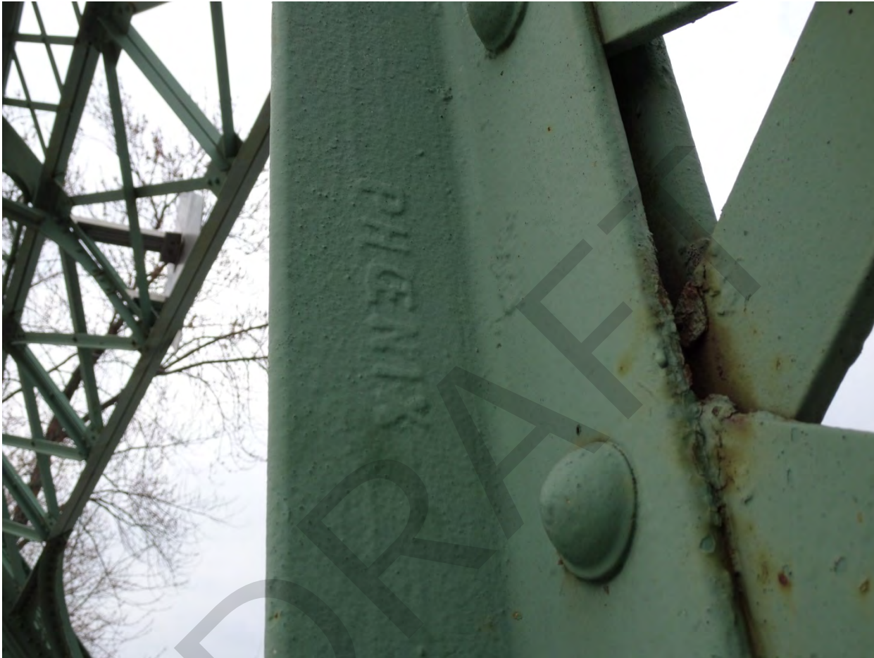
Photograph 10. Steel manufacturer's imprint, view west.
