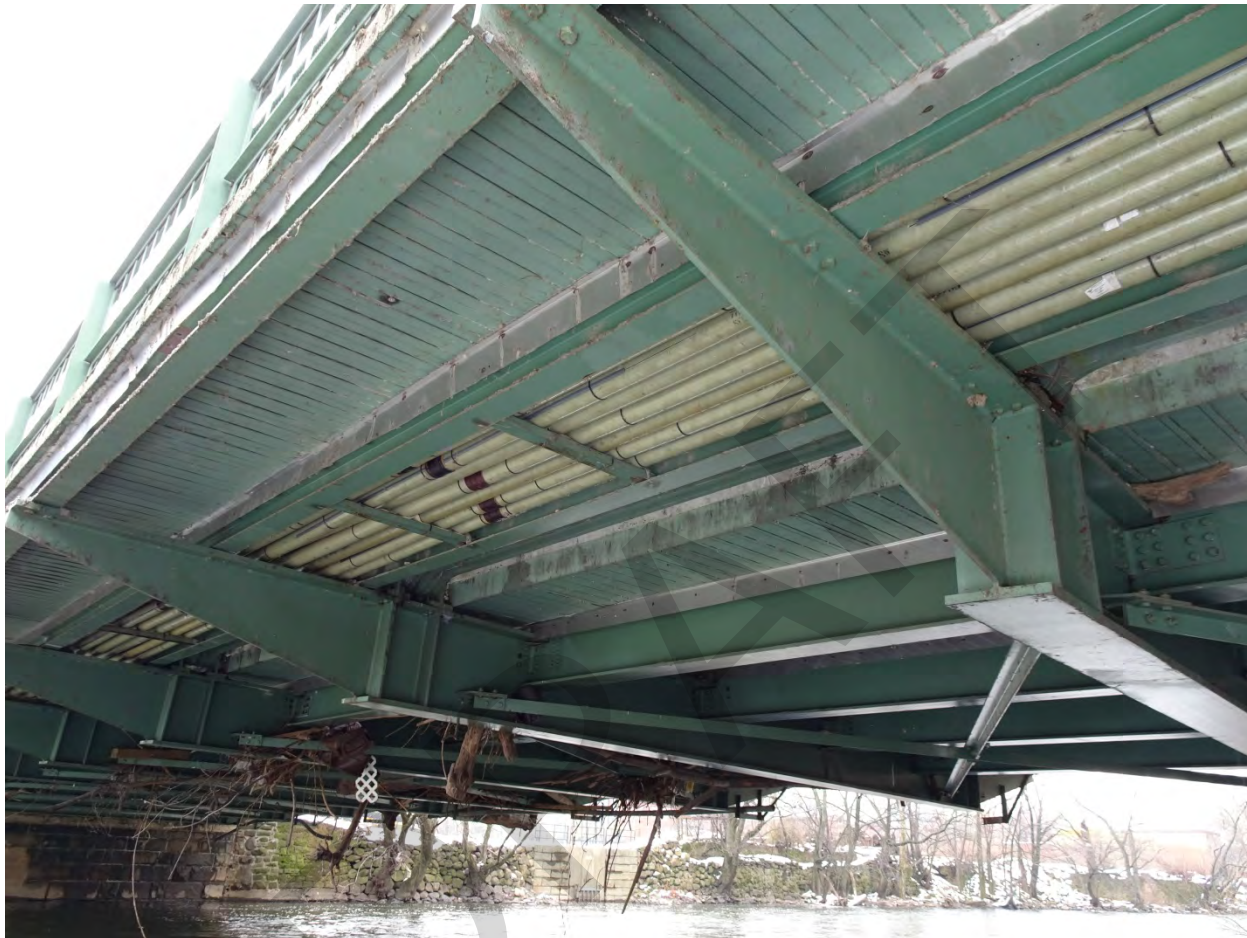
Photograph 13. View of the rehabbed floorbeam and stringer system and the debris caught in the substructure of the bridge, view south.
