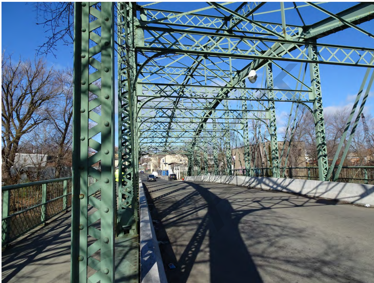
Photograph 12. View of the deck showing alterations such as a new decking and concrete Jersey barriers, view northwest.
