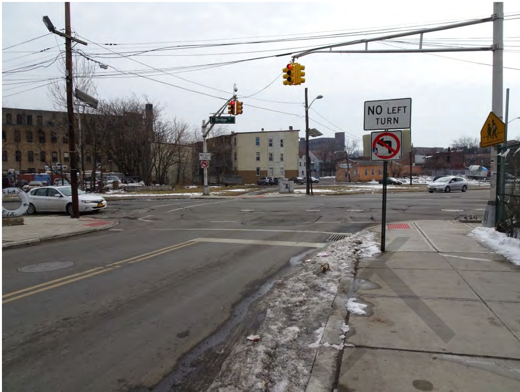
Arch Street Bridge over the Passaic River, City of Paterson, Passaic County Photo #3
