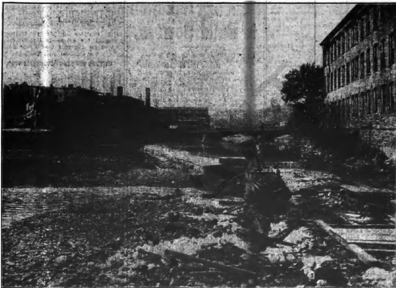
Figure 5. View southwest from the collapsed Arch Street Bridge in July 1905. The riverbed of the Passaic is seen dried out and littered with debris of all the collapsed bridges – almost two years after the Flood of 1903.
