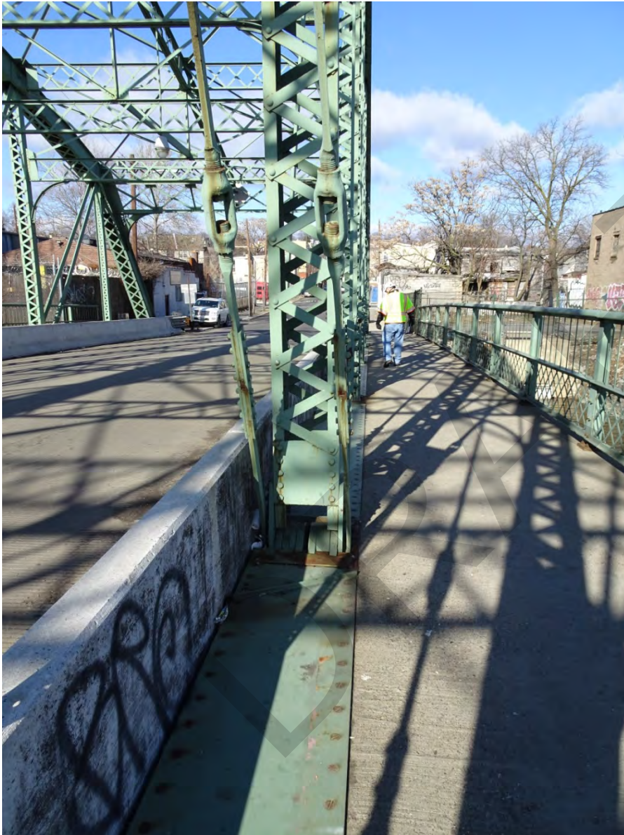
Photograph 11. View of the northern pedestrian walkway, view northwest.
