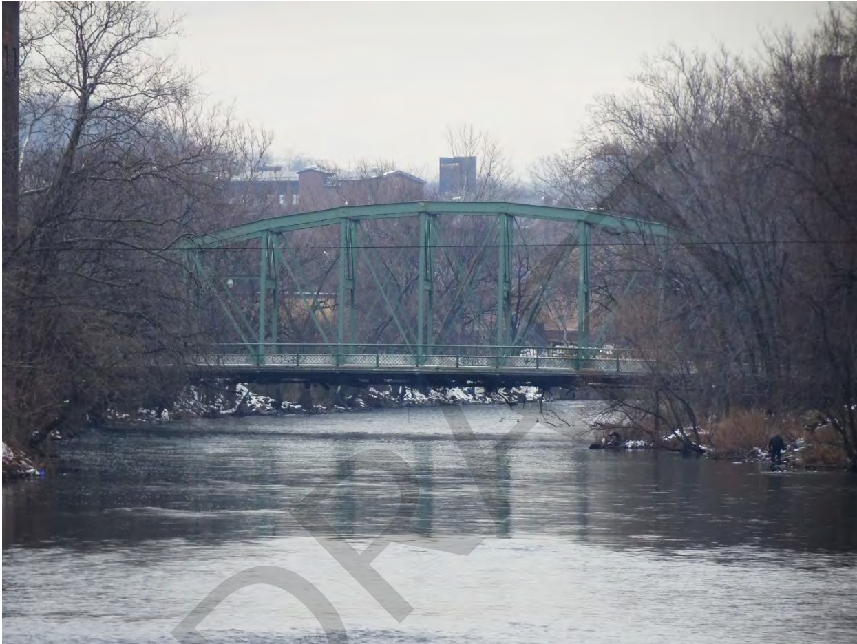
Photograph 6. Contextual view of the bridge from Straight Street Bridge, view southwest.
