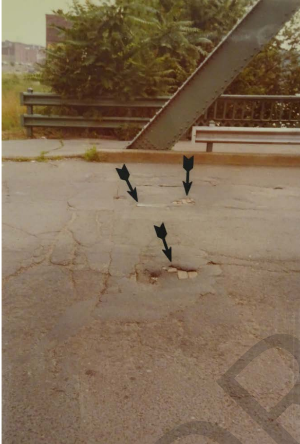
Figures 10, 11. Conditions of the bridge in 1979 during the first Bridge Inspection Report. Left: potholes in the road expose original vitrified brick deck material and trolley tracks visible beyond the patching. Right: Pedestrian walkway prior to rehabilitation. Note that the visibility of the verticals prior to the replacement of guardrails with jersey barriers.
