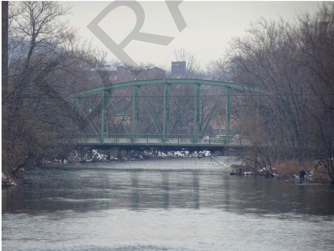
Arch Street Bridge over the Passaic River, City of Paterson, Passaic County Photo #6
