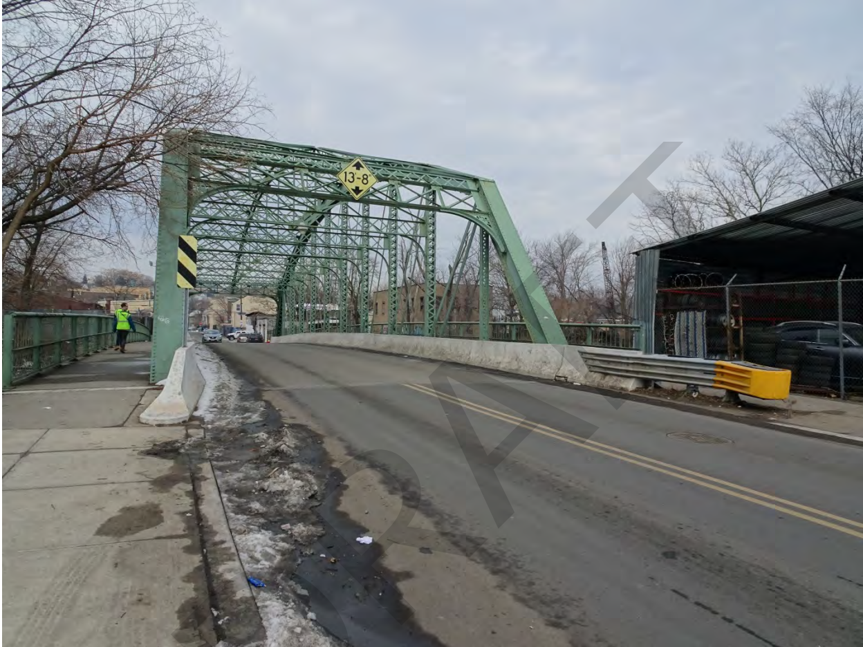
Photograph 2. Bridge approach from the north abutment, view southeast.
