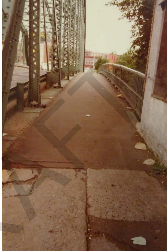
Figures 10, 11. Conditions of the bridge in 1979 during the first Bridge Inspection Report. Left: potholes in the road expose original vitrified brick deck material and trolley tracks visible beyond the patching. Right: Pedestrian walkway prior to rehabilitation. Note that the visibility of the verticals prior to the replacement of guardrails with jersey barriers.
