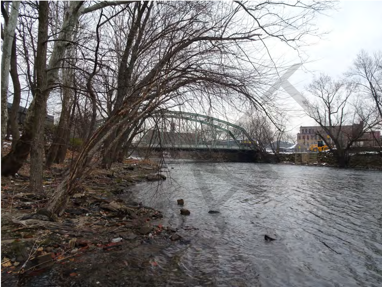
Photograph 15. Contextual view of the bridge from the banks of the Passaic River, view northeast.
