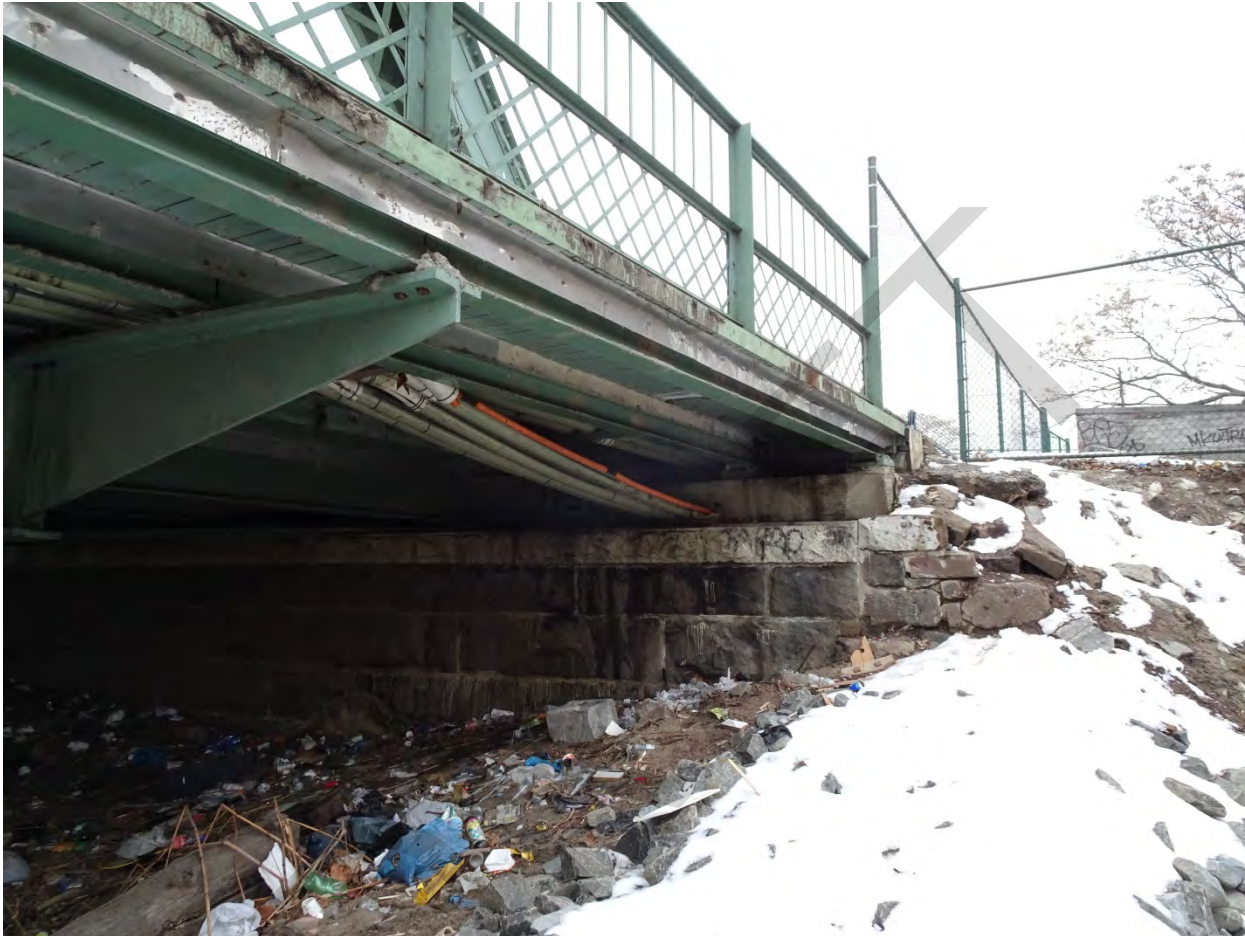
Photograph 4. North abutment, view northwest.
