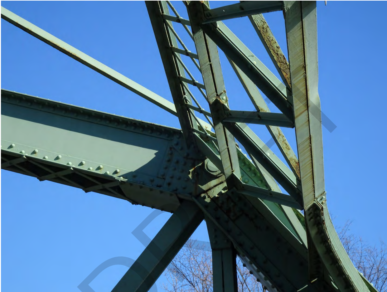
Photograph 9. Detail view of pinned connection, view southwest.
