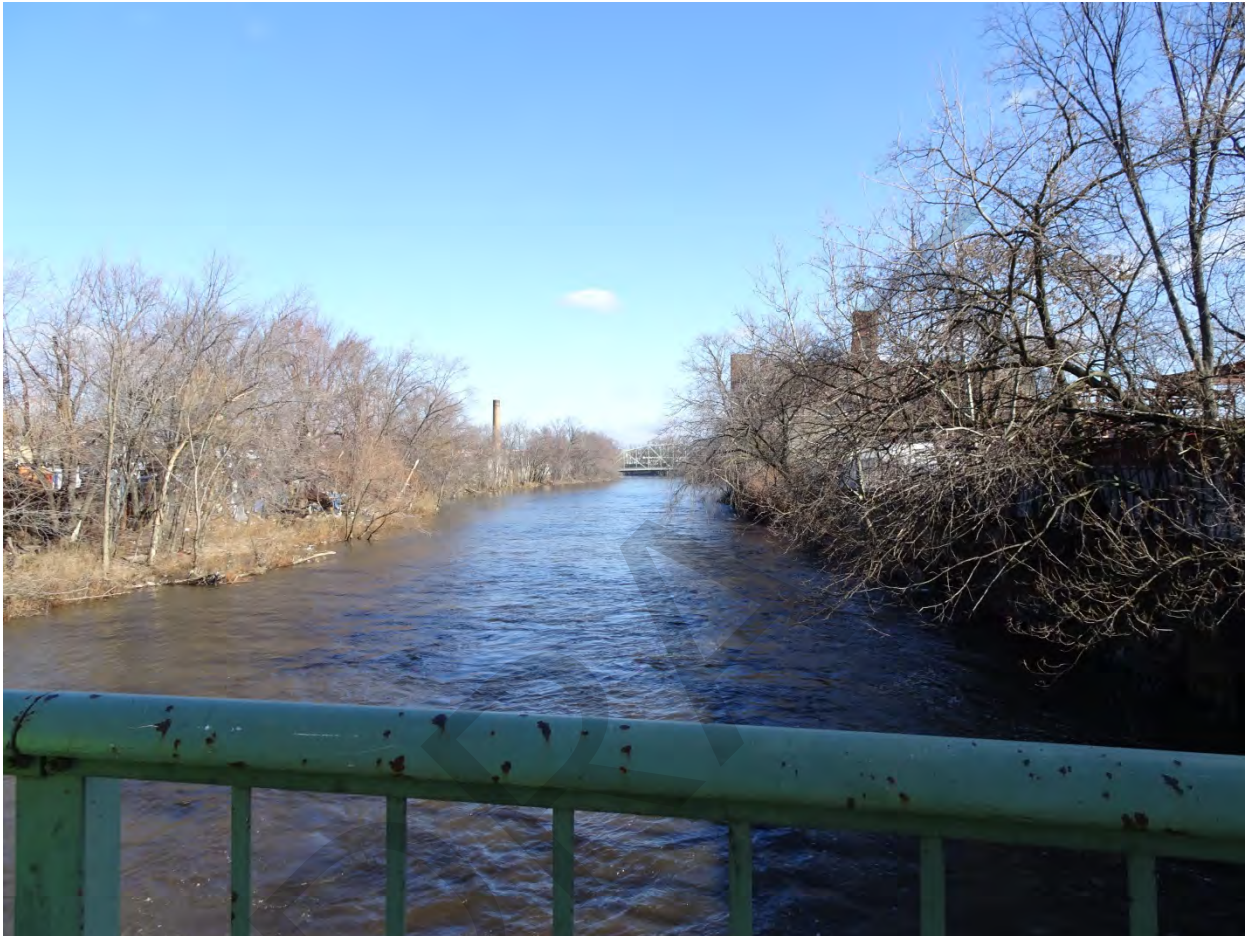
Photograph 14. Facing the Straight Street Bridge upstream, view northeast.
