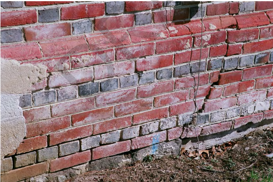
Figure 22 Banding, below the water table.
