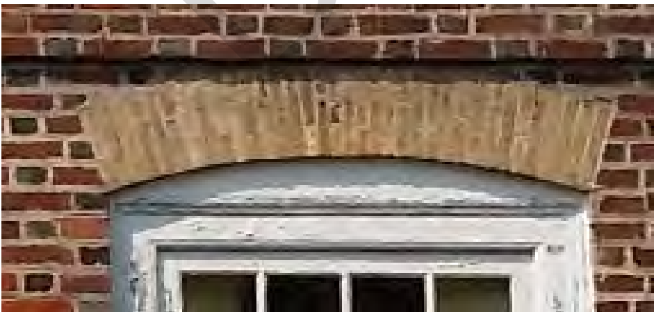
Figure 16 Off-white bricks, rubbed and gauged in a relieving arch.
