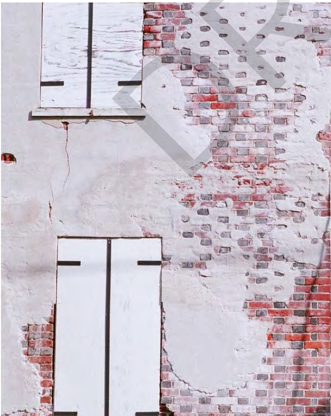
Figure 37 Stucco eroding away...
