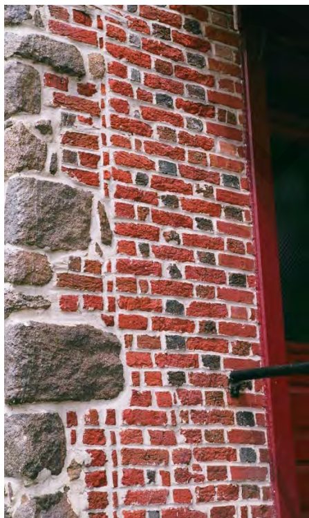
Figure 10 Mount Holly, NJ. Local stone was combined with patterned brickwork in some buildings.
