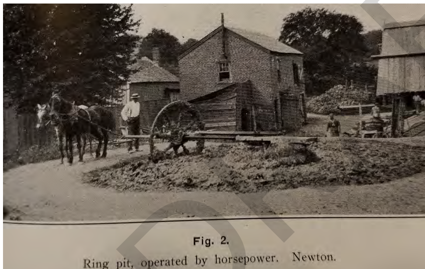
Figure 4 The same technology, still in use in a small, NJ brick operation, ca.1900.
