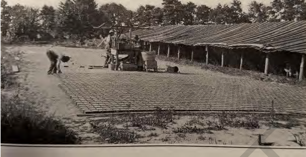
Figure 5 Laying the raw brick to dry, NJ, ca.1900. Note the drying shed in the background.
