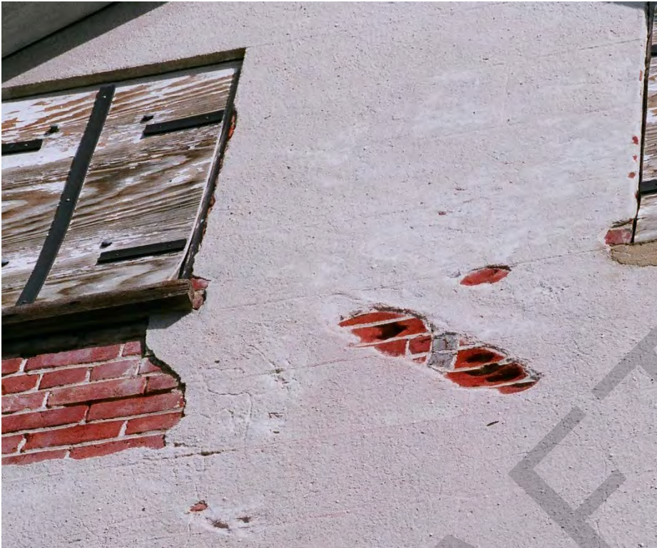
Figure 38 Stucco spalling, slowly revealing a date.
