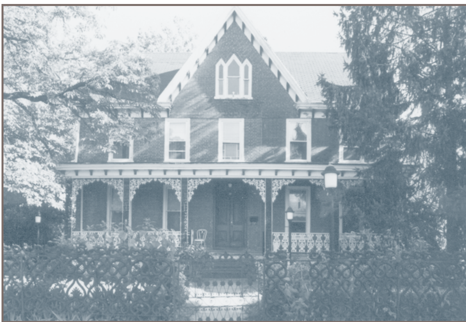
The historic Rulon House undergoing rehabilitation.
