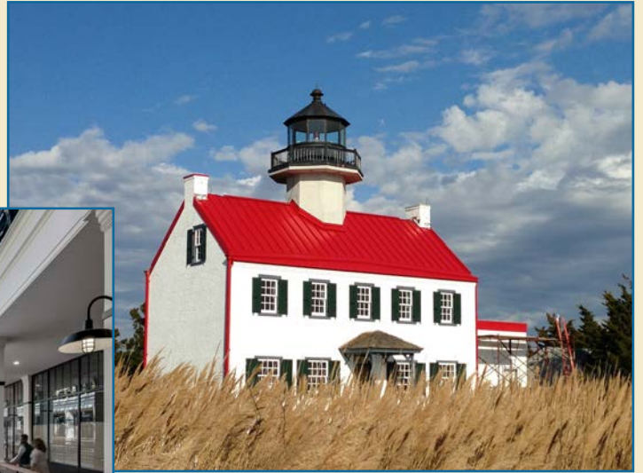
East Point Lighthouse, Maurice River Township, Cumberland County, Photo Credit: HPO staff
