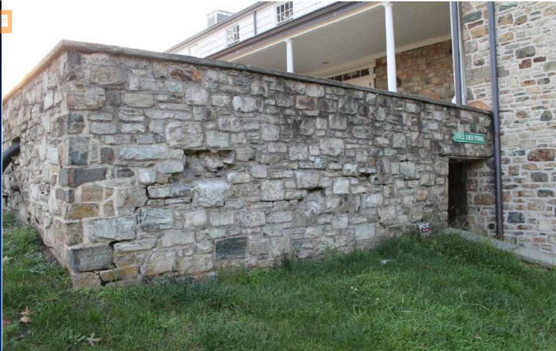
Deteriorating Terrace Wall, c. 2012
