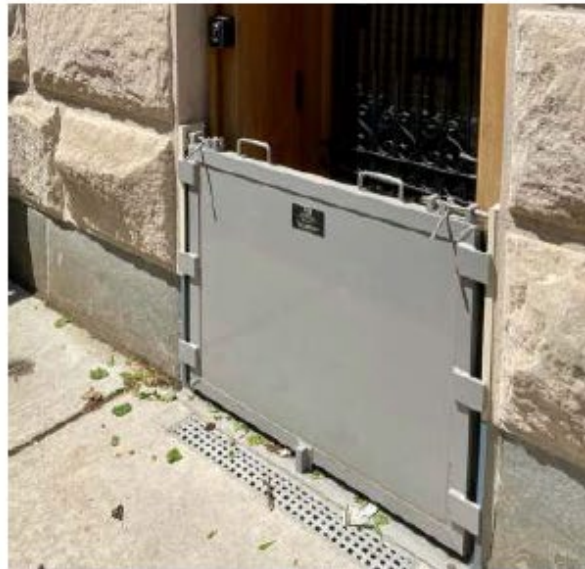
Temporary flood barriers should be attached to plain masonry and not impact character-defining elements
