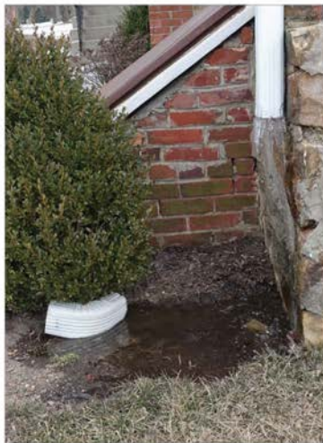
A key component of maintenance to reduce potential flood damage is to ensure that stormwater collected by gutters and downspouts flows away from a building rather than pooling adjacent to the foundation or support systems.
