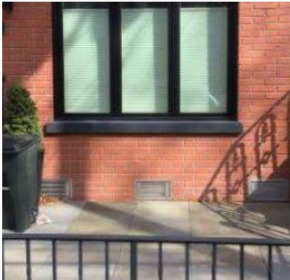
Engineered hydrostatic relief vents, a component of wet floodproofing, should be inconspicuously located
