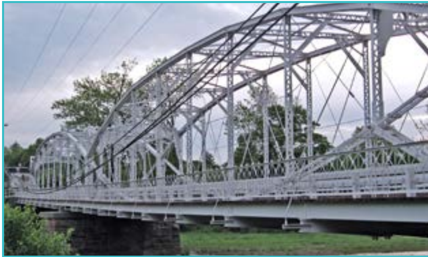
Elm Street Bridge, Neshanic Station, Somerset County.
