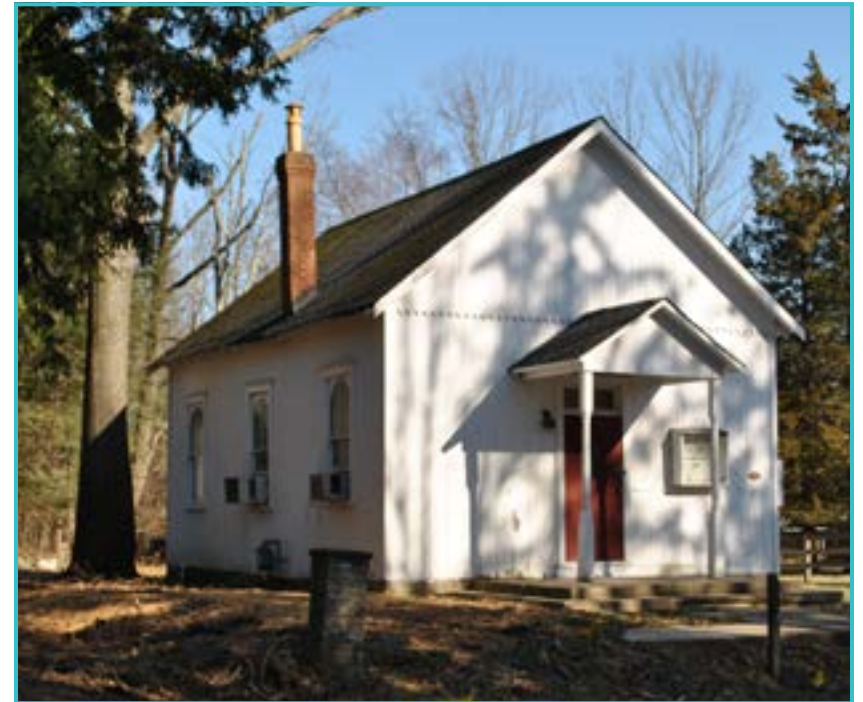
Mount Zion African Methodist Episcopal Church, Montgomery Township, Somerset County.
