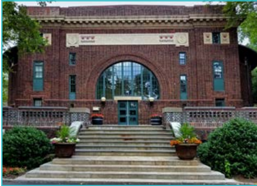
Walker Gymnasium, Hoboken, Hudson County.
