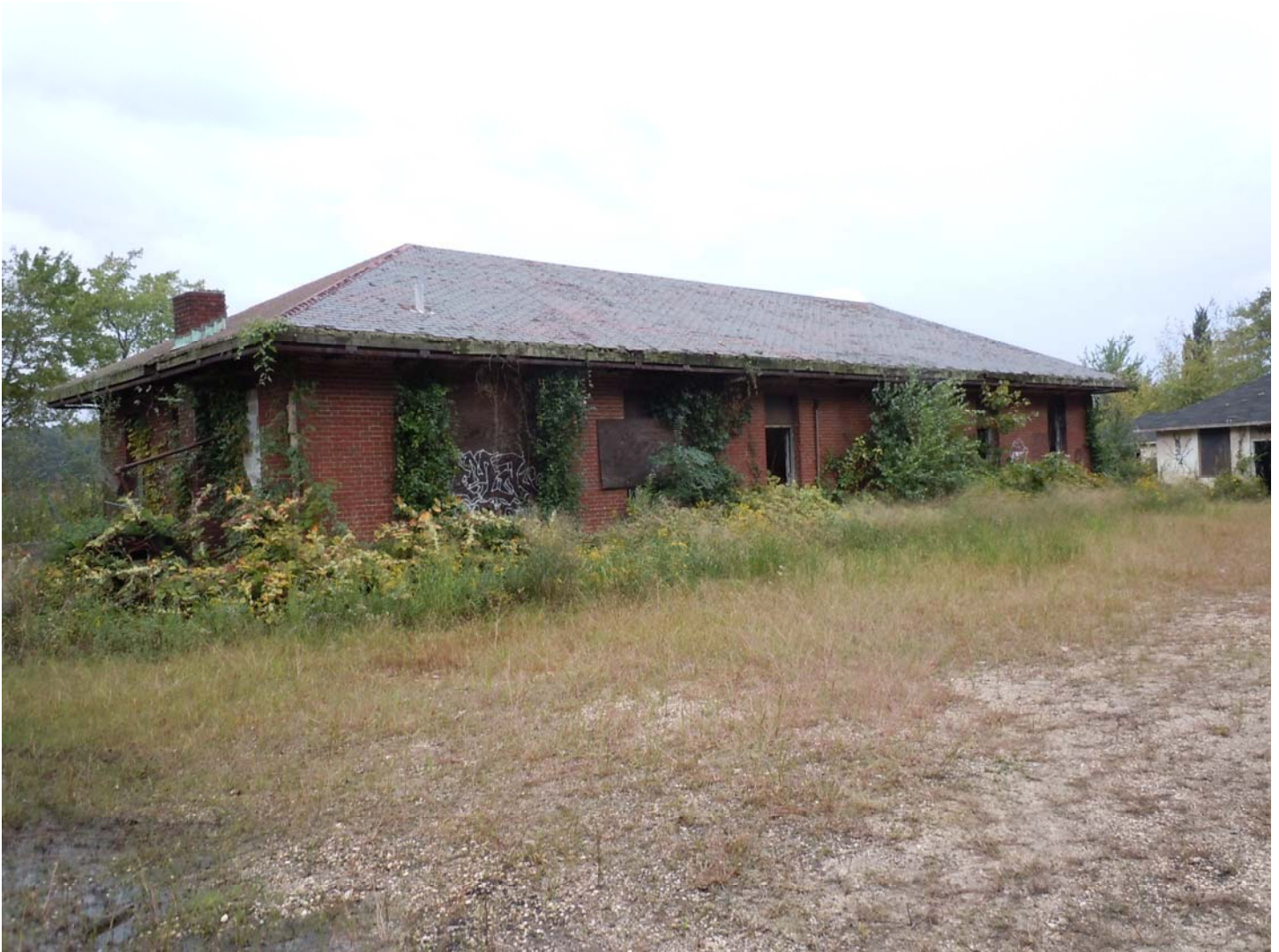
Photograph #4 Operations Building, #9004 (1914); north and west elevation. Robie S. Lange, September 29, 2011
