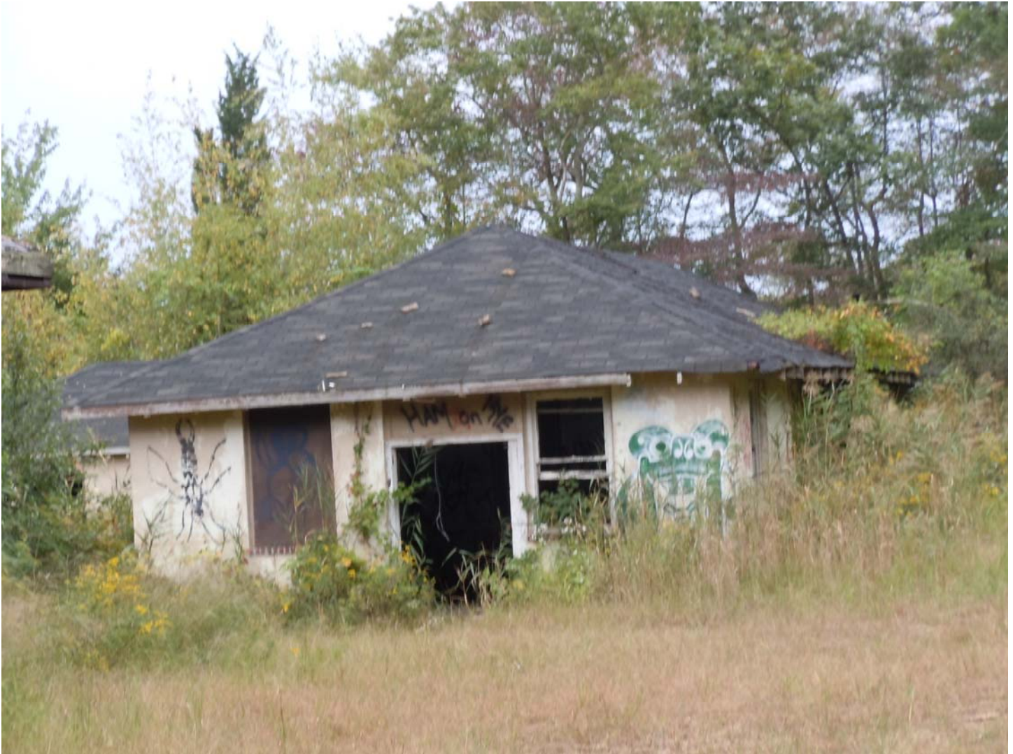
Photograph #5 Operations Annex, #9005 (ca. 1917); north elevation. Robie S. Lange, September 29, 2011
