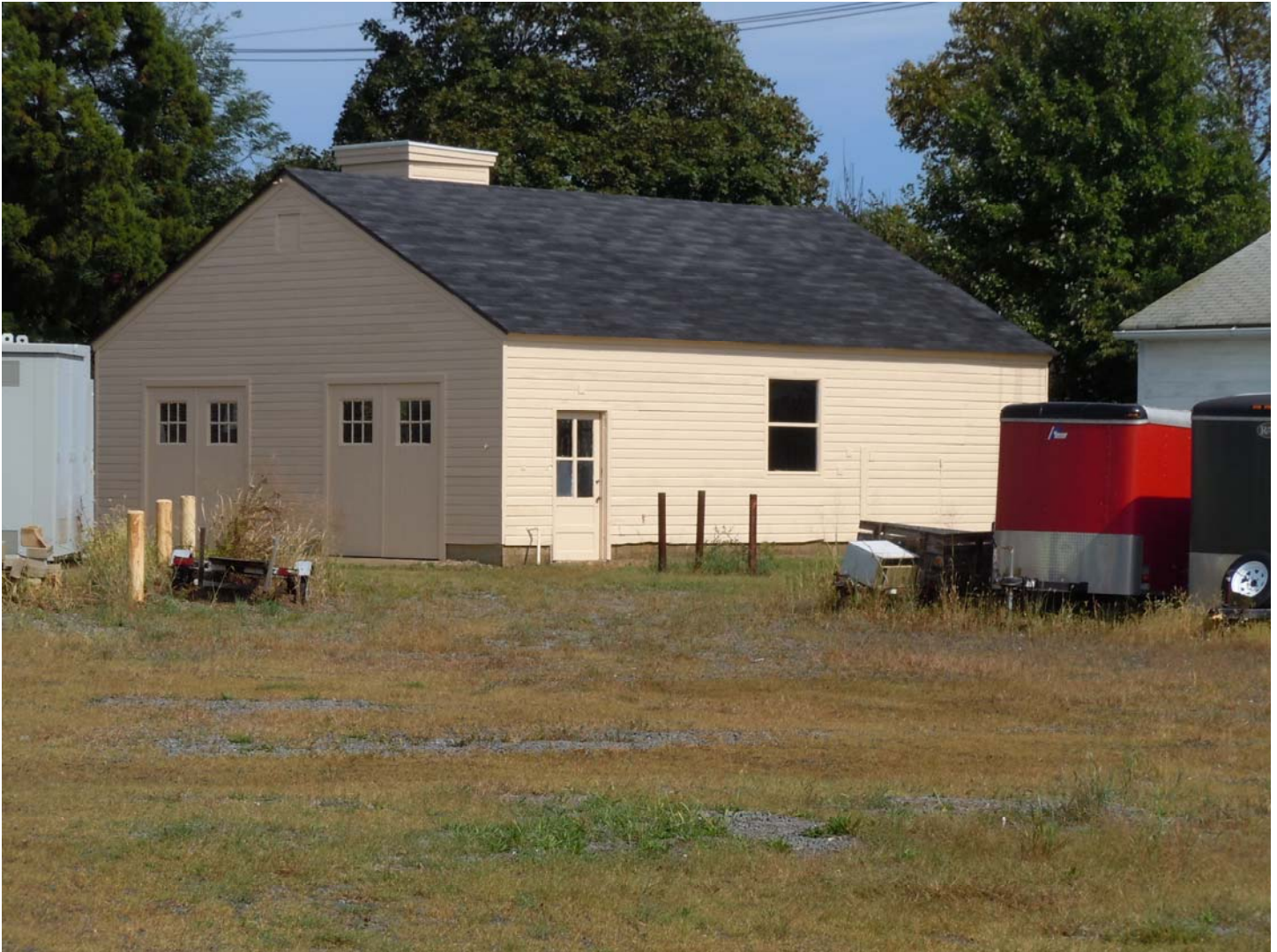
Photograph #16 Garage, #9057 (1942); northwest and southwest elevations. Robie S. Lange, September 29, 2011
