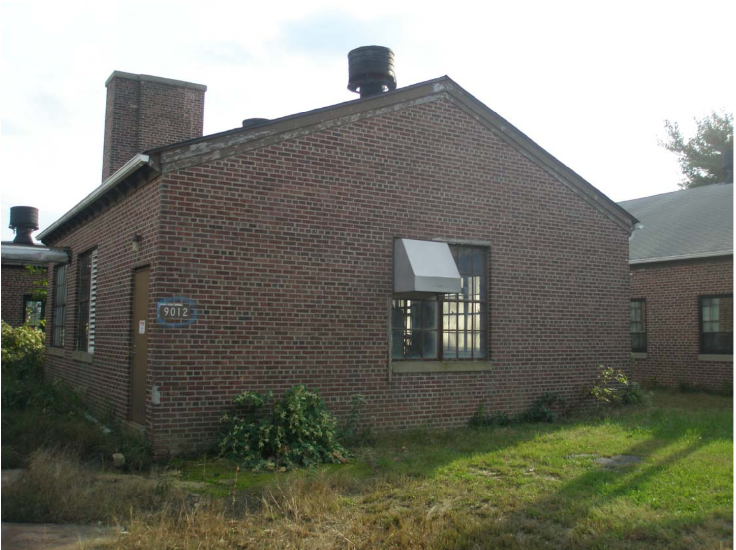
Photograph #11 Heat Plant, #9012 (1942), east and north elevations. Fred Carl, October 18, 2011
