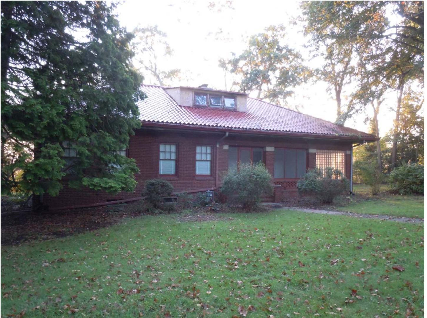
Photograph #2 Manager's Cottage, #9002 (1914); west elevation. Robie S. Lange, September 30, 2011
