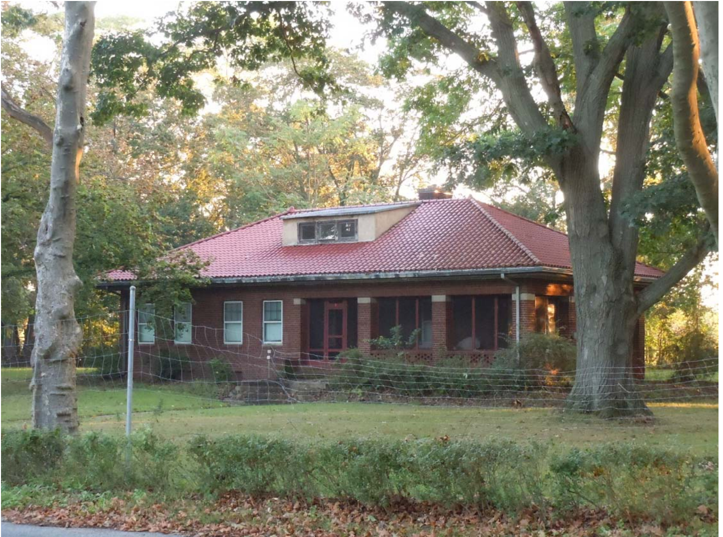
Photograph #3 Chief Engineer's Cottage, #9003 (1914); west elevation. Robie S. Lange, September 30, 2011
