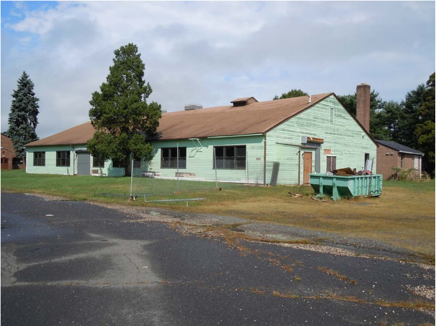
Photograph #15 Electric Shop, #9034 (1942-1943); west and south elevations. Robie S. Lange, September 29, 2011
