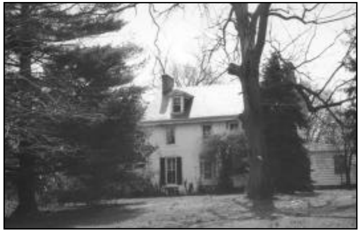
Above: North facade (1950's kitchen later demolished)
