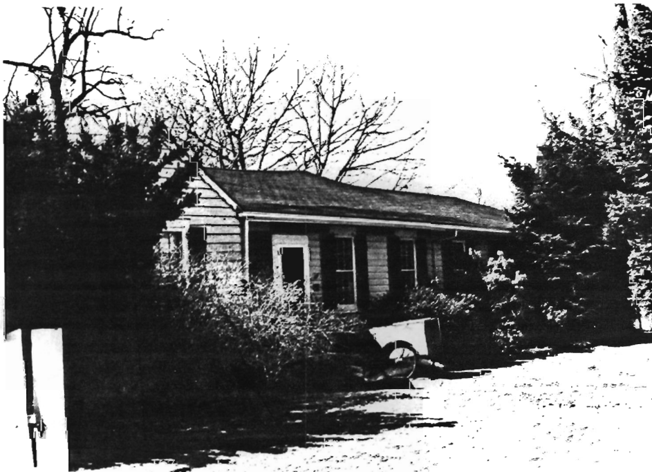
Rear addition, view to NW.
