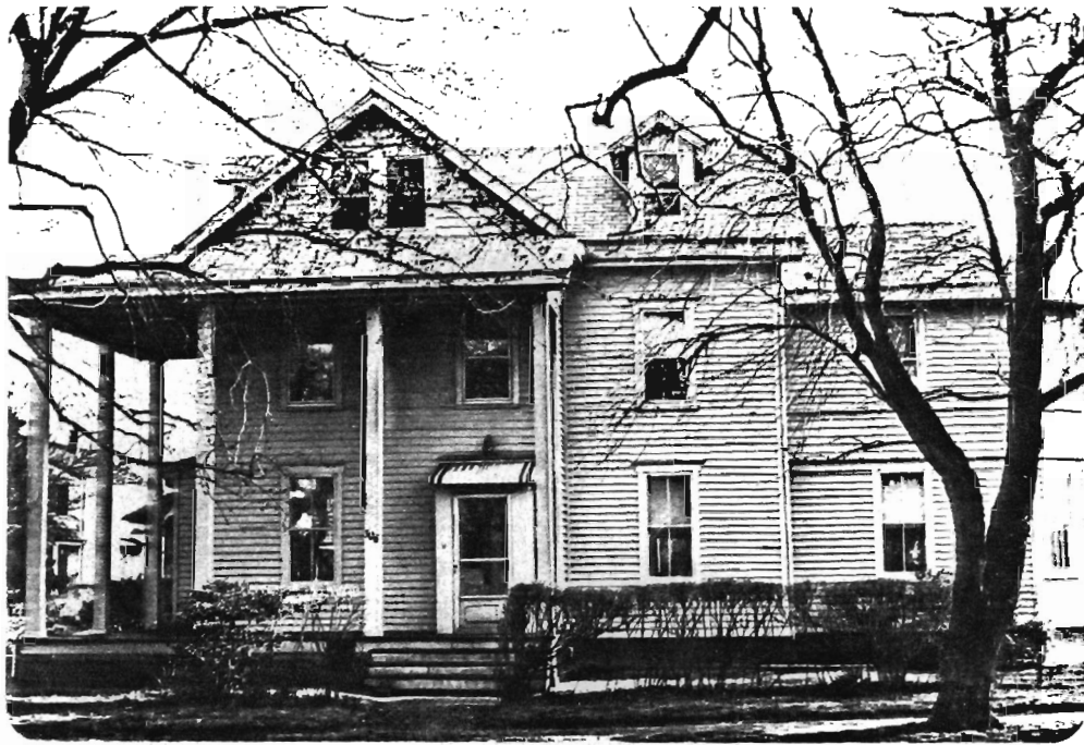
1306-13. 306 River Avenue. Block 22, Lot 7. Neg. File No. 1-17, 18. Vernacular Victorian house, 1880's. Complex plan; intersecting gable roof; interior end chimney; brick foundation; clapboard and wood shingle siding; 2/2 sash windows; 2 story porch with square posts. Projecting bay on the west end was added between 1890 and 1905.
