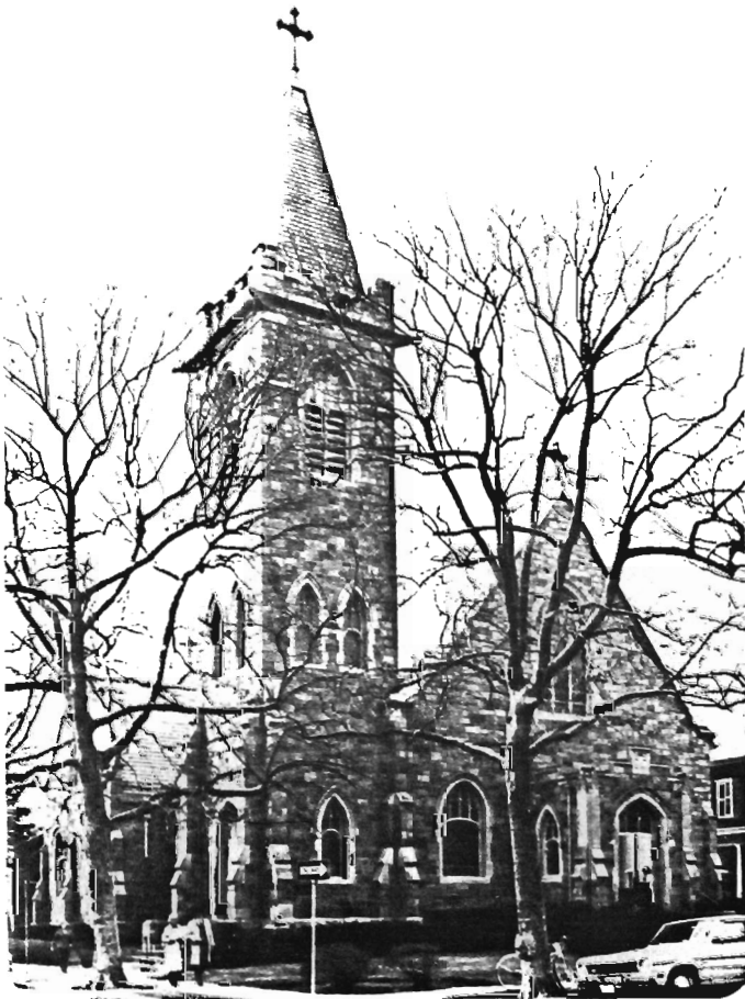
1306-15. 603 Seventh Avenue. Block 75, Lot 1. Neg. File No. 2-22, 23, 24. St. Roses's Catholic Church, 1926. Late Gothic Revival building, cruciform in plan with square tower on NE corner and ell on SW corner. Brick construction with stone facing (rock-faced, random-coursed) and limestone trim. Gable roof; 60' pyramidal spire; pointed-arch windows with tracery. Congregation organized in 1888; wooden church built in 1890. Convent, school, and rec- tory also on site.
