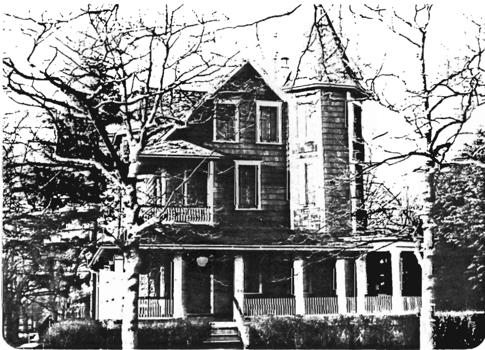
1306-2. 318 Eleventh Avenue. Block 102, Lot 10. Neg. File No. 1-34, 35. Vernacular Victorian house, 1880's, with 2½ story Picturesque plan; multiple intersecting gable roof and 3 story tent-roofed turret; brick foundation; wood shingle siding; porch on three sides with square posts; balcony on SW corner; 2/2 sash windows (shuttered for the winter); and double-hung door.
