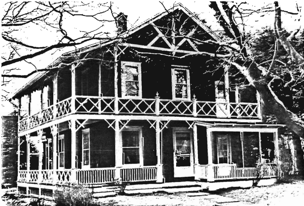
1306-17. 601 Sixth Avenue. Block 65, Lot 1. Neg. File No. 2-19, 20, 21. Vernacular Victorian house with Stick Style elements, c. 1880. 2½ story 3 bay by 3 bay plan with two-tiered porch on two sides. Gable roof; center ridge chimney; brick foundation; natural wood shingle siding; 1/1 sash windows with small cornices; Stick Style gable bracket and porch trim. Appears to have been altered (one bay added) on the west end. E.A. Braddock owner on 1889 atlas.
