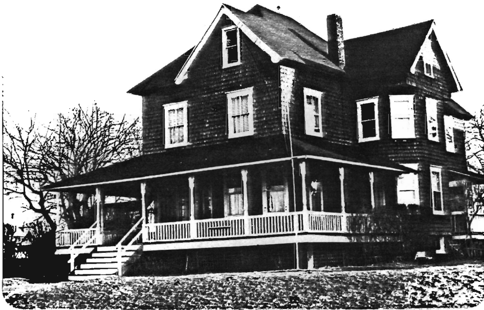
1306-18. 207 South Lake Drive. Block 61, Lot 2. Neg. File No. 1-30. Vernacular Victorian house, c. 1895. 2½ story complex plan with porch on three sides. Hip roof with intersecting gables and vergeboard; interior end chimney; brick foundation; natural wood shingle siding; 2/2 sash windows; multiple projecting bays; brackets and turned posts on porch.
