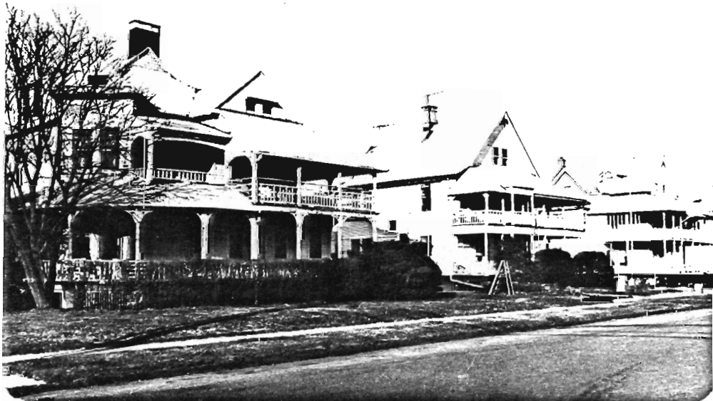
1306-14. 108, 110, and 112 Second Avenue. Block 10, Lots 6, 7, and 8. Neg. File No 1-7 through 12. Three Queen Anne summer "cottages," 1880's. 2½ stories with complex plans, multiple gable roofs, ridge chimneys, clapboard and shingle siding. Two-tiered porches with slender posts and latticed balustrades; double-hung sash windows of various sizes. Owned by Est. of I. Henderson (#108 and #110) and H. Hall (#112) on 1889 county atlas.
