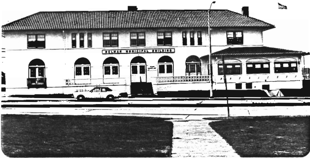
1306-1. SE corner Eighth Avenue and State Highway 35. Block 87, Lot 1. Neg. File No. 2-9, 10. American Legion Home, 1925. Now Belmar Municipal Building. 2 story stucco-faced brick Mission Style building constructed on a rectangular plan with an enclosed porch on the west end. Mission tile hipped roof with interior chimneys; symmetrical fenestration with paired 6/6 sash windows, narrow 4/4 sash, and double-hung doors with round-arch fanlights and hoodmolds.
