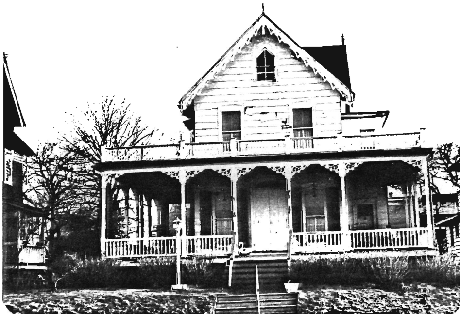
1306-19. 209 South Lake Drive. Block 61, Lot 3. Neg. File No. 1-31, 32. Vernacular Victorian house with Carpenter Gothic elements, c. 1890. 2½ story L-plan with veranda on three sides. Intersecting gable roof with finials and vergeboard; brick foundation; asbestos shingle siding (20th c. alteration). Symmetrically arranged 2/2 sash windows with segmental heads; full-length windows on first story; triangular-headed gable window; projecting bay on east side. Veranda has slender posts and balusters, and scroll brackets. Double door with elliptical transom.
