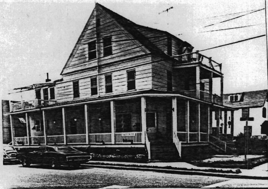
Tillson's / Lakeview Inn, 101 Bridge Avenue
