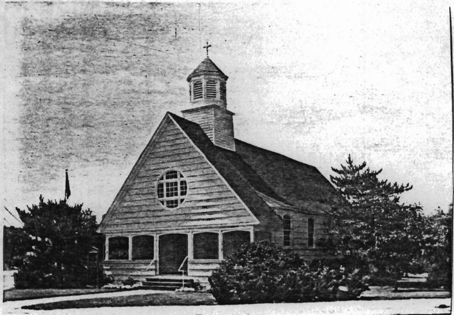
The Bay Head Chapel, Southwest corner, Bridge and Main Avenue
