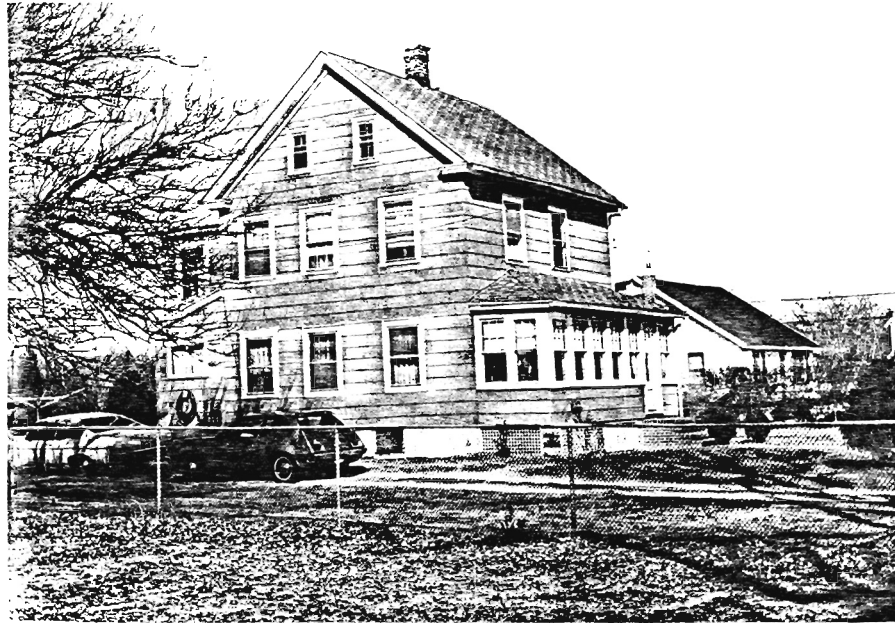
J.C. Johnson House / 2 West Street / Block 14 / Lot 3 West Creek
