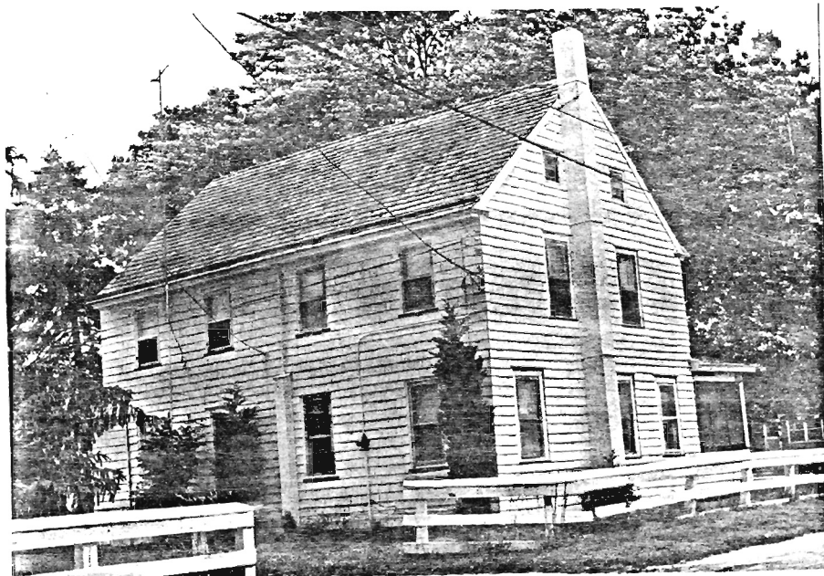
Shinn Farmhouse / Homestead Avenue / Block 22 / Lot 2 & 3 West Creek
