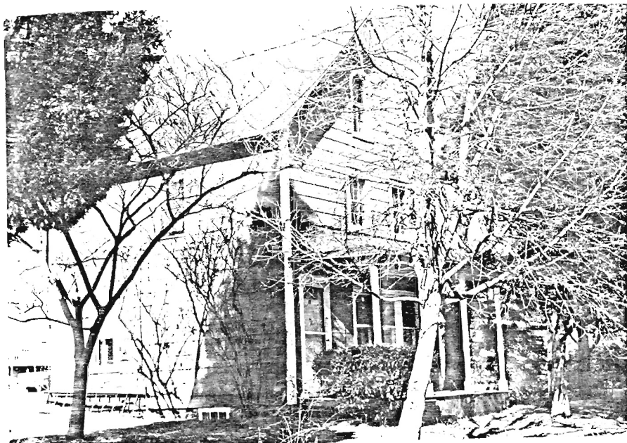
A.T. Willets House / Main Street / Block 16 / Lot 1 West Creek
