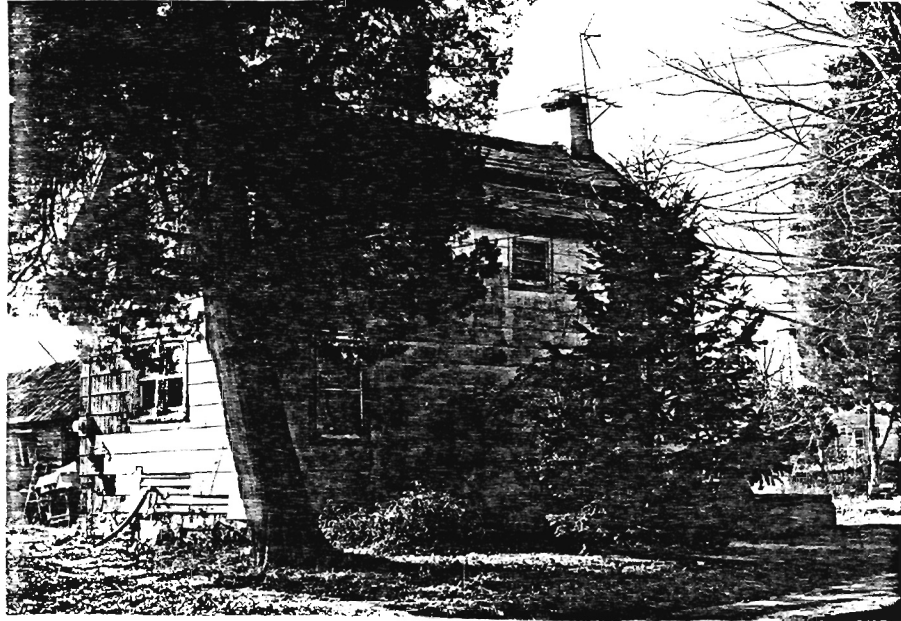
R.T. Pharo House / Mill Road / Block 22 / Lot 6 West Creek
