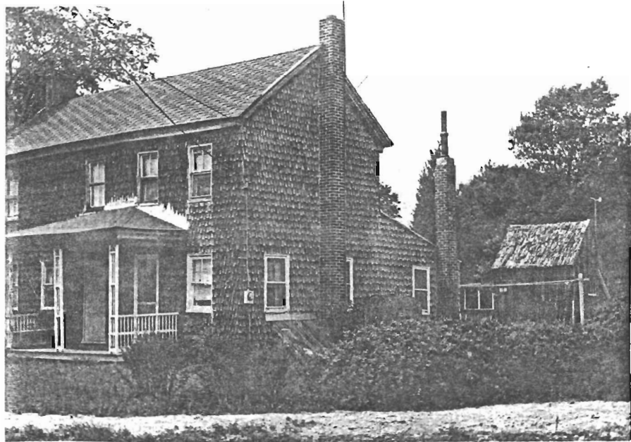
Center Street at southwest corner of Gale Road
