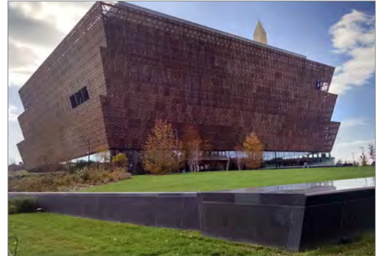
Flood wall (black granite, foreground) forms a perimeter barrier surrounding the National Museum of African American History and Culture and protects the museum from flooding by the Potomac River. Washington, DC.
