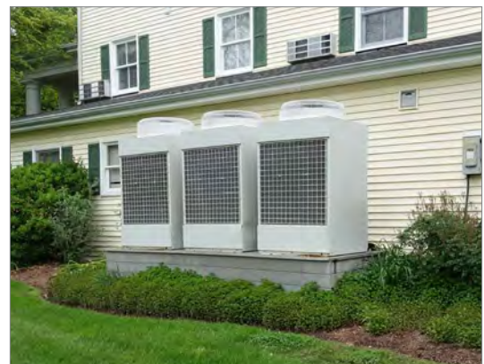
Elevating building systems and equipment can reduce damage from rising water and expedite repairs following a flood event. Appropriate screening is recommended.
