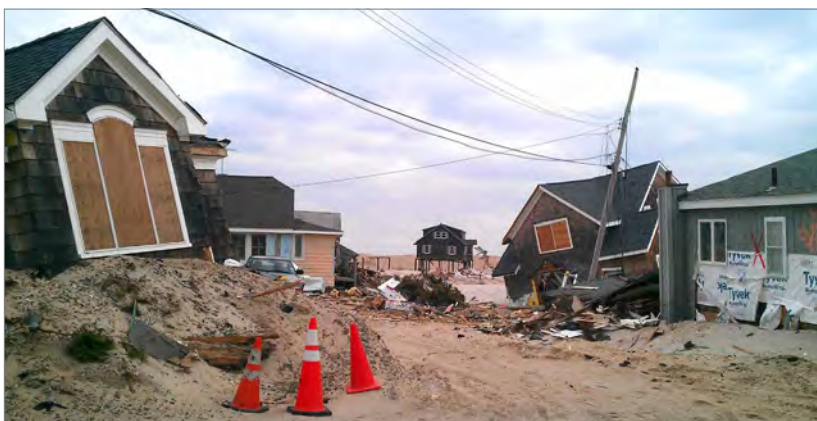
Building codes can be modified to require strong connections between the building and foundation to prevent shifting in flood waters. (Photograph courtesy of the NJ HPO.)
