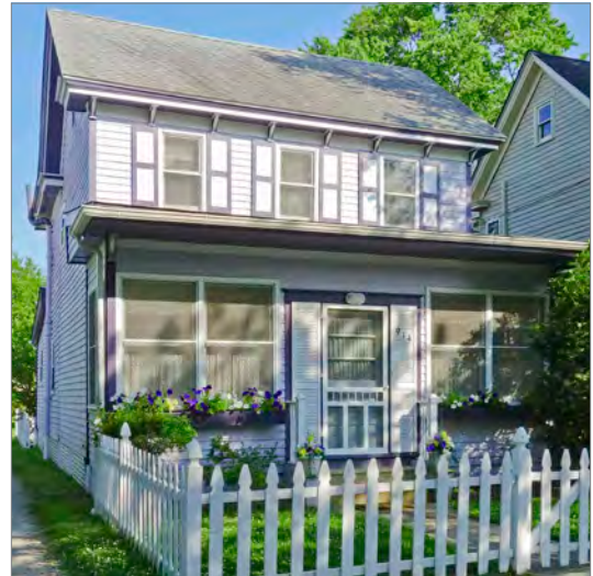
Buildings constructed prior to the issuance of Flood Insurance Rate Maps are referred to as pre-FIRM and are often vulnerable to flood damage if located within the Special Flood Hazard Area (SFHA).
