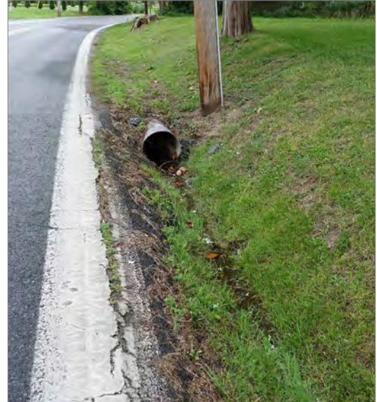
Drainage ditches are depressed channels, often located adjacent to roadways, that remove stormwater from land surfaces. When constructed of natural materials, they can promote stormwater absorption.
