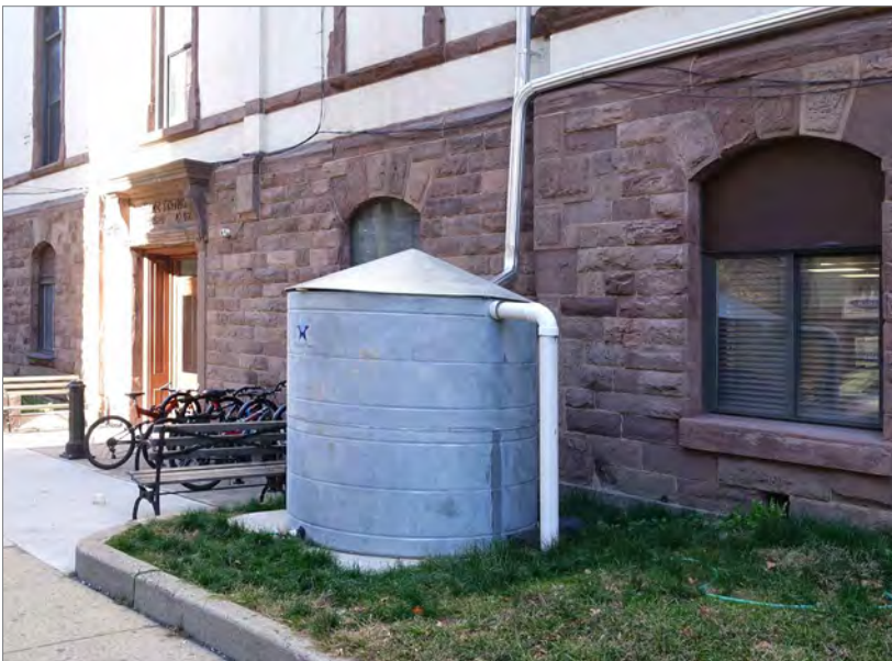
Although typically scaled for residential use, larger buildings can also harvest storm water in rain barrels.
