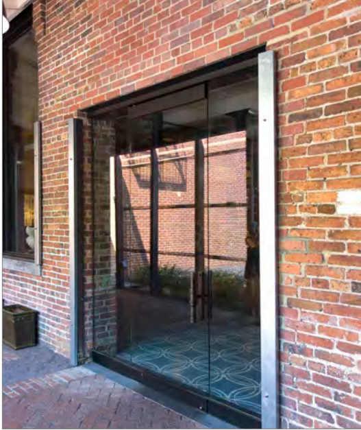
Window and door barriers and shields for dry floodproofing are generally inserted into pre-installed channels flanking window and door openings. They must be individually labelled and stored onsite in a convenient location, and installed by trained personnel immediately preceding a flood event.
