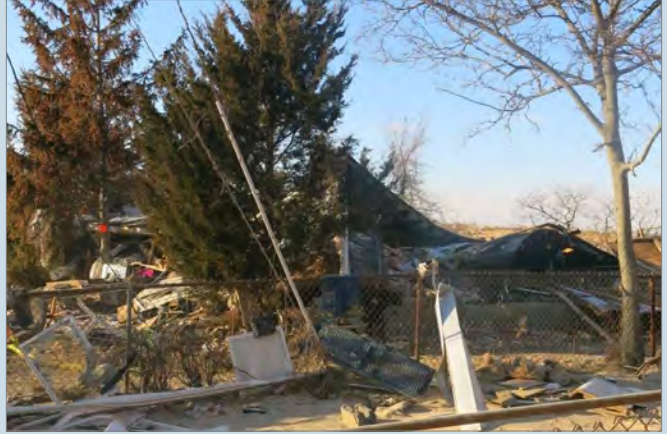
Criteria A: This building in old Bridge, Middlesex County is rubble. (Photography courtesy of the NJ HPO.)
