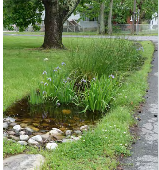
Rain gardens can limit stormwater runoff from a property onto roadways and into municipal stormwater management systems. Utilizing native plants further promotes absorption and minimizes required maintenance.
