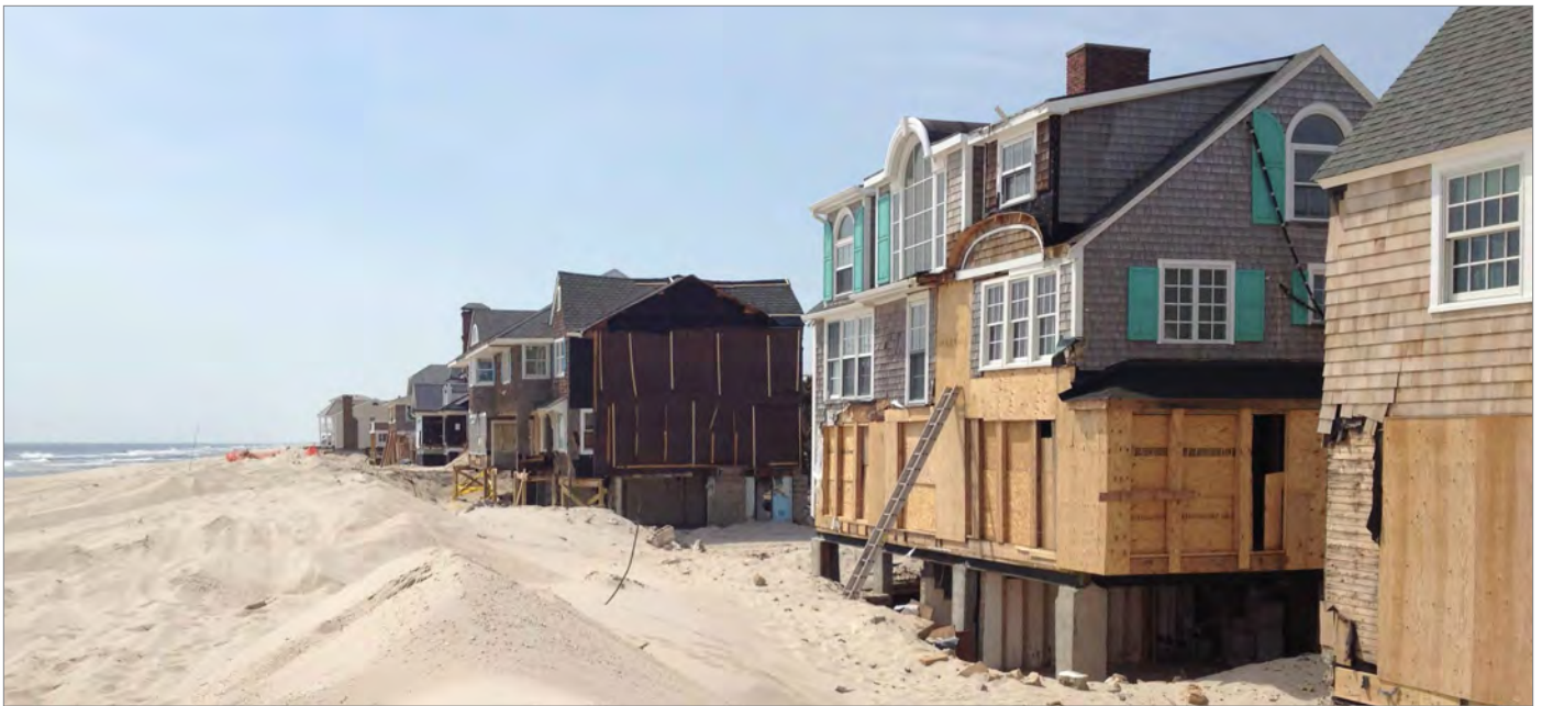
Property mitigation strategies should balance individual building protection with a strategy that maintains a sense of place. (Photograph courtesy of the NJ HPO.)
