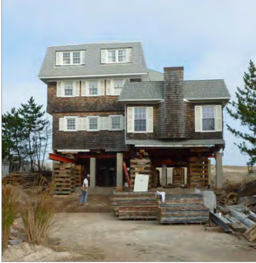
Elevation is a mitigation measure that is accepted by the National Flood Insurance Program for residential buildings. (Photograph courtesy of the NJ HPO.)
