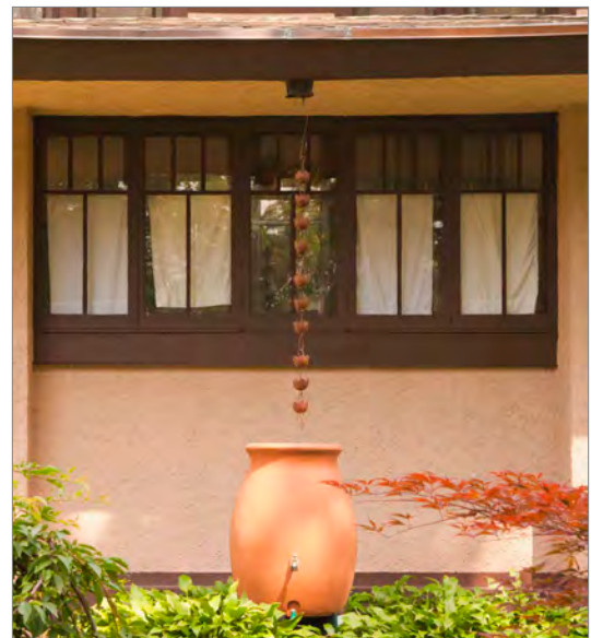
Rain barrels can collect stormwater discharge from roof surfaces and be used to water gardens.
