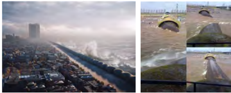
Figure 1a: Our visualisation of a pneumatic storm surge barrier positioned along the Rockaway Peninsula (NYC) and b the inflation of the Ramspl Bagstuw between two lakes (clockwise image credit maritiemnieuws.nl)
