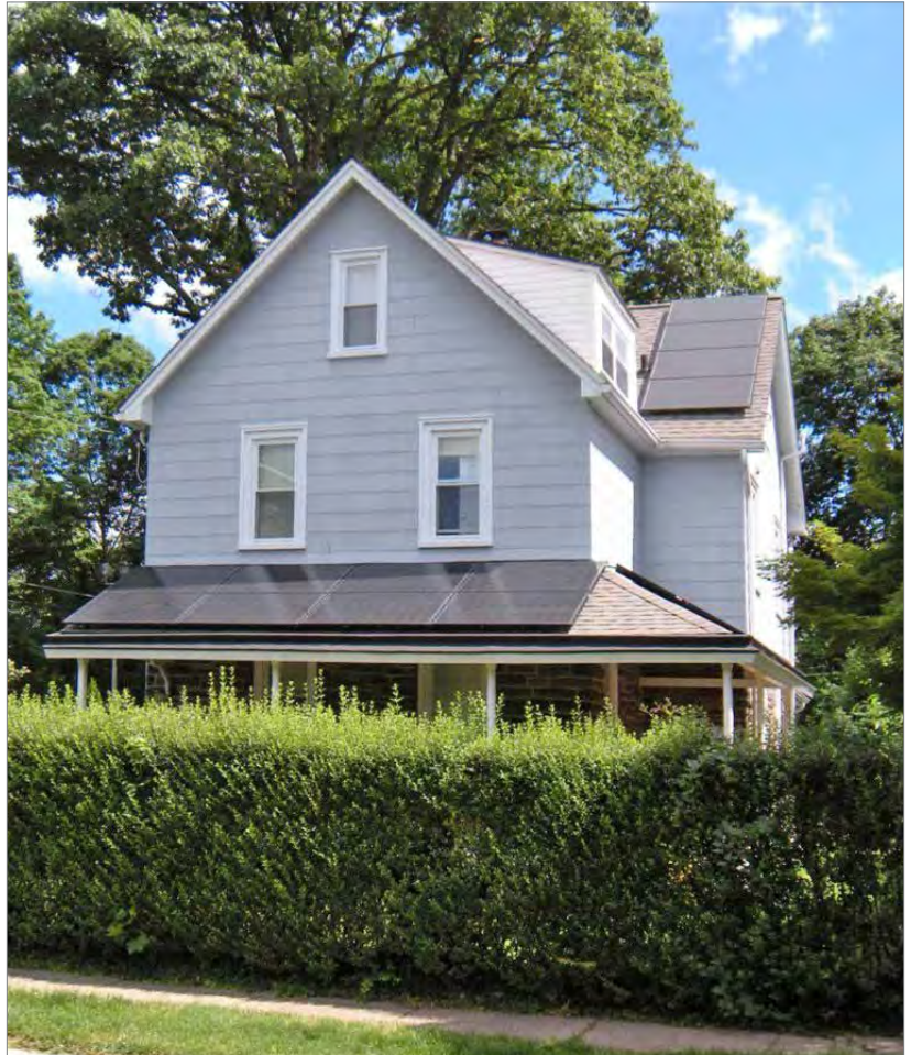
Secondary power sources, such as solar panels, can facilitate recovery from a flood, although their installation may be limited by HPCs, particularly on principal façades. However, locations for their efficacy may limit available options in some circumstances. The visual impact of solar panels can be mitigated with placement on secondary elevations; installation parallel to the roof surface; selecting a frameless panel that matches the roof color; and maintaining a consistent minimum offset of 6-inches from eaves, rakes, and ridges.
