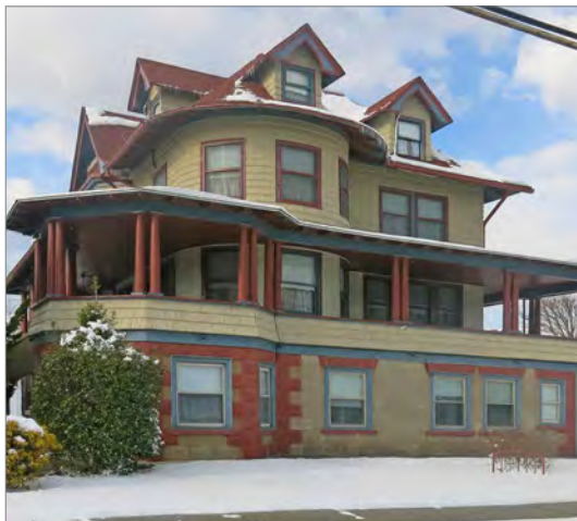
The design of the raised, closed foundation is compatible with the historic house. The colors, fenestration pattern, quoins, and window surrounds relate to the architectural detail on the upper floors. (Photograph courtesy of NJ HPO/FEMA.)
