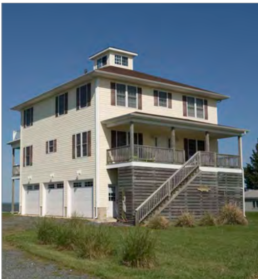
Extreme elevations to accommodate parking can greatly impact a building's relationship to the ground and should be avoided. Horizontal board foundation screening is rarely appropriate for historic buildings.
