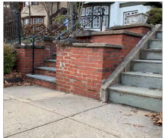
Masonry retaining walls can provide an effective grade transition for elevated sites and minimize storm water runoff onto adjacent parcels.
