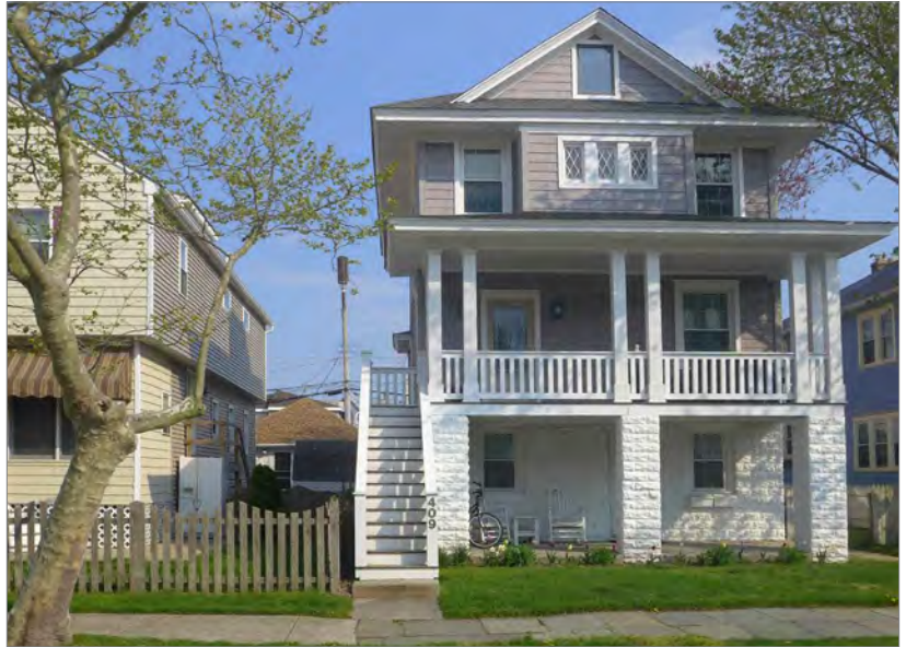
A straight-run stair would fit in the front yard, however, its placement in the side yard takes advantage of the porch depth and allows for a direct approach from the sidewalk. Side yard construction may be limited in some municipalities. (Photograph courtesy of NJ HPO/FEMA.)
