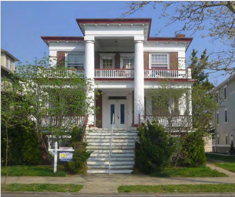
The wide, central stair is a significant compositional feature of this building, creating a prominent alignment for the composition. The side-yard driveway is visually a secondary access route. Evergreen shrubs provide year-round screening for elevated foundations. (Photograph courtesy of NJ HPO/FEMA.)
