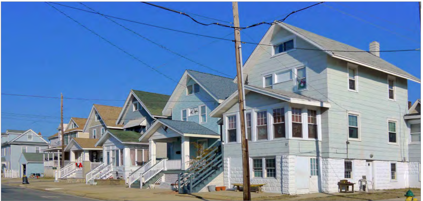
A consistent elevation height can help maintain a cohesive neighborhood character. (Photograph courtesy of NJ HPO/FEMA.)
