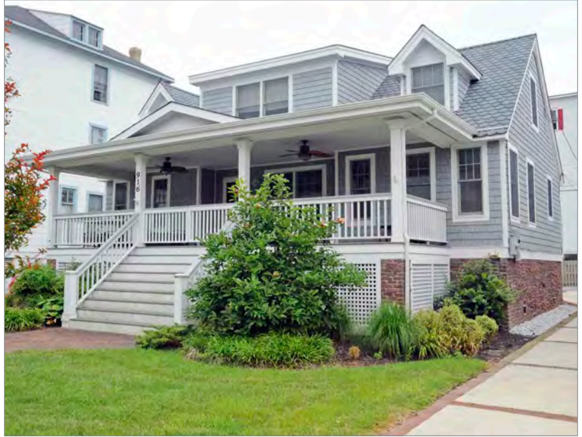
Square lattice provides foundation screening between the piers. The use of diagonal or square lattice should be appropriate for the building's style. The central stair maintains the orientation to the front door and the brick foundation of the house includes flood vents at the side elevation facing the driveway.
