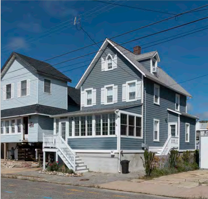
The Town of Beach Haven's HPC established protocols after Superstorm Sandy that addressed local floodplain management concerns while preserving the historic character of their community. This included establishing maximum building elevation heights relative to the local BFE.
