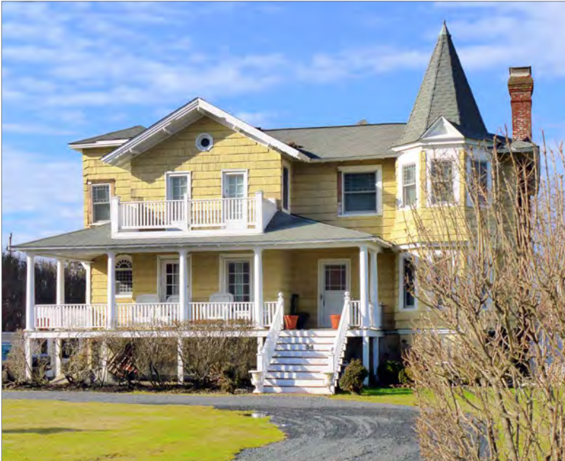
The house retains its highly decorative character-defining features including the tower, balcony, porch, windows, doors, chimney, and wood shingle cladding. The wide, prominent stair, maintains its frontal access and includes railings and newel posts that are similar to the balustrade. The porch piers are aligned with the columns above and partially obscured by shrubs. (Photograph courtesy of NJ HPO/FEMA.)
