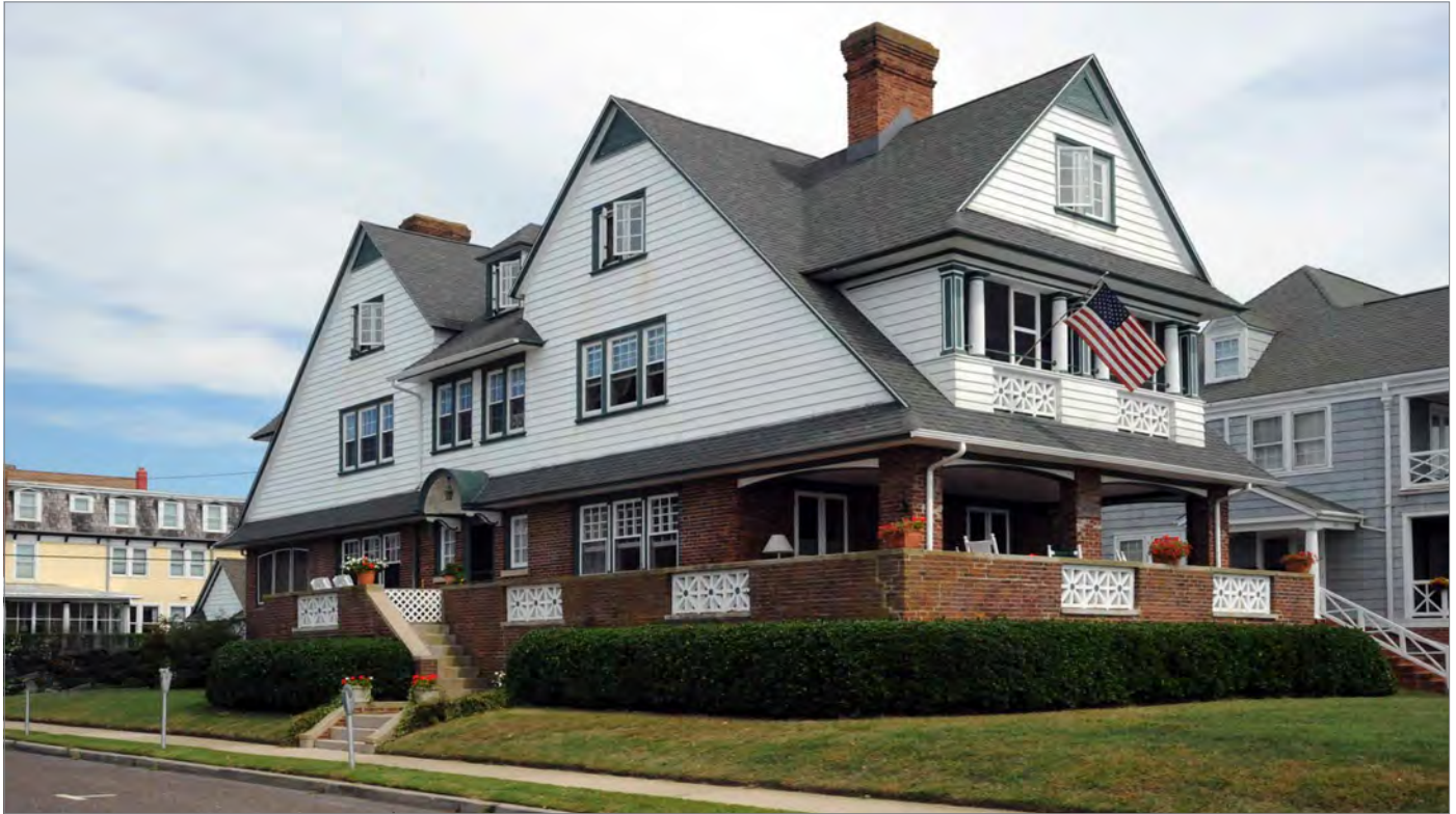
The parcel size allows the ground plane to be elevated above the street level and the house is supported on a raised brick foundation, elevating the first floor level well above the street level. The continuous evergreen shrubs obscure the raised foundation.
