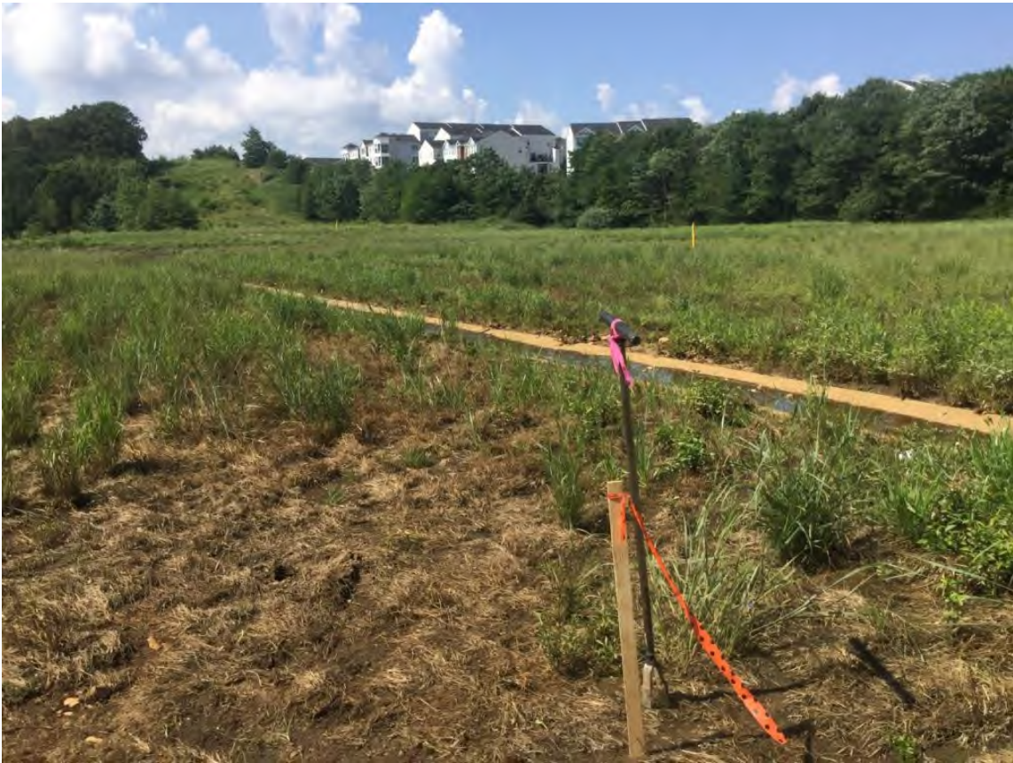
ID:W-T01-011A-1 Date:08/20/2016 Direction:W Position:Wetland Overview
