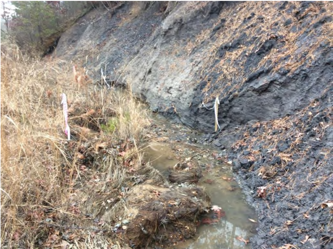
ID:WW-T15-004A Date:12/10/2016 Direction:SW Type:Intermittent Position:Downstream
