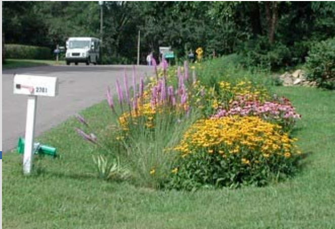
A swale converted to a rain garden.
