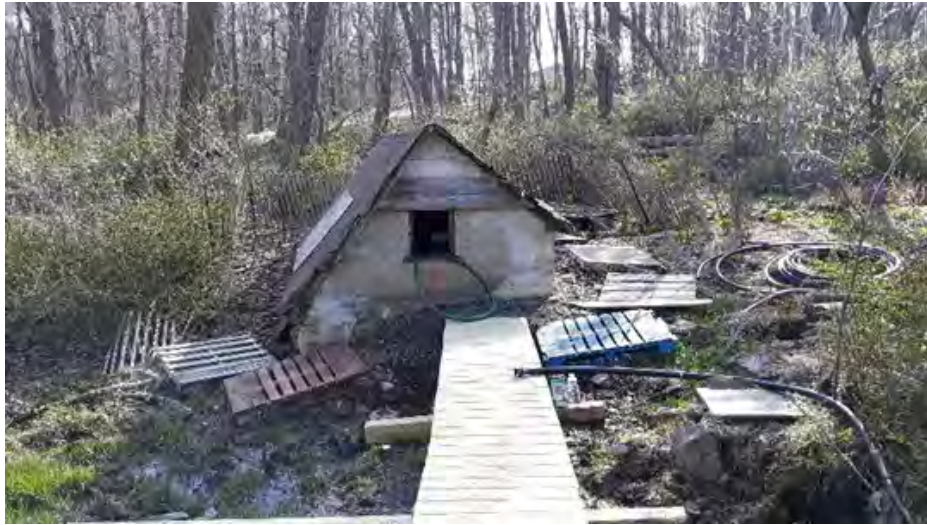
Figure A-67. Springhouse at Highlands Ridge Park. Photo, T. Pallis.
