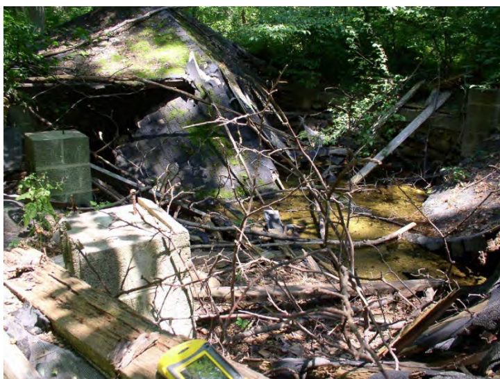
Figure A-32. The remains of a collapsed roof of the Kuser Mountain Spring springhouse. The cinderblock catch basin is still visible. Photo, W. Marzulli.
