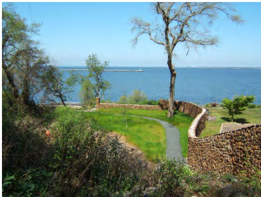
Figure A-45. Top left. View of the wall. Photo, S. Domber.
