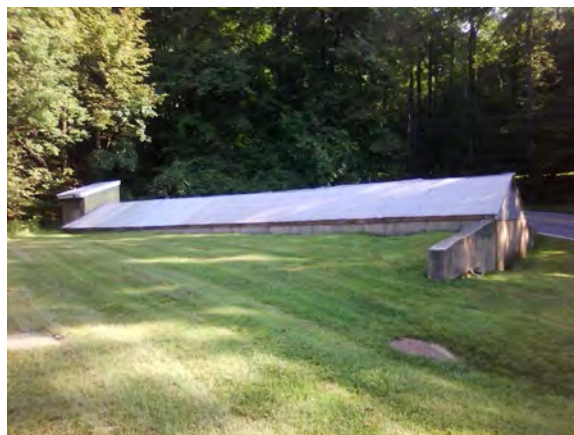
Figure A-74. Washington Township Municipal Utilities Authority water system, Schooley's Mountain water supply springhouse. Photo, T. Pallis.
