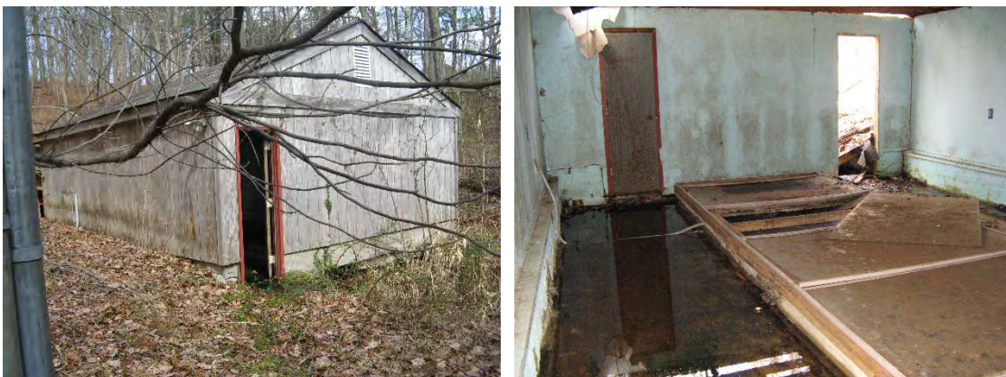
Figure A-50. Left, Indian Lady Hill Spring springhouse. Photo, T. Pallis, Figure A-51. Right, Inside Indian Lady Hill Spring springhouse. Photo, S. Domber.
