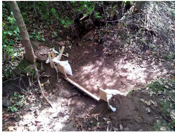
Figure 14. Weir being constructed when Brau Kettle was dry. Photo, T. Pallis.
