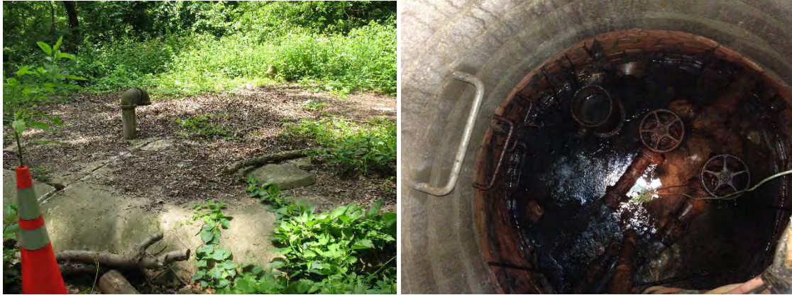
Figure A-5. Left. Surface view of source area of the Great Bear/Trinity Spring cement basin. Photo, T. Pallis.
