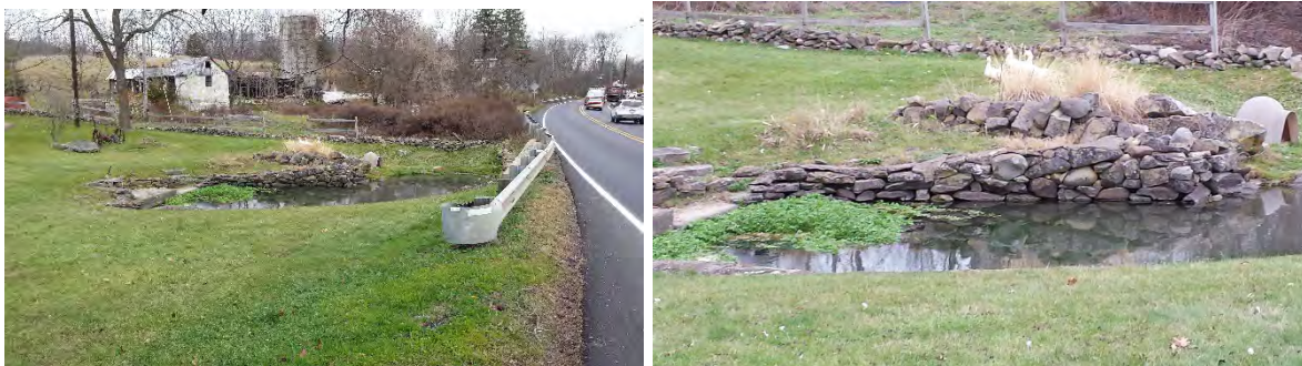
Figure A-93. Left, Big Springs (North Church) along Route 94. Photo, T. Pallis.
