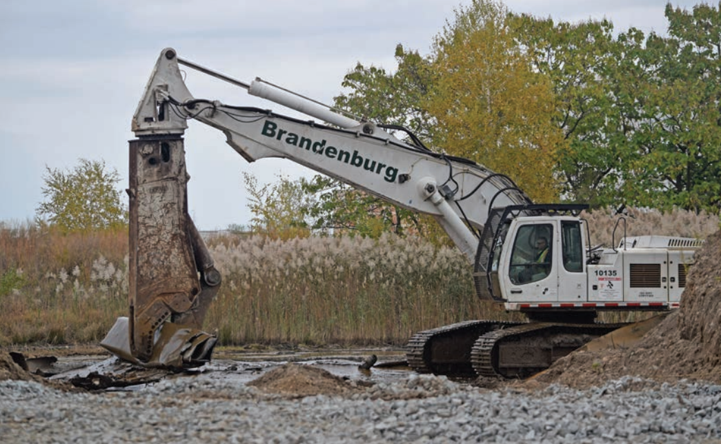
Demolition Contractor at Work. CITGO hired demolition contractor Brandenburg who made quick work of removing all vestiges of the old tank field.
