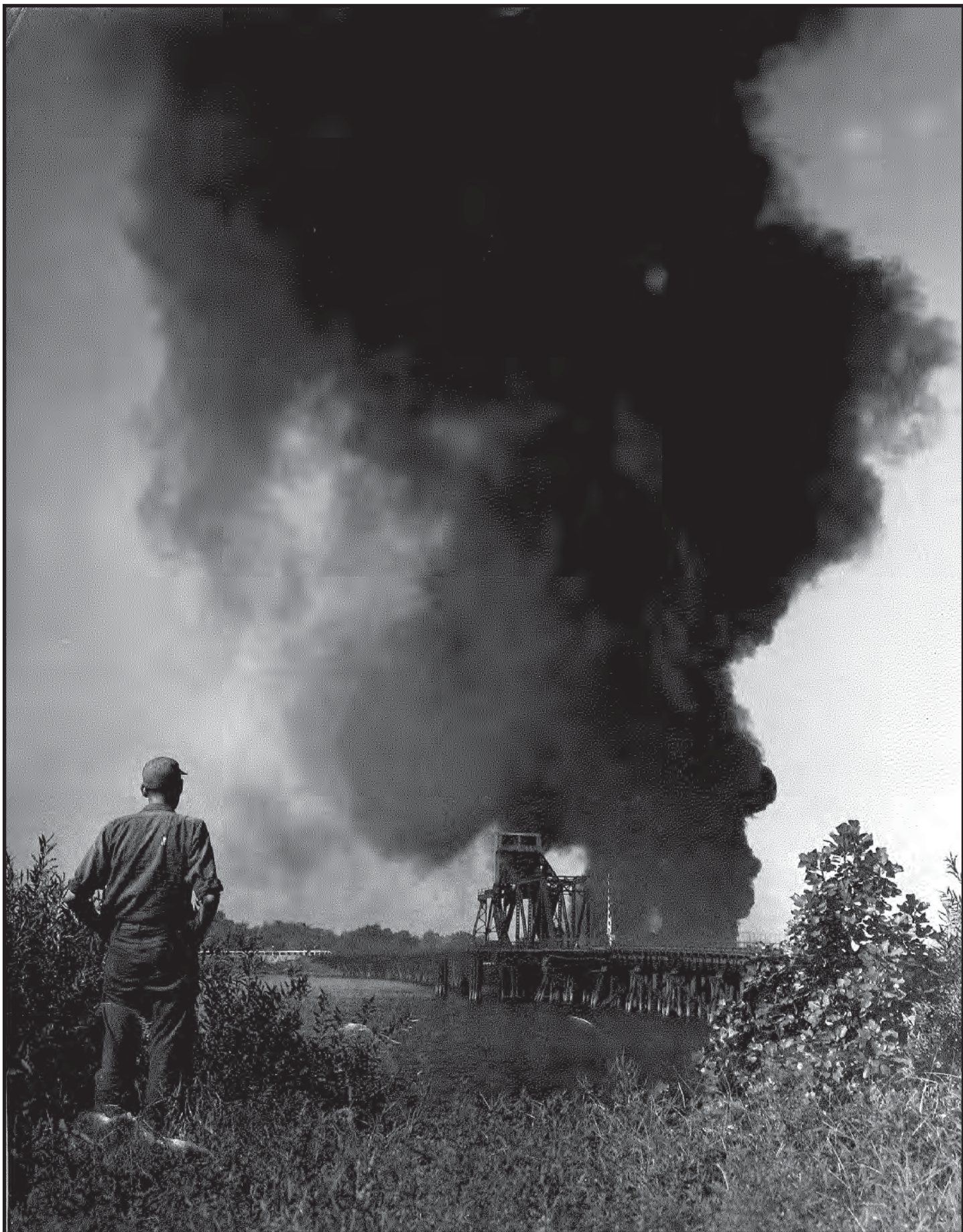
Image B.34. Fire on Petty's Island. View looking northwest from the Pennsylvania Railroad Drawbridge. Circa 1950. Source: Camden County Historical Society.
