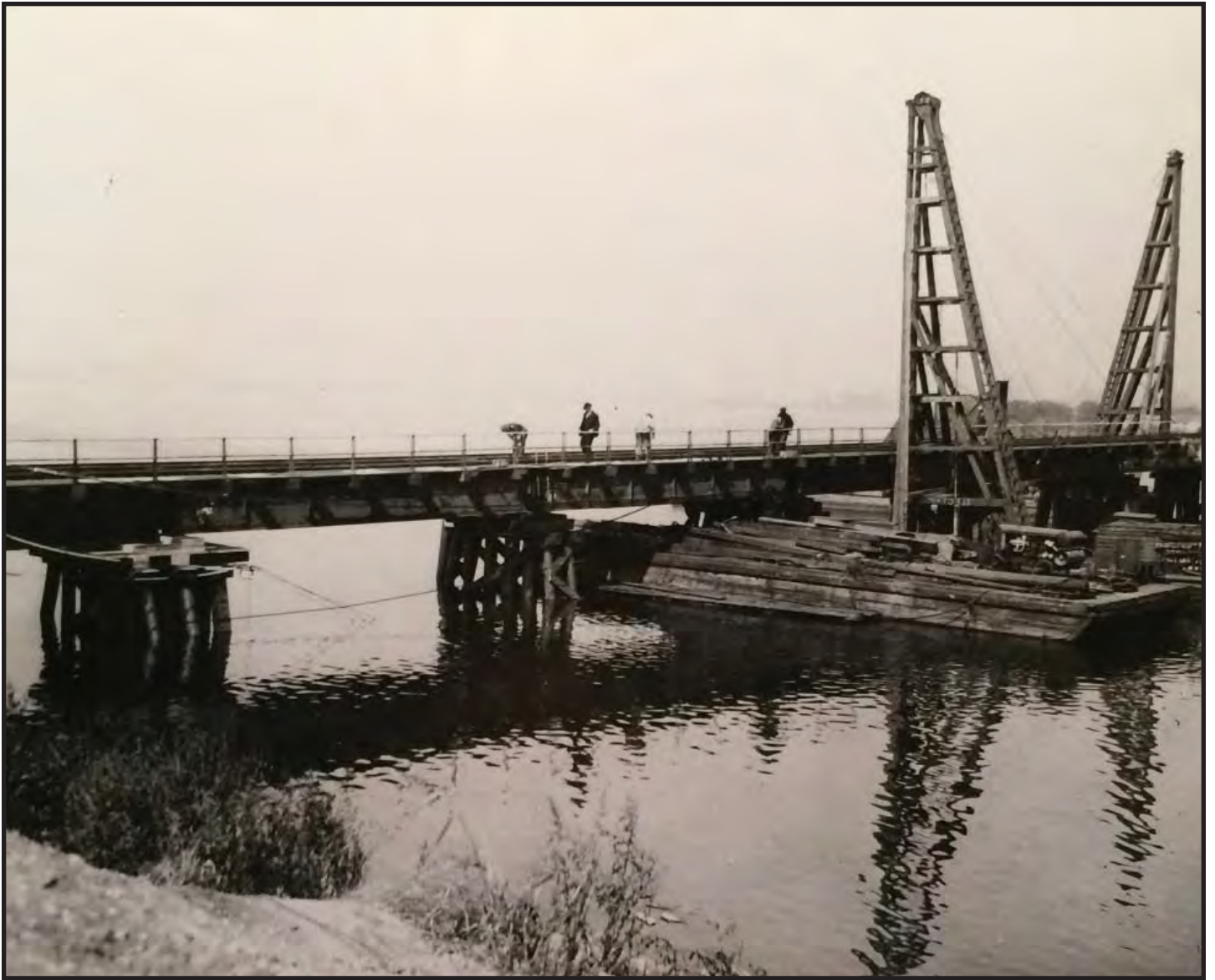
Image B.31c. Reconstructing Petty's Island Railroad Bridge. October 1935. Source: Philadelphia Record Photograph Collection, Historical Society of Pennsylvania.
