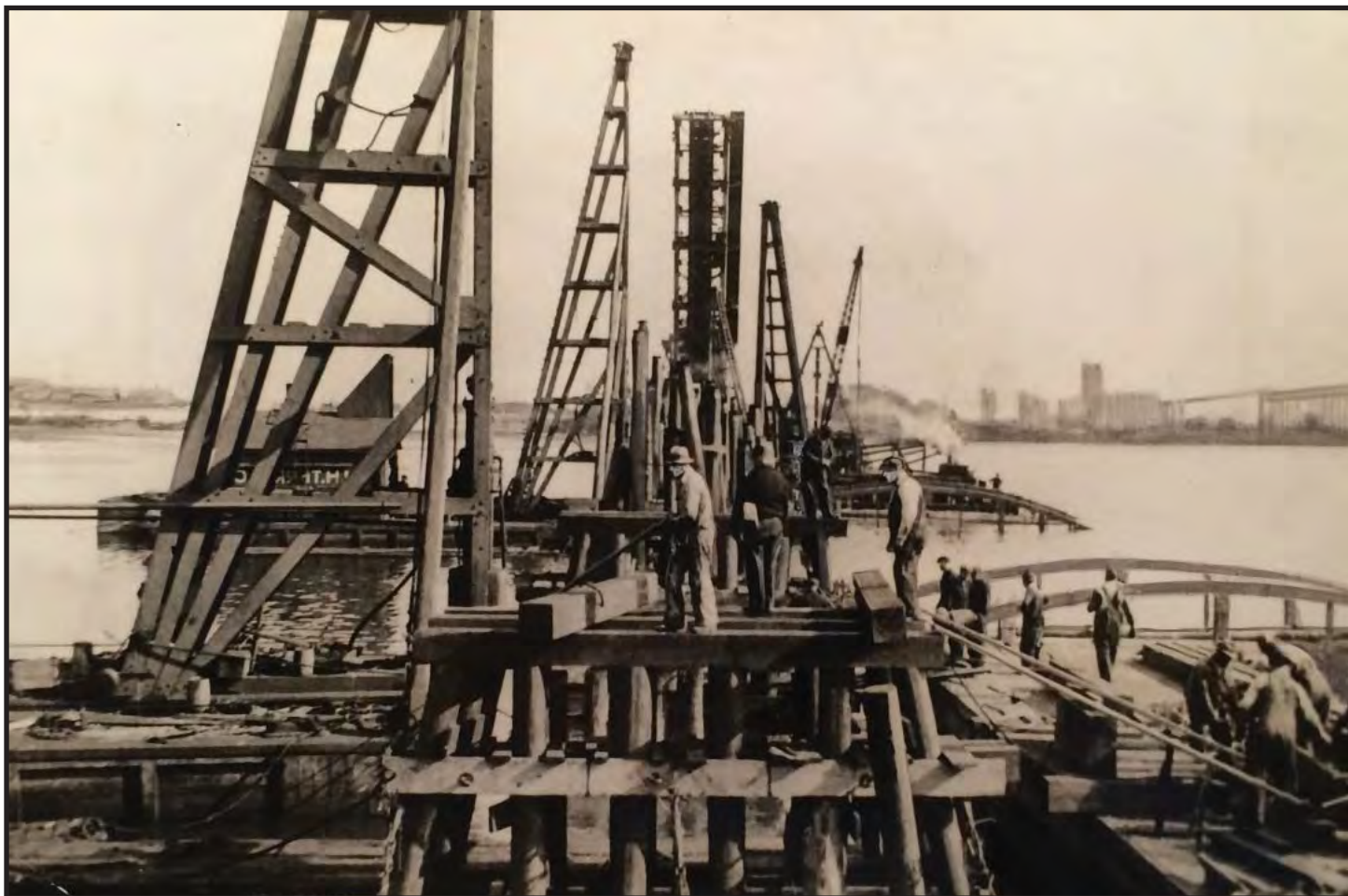
Image B.31a. Reconstructing Petty's Island Railroad Bridge. October 1935. The earlier bridge of 1916 was damaged by fire. The Philadelphia Record reported that the new bridge was completed in less than two weeks in order to keep 500 men working on the island at the refinery and other industries. Source: Philadelphia Record Photograph Collection, Historical Society of Pennsylvania.
