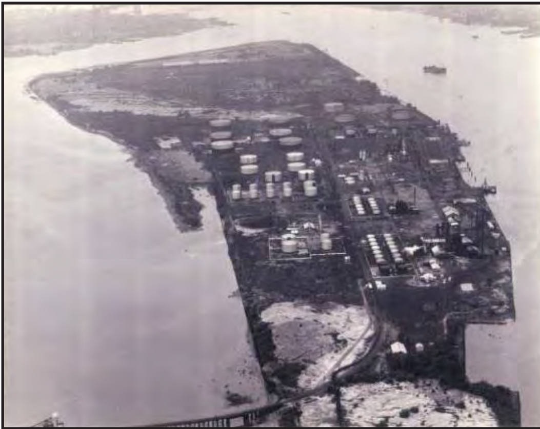
Figure A.61. Dallin Aerial Survey Company. Crew Levick Company, Petty's Island. 1938. View looking southwest (downriver).
