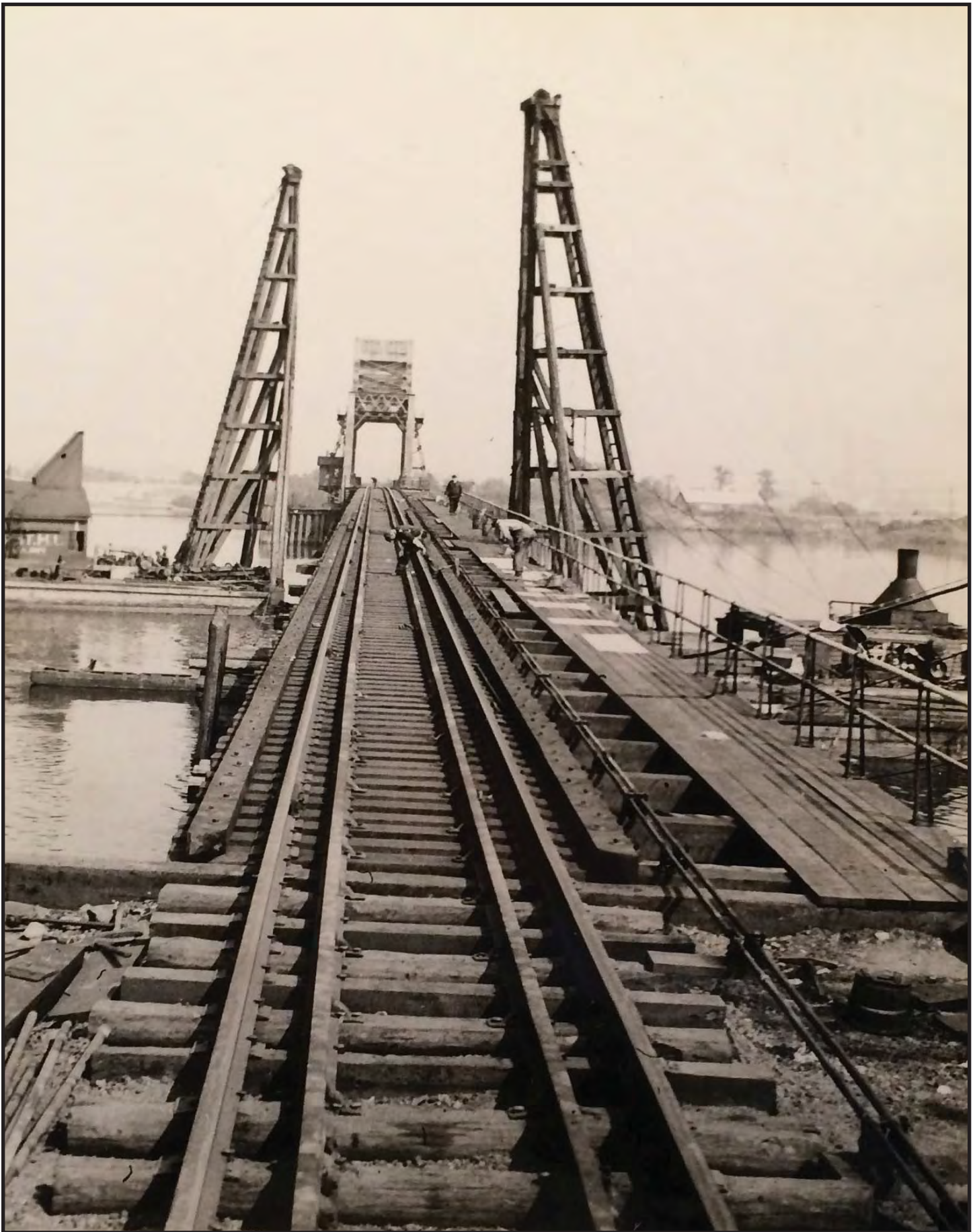
Image B.31b. Reconstructing Petty's Island Railroad Bridge. October 1935. Source: Philadelphia Record Photograph Collection, Historical Society of Pennsylvania.
