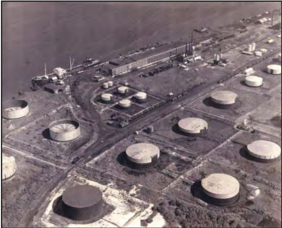
Figure A.63. Dallin Aerial Survey Company. Crew Levick Oil Company, Petty's Island. 1939. View looking southwest (downriver).
