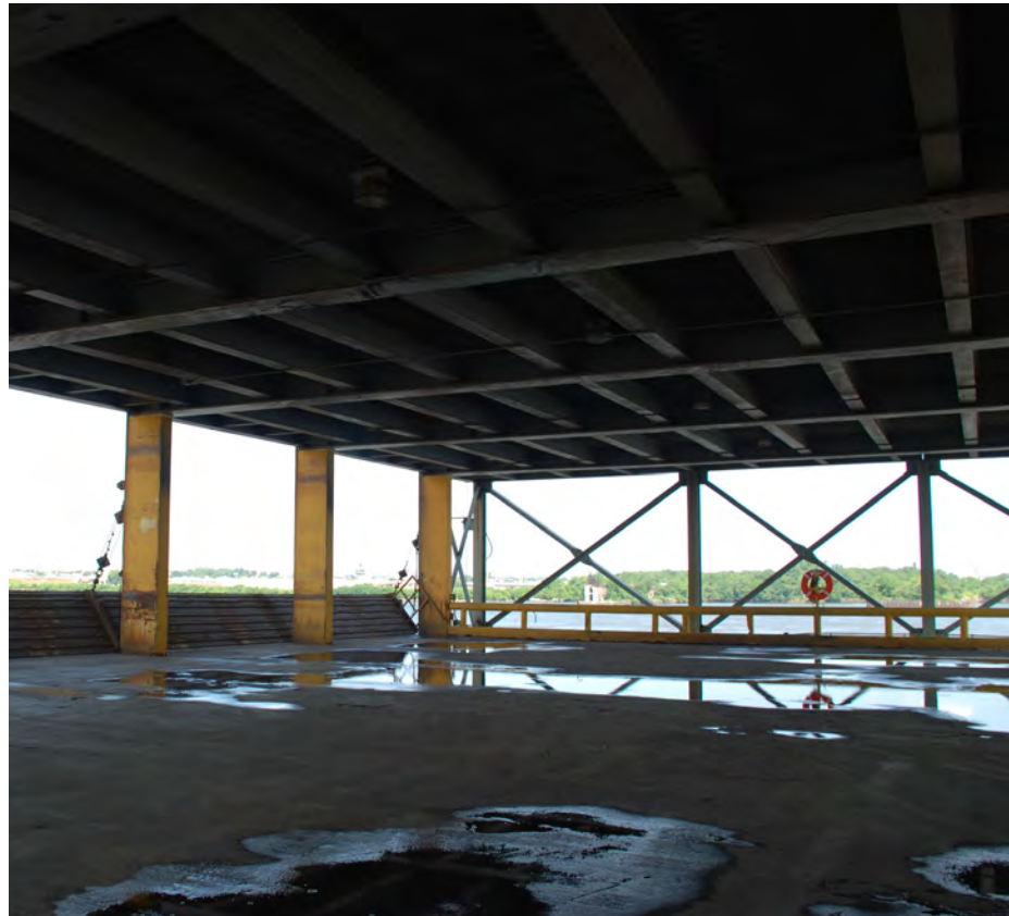
Existing Second Level of shipping terminal showing exposed structure.
