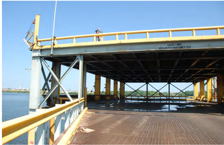
Existing shipping terminal with loading indicated on beam.
