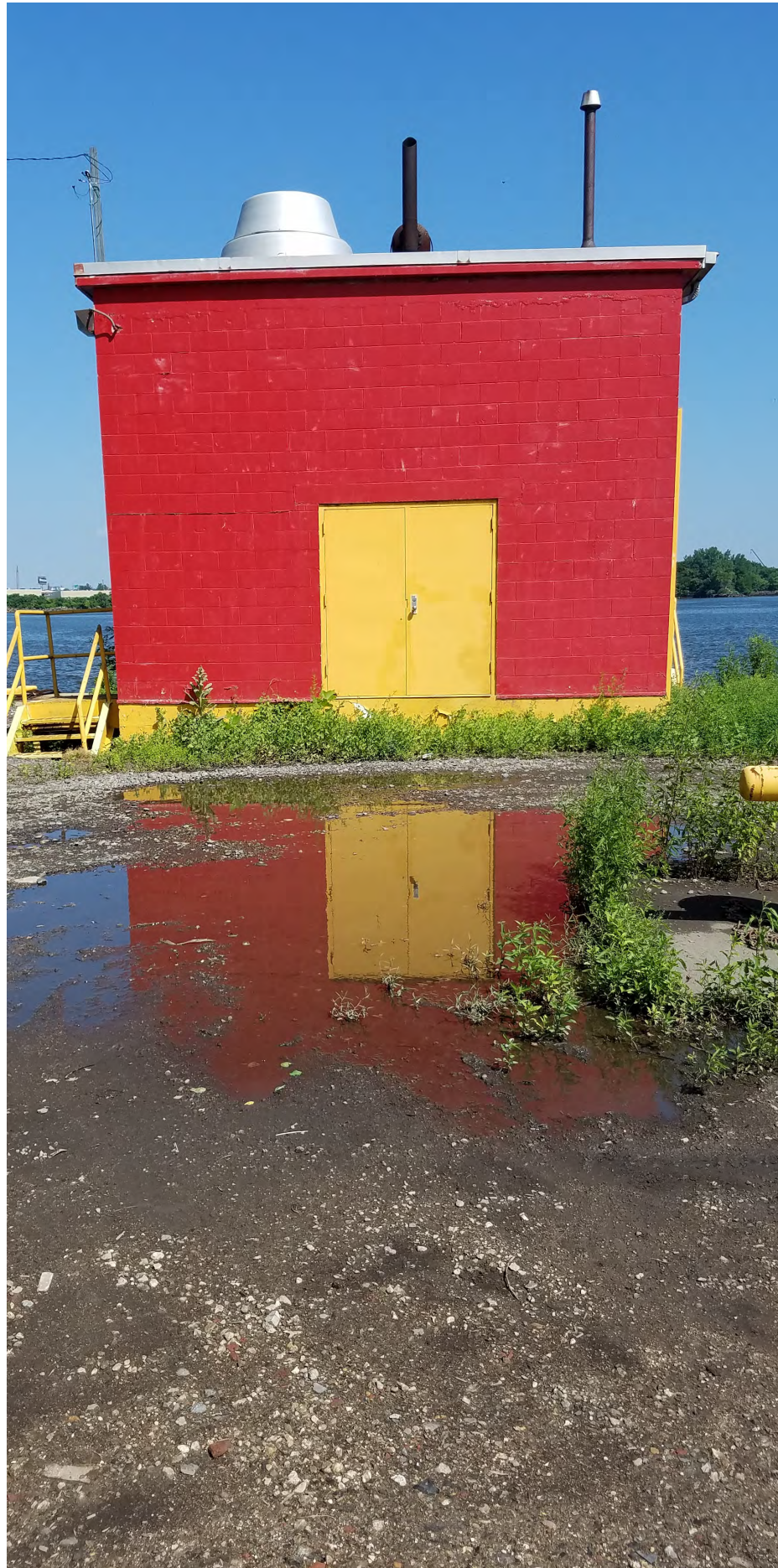
Existing fire pump building.
