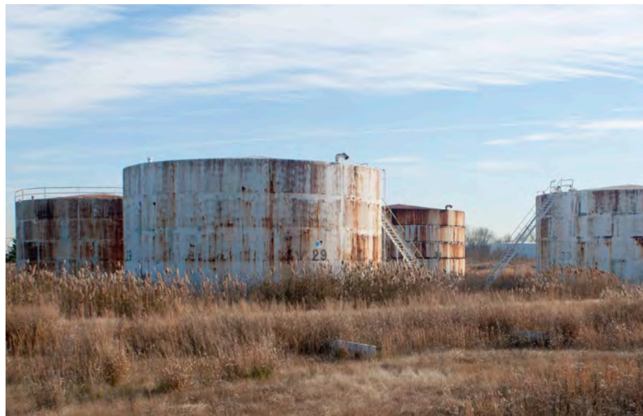
Existing oil tanks to be removed.
