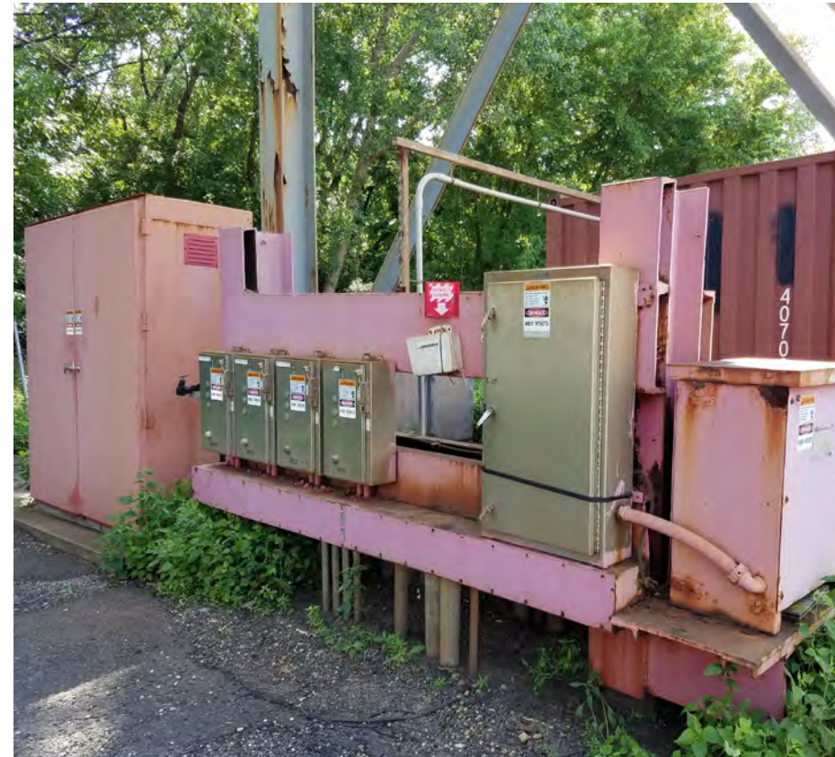
Existing electrical transformer.
