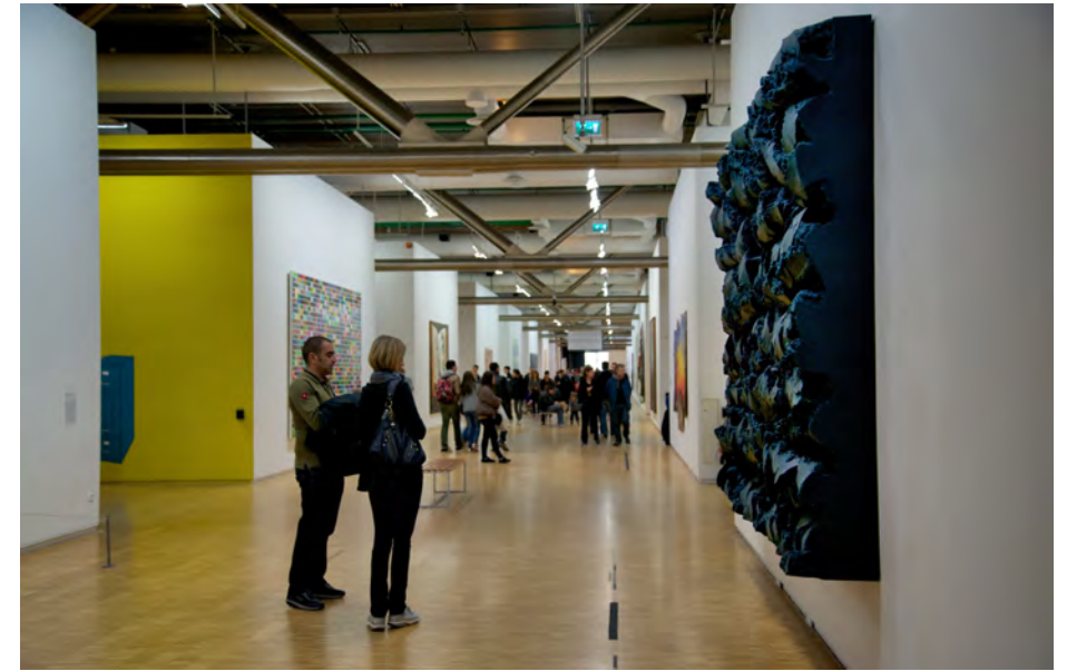
Image showing how walls will not go to underside of slab.
