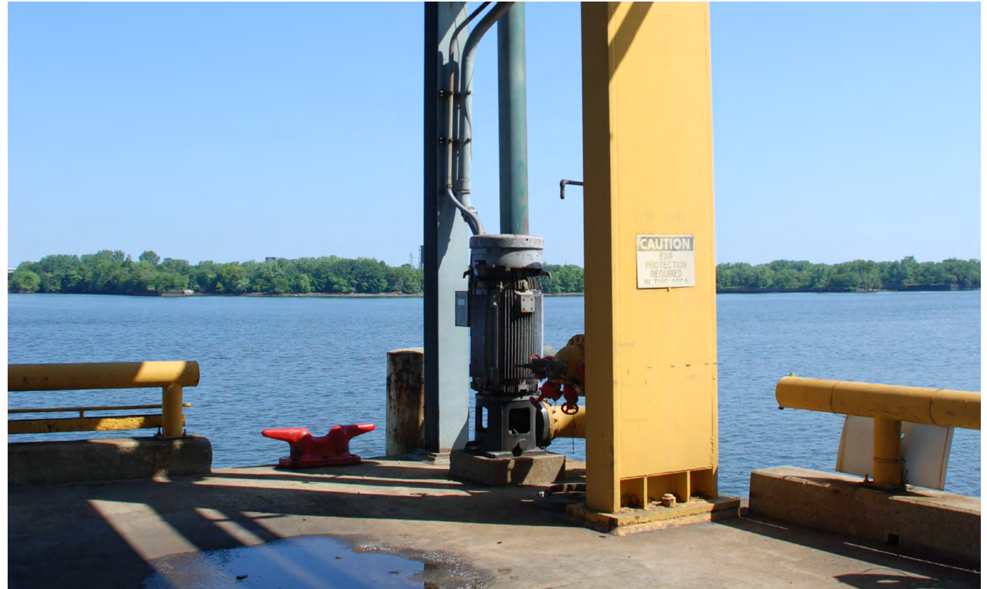
Existing fire pump at the shipping terminal.
