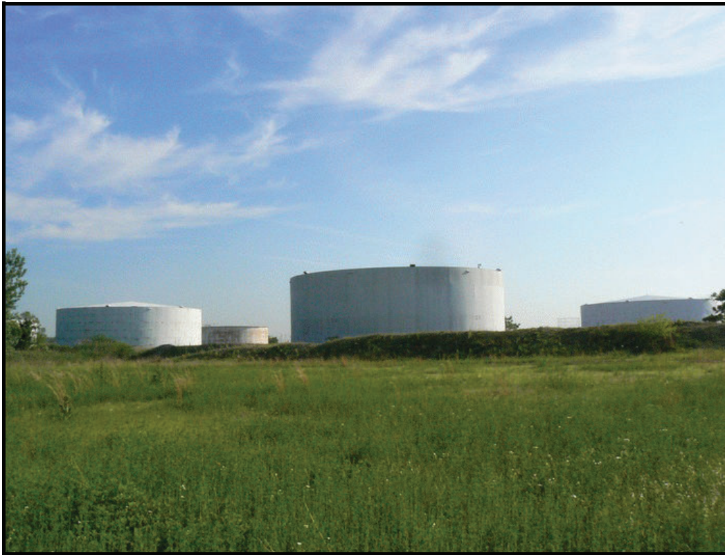
Figure 5. A large field of oil storage tanks lies in the center of the island. Herpetological Associates, Inc. 2010.
