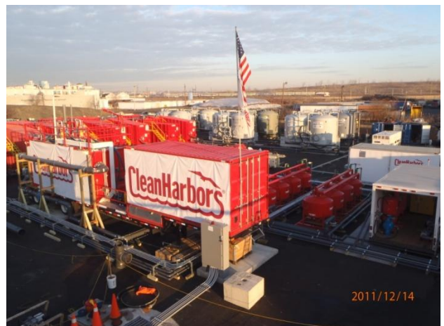
Assembled water treatment system
