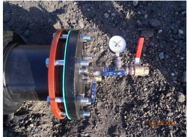
Hydraulic pipeline pressure testing
