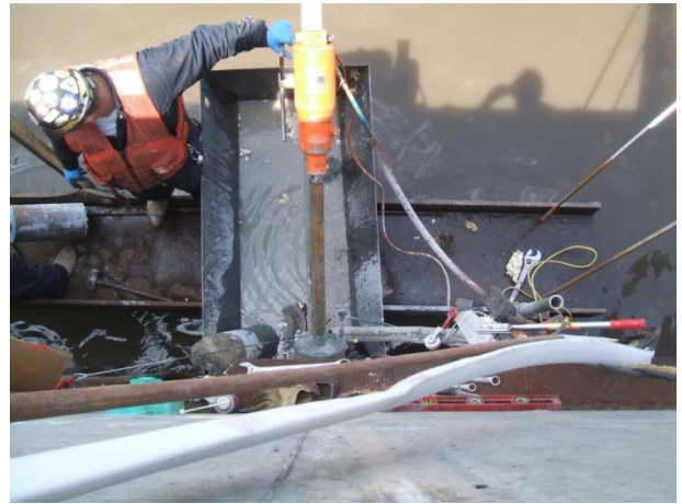
Coring of the OU-1 flood wall
