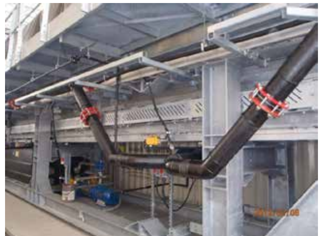
Installed piping for the sediment processing system
