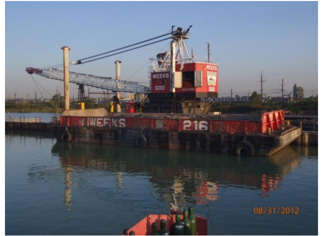
Enclosure backfill operations
