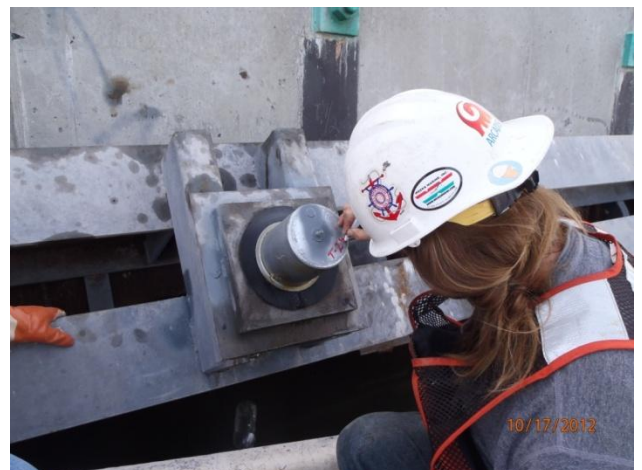
Marking tiebacks during final inspection
