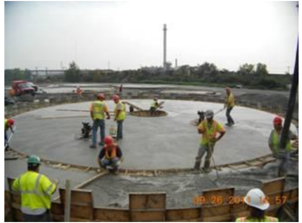
Concrete finishing being performed on the gravity thickener
