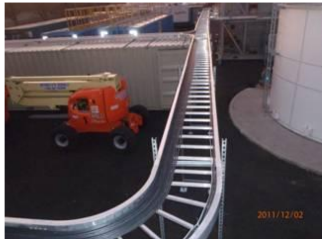
Cable tray and electrical installation for the sediment processing system
