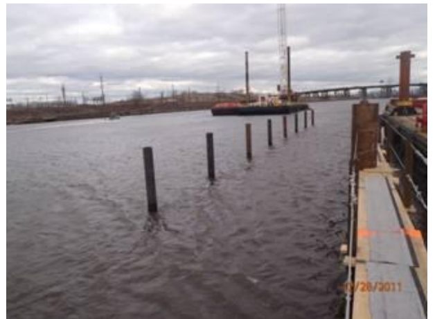
Installation of enclosure monopiles
