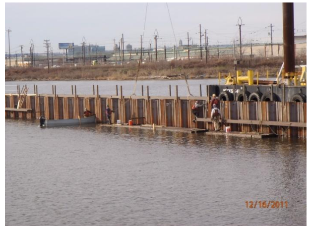
Wale installation along the north wall of the enclosure
