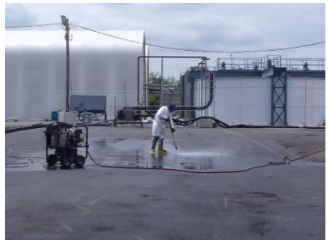
Cleaning of asphalt surfaces at the UPF
