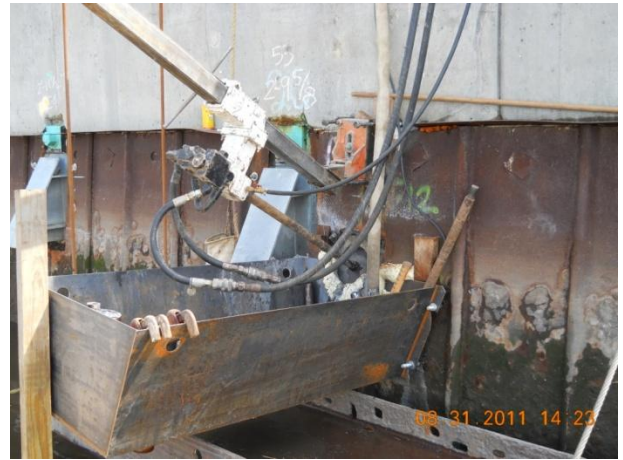
Concrete coring equipment installed
