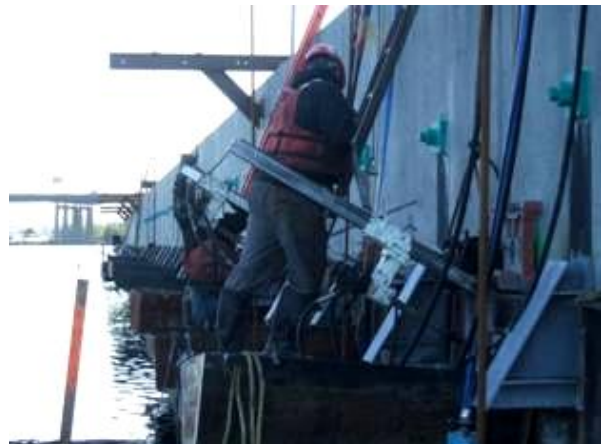
Core drilling activities along the OU-1 flood wall
