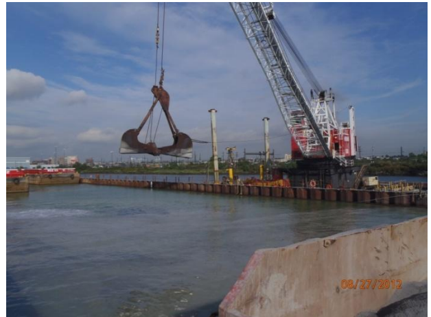
Enclosure backfill operations
