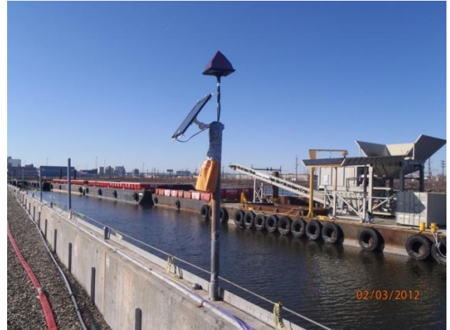
Eagle Eye bird deterrence system installed
