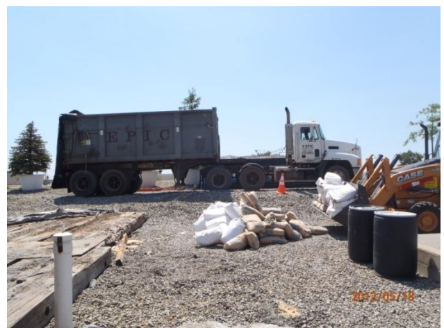
Truck and intermodal container staged for debris load-out
