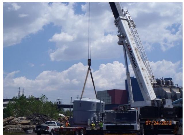
Removal of water treatment equipment
