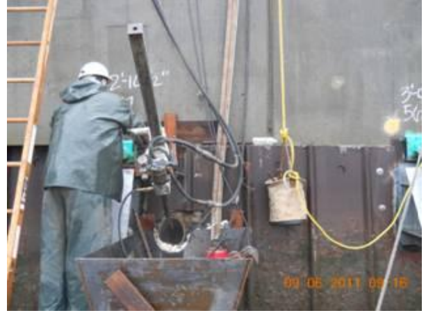
Concrete coring of the OU-1 flood wall
