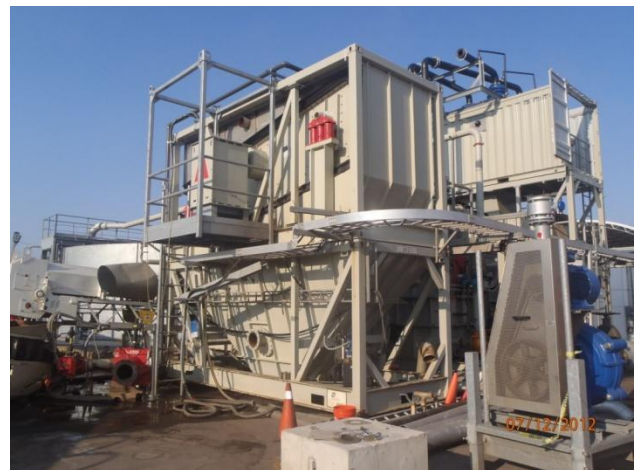
Coarse solids separation equipment clean
