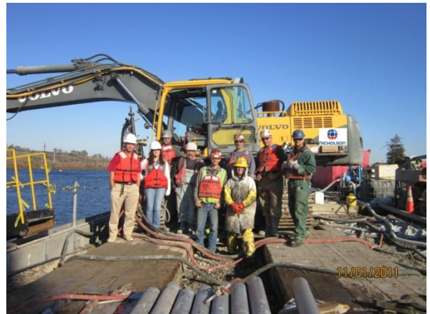
Nicholson tieback drilling crew
