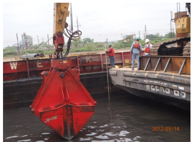
Performing an elevation check of the dredge bucket
