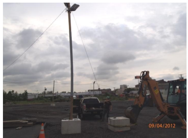
Team retensioning and adjusting light poles at the UPF
