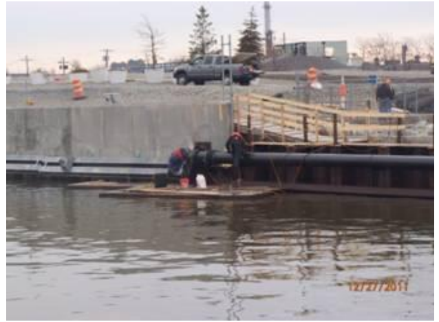
Installation of piping for the reroute of storm water from the OU-1
