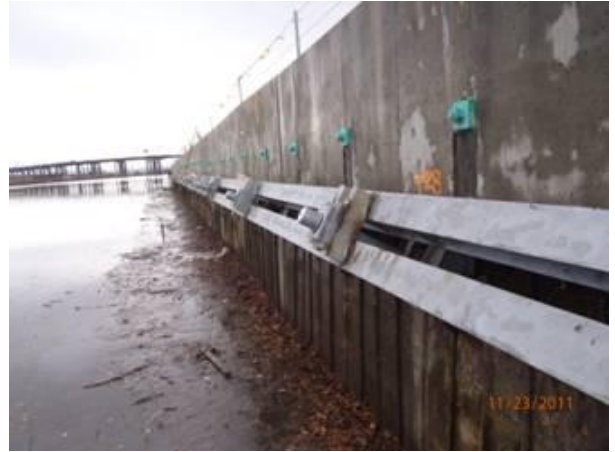
Completed tiebacks along the OU-1 floodwall
