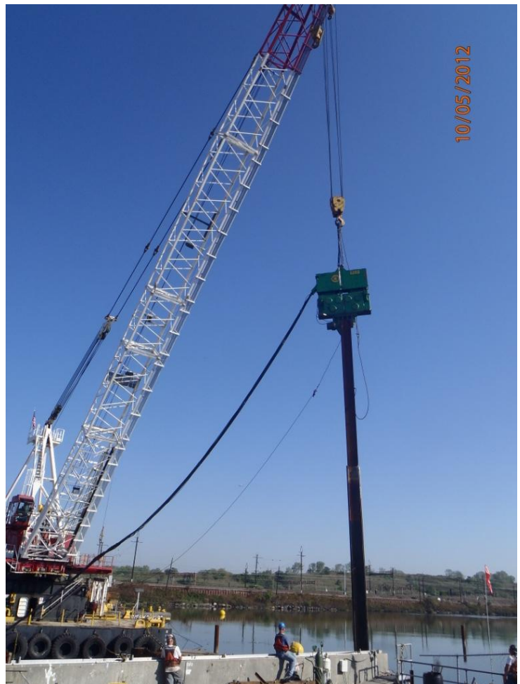
Removal of one of the final piles of the sediment removal enclosure
