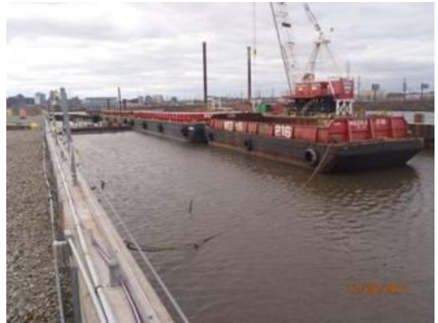
Moving work barges inside the enclosure
