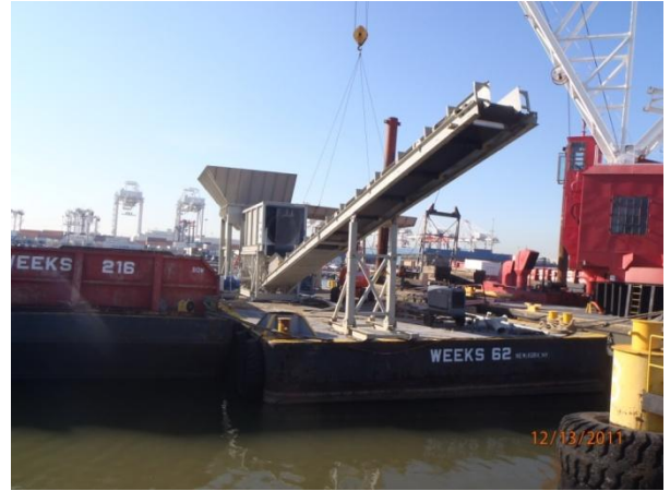
Assembly of barge-mounted sediment screening system at Weeks Yard
