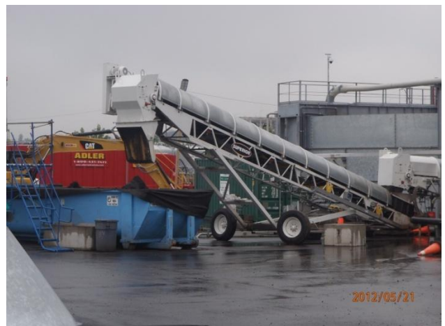
Conveyor operating at the coarse solids operation
