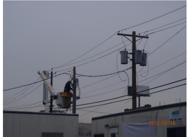
PSE&G installing electrical service to the UPF
