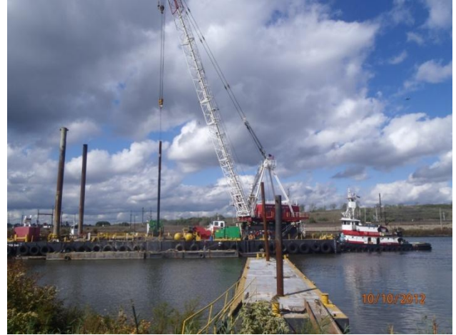
Removal of the final monopile near the UPF
