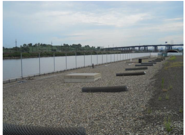
The fence at the OU-1 Property during removal
