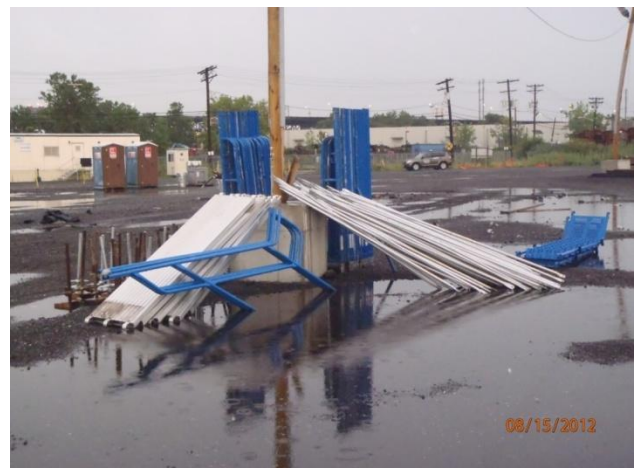
Scaffolding system disassembled and awaiting pickup
