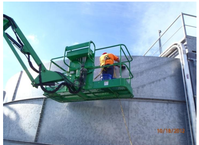
Disassembly of the gravity thickener
