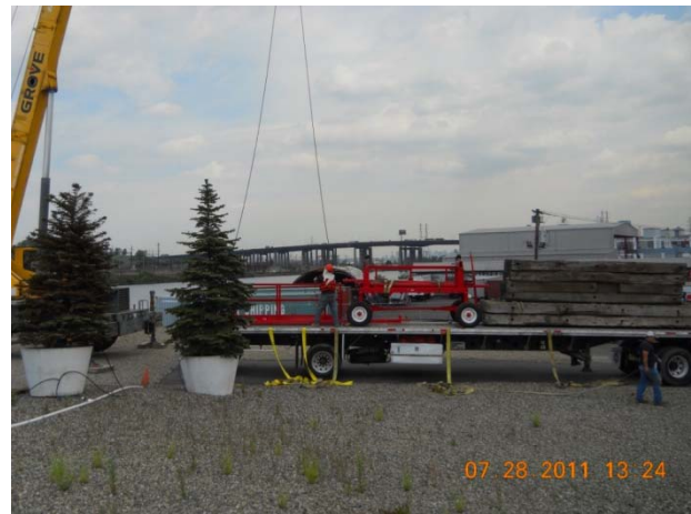
Off loading equipment for core drilling at OU-1 property
