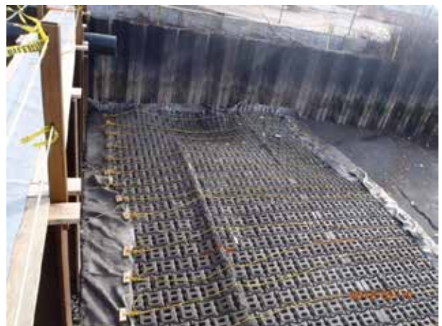
Installed concrete mattress adjacent to the Sherwin-Williams property
