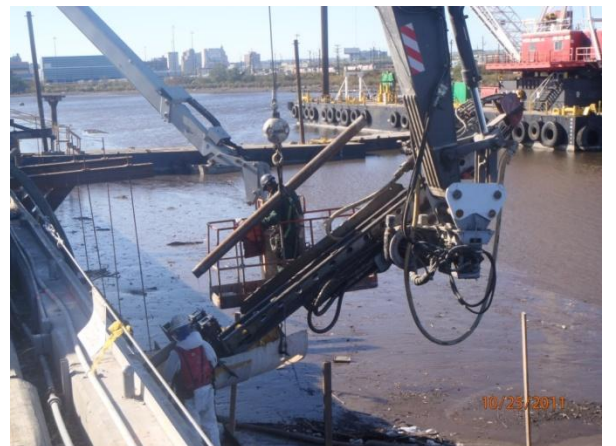
Tieback drilling along the OU-1 flood wall
