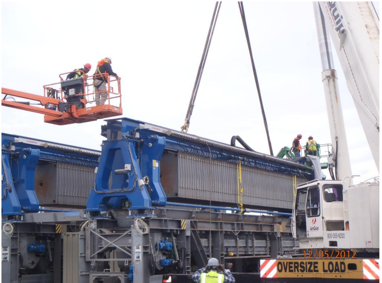
Rigging of filter press for removal
