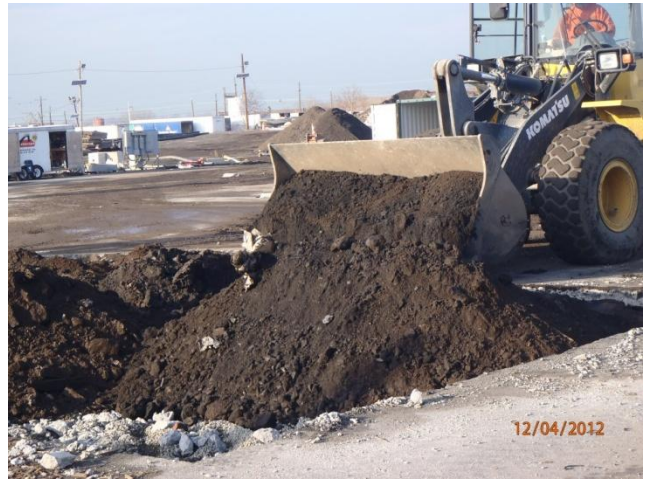
Backfill of equipment pads
