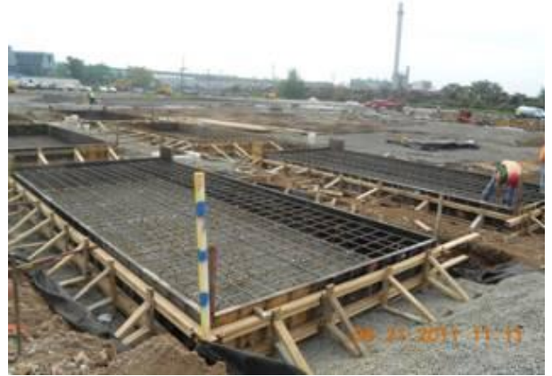
Reinforcement bar and forms for the Carbon Adsorber Pads
