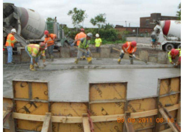
Installation of concrete for Equipment Pad #9
