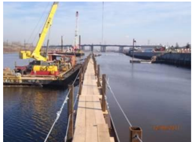
Walkway installation along the north wall of the enclosure
