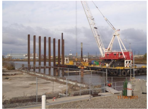
Enclosure construction for the west wall
