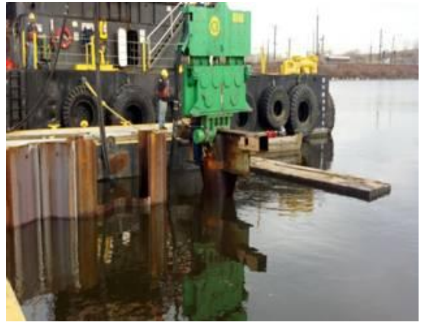
Vibratory hammer installing the template for enclosure wall construction
