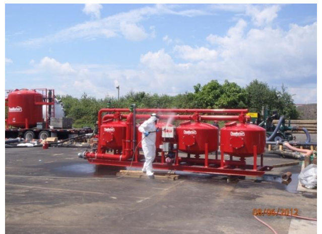
Decontamination of water treatment system
