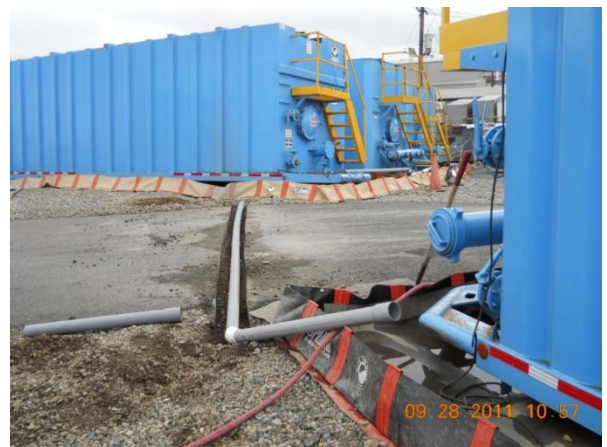
Tieback fluids pre-treatment system during installation
