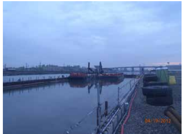
Sediment screening barge within the enclosure
