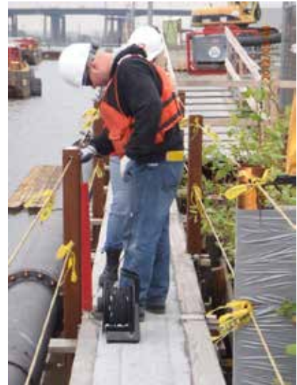
Monitoring of the enclosure inclinometers
