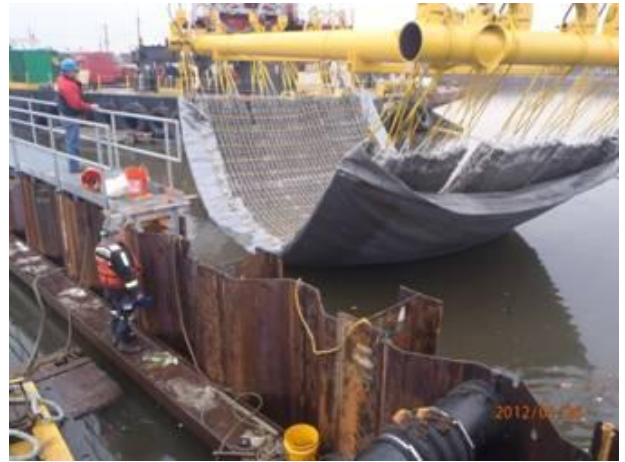
Installation of concrete mattresses for scour protection
