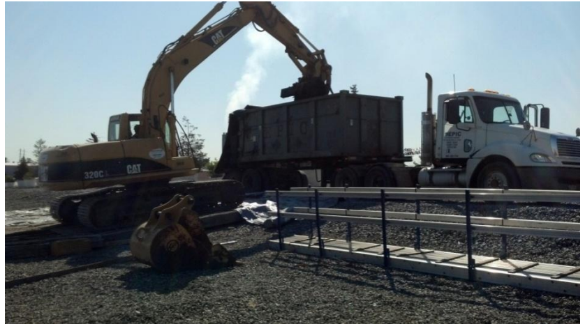
Loadout of dredged debris material at the OU-1
