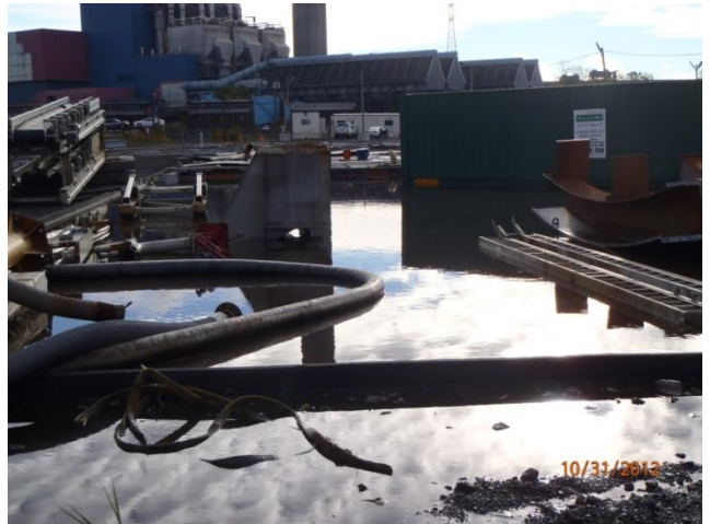
Remaining floodwaters from Hurricane Sandy at the UPF Site
