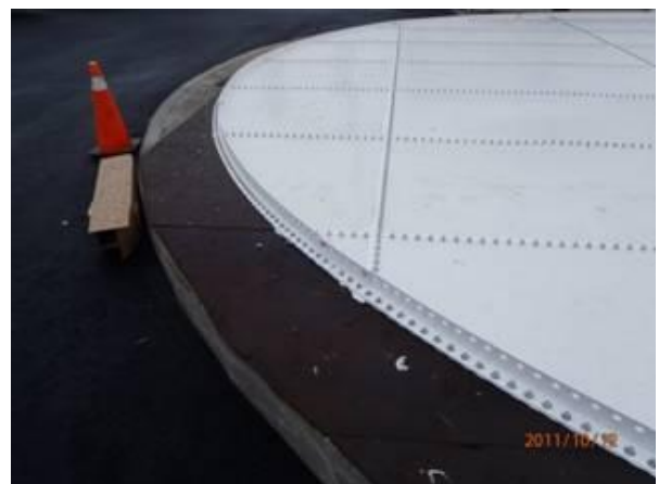
Sludge holding tank during installation
