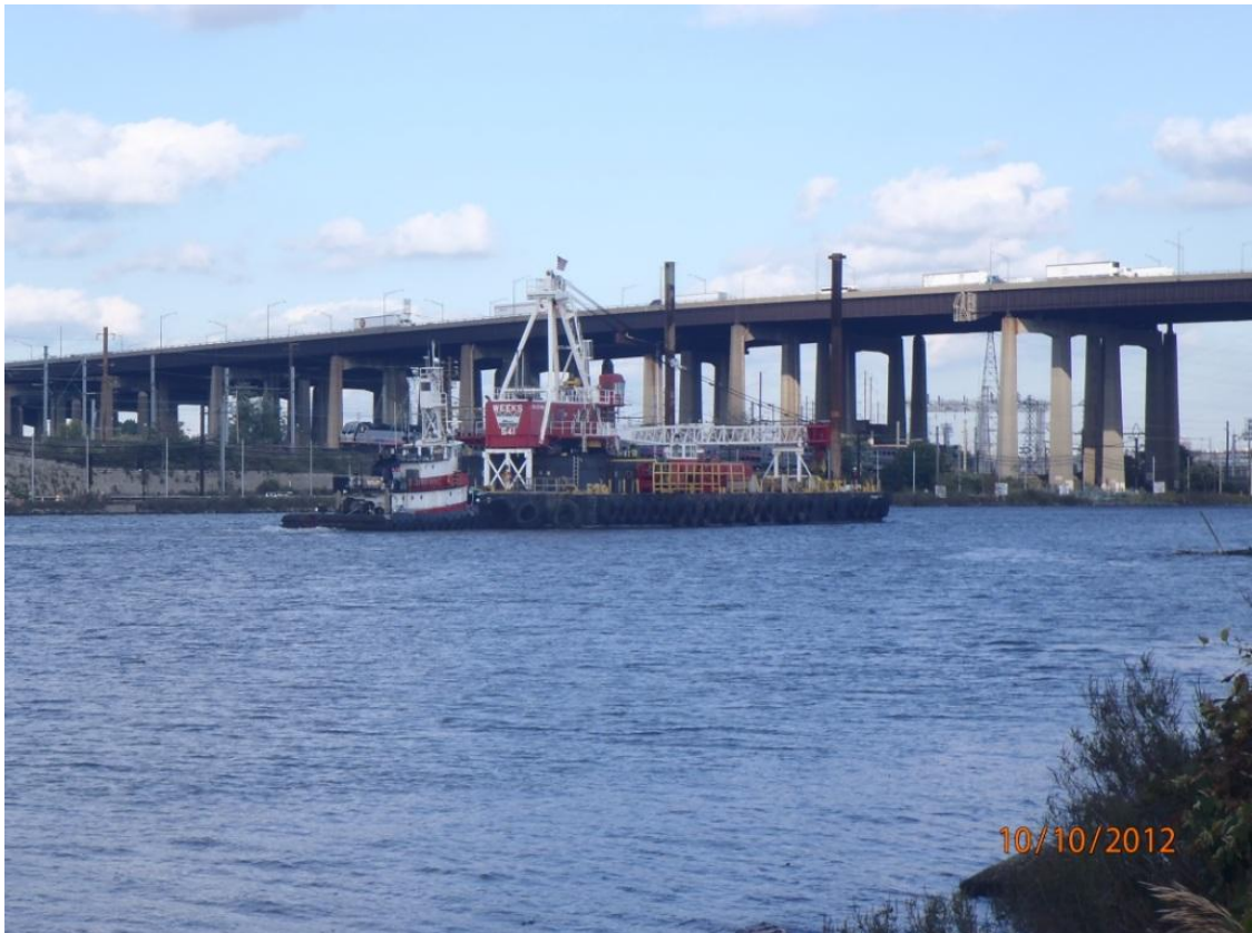
Demobilization of Weeks crane from the Site
