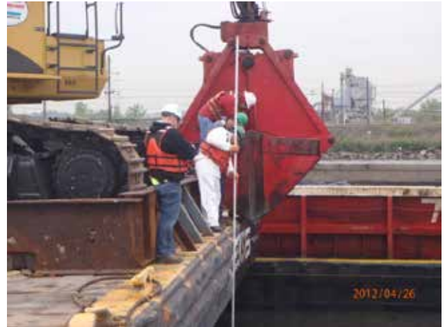
Bathymetry checks for dredging
