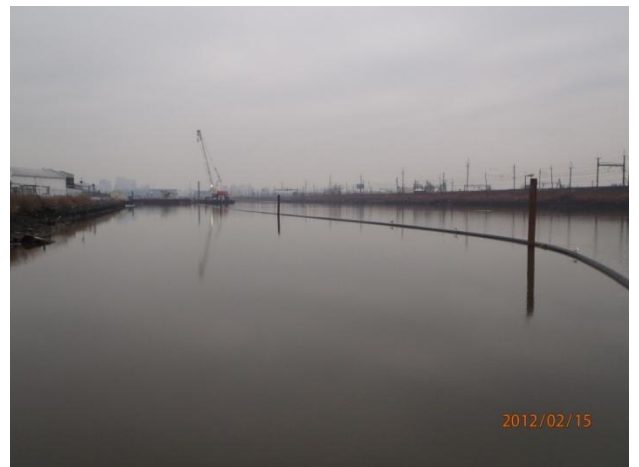
Hydraulic pipeline installed
