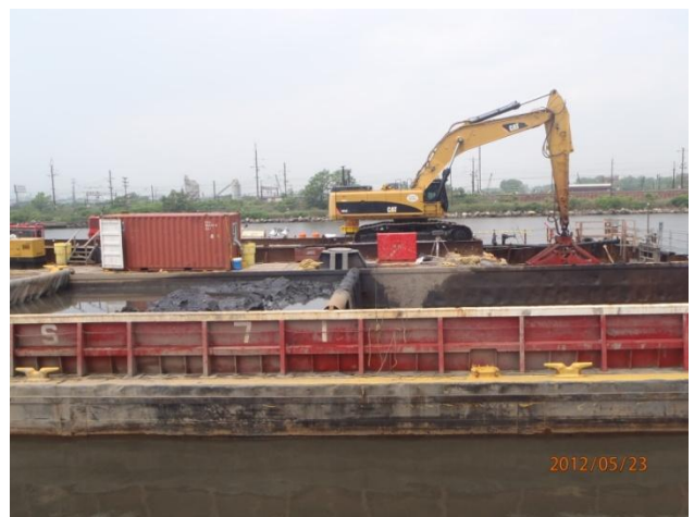
Dredge and material barge
