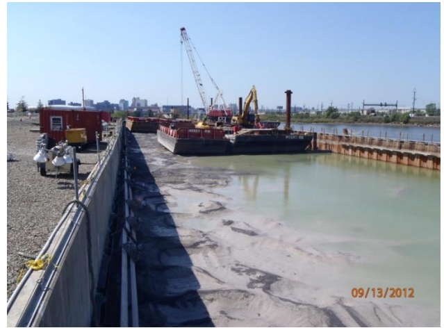
View of the backfilled enclosure
