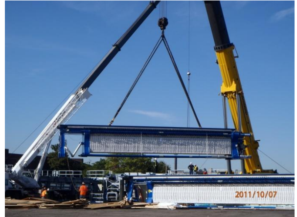
Off-loading of a membrane filter press
