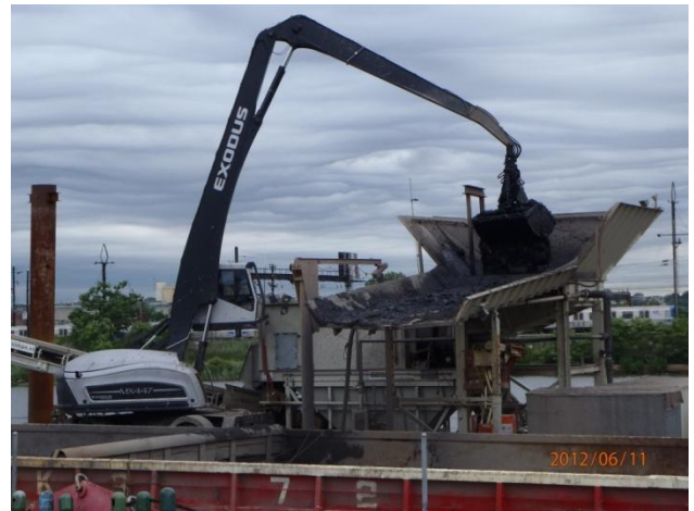
Screening of the final material dredged
