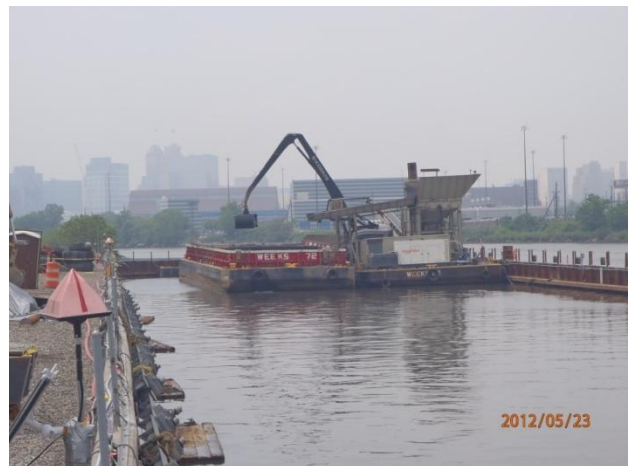
Sediment screening operation at the west end of the enclosure
