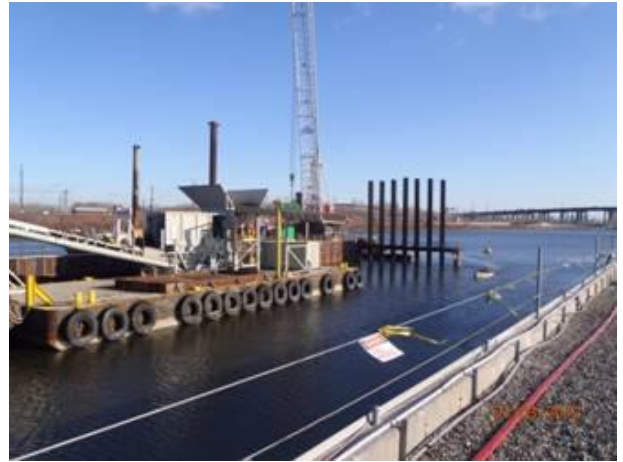
Installation of the east wall of the enclosure
