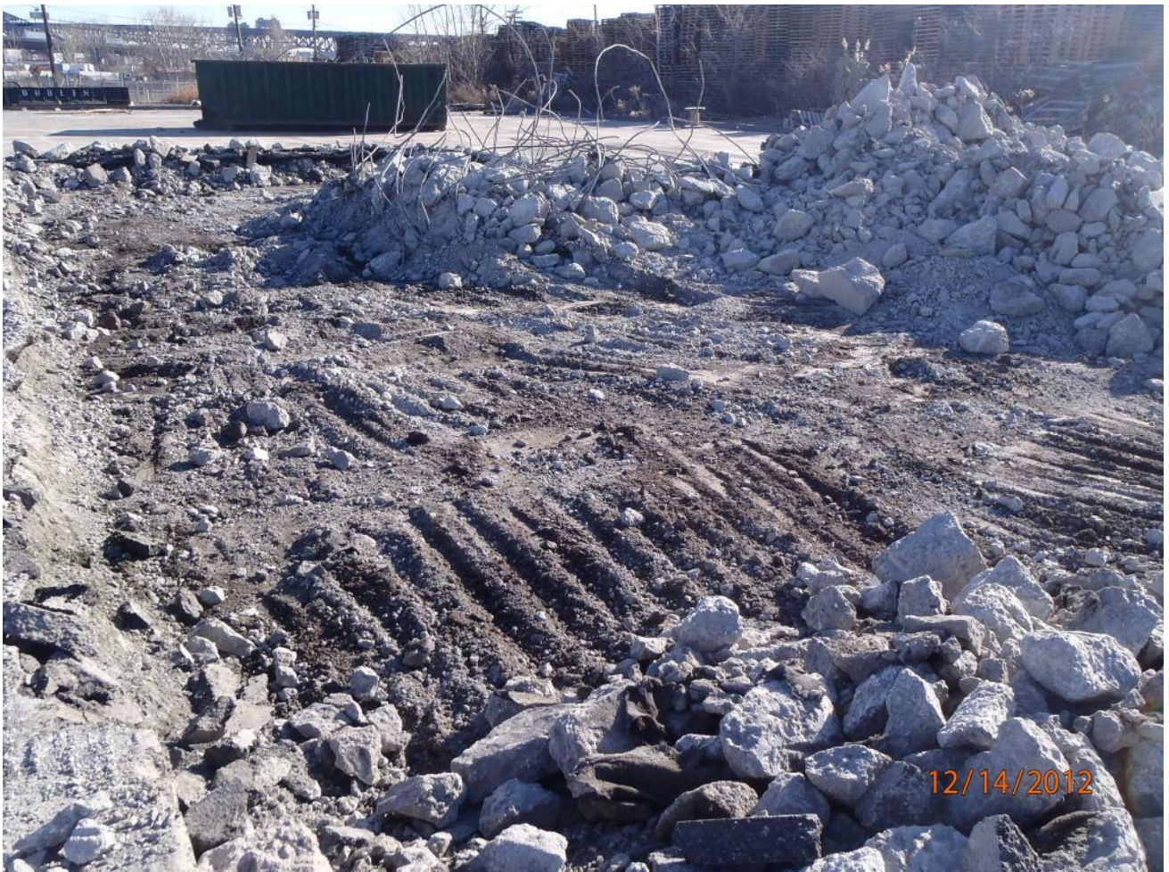
Breaking and removal of membrane filter press pads
