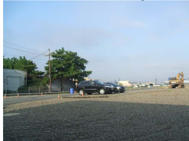
Temporary parking area at the OU-1 Property
