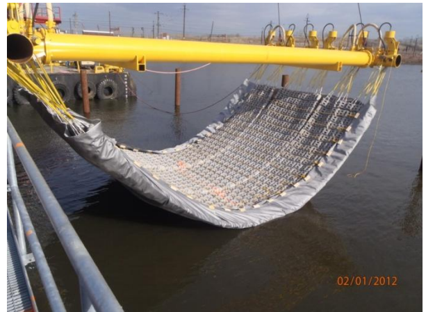
Installation of concrete mattress for scour protection
