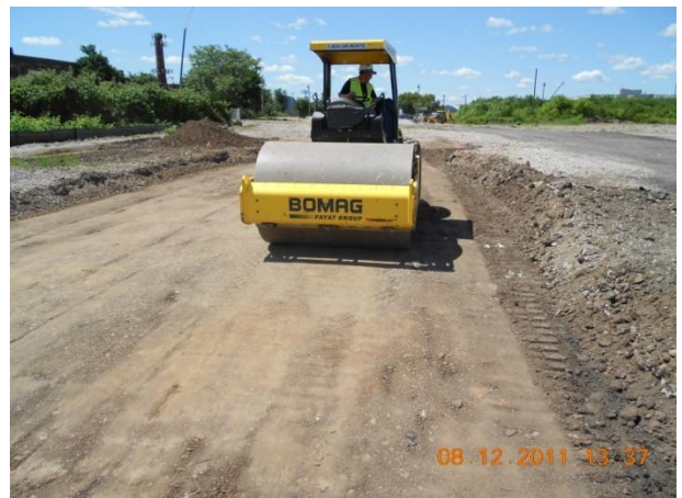
Compacting subgrade for sediment processing pad construction
