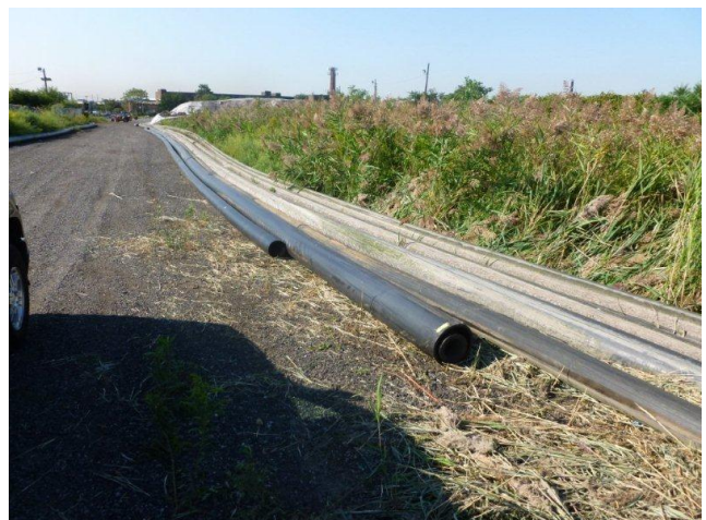
Hydraulic pipeline removed and staged at the UPF
