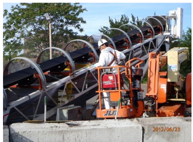
Inspection and decon of the coarse solids conveyor
