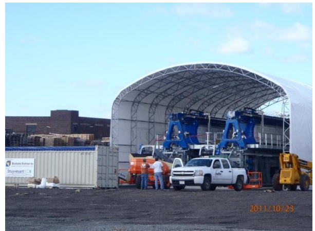
Completed south canopy over the membrane filter presses
