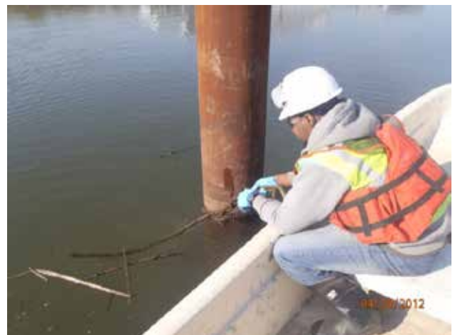
Pipeline inspection activities
