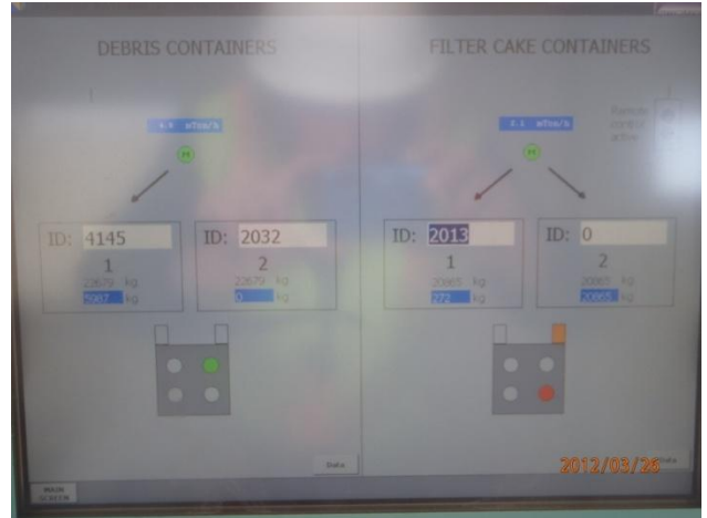
Computer display in the sediment processing system control room
