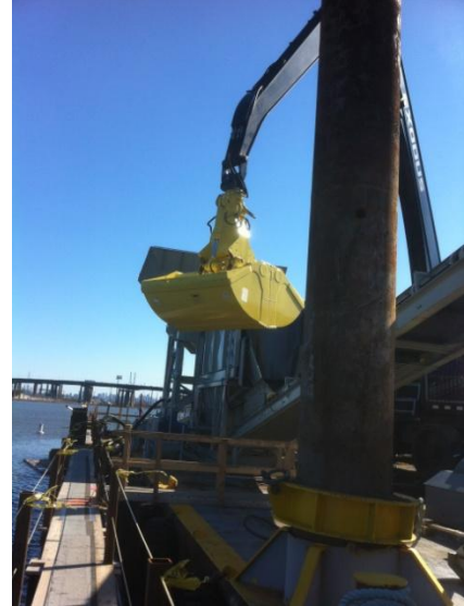
Bucket installed on excavator on sediment screening barge
