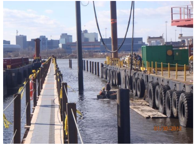
Installation of protective monopiles and dolphins
