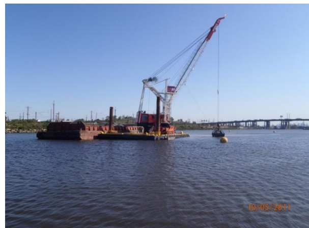
Grit placement for scour protection installation
