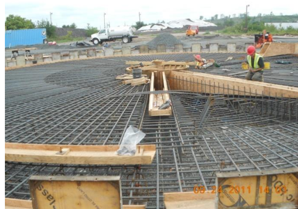
Reinforcement bar and forms for the Gravity Thickener
