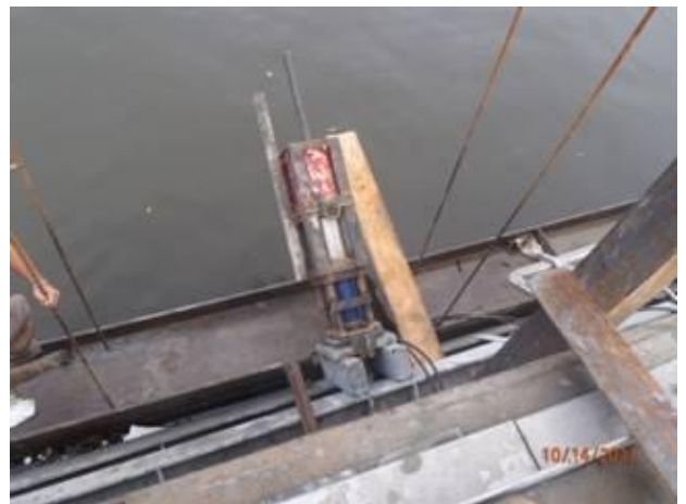
Performance testing equipment on Tieback T-7
