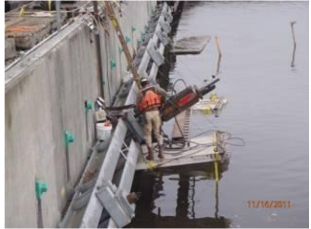
Stressing and performance testing of tiebacks along the OU-1 floodwall
