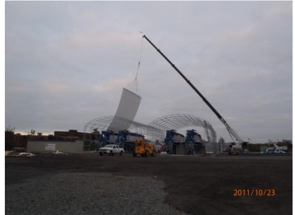
Fabric being installed on the south canopy
