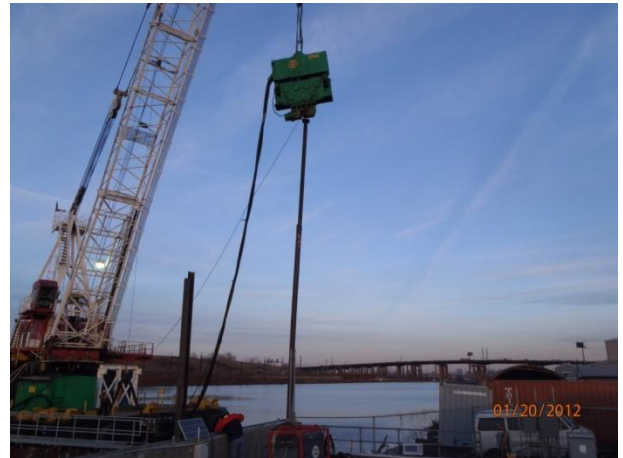
Working on the final sheeting at the south east corner of the enclosure
