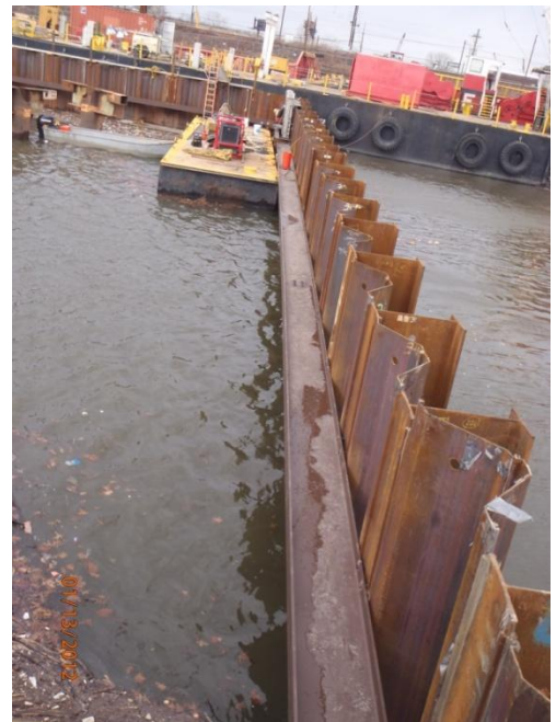
View of the east wall of the enclosure
