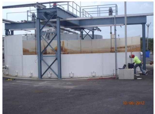
Removal of a sludge storage tank at the UPF
