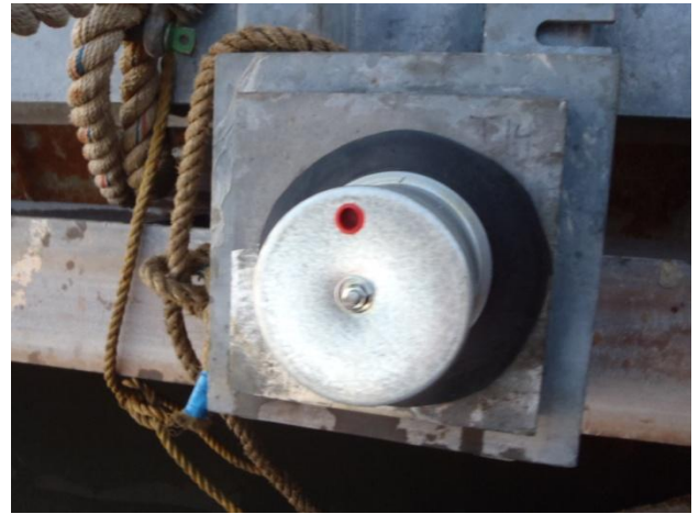
Tieback caps for inspections
