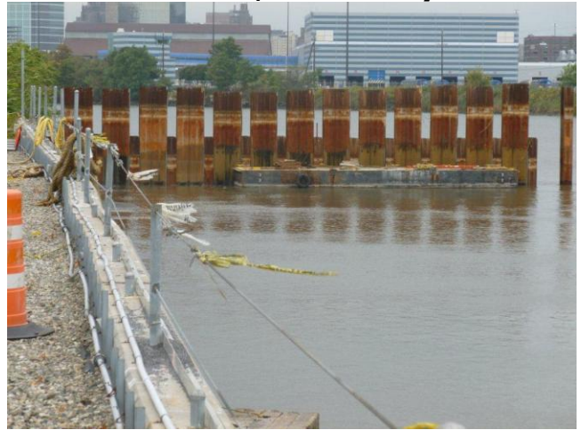
West wall sheets ready for removal
