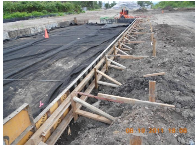
Formwork for the south filter press pad
