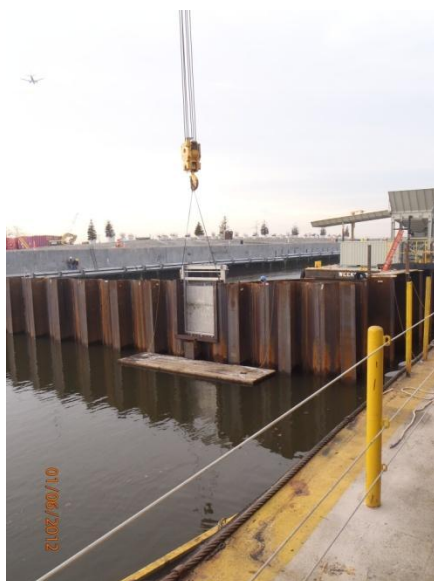
Weir gate installation in the east wall
