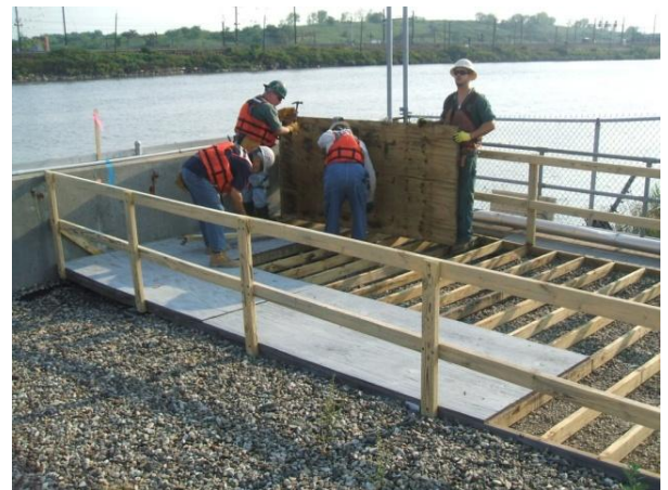
Workers removing platform at edge of OU-1 flood wall
