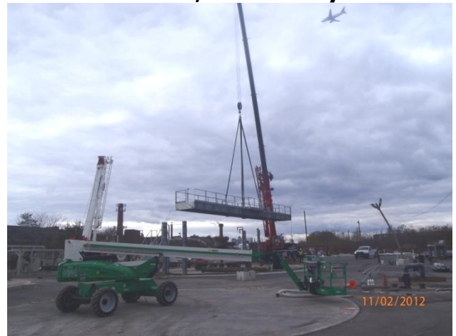
Removal and disassembly of the gravity thickener bridge of the sediment processing system
