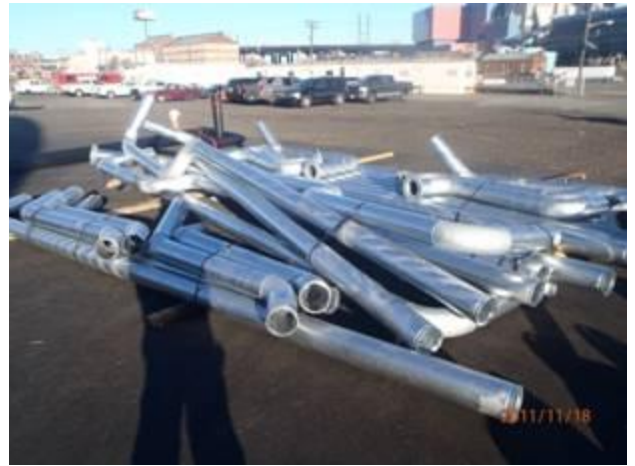
Piping fabrication for the sediment processing system
