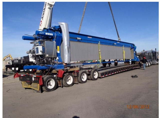
Loading of filter press for demobilization
