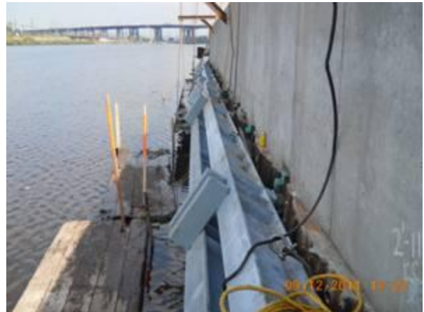
Wales installed along the OU-1 flood wall
