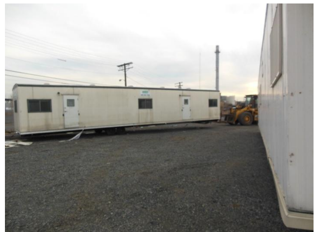
Removal of flood damaged trailers from the site
