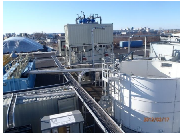
Coarse solids screening system for sediment processing
