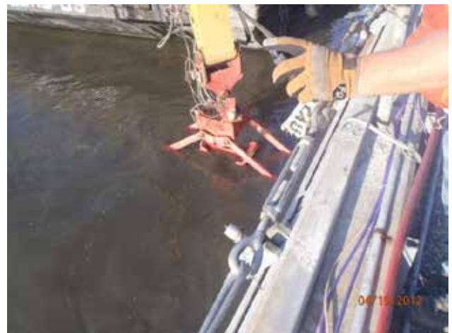
Dredging activities in Cell 6
