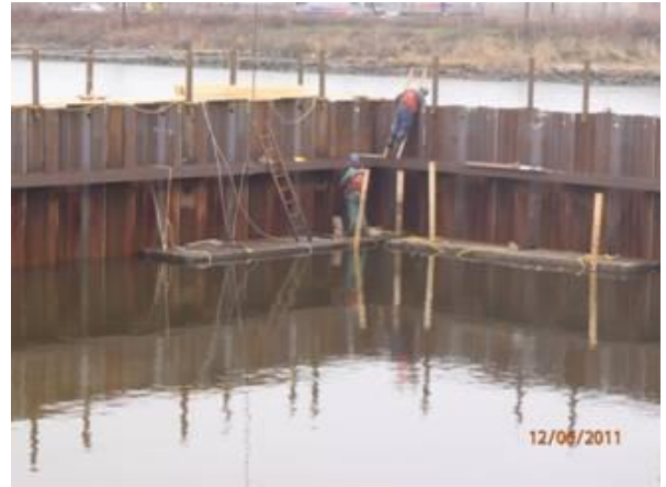
Wale installation in the northeast corner of the enclosure
