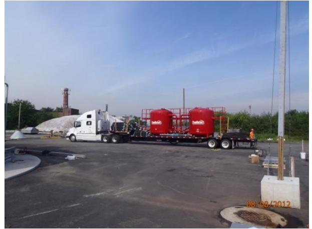
Demobilization of temporary treatment system
