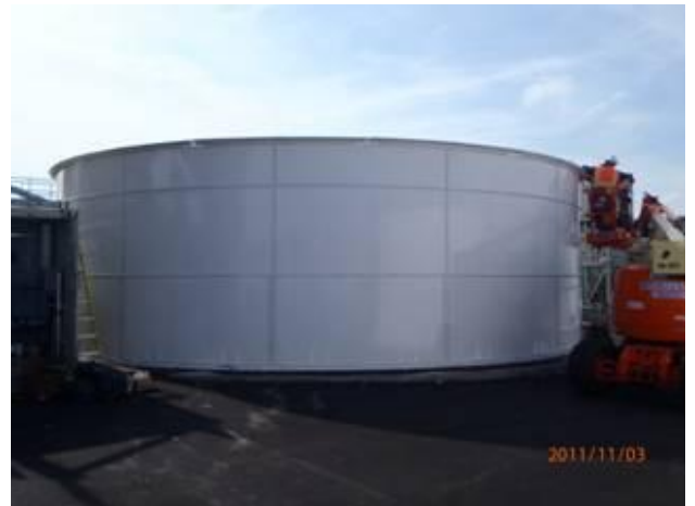
Installation of a sludge holding tank
