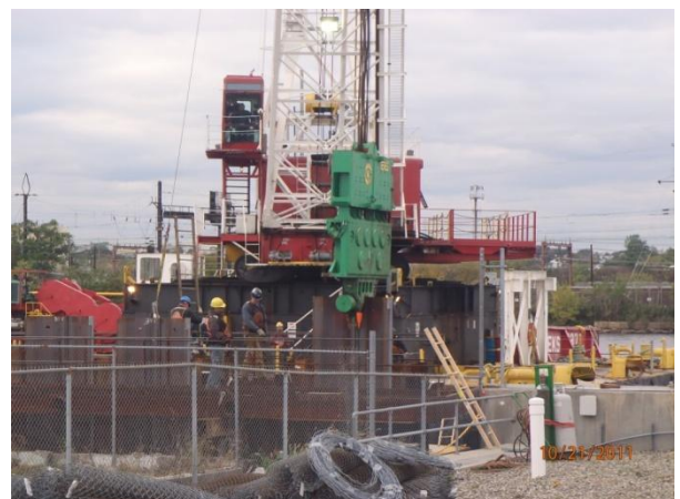
Combination wall installation in front of the Sherwin Williams property
