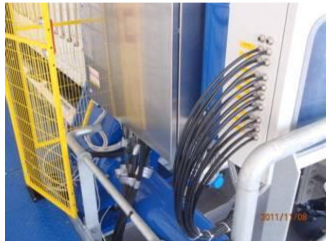
Electrical installation of sediment processing equipment
