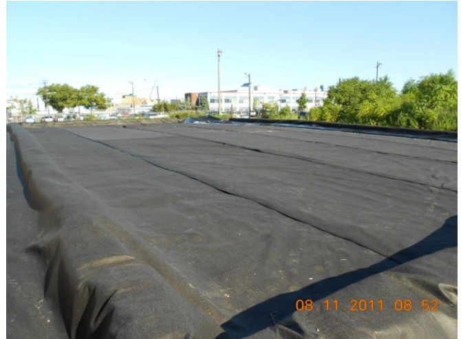
UPF material stockpile pad
