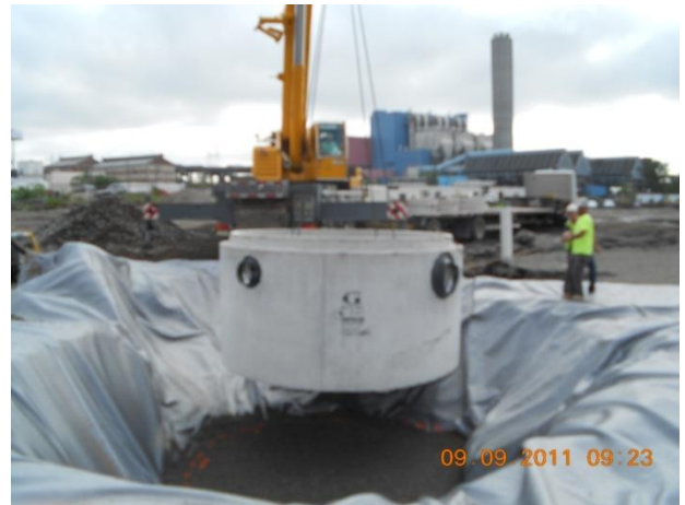
Pump station manhole during installation
