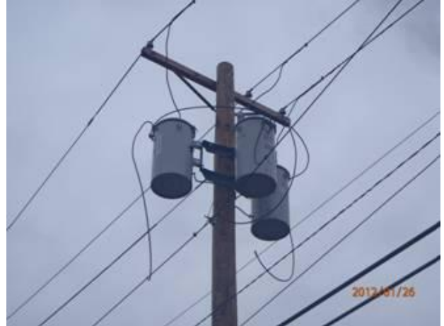
Power transformers installed by PSE&G for the UPF Site.
