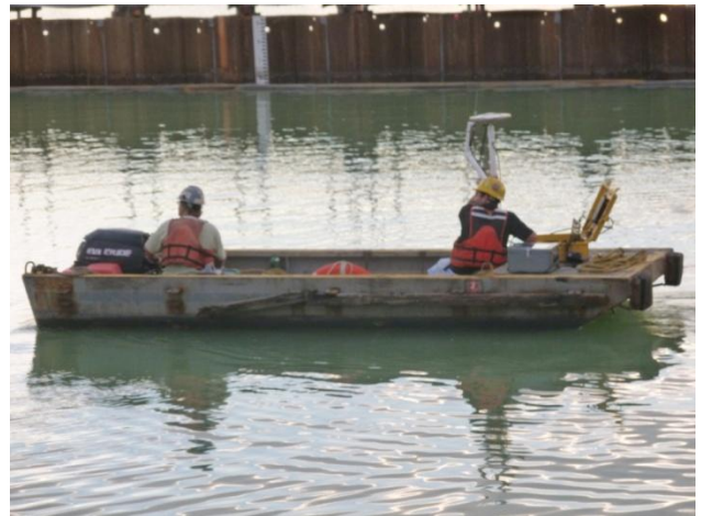
Team performing sounding for backfill placement
