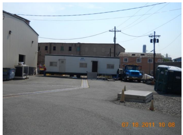
Weeks Marine construction trailer during installation
