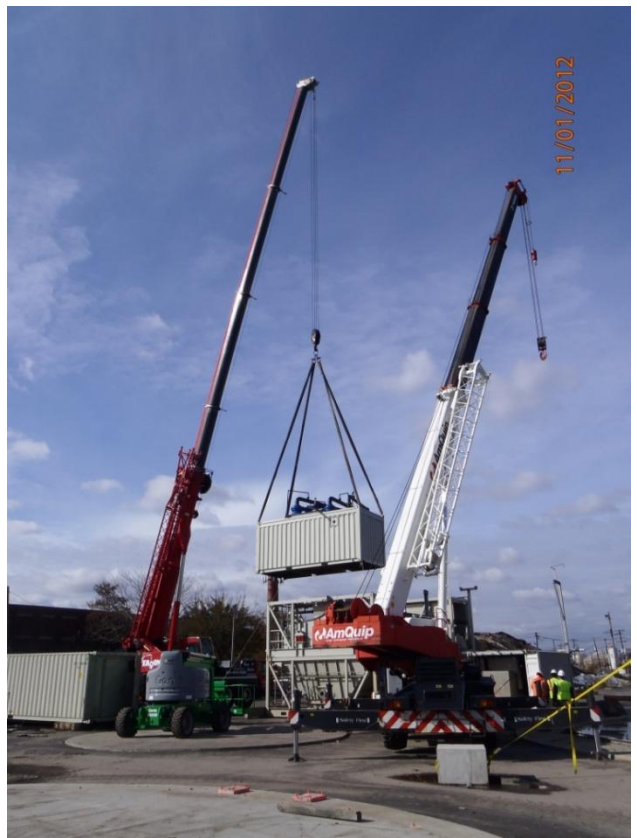
Removal and Disassembly of shaker screen equipment of the sediment processing system
