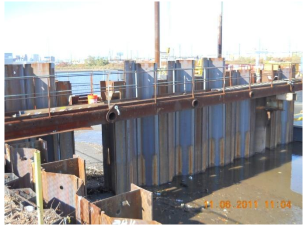
Enclosure construction for the west wall
