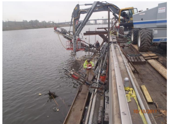
Tieback stressing and performance testing
