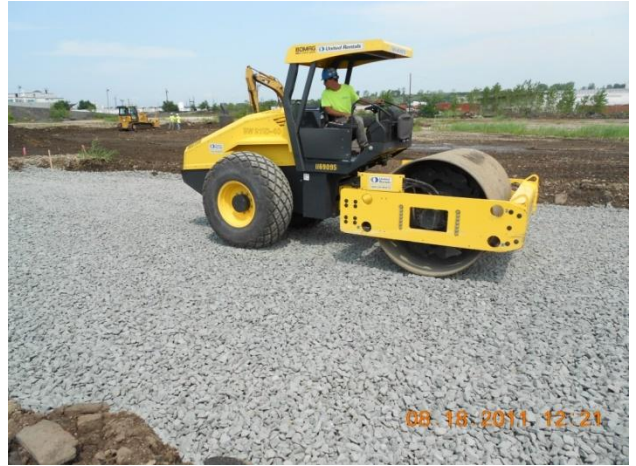
Proof rolling subgrade materials at the UPF
