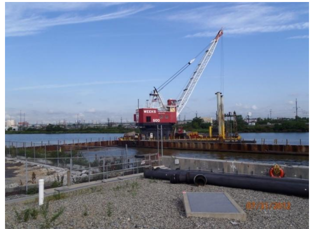
Enclosure backfill operations
