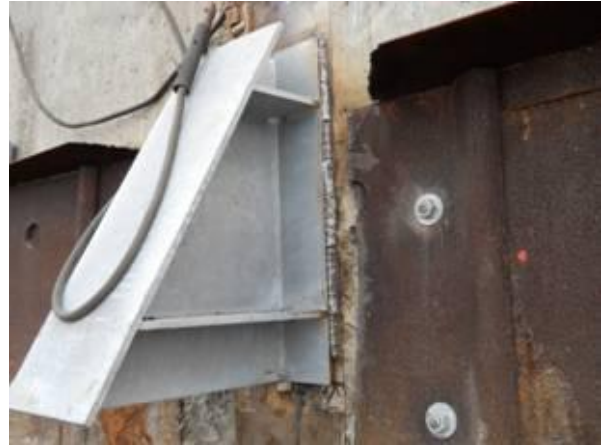
Shoes installed along the OU-1 flood wall
