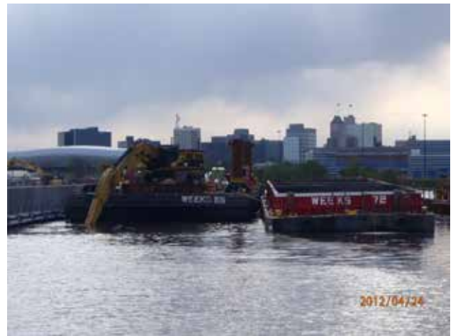
Dredging in the west half of the enclosure
