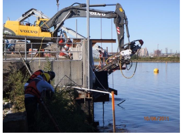
Tieback installation along the OU-1 flood wall
