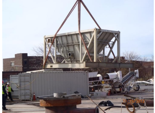
Removal and disassembly of the hopper on the sediment screening system
