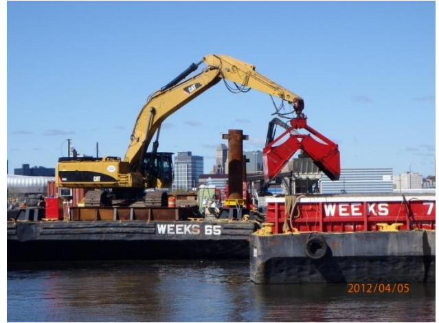
Dredge excavator dredging sediment
