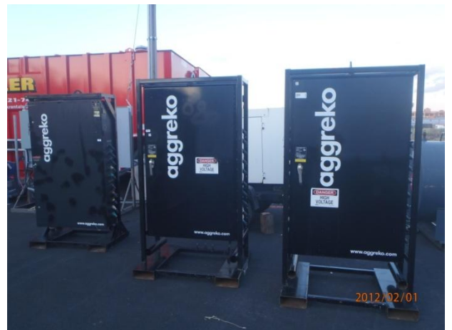
Generator panels for sediment processing
