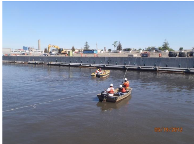
Collection of sediment sounding data
