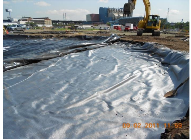
Liner and geotextile materials during installation of Equipment Pad #8.
