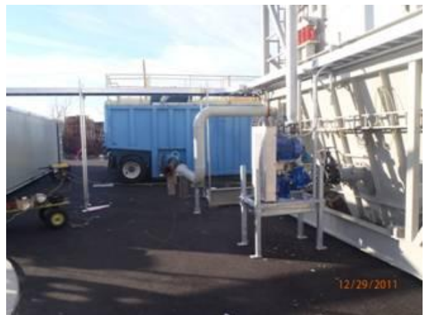
Installation of piping for sediment processing system
