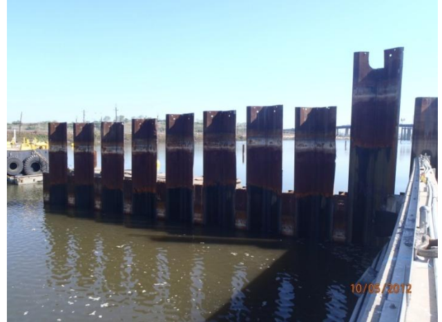
Removal of the east wall of the enclosure
