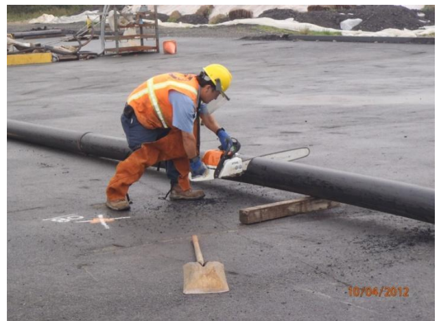
Sectioning of discharge piping
