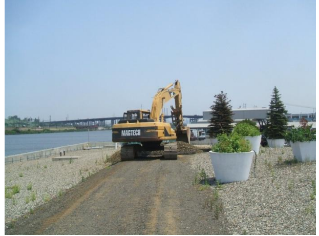
Access road construction at the OU-1 Property
