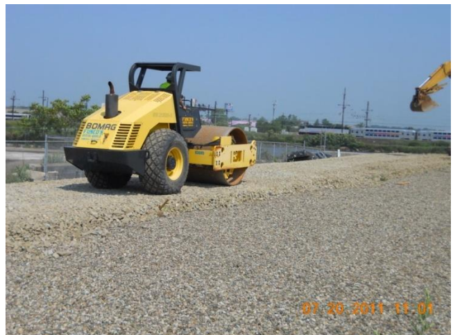
Compaction of access road improvements at the OU-1 Property
