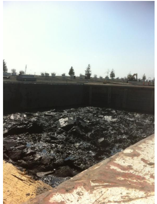
Dredged material in the material barge during dredging
