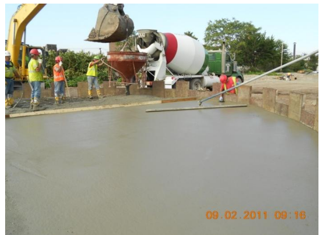
Installation of concrete for Pad #11
