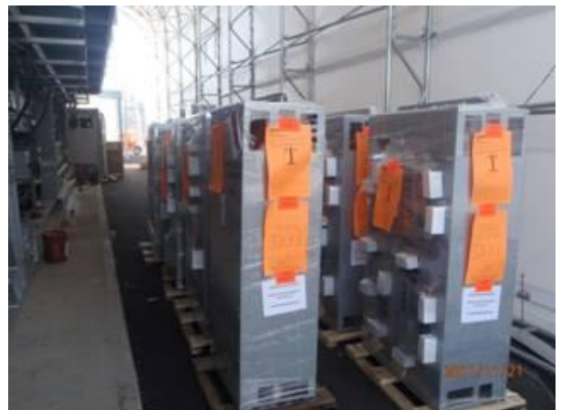
Motor control panels for the sediment processing system
