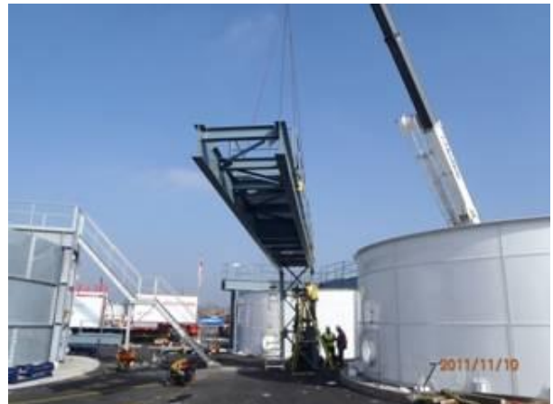
Bridge installation on one of the sludge holding tanks
