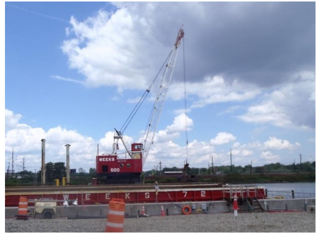
Enclosure backfill operations
