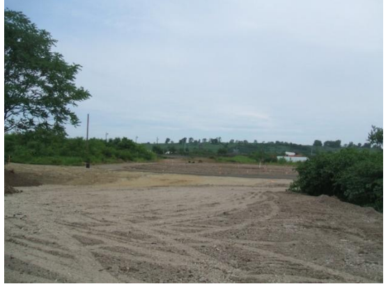
UPF after grading by the Property Owner
