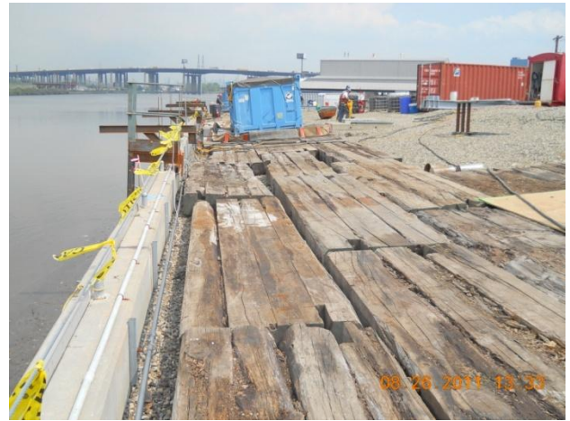
Work areas along the OU-1 Floodwall
