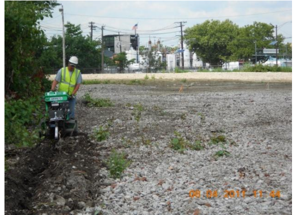
Silt fence installation along southern property boundary at UPF site
