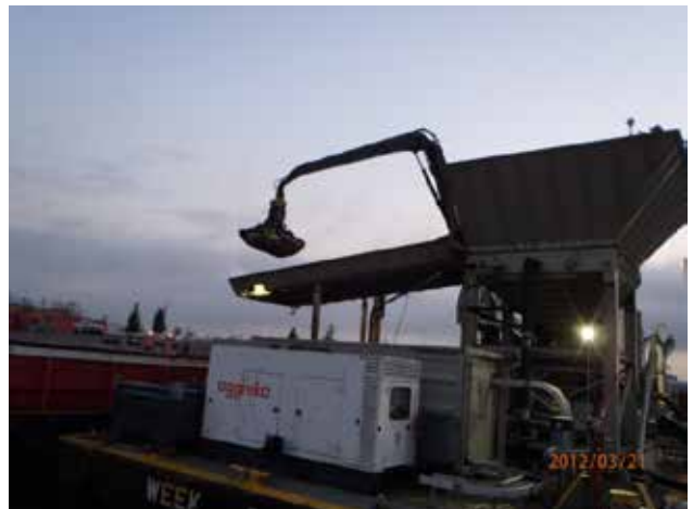
Screening dredged material at the enclosure
