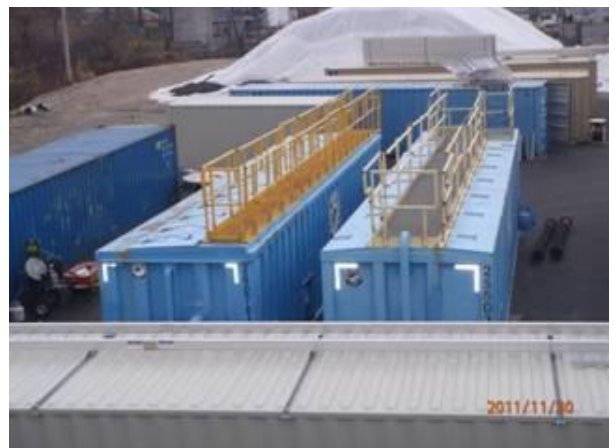
Sediment processing system contingency tanks
