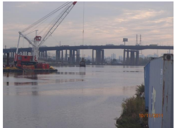
Scour protection material placement
