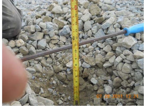
Performing quality control confirmation measurements on improved access road at the OU-1 Property
