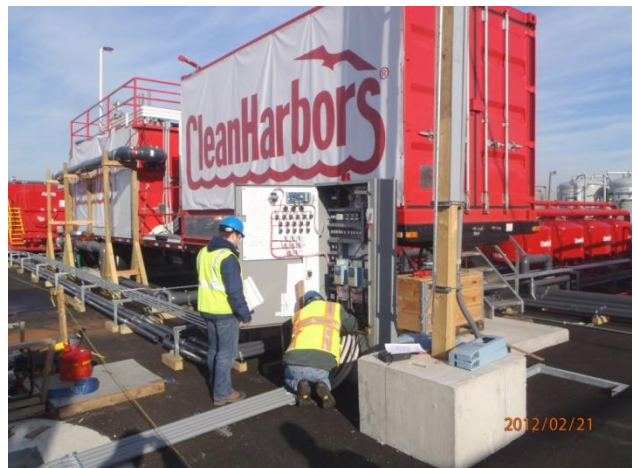
Energizing the storm water pump system
