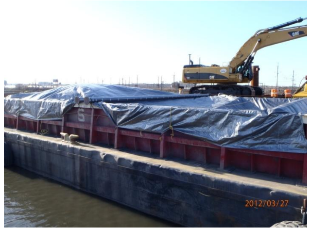
Tarped material barge at the enclosure
