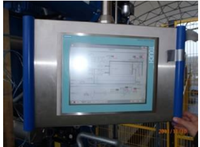
Membrane filter press control panel energized
