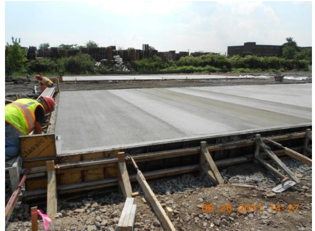
North filter press pad poured and screed
