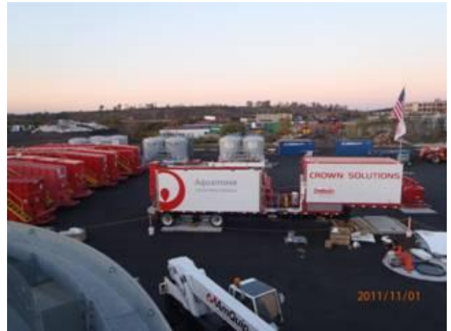
View of water treatment system from the filter presses
