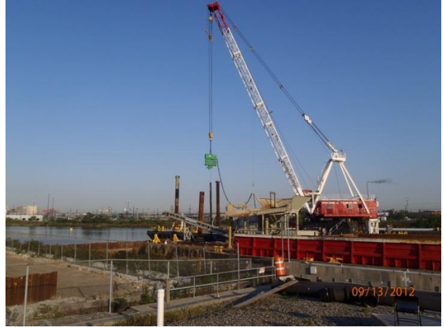
Removal of piles on the west wall of the enclosure
