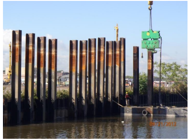
Removal of king piles in front of the Sherwin Williams property
