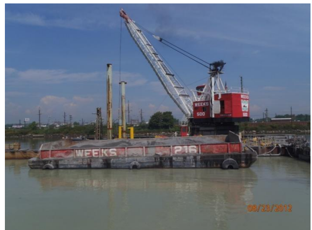
Enclosure backfill operations
