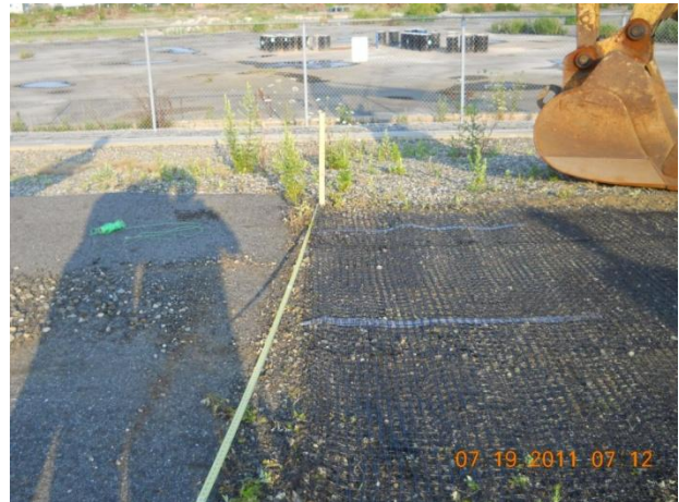
Geogrid material during access road construction
