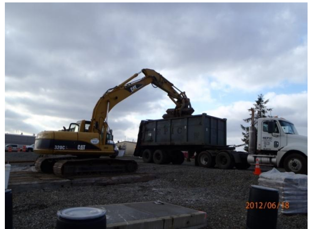
Debris load-out activities at the OU-1
