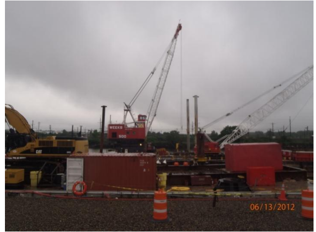
Mobilization of crane for concrete mattress removal and backfill activities
