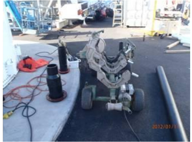
HDPE fusion welder for piping at the sediment processing system
