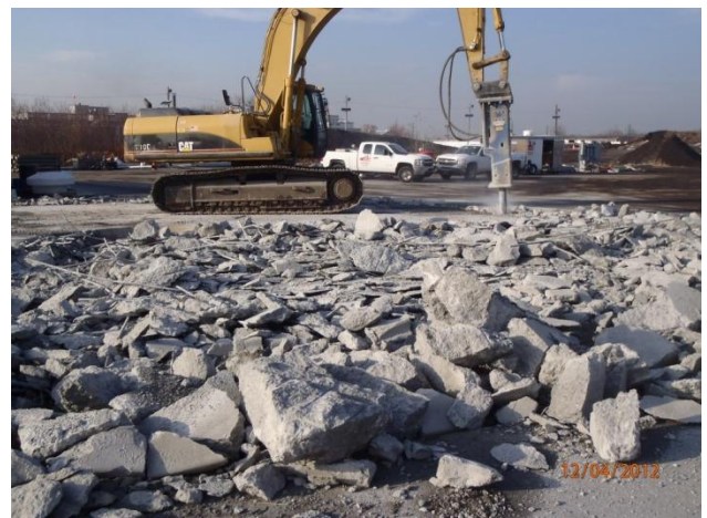
Gravity thickener pad removal
