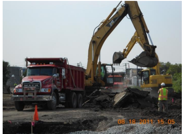
Excavation and grading of UPF soils
