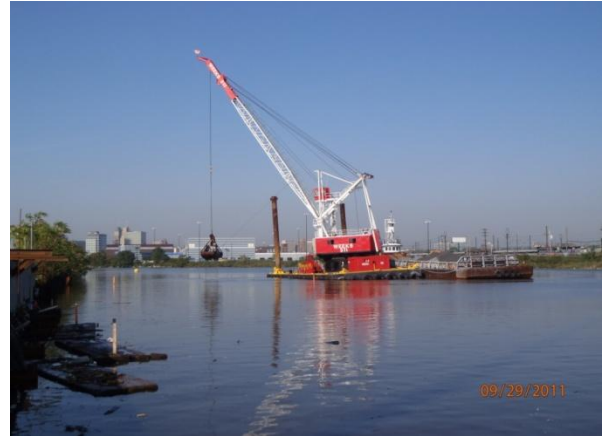
Barge crane installing scour protection material
