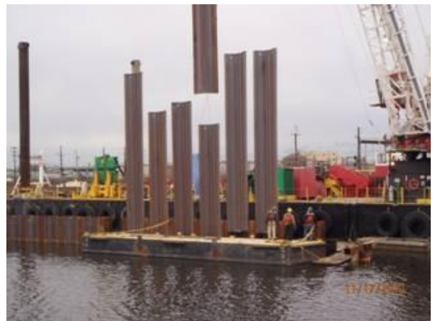
Pile installation for the north wall of the enclosure
