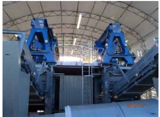
Filter press deck
