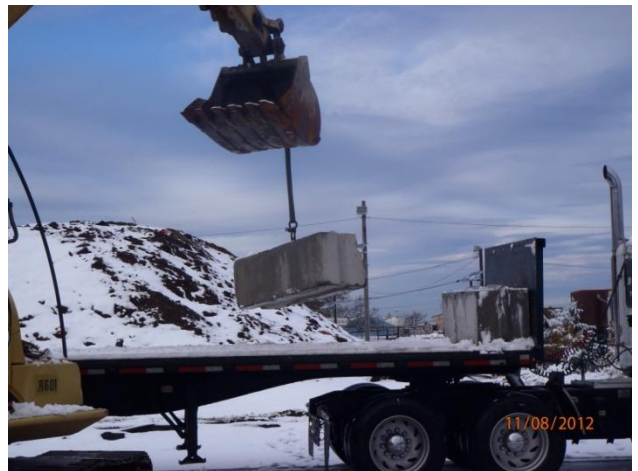
Removal of concrete blocks from the UPF
