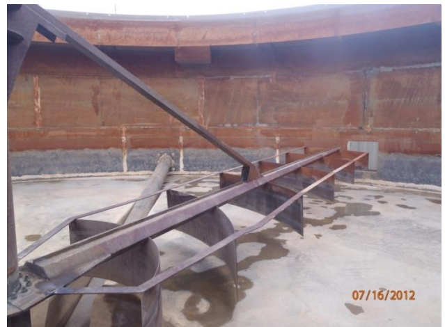
Cleaned interior of the sludge thickener tank
