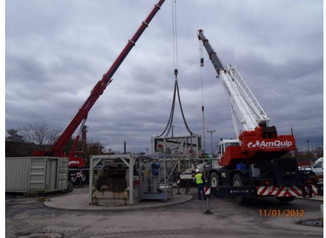
Removal and Disassembly of shaker screen equipment of the sediment processing system
