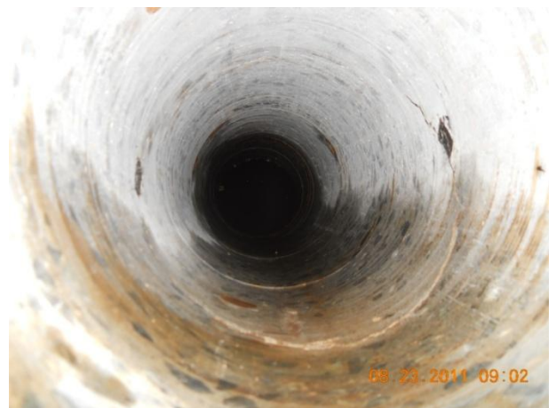
View into a concrete core into the OU-1 Floodwall
