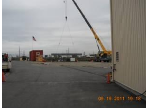
Wale installation along the OU-1 flood wall
