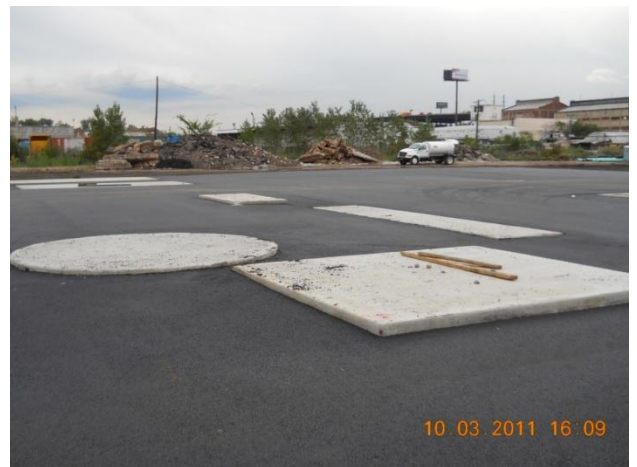
Finish asphalt and equipment pads at the UPF
