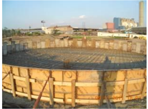
Equipment Pad 10 prior to concrete pour
