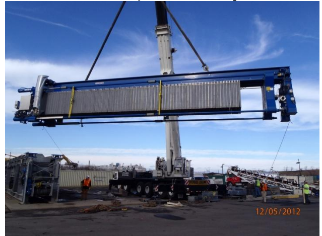
Removal and loading of filter press
