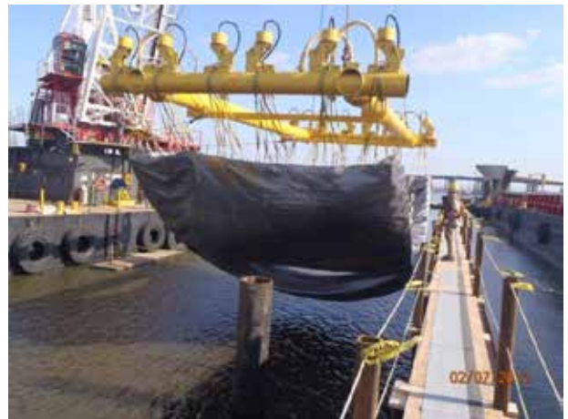
Installation of concrete mattress for scour protection
