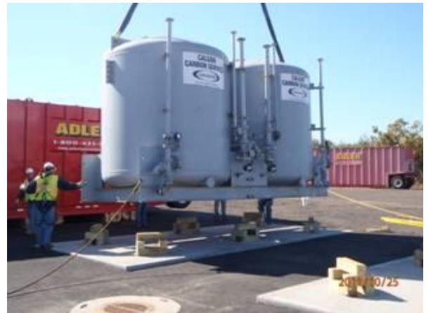
Installation of carbon vessels for water treatment system
