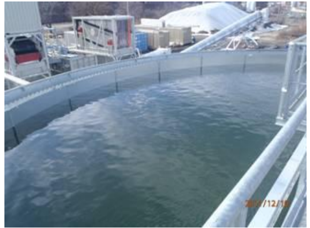
Gravity thickener with water for system operational and leak testing
