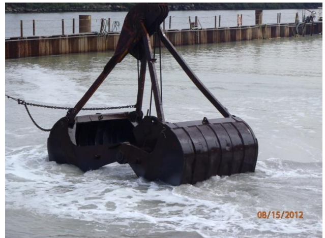
Enclosure backfill operations
