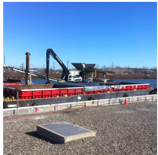
First material barge in position for offloading dredged material
