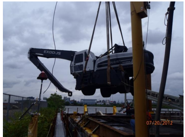
Offloading of excavator from the barge
