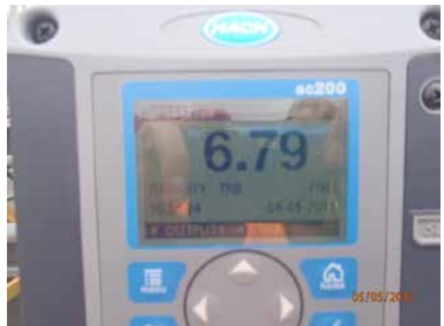
Turbidity monitoring for the water treatment system
