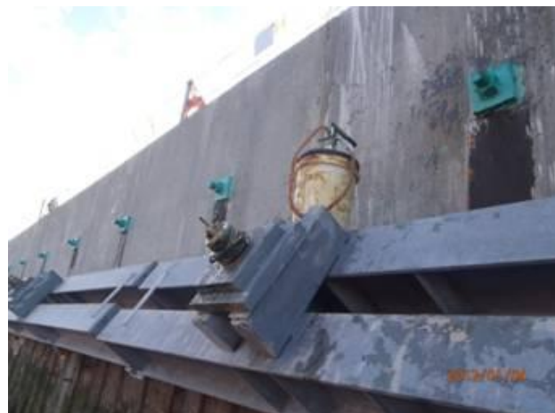
Finishing and corrosion protection activities for the tiebacks
