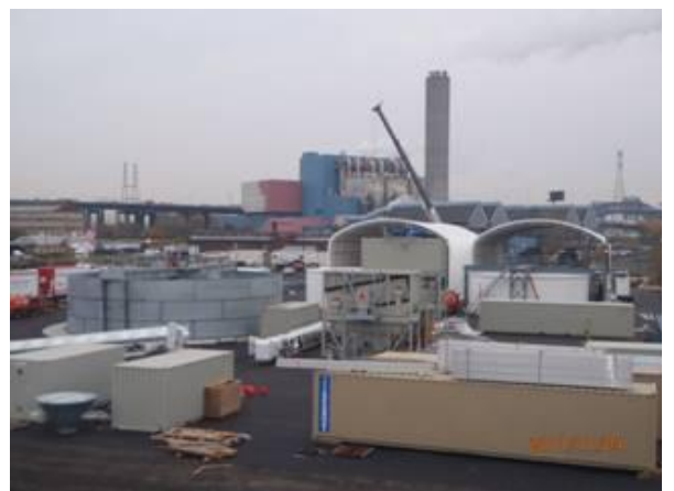
Sediment processing system construction looking east
