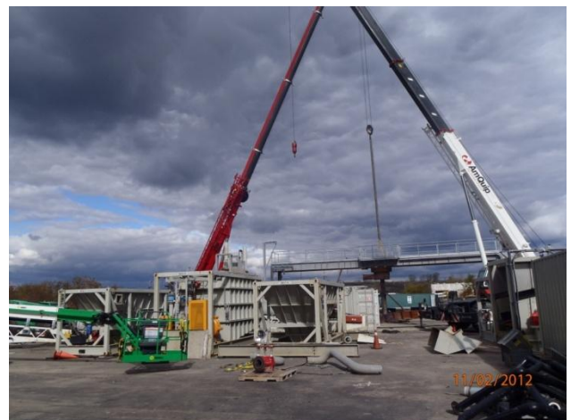
Removal and Disassembly of gravity thickener bridge of the sediment processing system
