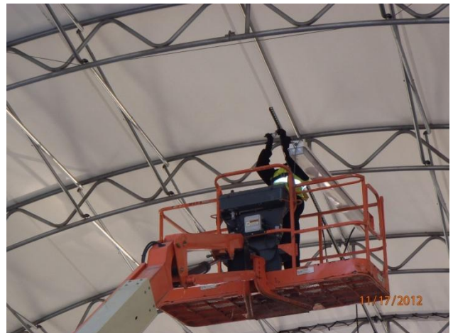
Removal of lighting in preparation of canopy disassembly
