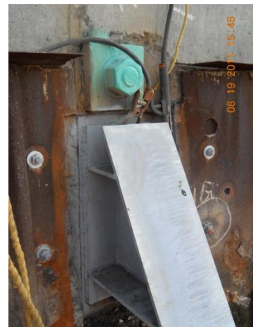
Shoe for the wale installed on the OU-1 flood wall
