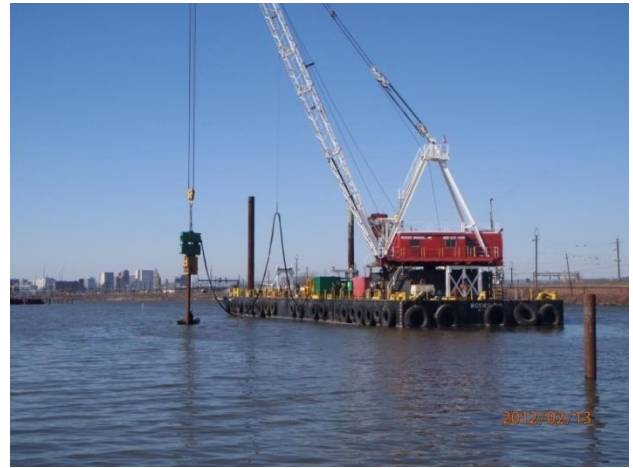
Installation of anchoring monopile for the hydraulic pipeline
