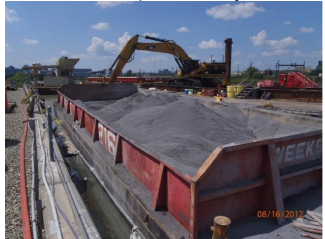
Enclosure backfill operations
