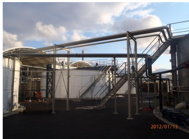
Sediment process piping installed
