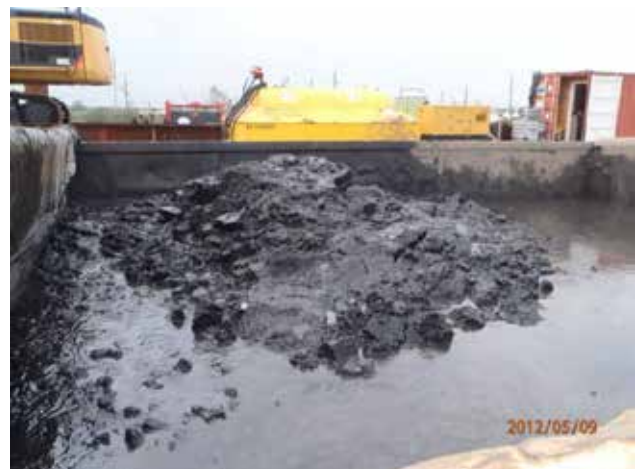
Dredged sediment in a material barge
