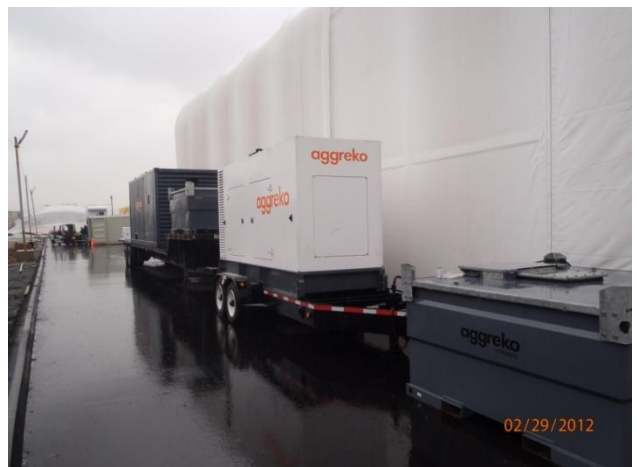
Generators for sediment processing system
