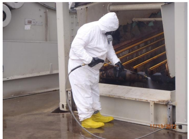
Final decontamination of equipment during disassembly
