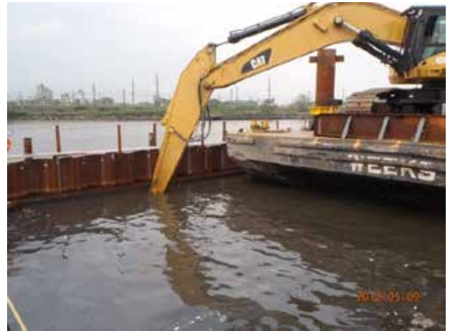
Dredging along the enclosure wall
