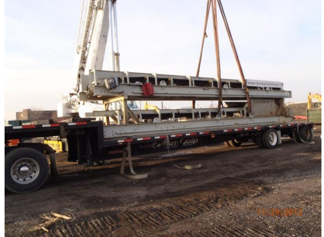
Removal and disassembly of the conveyor on the sediment screening system
