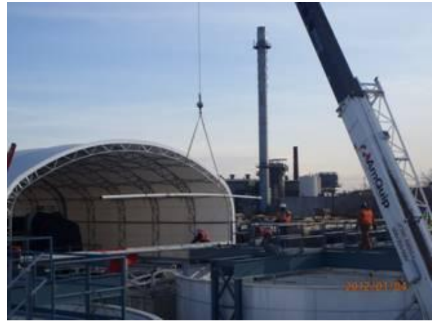
Installation of piping for sediment processing system
