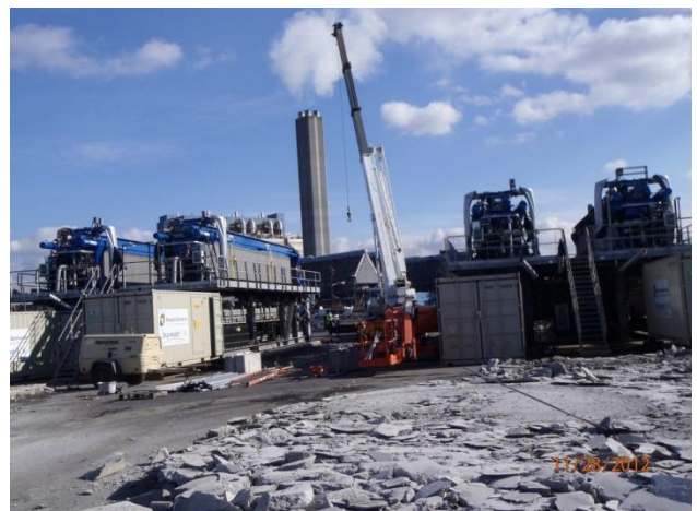
Canopy removal from the filter presses
