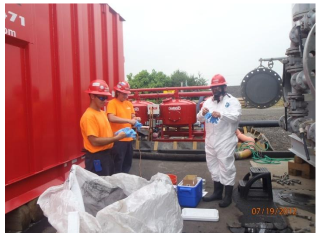
Crew working on cleaning water treatment equipment
