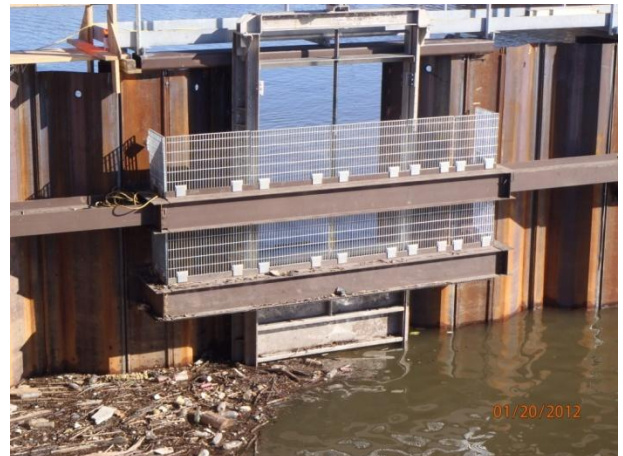
View of weir gate in the east wall of the enclosure
