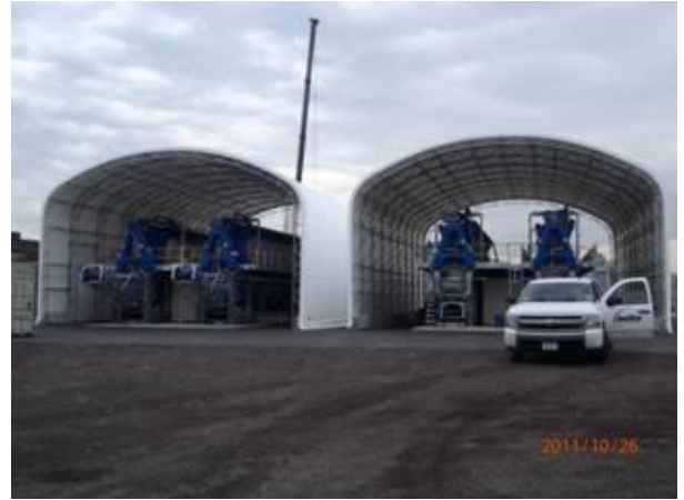
Completion of canopies over the membrane filter presses
