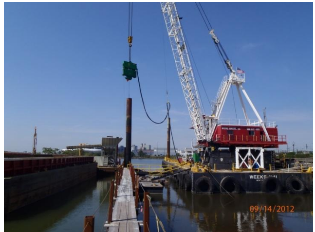
Removal of piles on the north wall of the enclosure
