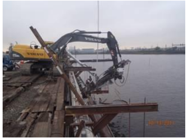
Tieback installation along the OU-1 flood wall
