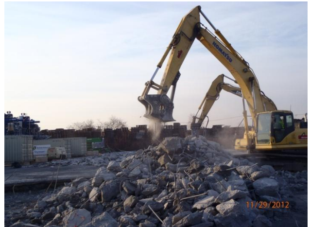
Processing of foundation pad material
