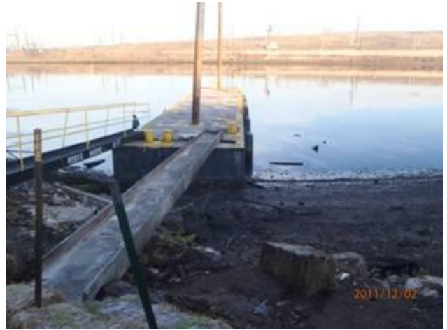
Beginning to establish support structures at the river's edge at the UPF
