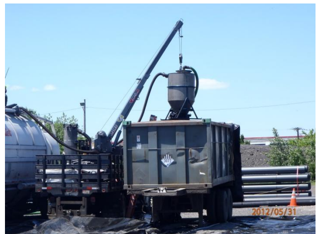
Spent carbon placement in intermodal containers
