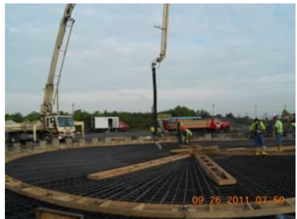
Reinforcement bar and forms for the Gravity Thickener
