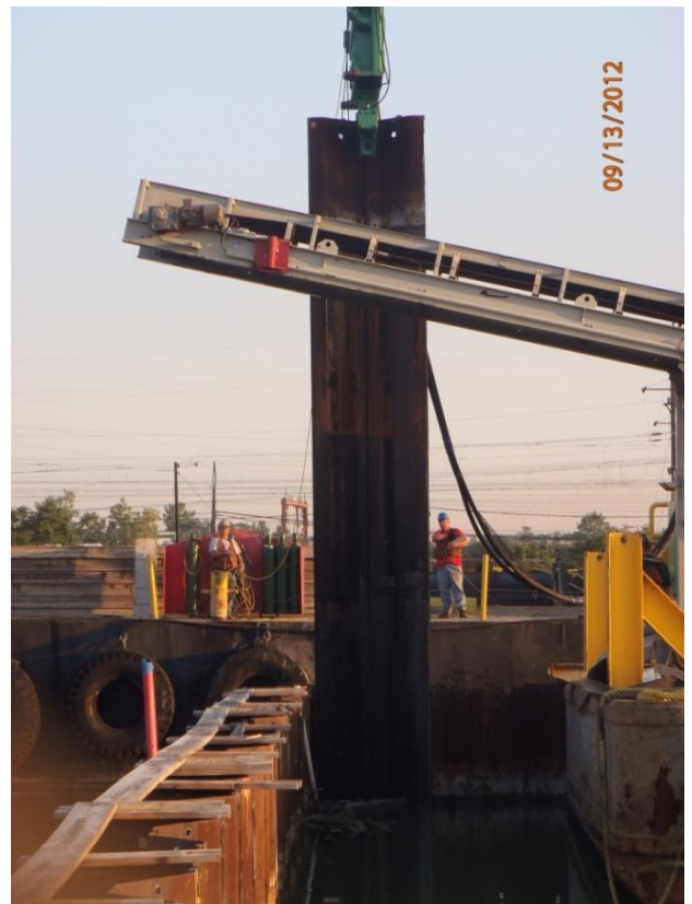
Removal of the first pile from the enclosure
