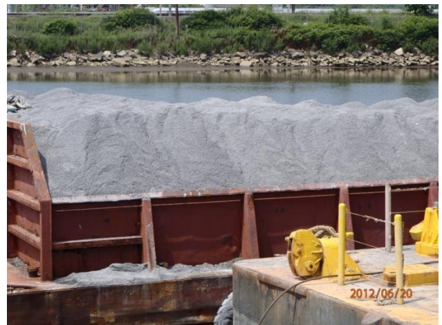
Delivered backfill material
