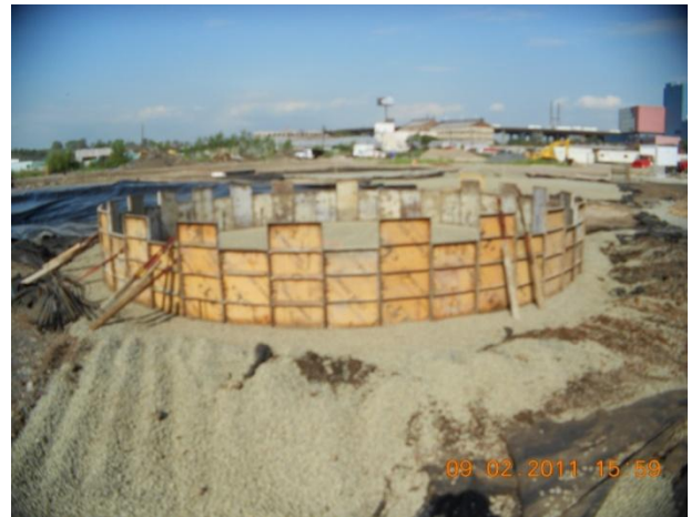
Concrete forms during installation of Equipment Pad #9.
