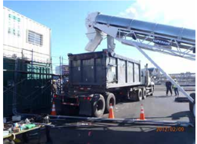
Testing and programming of the UPF conveyors
