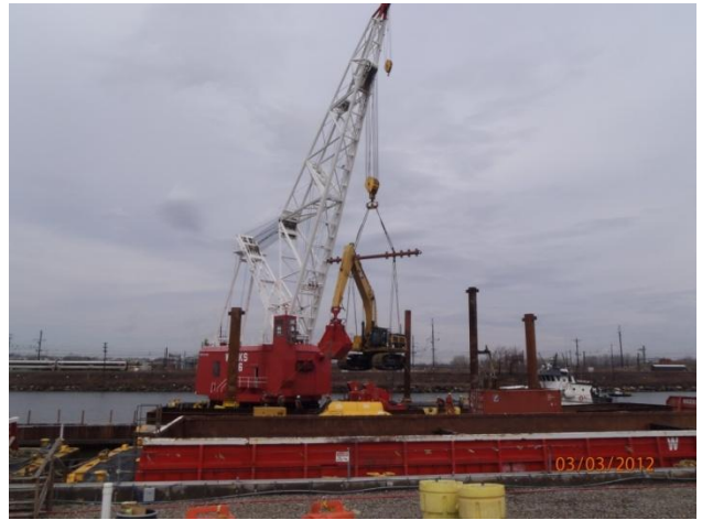
Loading the dredge excavator on to the barge within the enclosure
