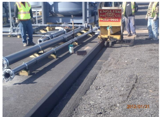
Curb installation at the UPF
