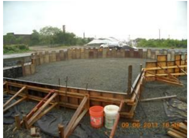
Forms installed for Equipment Pad #9
