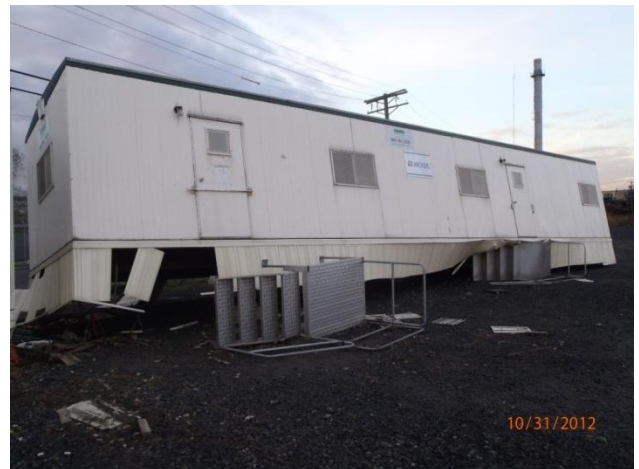
Impact to site support equipment from Hurricane Sandy
