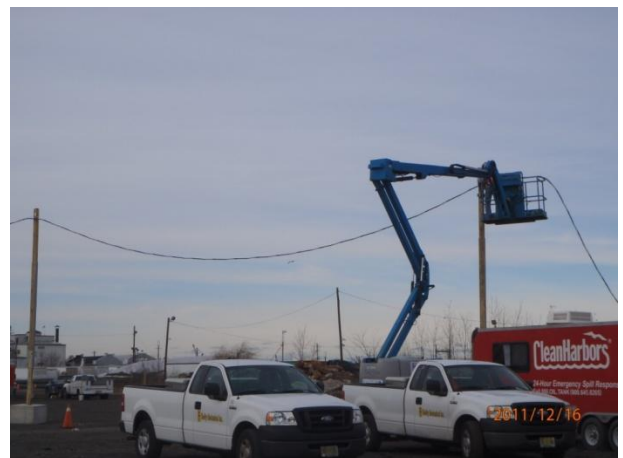
Installation of site electrical and lighting
