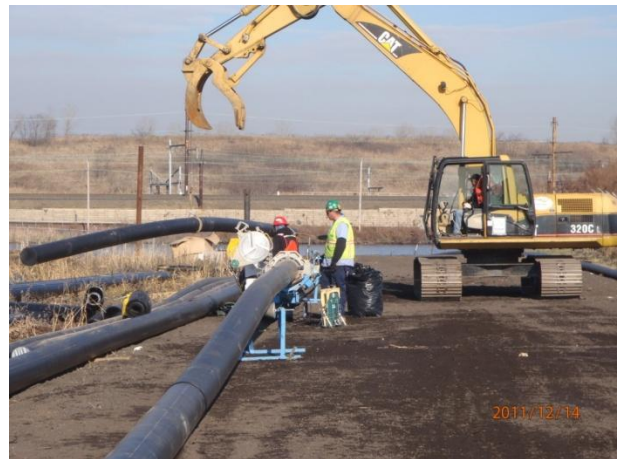
Welding of sections of the hydraulic pipeline
