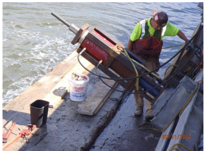
Restressing of an OU-1 tieback
