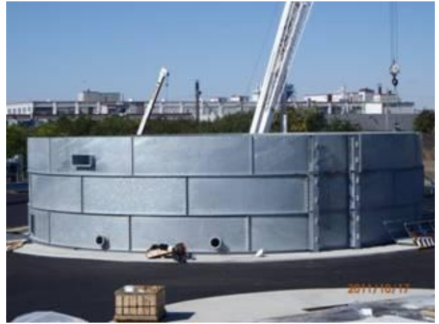
Gravity thickener tank installed at the UPF
