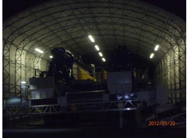
Filter presses at night
