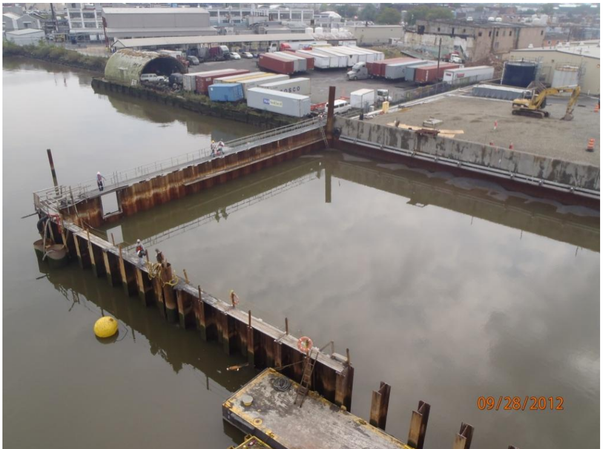
View of the remaining installed portion of the enclosure north and east walls
