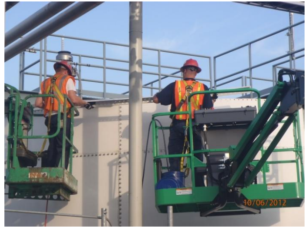
Disassembly of a sludge storage tank at the UPF
