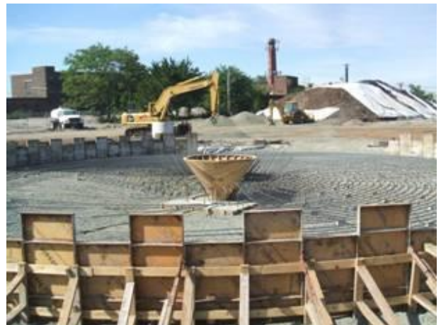
Reinforcement bar and forms during installation for gravity thickener
