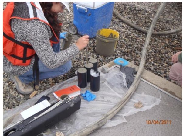
Grout sample collection for tieback installation
