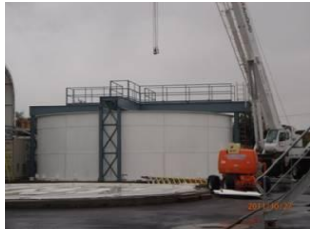
Installation of the bridge for the gravity thickener
