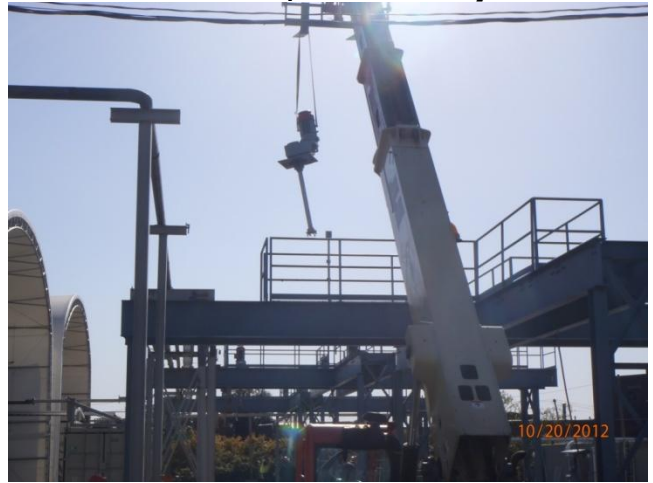
Removal of agitation motors from a sludge holding tank
