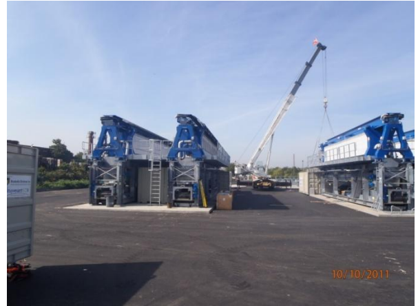
Membrane filter presses installed at the Site
