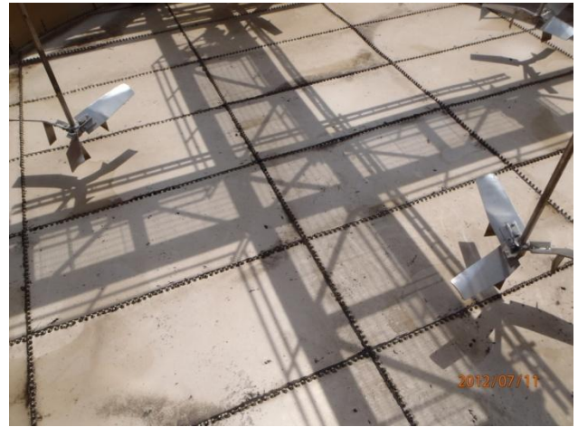
Inside of cleaned sludge storage tank
