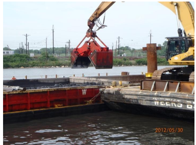
Dredge and material barge
