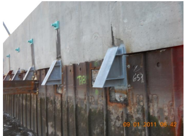
Shoes for OU-1 Flood Wall wale installed
