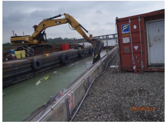
Enclosure backfill operations
