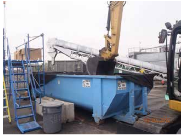
Coarse solids solidification and loading operation
