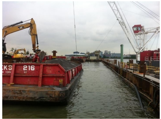
Enclosure backfill operations
