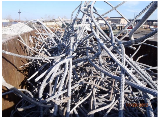
Rebar from the pad foundations separated for recycling
