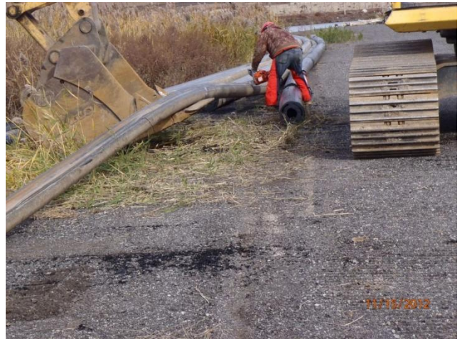
Preparation of HDPE piping for removal from the UPF
