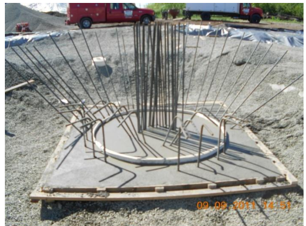
Gravity thickener slab base poured
