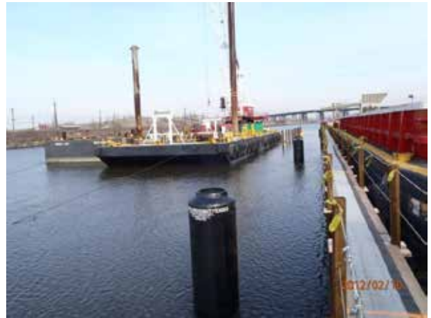
Installation of dolphins and protective donuts
