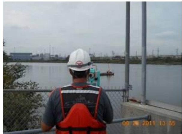
Construction staking of the enclosure limits
