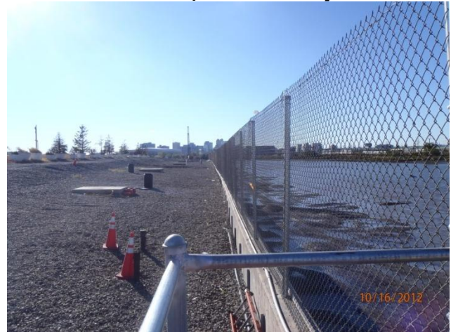
Reinstalled fence along the OU-1 Floodwall
