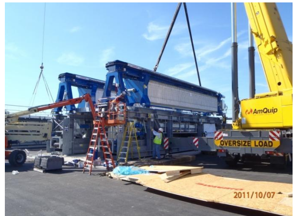
Installation of membrane filter presses
