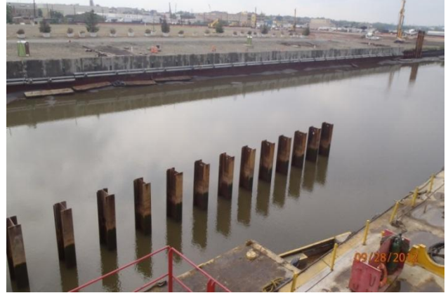
Portion of north wall with sheet piles removed
