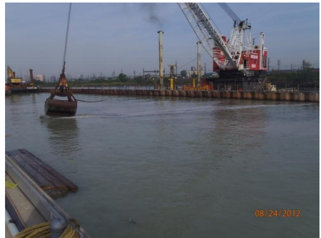
Enclosure backfill operations
