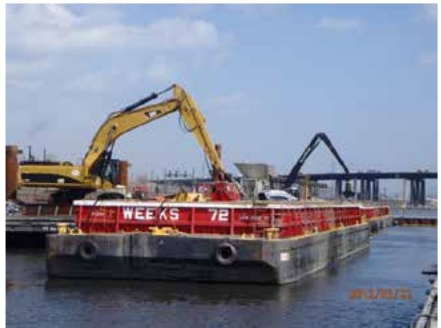
Placement of dredged sediment in a material barge
