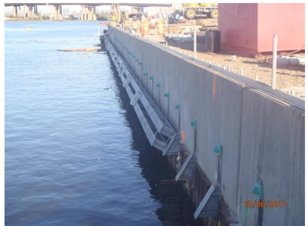
Wales installed along the OU-1 flood wall
