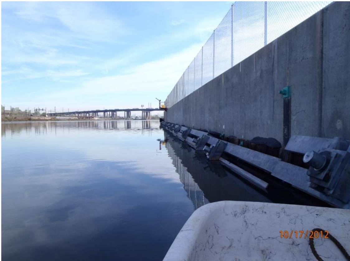
Sediment removal area and OU-1 Floodwall upon completion of work activities
