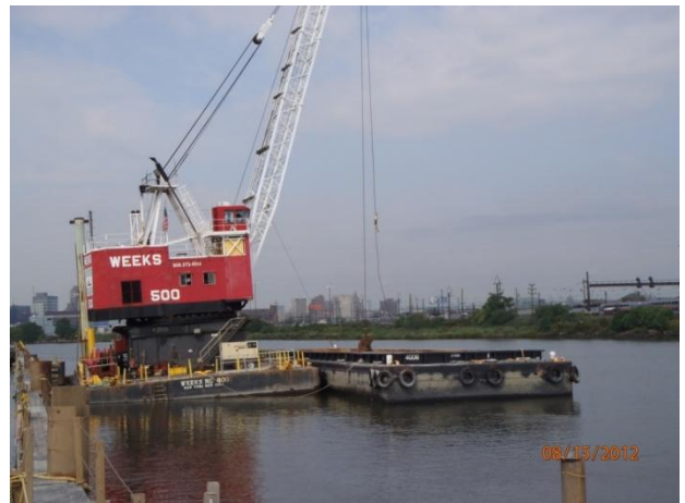
Enclosure backfill operations
