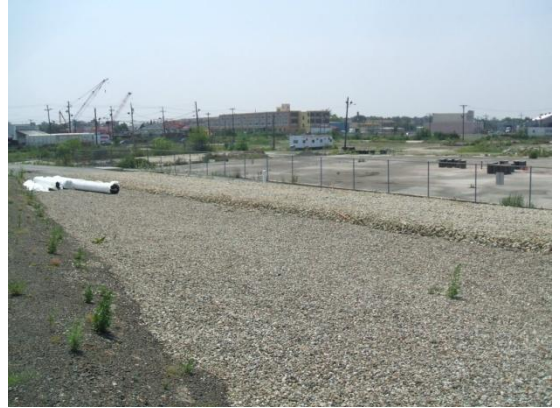
Completed improved access road at the OU-1 Property
