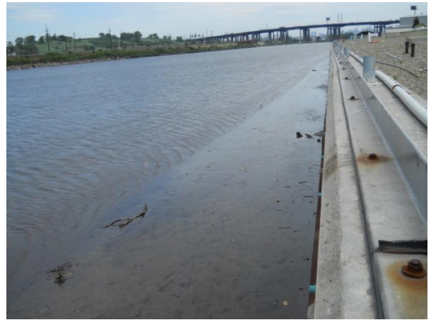
View along the OU-1 Property floodwall with fence removed
