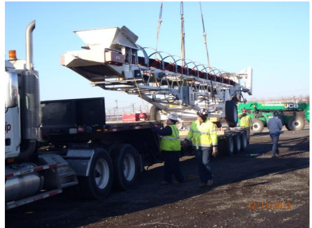
Loading of conveyor for demobilization
