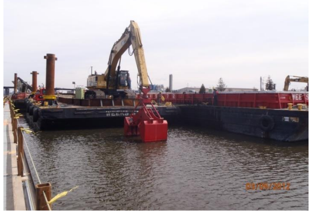
Dredging operations inside the enclosure
