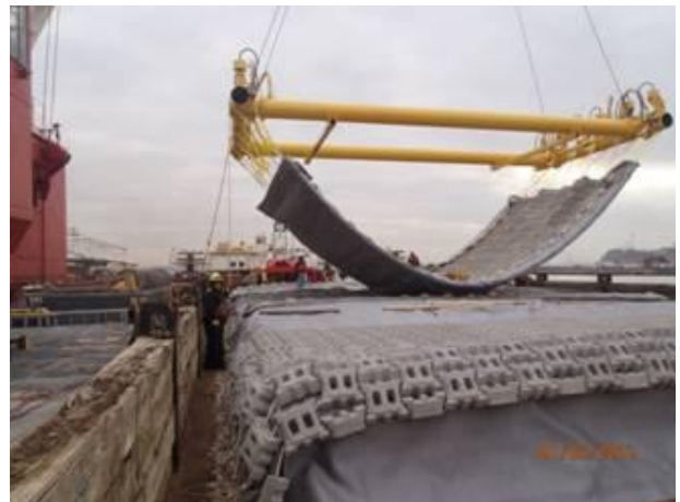
Test of spreader bar from concrete mattress installation
