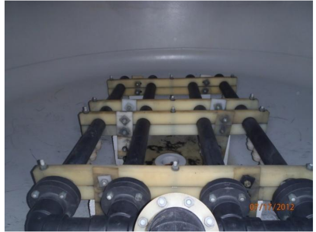
Cleaned interior of the carbon vessels
