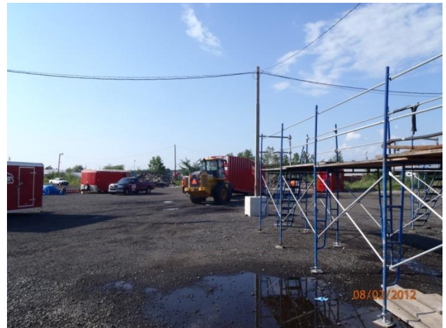
Demobilization of treatment system components
