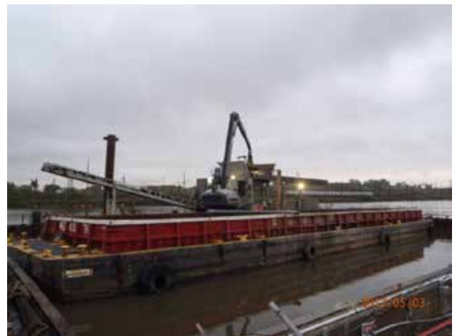
Removing material from the material barge for screening
