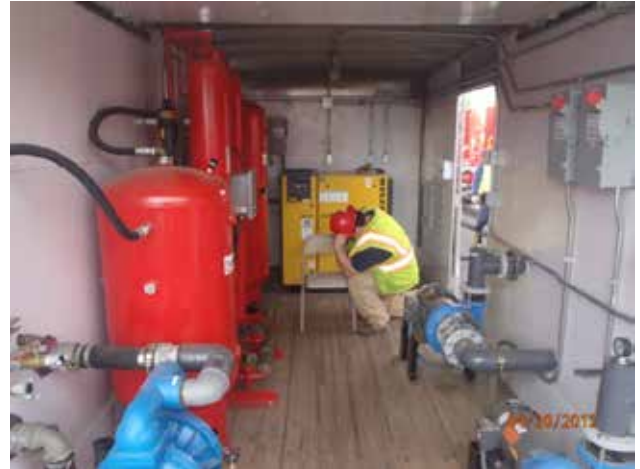
Operation and Maintenance Activities in the Water Treatment System
