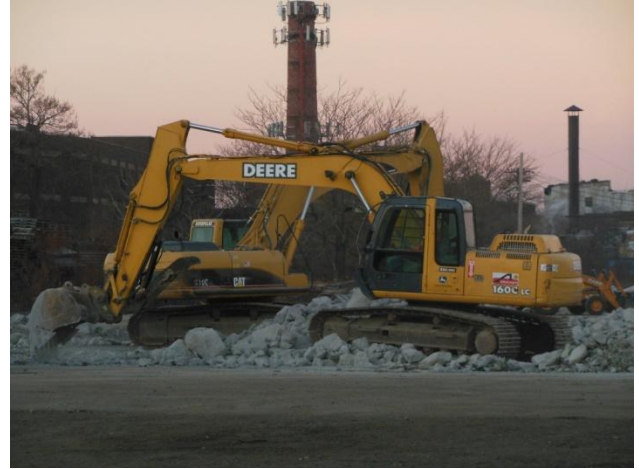
Removal of equipment pads and preparation of concrete material for crushing
