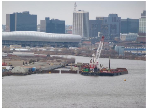
Enclosure and barges as seen from the East
