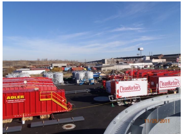
Water treatment system
