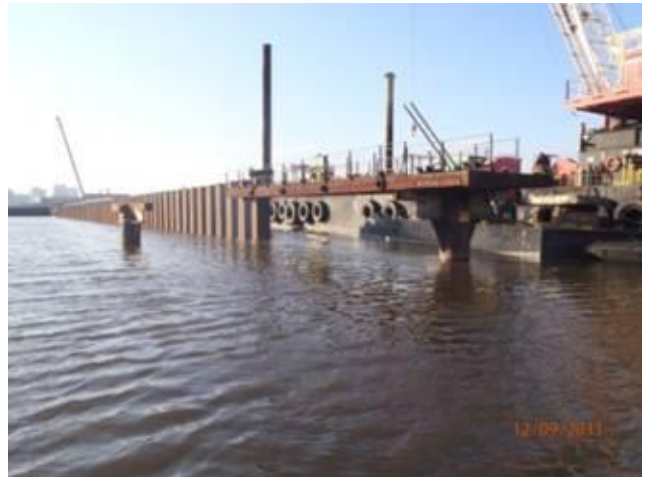
Installation of the final template for the north wall
