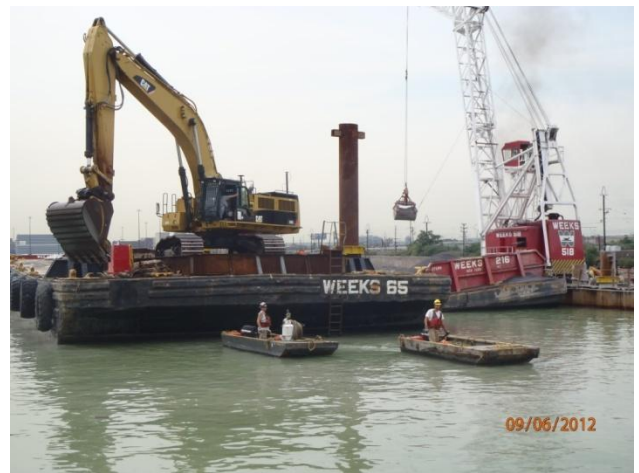
Enclosure backfill operations
