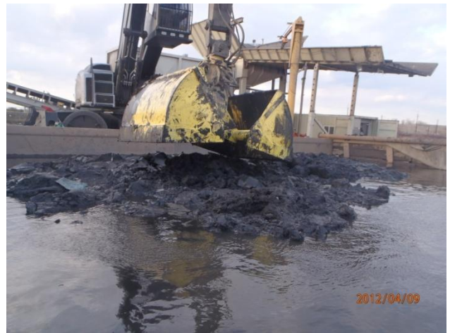
Removal of dredged material from barge for screening
