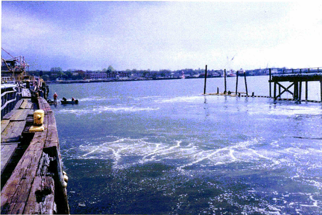
Photo 1 - Air Curtain Operation, View from Pier 3 Facing KVK Channel
