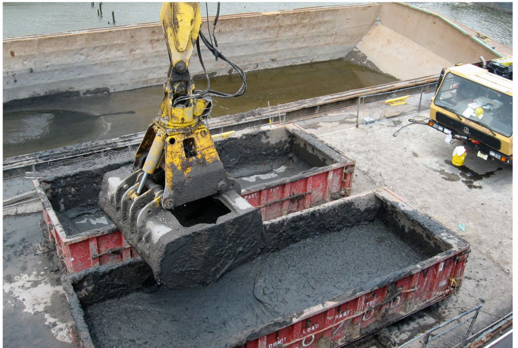
Clean-out of Upfront Storage Facility (clockwise from top: Loading Box with Residual Sediment, Lifting Box Overhead, Unloading Box into Scow, Pressure Washing Cargo Hold)
