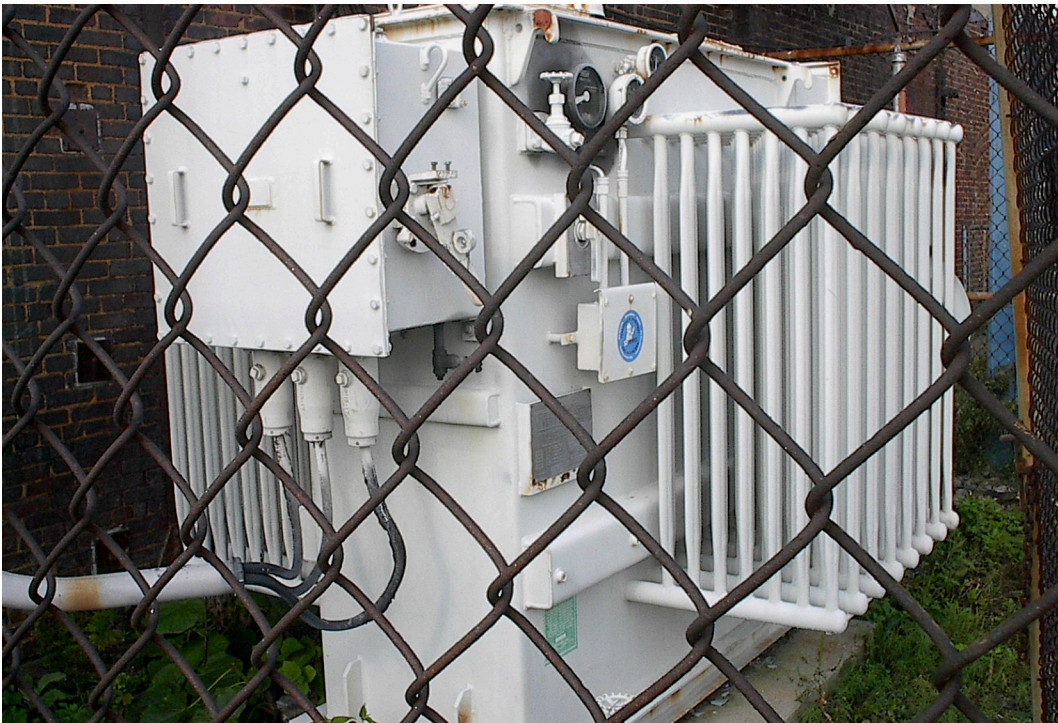
Power Supply (clockwise from top: Main Generator, Secondary Generator, Transformer)
