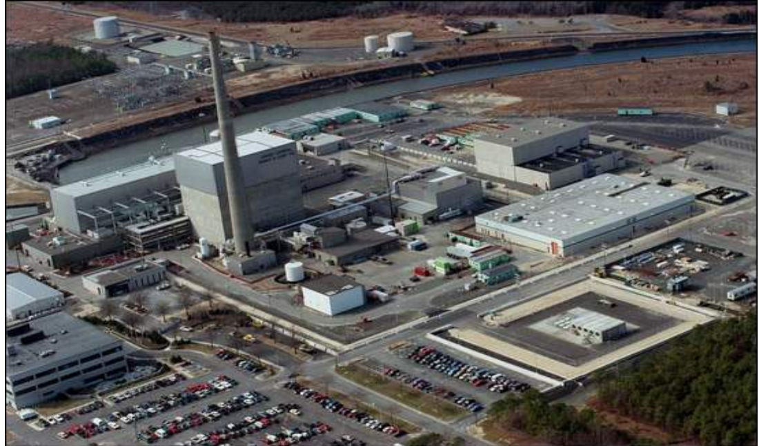
Figure 5 – Oyster Creek Nuclear Generating Station, Forked River, NJ
