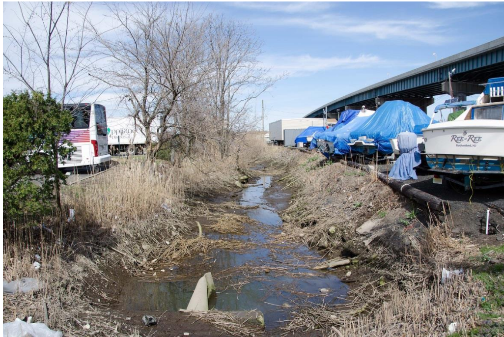
Existing conditions at ditch #2
