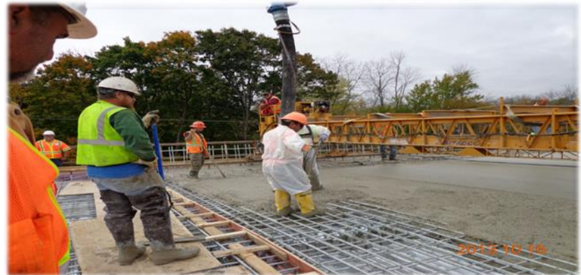
20131016 PC E07 11 32 36 Concrete deck placement
