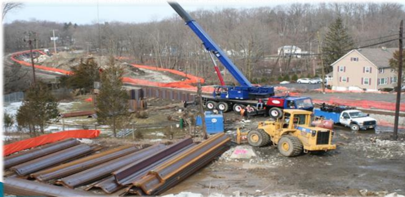
20131015 PC E07 Driving pier 25 004
