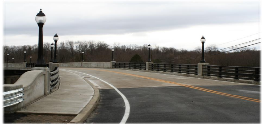
20131230 PG 507 Site viewed from Fowler St Intersection looking NW 004
