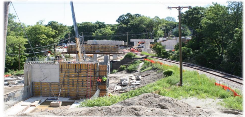
9-07-20130303 Site viewed from small storage at west end 030 v3
