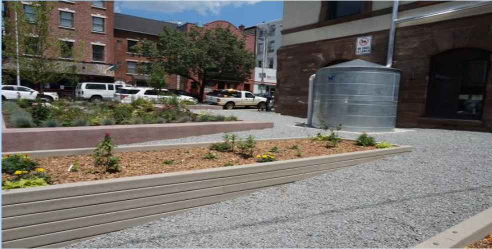
Porous Pavement & Rain Garden - Hoboken City
