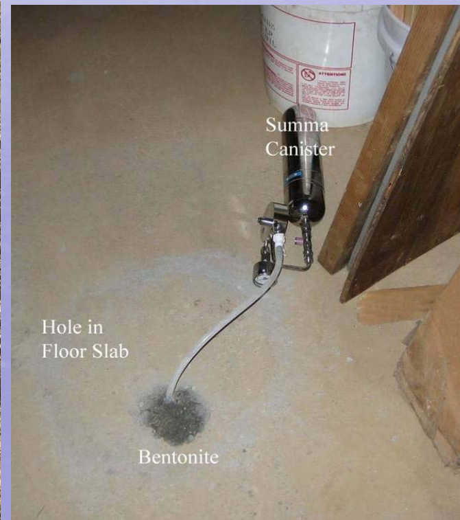
Typical Sub-Slab Vapor Sampling
