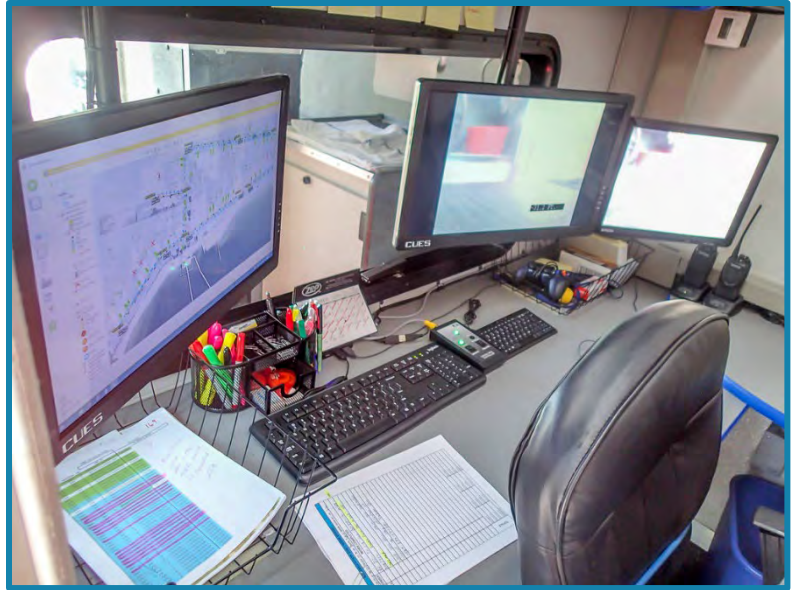
Toms River Municipal Utilities Authority Equipment Purchase
