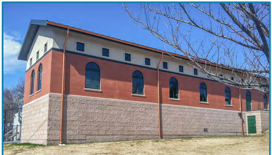
Milltown Borough Electrical Substation Relocation
