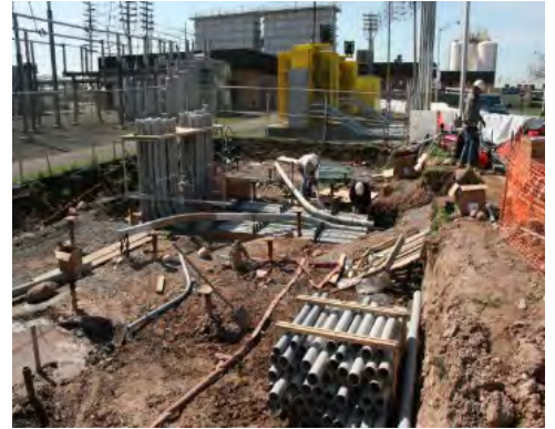
Passaic Valley Sewerage Commission Electrical Substation
