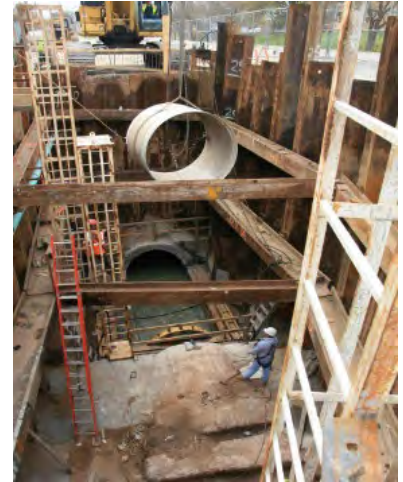
Passaic Valley Sewerage Commission Interceptor Slip Lining
