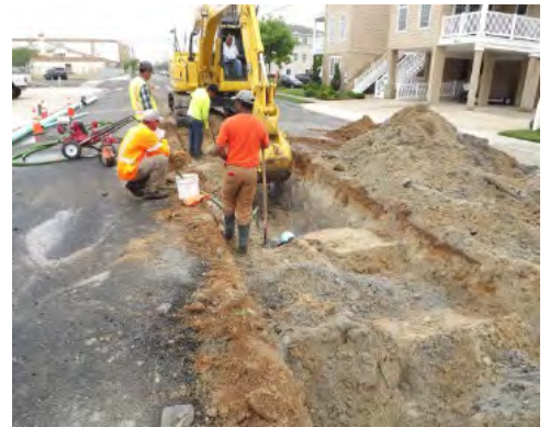
North Wildwood Sewer, Storm, and Street Restoration
