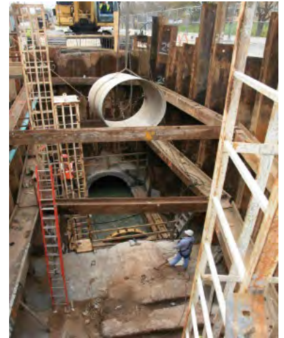
Passaic Valley Sewerage Commission Interceptor Slip Lining
