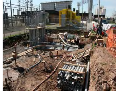
Passaic Valley Sewerage Commission Electrical Substation
