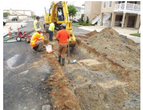
North Wildwood Sewer, Storm, and Street Restoration
