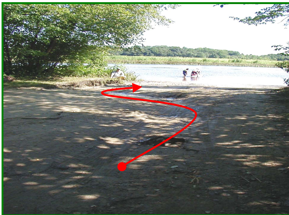
The arrow in this photograph delineates the gully that has formed due to upland runoff.
