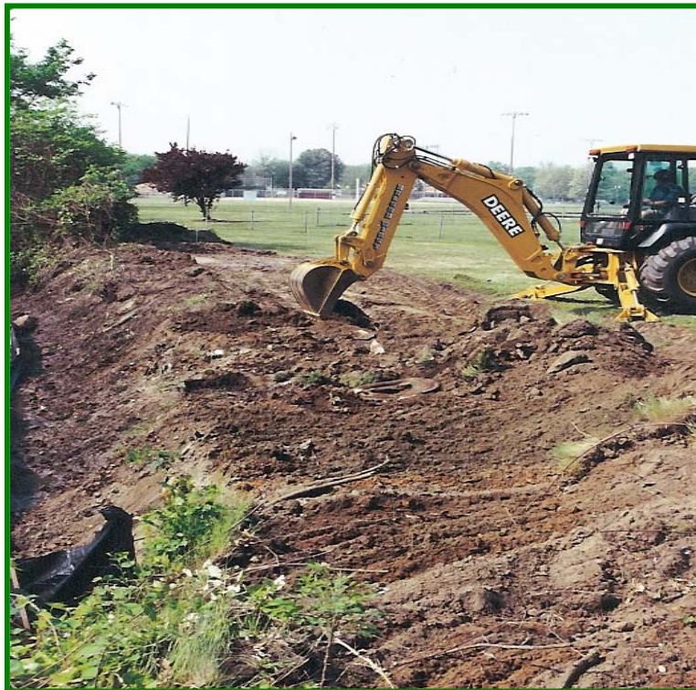
The excavation and re-shaping of the shoreline begins.
