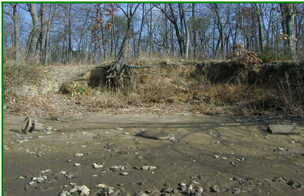
Implementing stabilization methods on this slope would prevent additional erosion.
