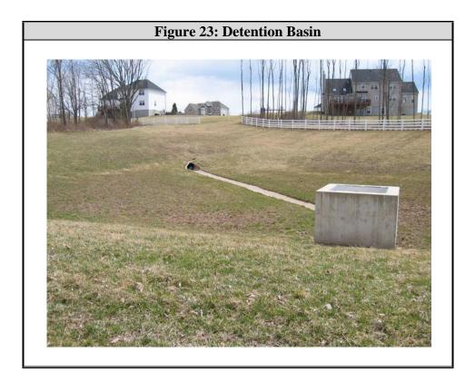
This type of structural BMP still has utility, especially in larger catchments, but is reflective of an older design philosophy less concerned with treatment and volume reduction and primarily focused on peak flow attenuation. For new development it is recommended that these systems be replaced with other structural BMPs such as
