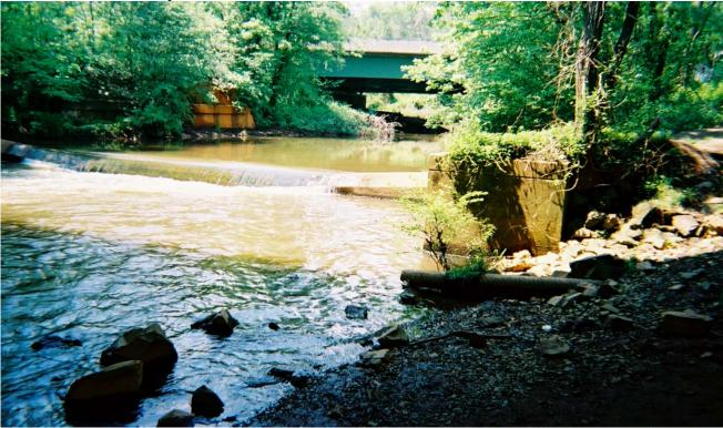
Run-off to Manasquan River at USGS Station 01408000 (Manasquan River at Squankum). Unconsolidated soil covers an unprotected slope and is washed down by runoff to a pool formed by a Squankum dam. The water quality sampling site 01408000 is approximately 60 feet from this site.
