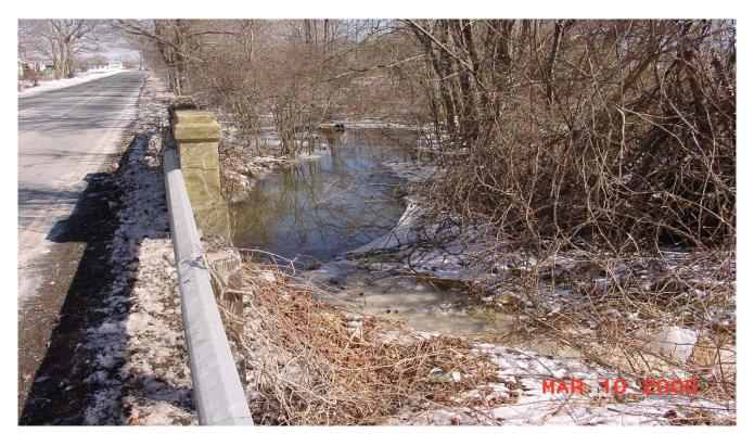
Long Brook at Howell. Fine sand and silty material is deposited into the stream bed by the runoff water. Sitly deposit fills approximately <sup>3</sup>/<sub>4</sub> of the total channel width.
