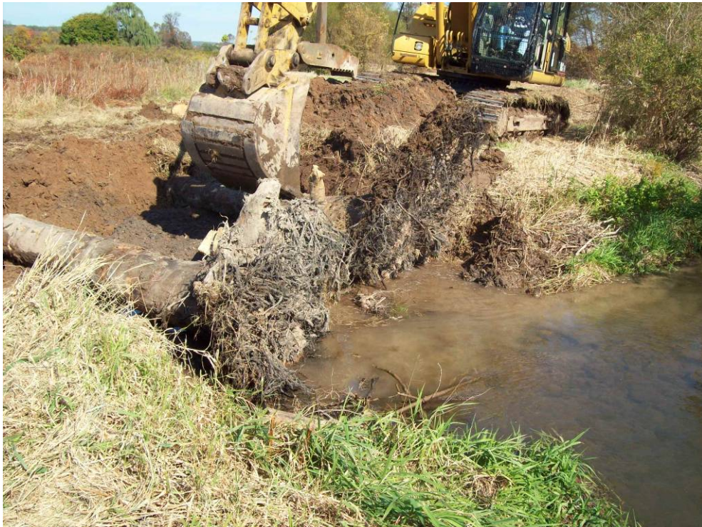
Figure 47: Rootwad Placement
