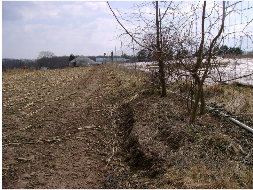
Figure 56: Eroded Ditch
