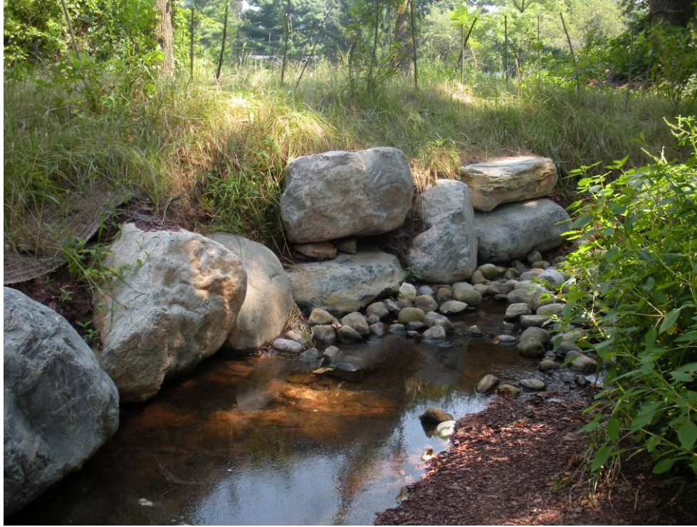
Figure 48: Boulder Toe Protection
